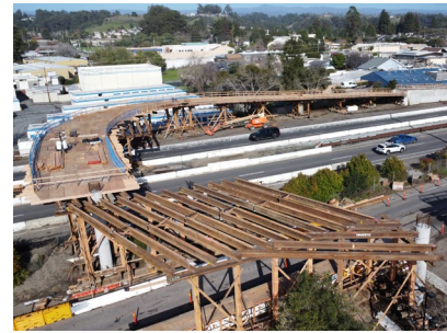
Construction of Bicycles and Pedestrian Overcrossing
