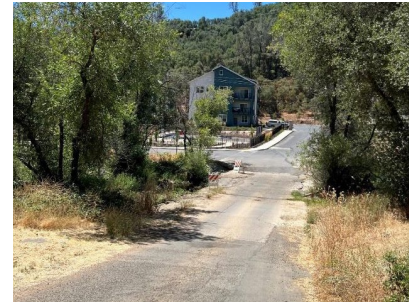
Fournier Road during normal conditions
