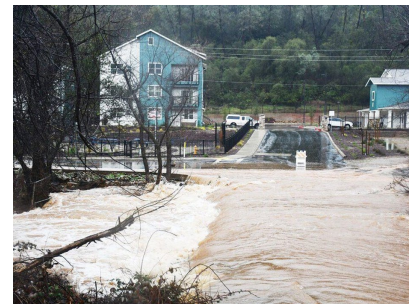
Fournier Road during flood conditions
