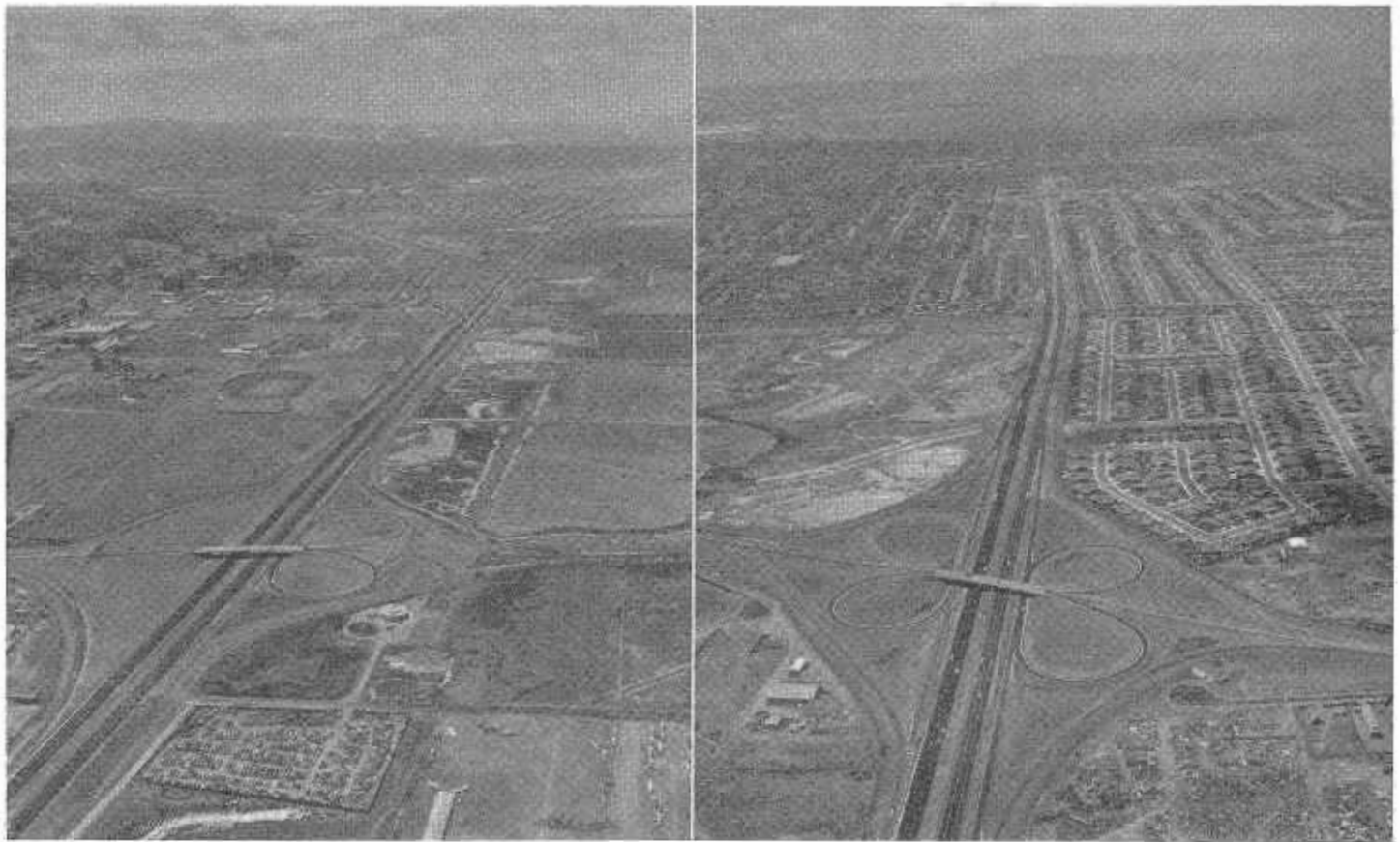
LEFT—View of recently completed five-mile section of Bayshore Freeway between San Mateo and San Carlos. Holly Street Interchange at San Carlos in foreground. RIGHT—View of recently completed section of Bayshore Freeway in San Mateo. Tenth Avenue Interchange in foreground.
