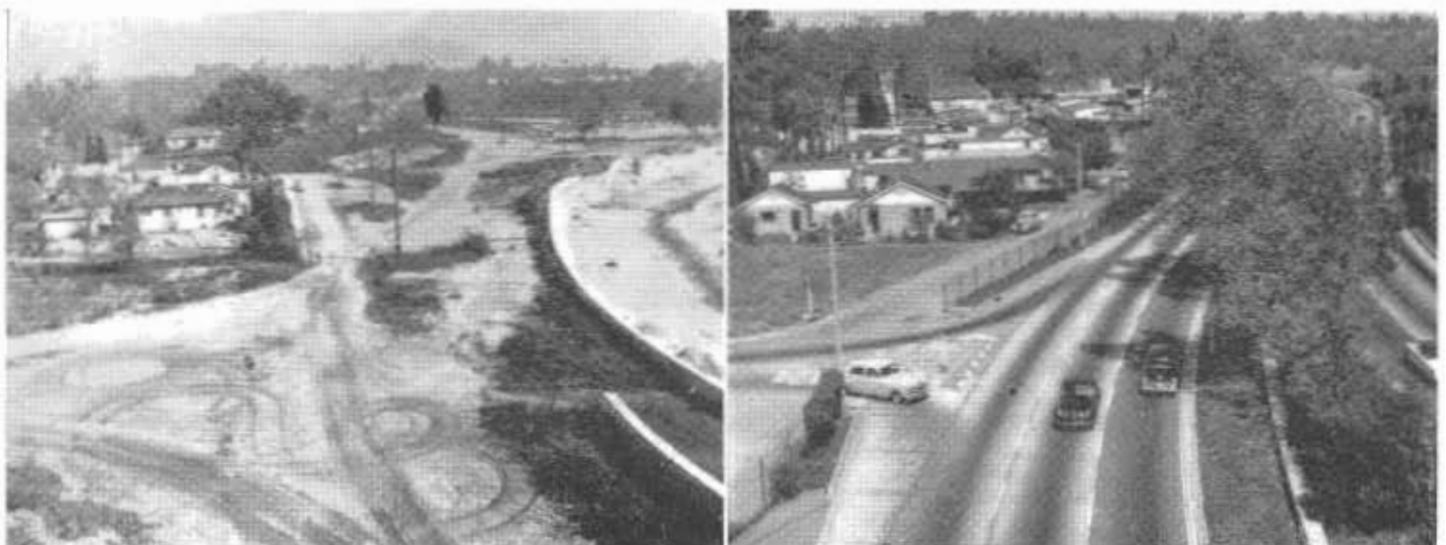
LEFT—Looking northeasterly along Arroyo Seco Freeway location toward City of South Pasadena in background. Photo taken in 1940. RIGHT—Photo taken at same location in May, 1955.
