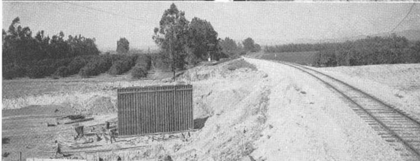
UPPER—View of Santa Ana River Bridge on Route 175 looking southerly from north end of bridge. LOWER—Shoofly for Santa Fe Railroad and start of bridge work at the Olive Undercrossing.
