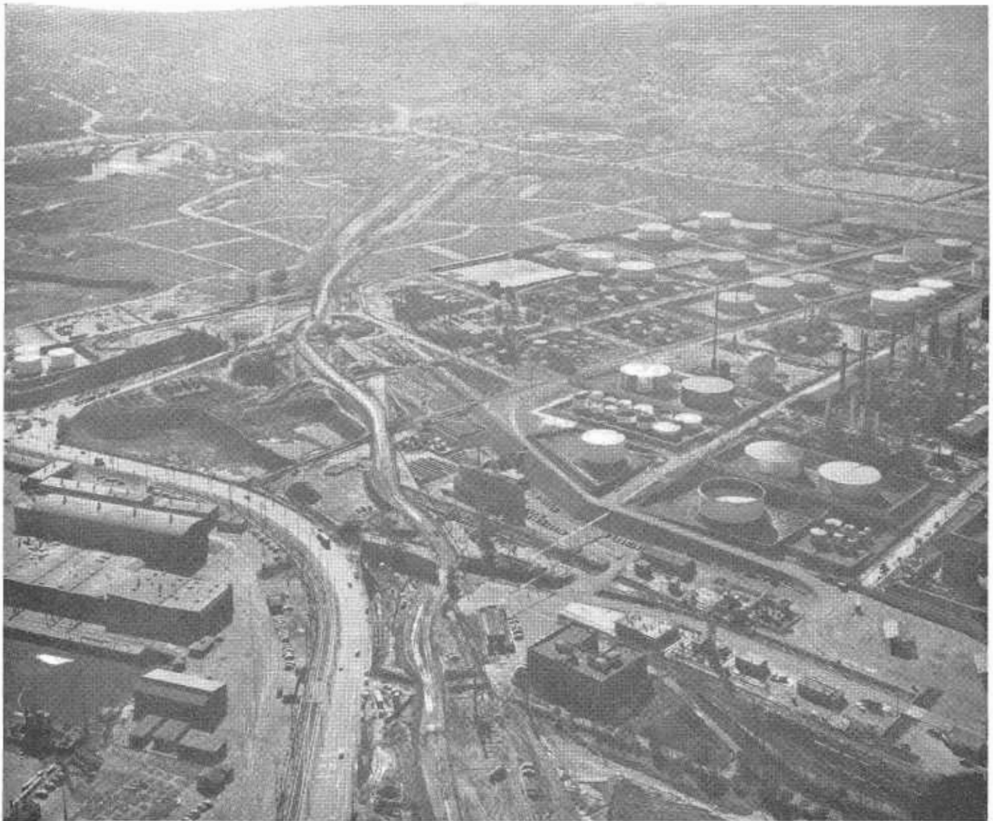
Aerial view looking southerly at excavation area and haul road through oil refinery. At left is Wilmington-San Pedro Road. Traffic artery shown in background is Gaffey Street extending into San Pedro.
