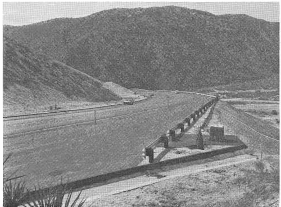
A safety rest area and drinking fountain along the freeway.
