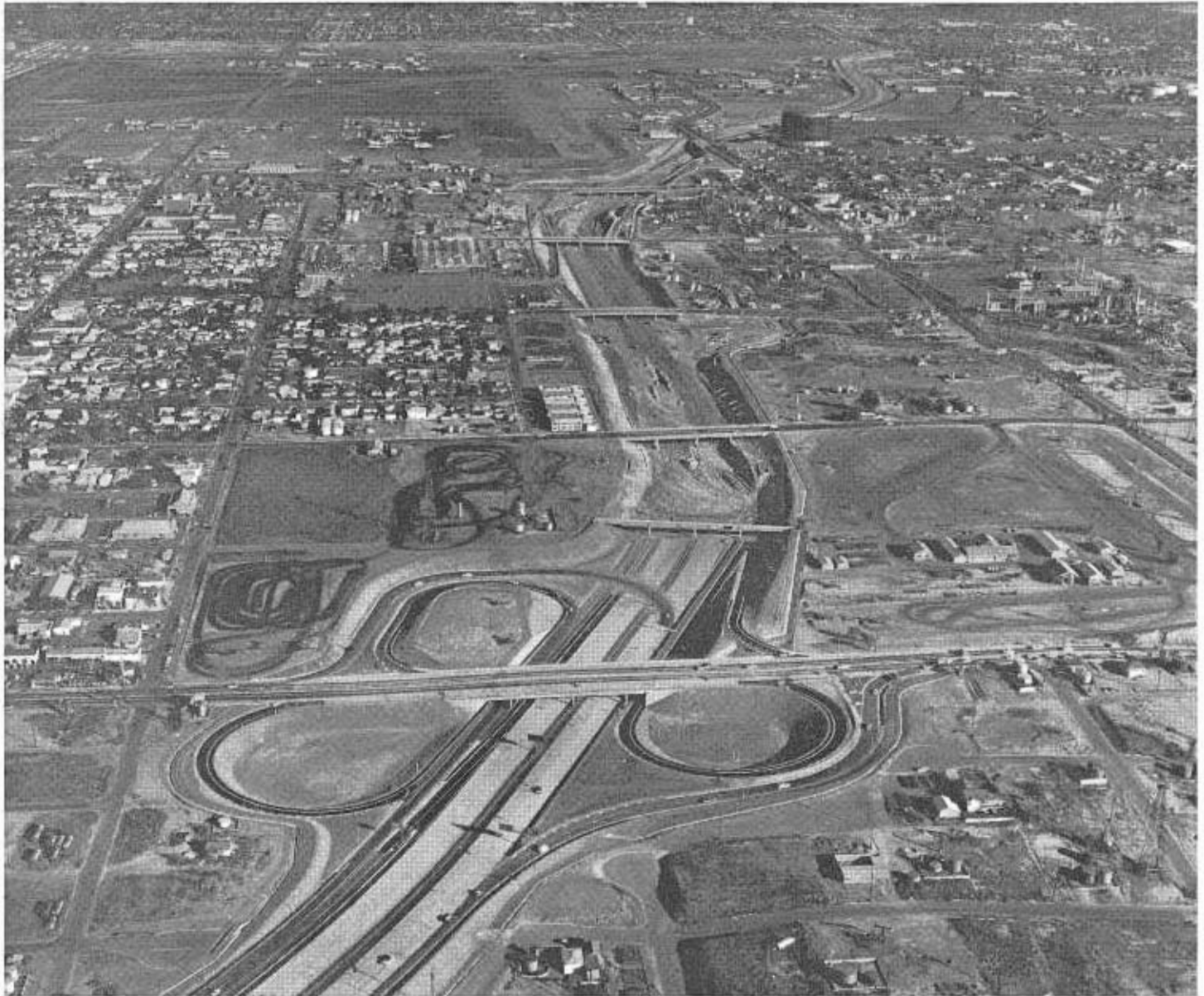
District VII's first freeway opening of 1964 was a 1.8-mile segment of the San Diego Freeway between the Long Beach Freeway and Atlantic Avenue in Long Beach, on January 15. From Atlantic Avenue (center of photo) the freeway is under construction to the Orange county line, a distance of 5.4 miles, with completion expected in the latter part of this year. Further construction is in progress across Orange County as far as Beach Boulevard in Westminster.
