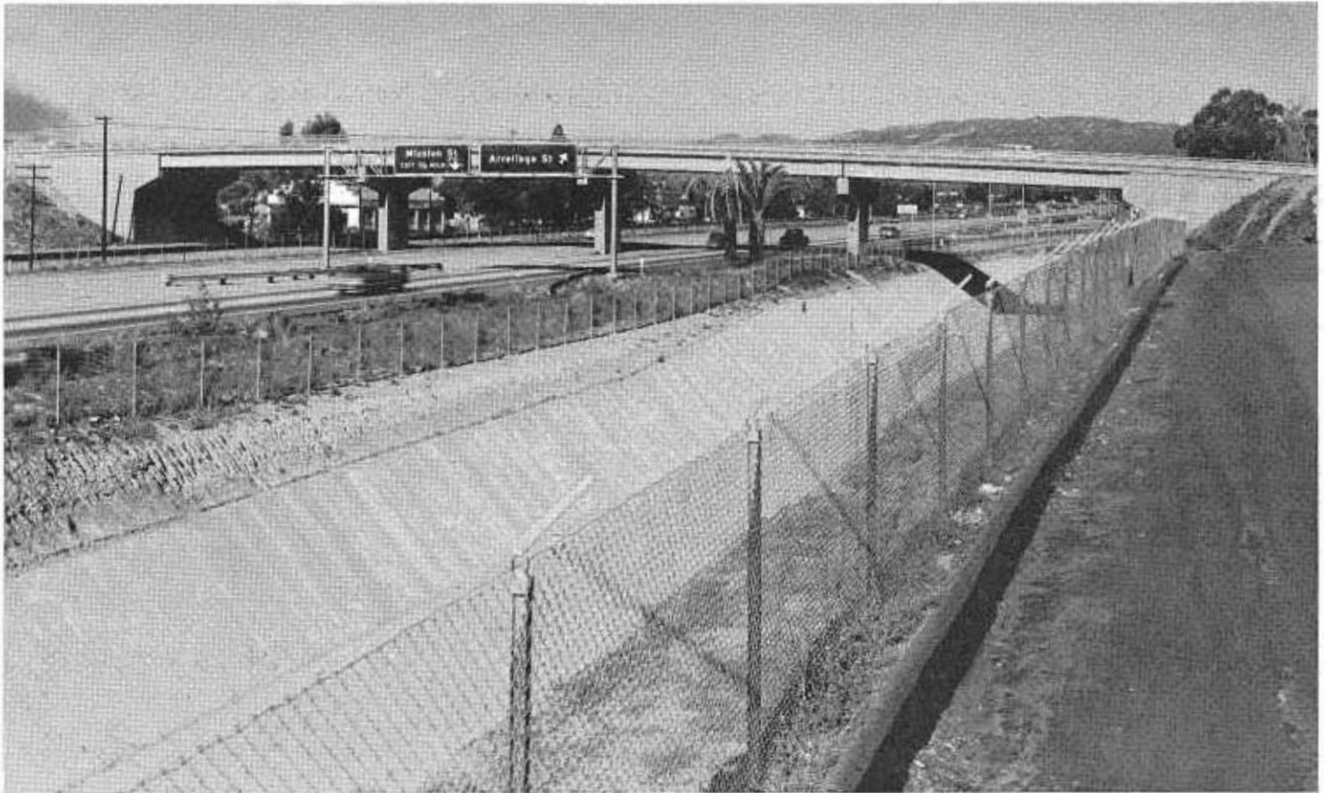
The Mission Creek channel change parallels the freeway to the right beginning left foreground. The Southern Pacific Railroad is on the other side of the freeway. The view is westward toward the Micheltorena Street overcrossing.
