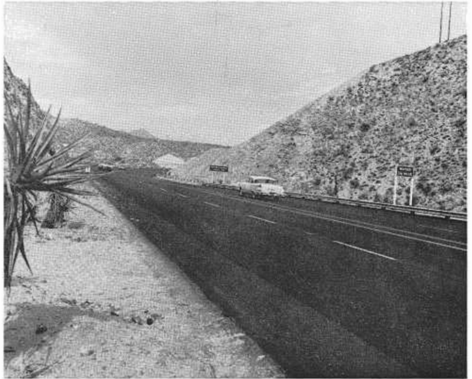
Approaching the safety rest area about halfway through the canyon.
