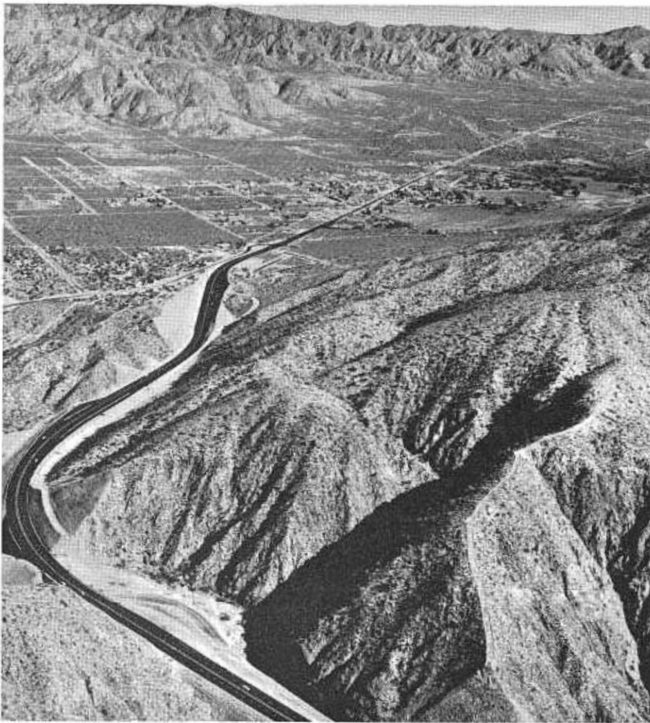
An aerial view northward across the community of Morongo Valley. The bridge can be seen left foreground and just beyond, the safety rest area and drinking fountain.
