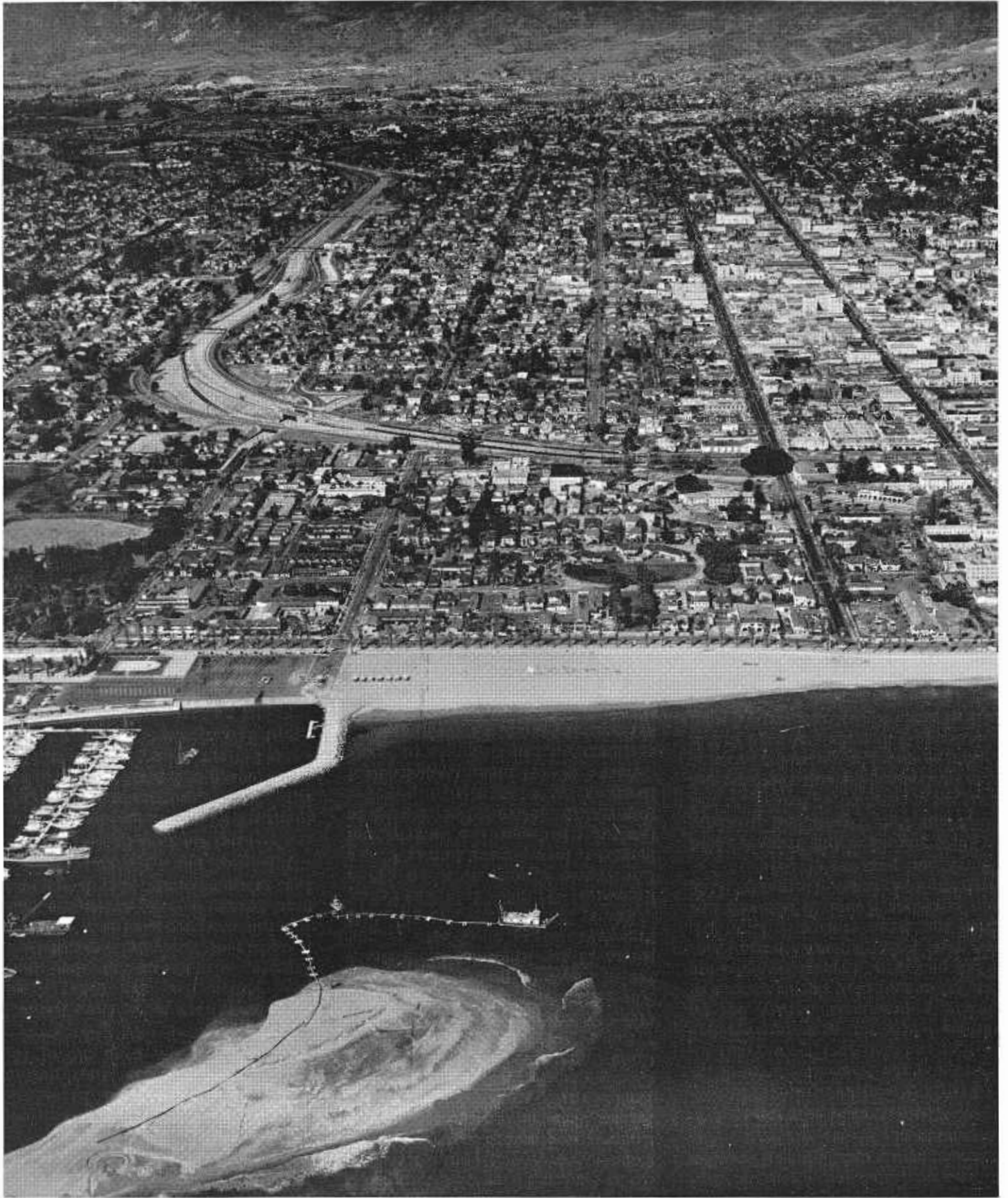
An aerial of the freeway area through Santa Barbara. The sand dredge is in the foreground with the Marina to the left. The Moreton Bay fig tree is right middle ground with the central business district beyond and to the right of the tree.
