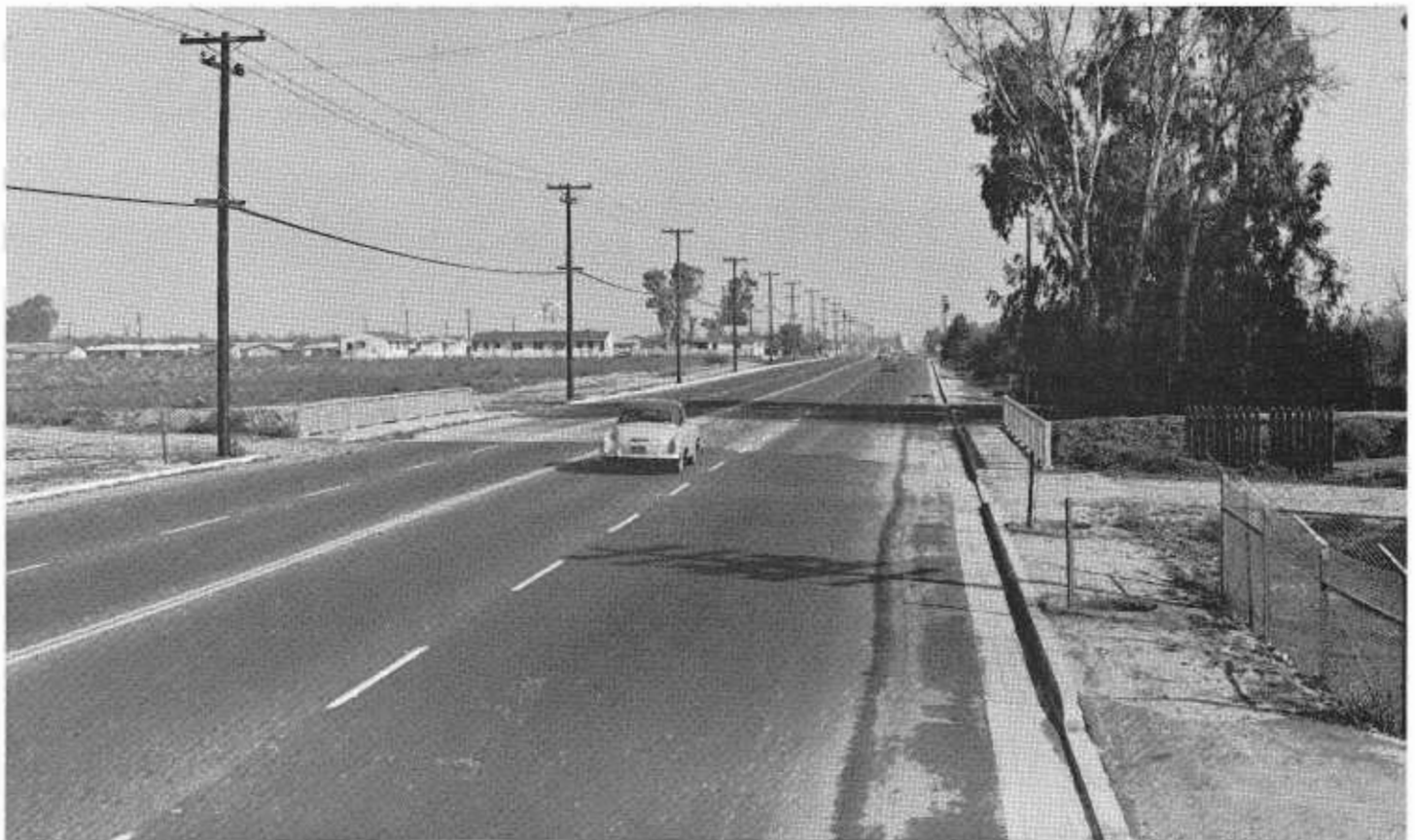
Looking east along the completed Bellevue Road improvement at the Livingston Canal crossing.
