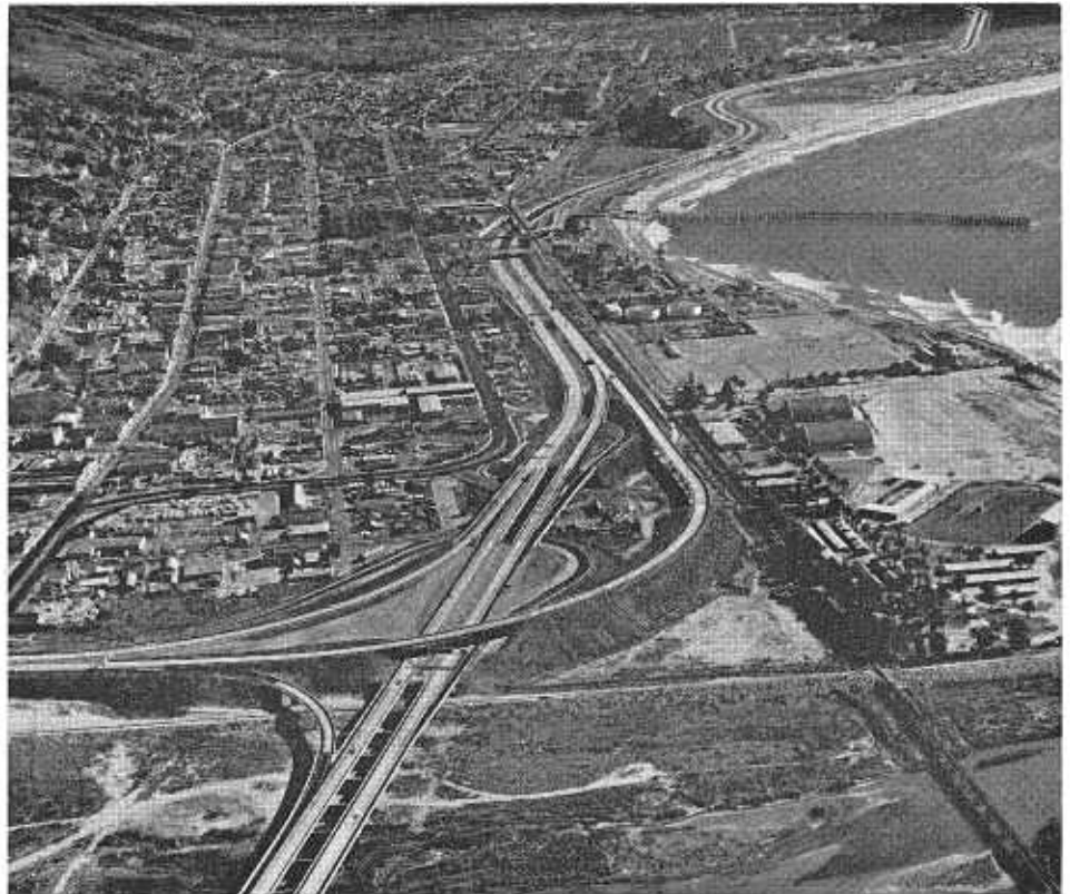
Completion of the Ventura Freeway through the City of Ventura last June relieved traffic congestion on city streets and gave motorists a scenic drive along the shore. This view is southeast along the new freeway, with the Ojai Freeway curving off to the left.
