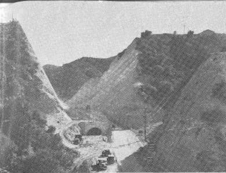
In 1938 a cut was made straight through the ridge and the troublesome old tunnel removed.
