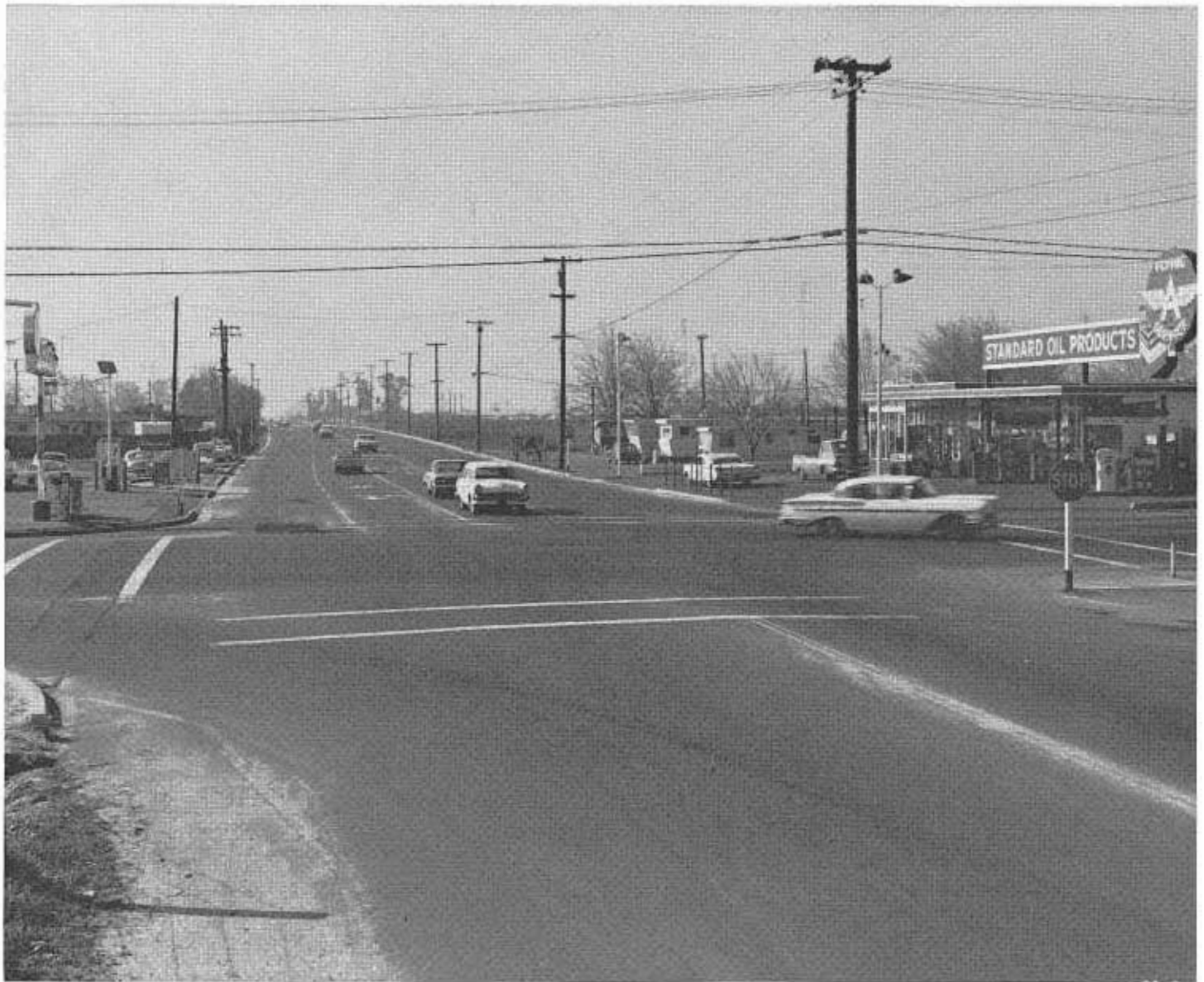
The east end of the project at the intersection with Buhach Road. The view is westward.
