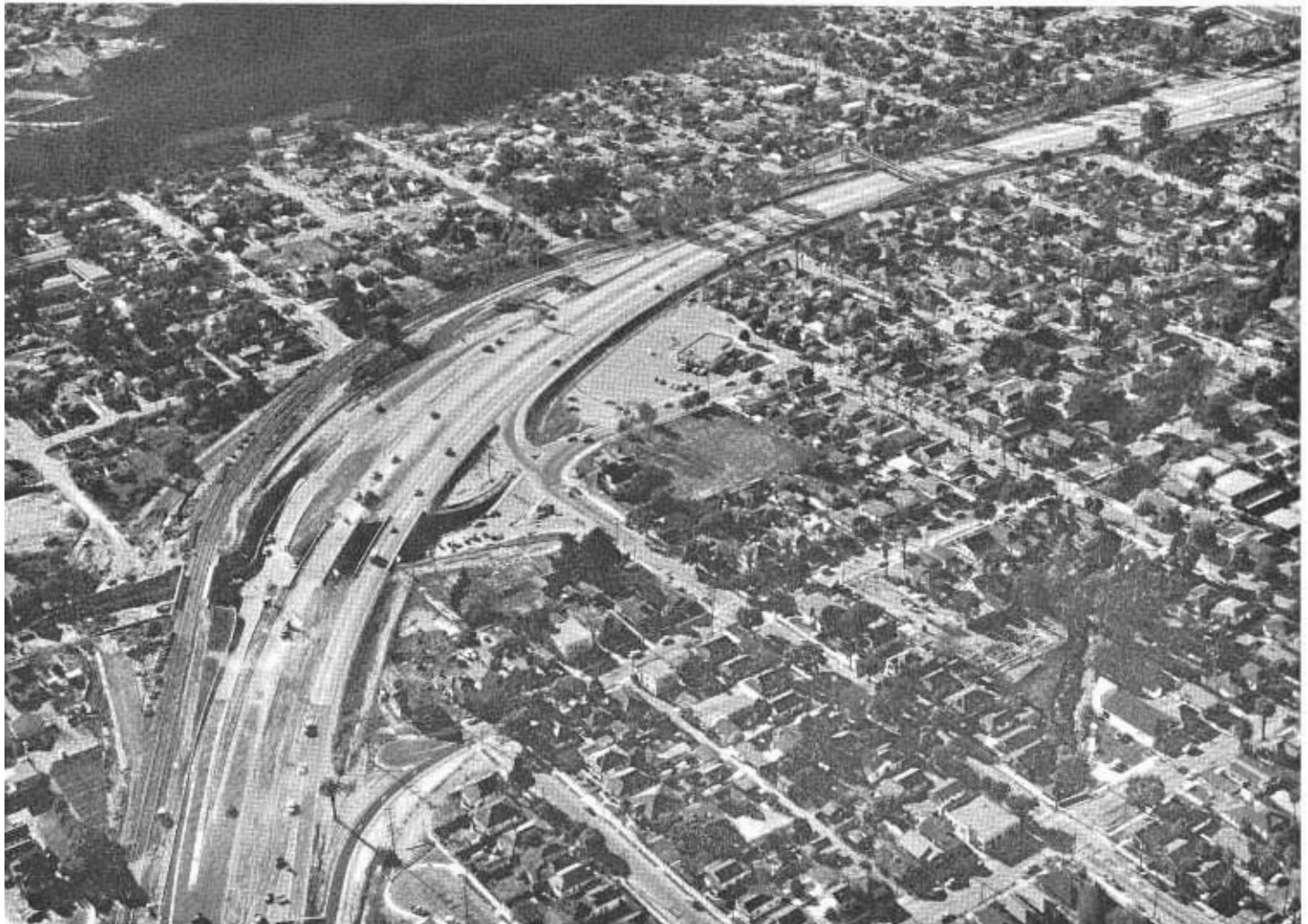
This aerial of the Castillo Street undercrossing (near completion) shows the routing of traffic to the northbound lanes while the southbound lane is being finished. It also shows some of the railroad relocation in the curve at the left.
