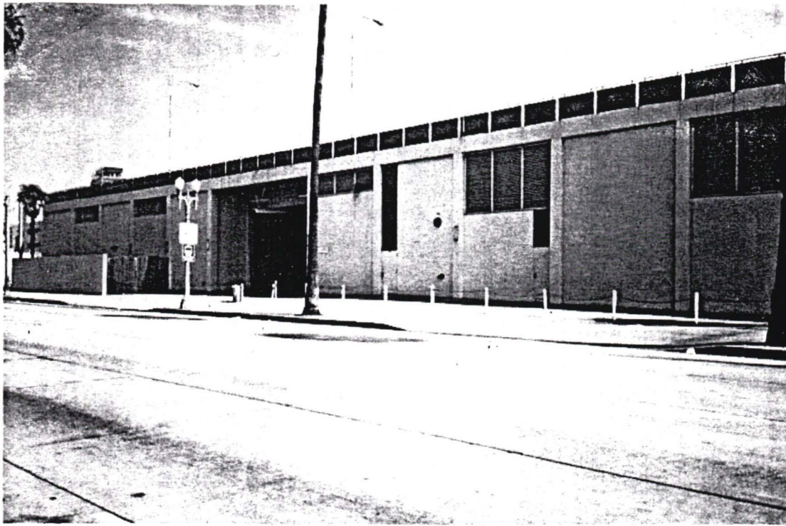
Photo 7: L.A. Trade Tech driveways on the east side of Flower Street south of Washington Boulevard. Light rail operations on the east side of Flower Street could require either closure of the driveways or the installation of warning devices.
