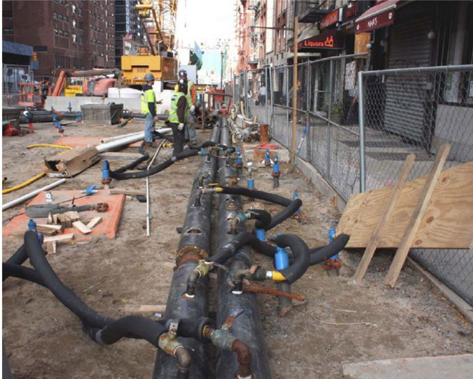
**Figure 4-12: Ground Freezing Operation**
