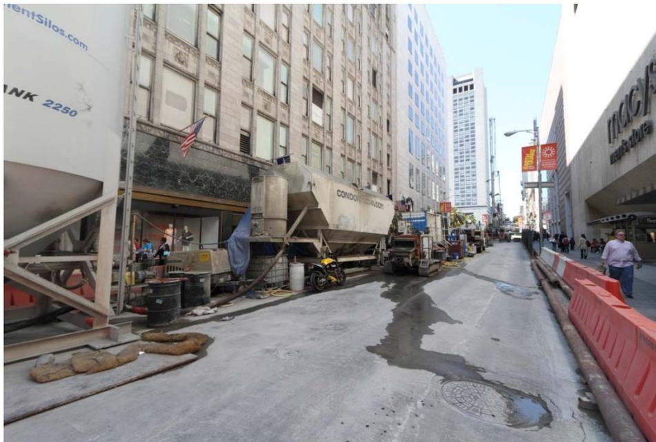
Figure 4-8: Surface Jet Grouting Operation
