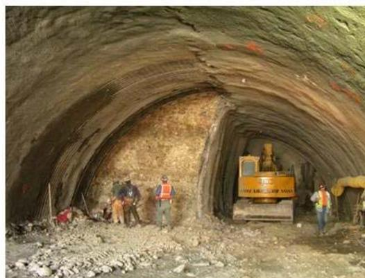
Small tunnel sections are excavated and temporarily supported in a specific sequence.
