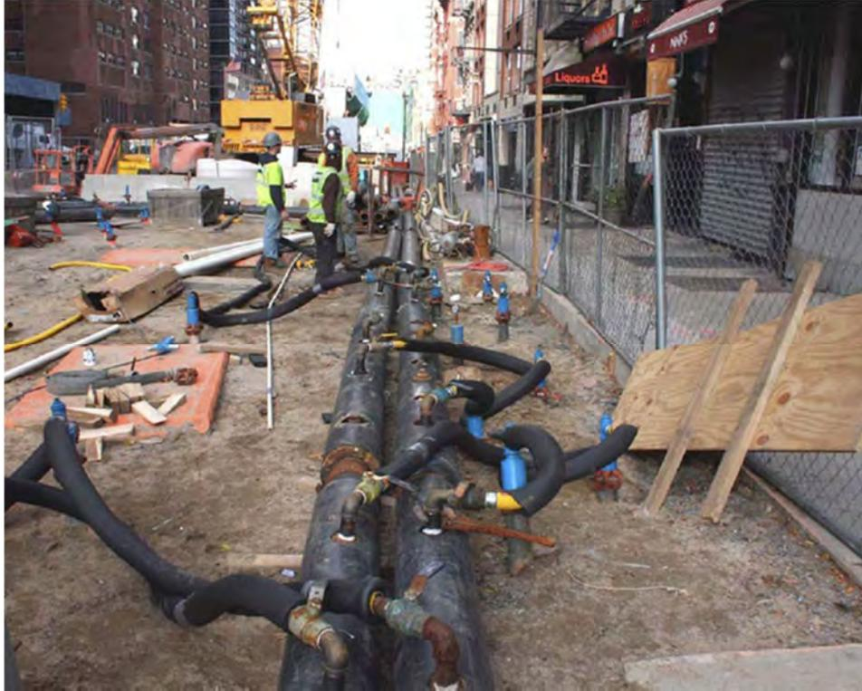
**Figure 4-12: Ground Freezing Operation**
