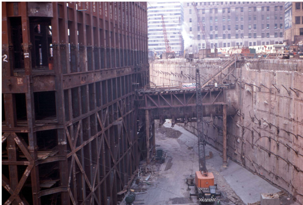
FIGURE 4-16. SLURRY WALL
