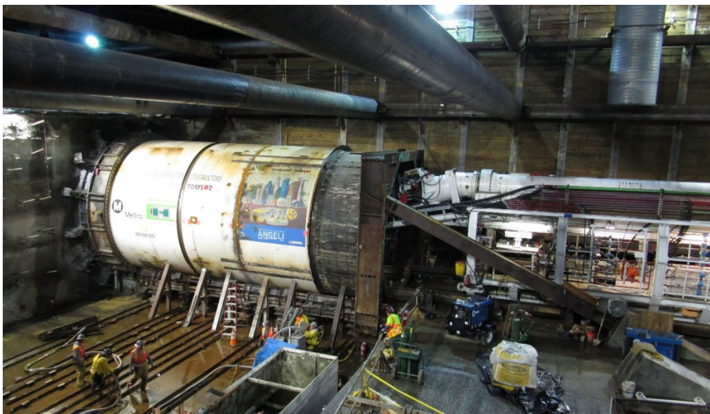
FIGURE 4-6. TBM LAUNCHING
