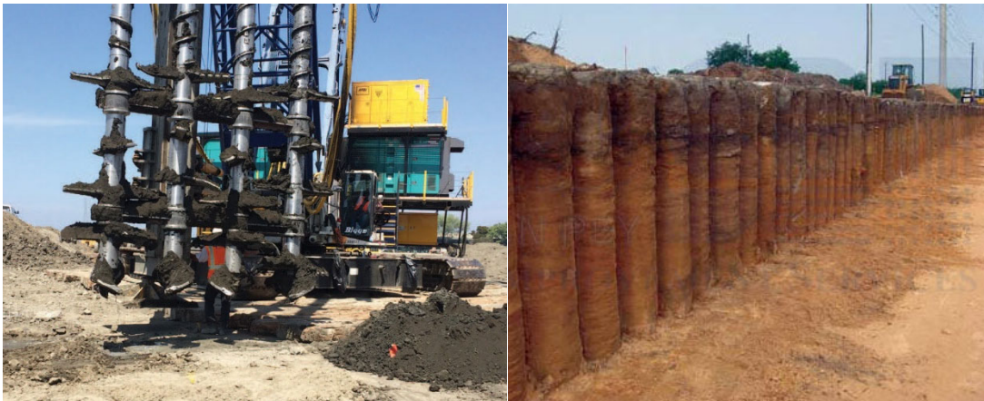
FIGURE 4-13. DEEP SOIL CEMENT MIXING WALL
