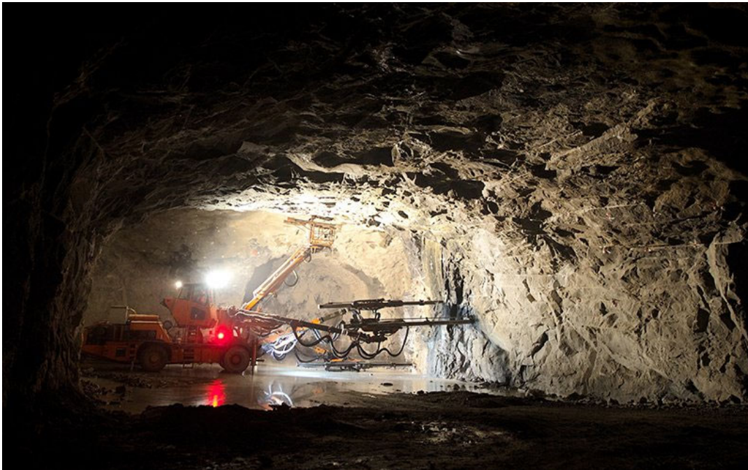
FIGURE 4-3. DRILL-AND-BLAST OPERATION
