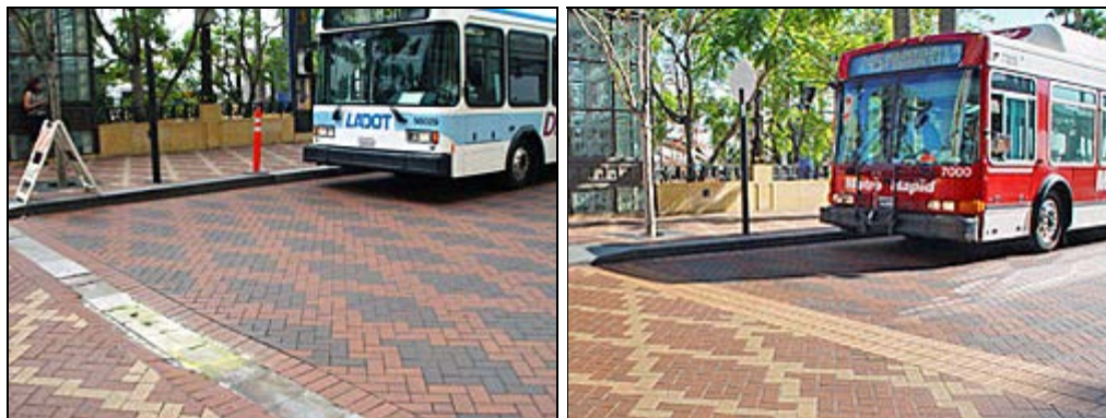
Before and after: Above, workmen replaced paver bricks from the deck of the south end of the roadway that had buckled under the weight of buses. Below, workers removed damaged granite and replaced it with colored brick to mark pedestrian walkways.
