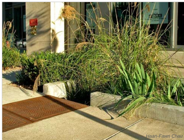
A curb cut that directs water from the street and sidewalk into a bioswale. 1100 S. Hope Street in downtown Los Angeles.
