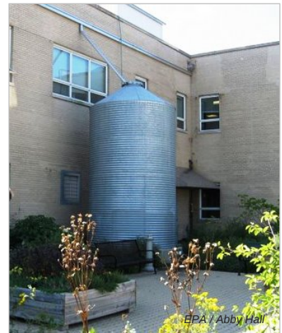
A large cistern collects roof runoff from a commercial building in Chicago.
