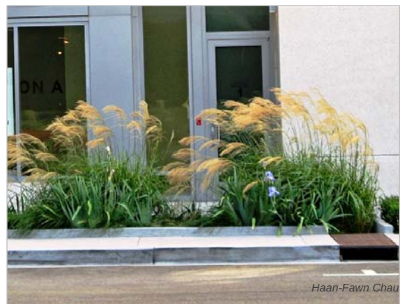
A curb cut and bioswale at 1100 S. Hope Street in downtown Los Angeles.
