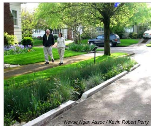
Curb bump-outs on NE Siskiyou Street in Portland, OR.
