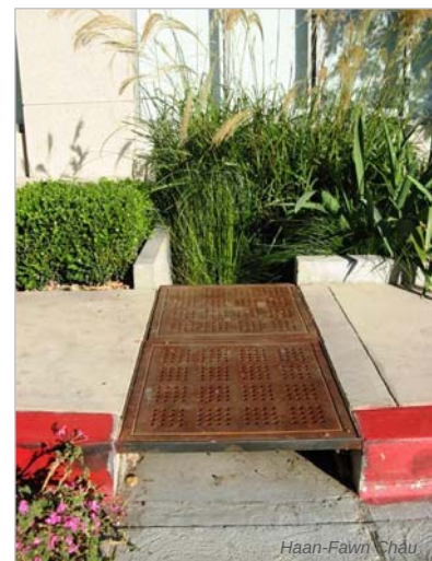
A curb cut that directs water from the street into a bioswale. 1100 S. Hope Street in downtown Los Angeles.
