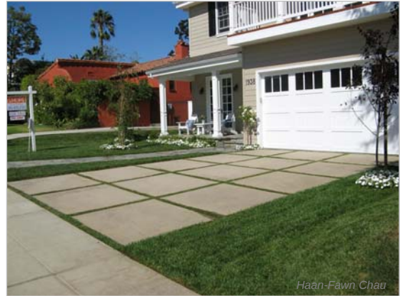
A driveway that allows for infiltration (Los Angeles)
