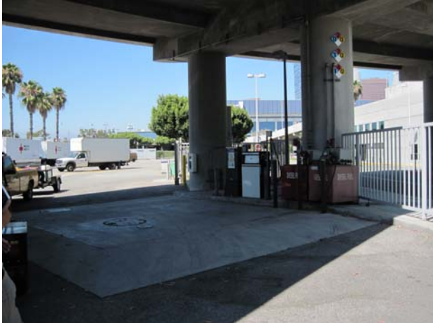
PHOTO M: View of the gasoline & diesel motor vehicle fueling area, located southwest of the South Hall
