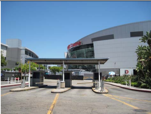
PHOTO C: Looking east toward the western face of the STAPLES Center
