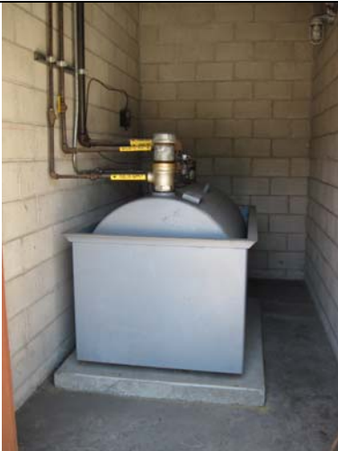
PHOTO I: View of the diesel AST in the West Hall
