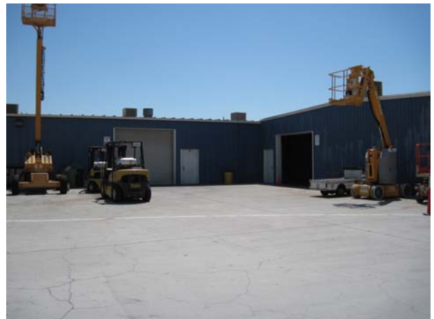
PHOTO J: View of LACC storage & paint shop area at the West Hall, near the southwestern corner
