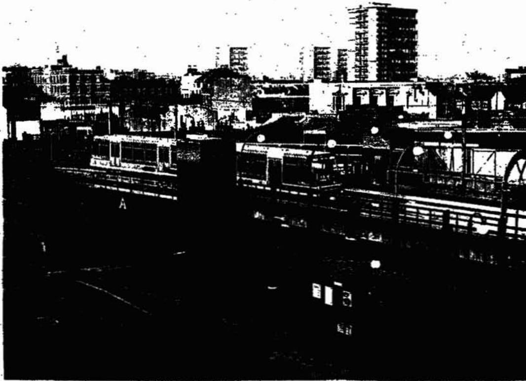
**Above: Limehouse Station. Line constructed on disused 1839 brick viaduct of the old London and Blackwell Railway.**
