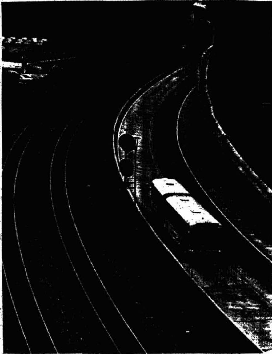
The busway alignment required relocation of the Conrail main line, seen at left. The busway itself has two lanes and a single shoulder in this segment.
