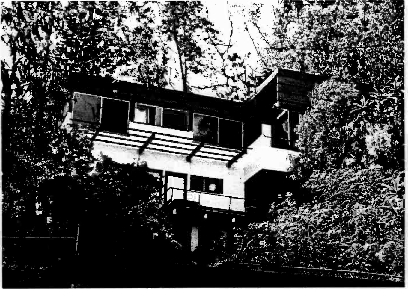
John De Keyser Duplex 1911 North Highland Avenue
