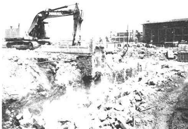
DEMOLITION OF EXISTING LAUPT UTILITY TUNNEL AND PASSENGER TUNNEL RAMP
