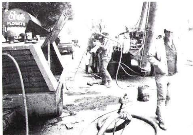
COMPACTION GROUTING OPERATIONS ON 7TH STREET. DRILL IS BEING USED TO REAM OUT GROUT HOLES, TRUCK IS THE PORTABLE BATCH PLANT FOR COMPACTION GROUT
