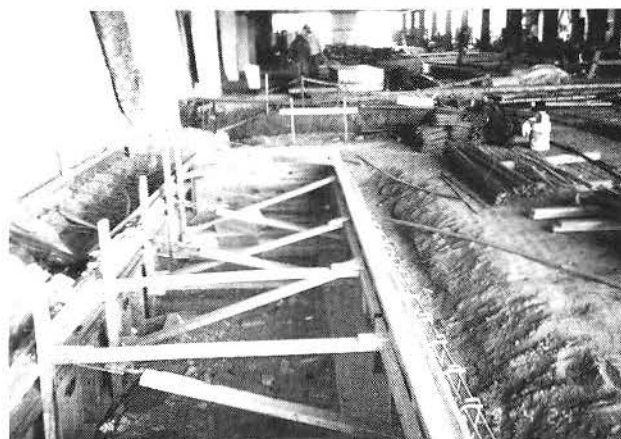
WHEEL PRESS MACHINE PIT BOTTOM SLAB AND WALL FORMS
