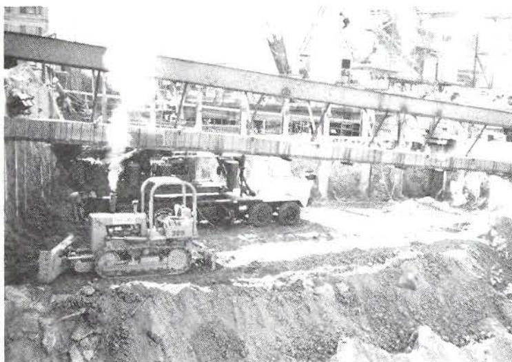
TELEPHONE DUCTBANK SUPPORT IS SHOWN ABOVE THE CURRENT EXCAVATION AND EXCAVATION SUPPORT BEING PERFORMED AT THE A171/A175 INTERFACE
