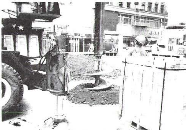
PHASE II PILE DRILLING OPERATIONS IN YARD I, THE STATION'S SOUTH ENTRANCE
