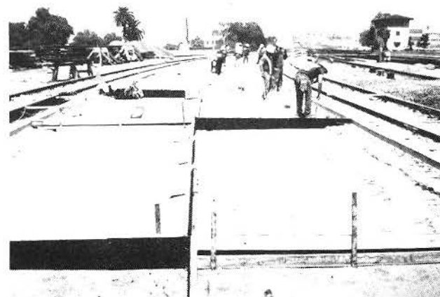
CONSTRUCTION OF FORMS FOR PLATFORM #3 EXTENSION
