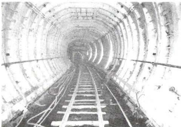
ARCH FORMS IN PLACE AL TUNNEL
