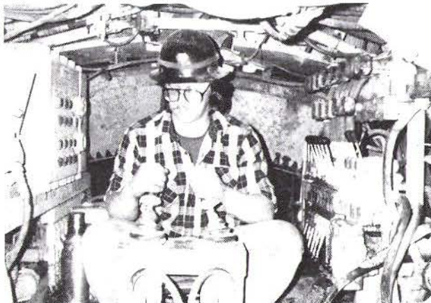
OPERATOR AT TUNNELING MACHINE CONTROLS
