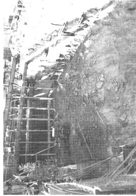
EXCAVATION AND SUPPORT OF EXCAVATION AT A171/A175 INTERFACE
