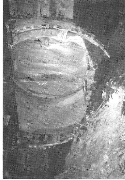
CONCRETE BULKHEAD AT A165/A171 INTERFACE HAS BEEN REMOVED. A171 AL TUNNEL LINING HAS BEEN PLACED
