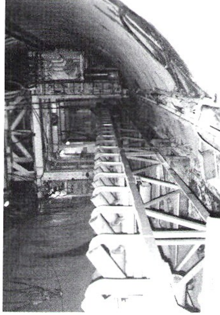
TEMPORARY MUCK REMOVAL CONVEYOR INSTALLED IN AR TAIL TUNNEL
