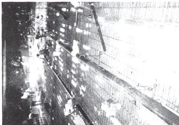
OVERVIEW OF THE REBAR PLACEMENT ACTIVITIES IN THE STATION'S SOUTHERN END (INVERTS 12 THRU 16)
