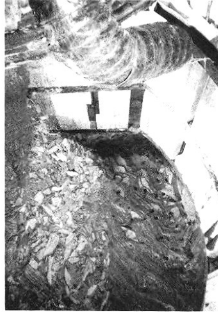
EXCAVATING CROSS PASSAGE AT STATION 139+63 FROM AR TUNNEL
