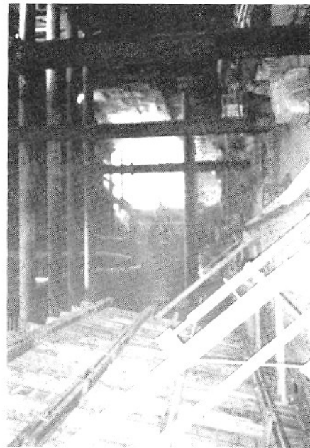
RED LINE STATION, 7TH ST. - LOOKING WEST
