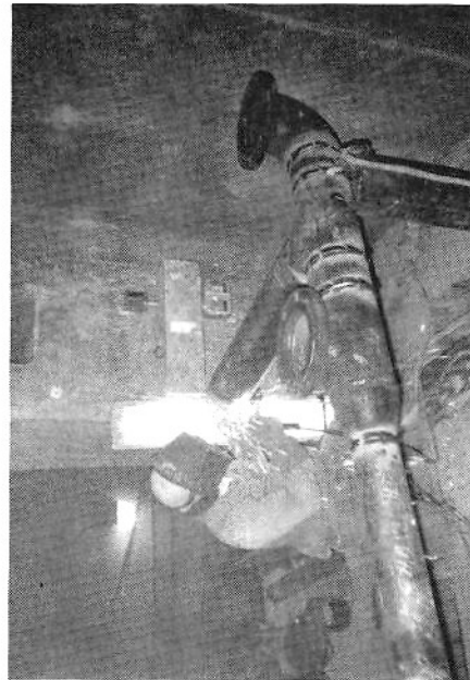
FABRICATION/INSTALLATION OF SUMP DISCHARGE PIPING
