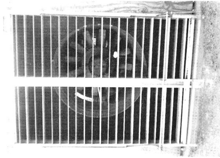
SUBWAY VENT FAN & DAMPER BEING TESTED FOR TRANSIENT PRESSURE CHARACTERISTICS
