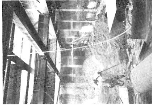
STATION'S INVERT 15/14 - ALSO VISIBLE ARE THE COLUMNS AND EXTERIOR/INTERIOR WALLS AND THE SCAFFOLDING FOR MEZZANINE SLAB AREA 14
