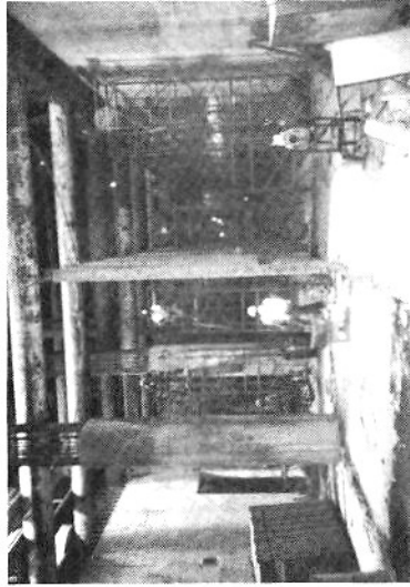
STATION'S INVERT 15/14 - ALSO VISIBLE ARE THE COLUMNS AND EXTERIOR/INTERIOR WALLS AND THE SCAFFOLDING FOR MEZZANINE SLAB AREA 14
