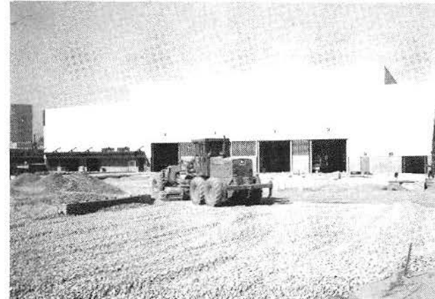
SPREADING BALLAST SOUTH OF MAIN SHOP BUILDING
