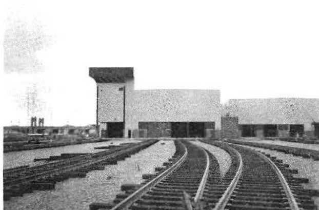
SERVICE AND INSPECTION TRACKS TIE-IN TO A112 MAIN SHOP BUILDING (NORTH SIDE OF MAIN SHOP BUILDING)
