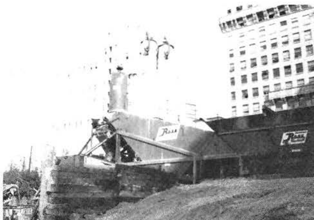
CONCRETE BATCH PLANT AT SITE
