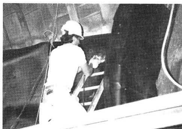
WORKMAN INSTALLING HDPE IN CROSS PASSAGE #9
