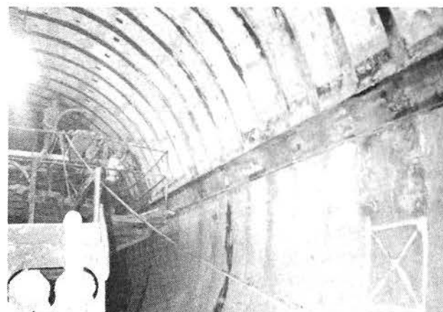
PREPARING AIR TAIL TUNNEL FOR HDPE INSTALLATION
