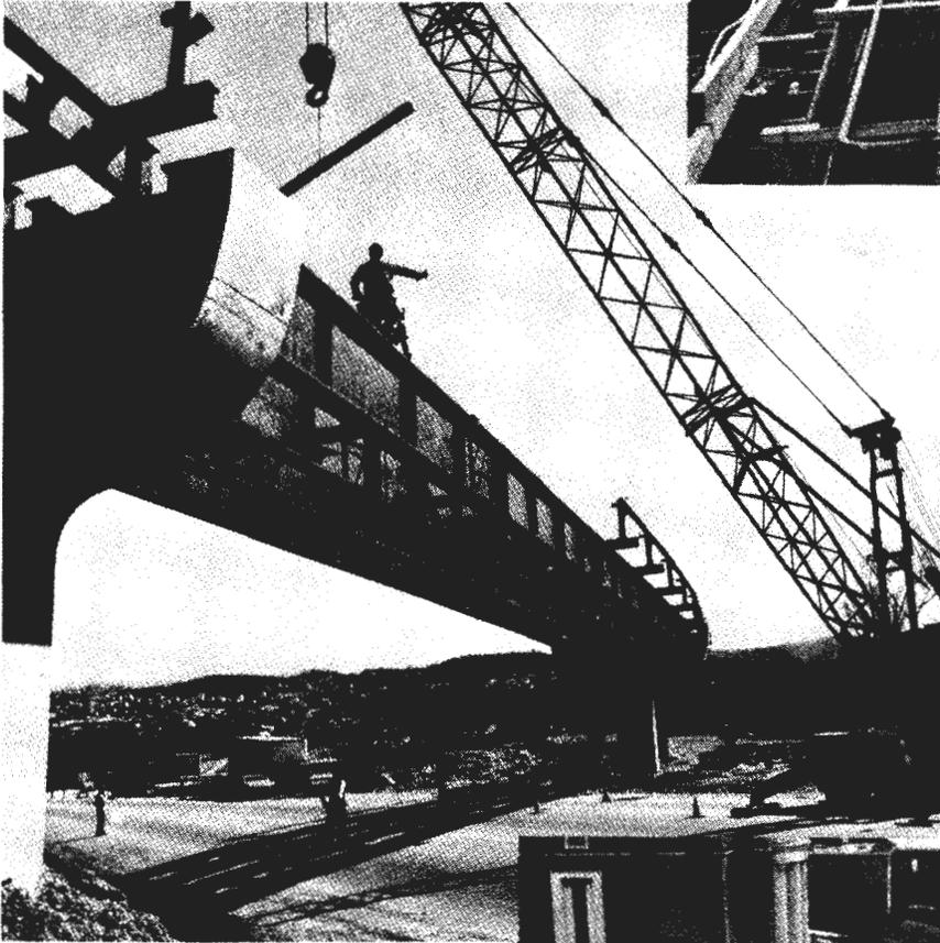
(b) GUIDEWAY BEAMS AND CAST IN PLACE CONCRETE SUPPORTS
