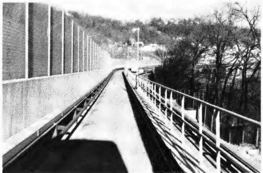
FIGURE 3.32 : STEPPED DESIGN OF AT-GRADE GUIDEWAY
