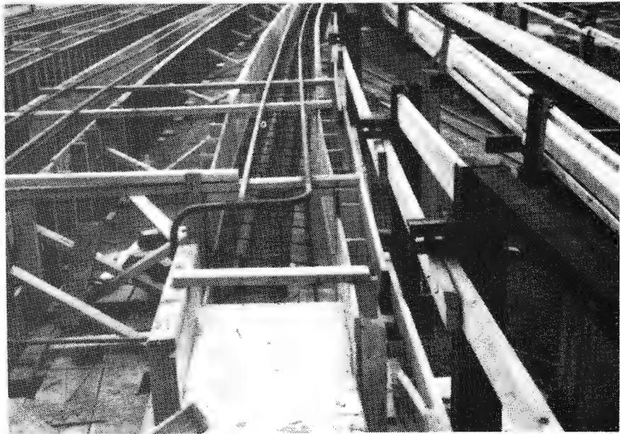
FIGURE 3.45: GUIDEWAY HEATING PIPES EMBEDDED ONLY IN RUNNING PADS OF ELEVATED GUIDEWAY
