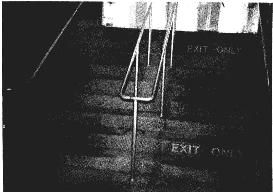
(b) EFFECTIVE STAIRWAY WIDTH REDUCED BY DOUBLE HANDRAIL
