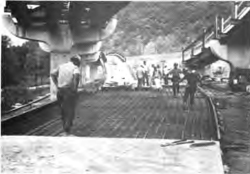
FIGURE 3.44: GUIDEWAY HEATING PIPES EMBEDDED IN THE SURFACE OF AT-GRADE GUIDEWAY
