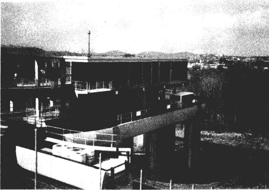
FIGURE 4.15 : CENTER ISLAND PLATFORM STATIONS REQUIRE VERTICAL ACCESS
