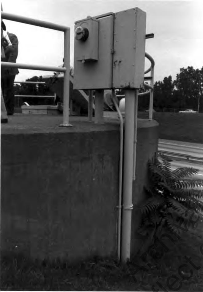
Underground service to externally-mounted meter with shunt-trip to main circuit breaker
