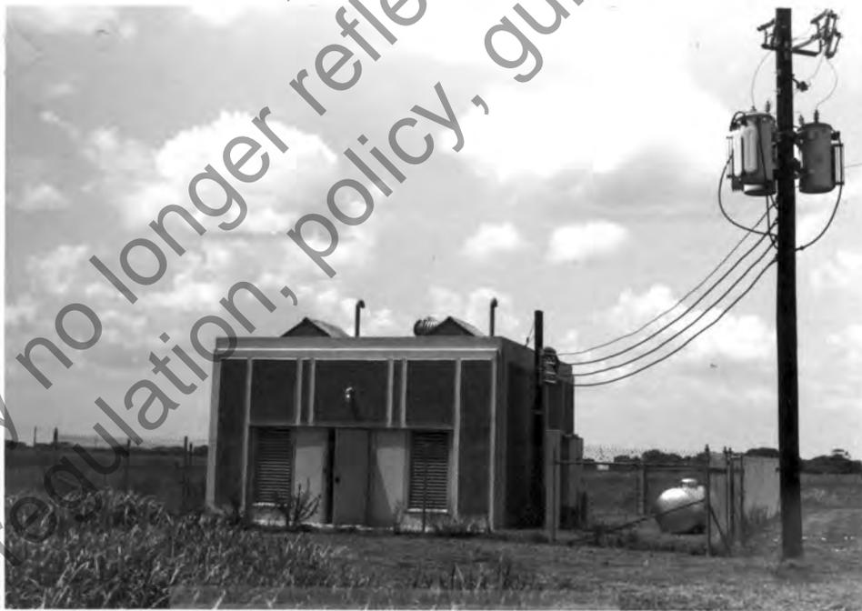
FIGURE 2-15. SMALL WET-PIT PUMP STATION, US 59, TEXAS
