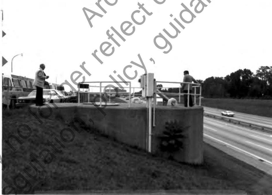
FIGURE 2-8. WET-PIT PUMP STATION, CAISSON TYPE,
