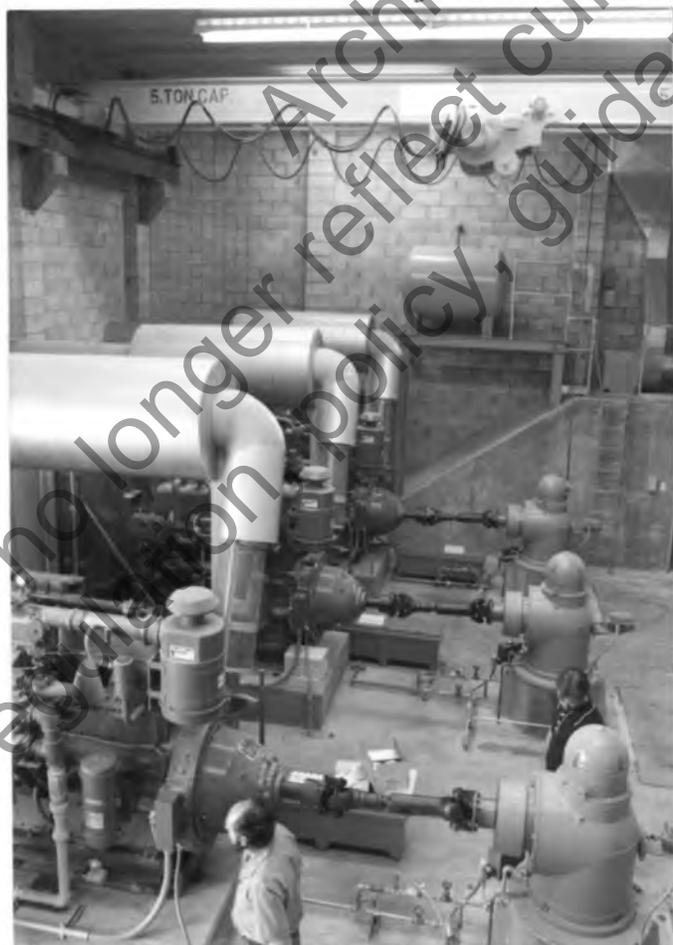
View from office showing engines. Light-angle gears and overhead crane as construction neared completion.
