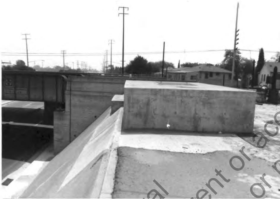
FIGURE 3-1. DRY-PIT PUMP STATION AT RAILROAD UNDERPASS
