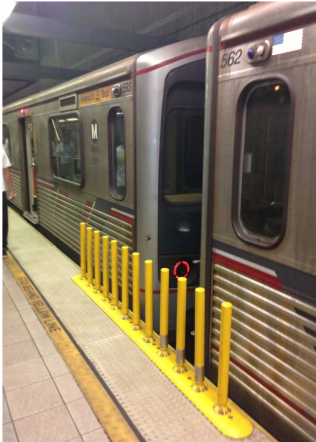
Between Car Barriers & Tactile Warning Strip
