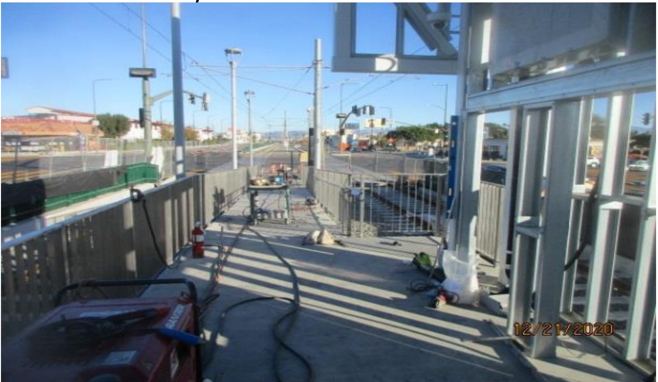
PARK MESA – Continue guardrail installation at the north entrance ramp.
