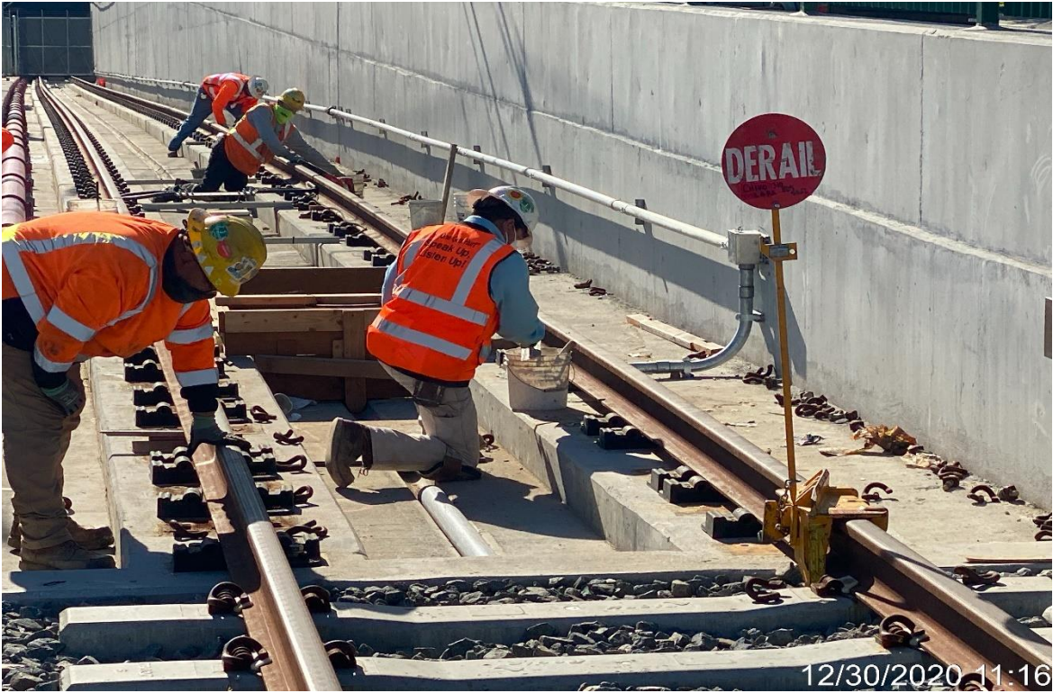
UG3 – WSCC resurfacing and patching plinths at UG-3 SB.
