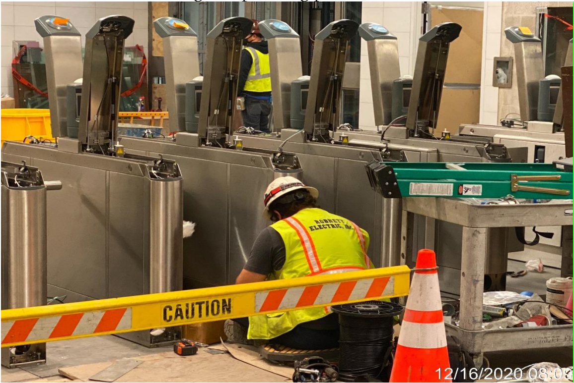
UG3 – Robnet preparing to install turnstiles at Vernon.
