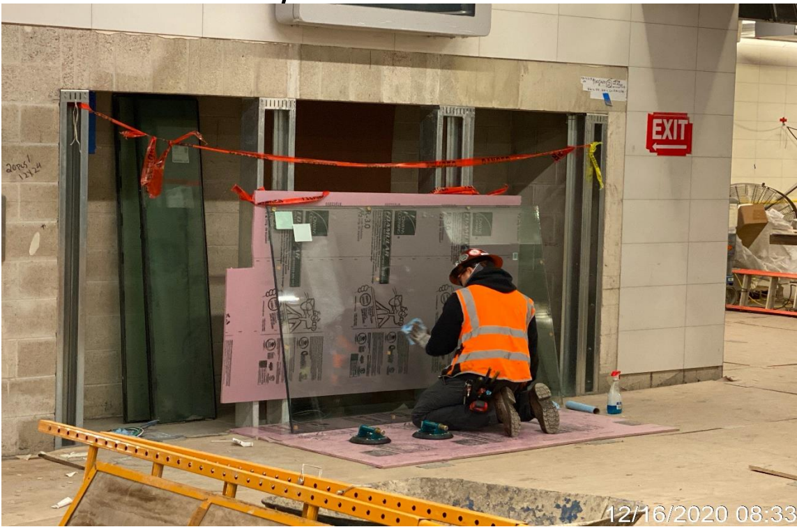
UG3 – Giroux installing glass in elevators 3 and 4 at Vernon.
