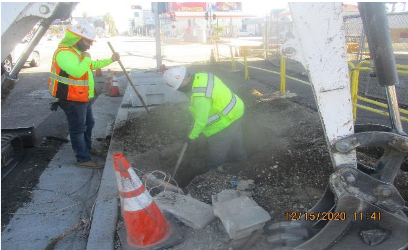
AVIATION/CENTURY - DB Excavating conduit trench at Century and Aviation.
