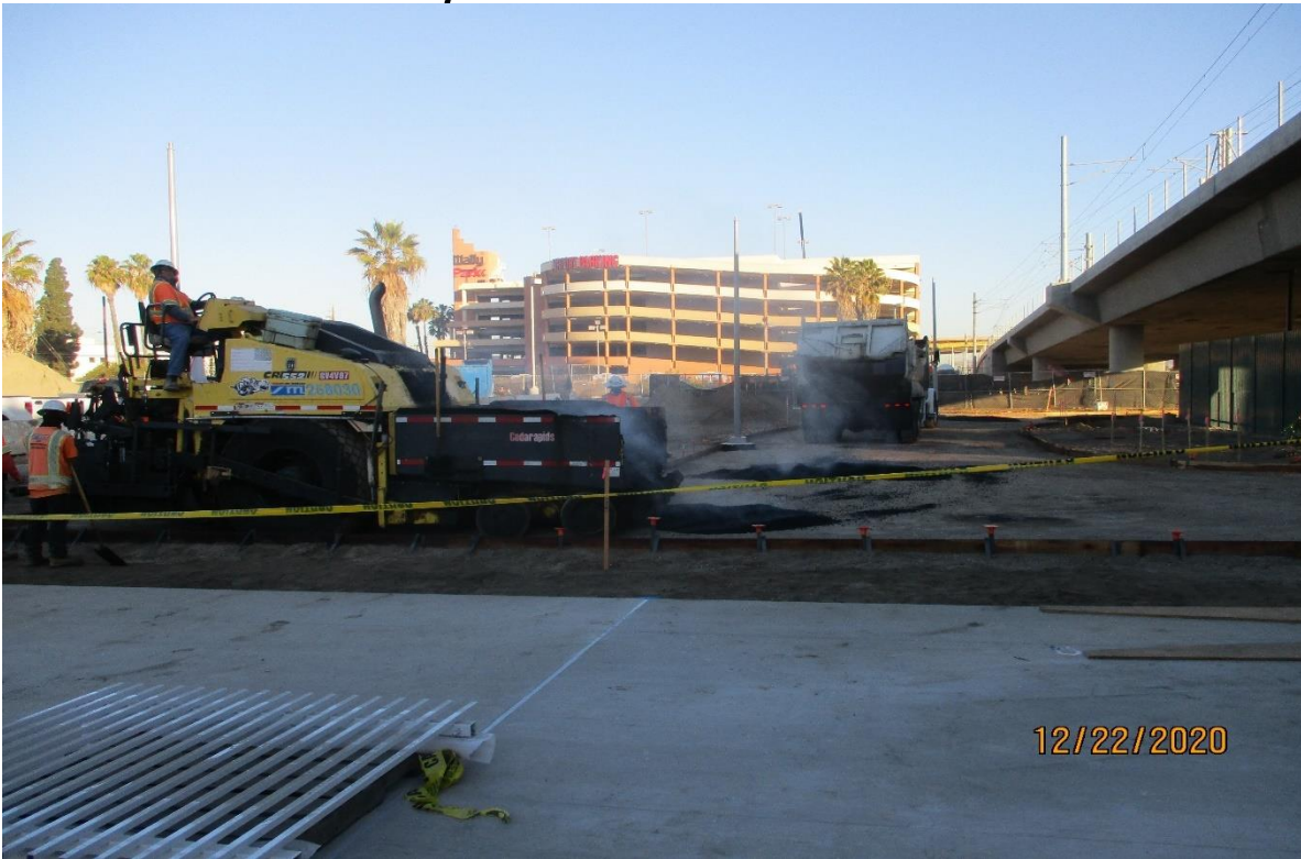
AVIATION/CENTURY- AC placement for the Aviation Station service driveway.
