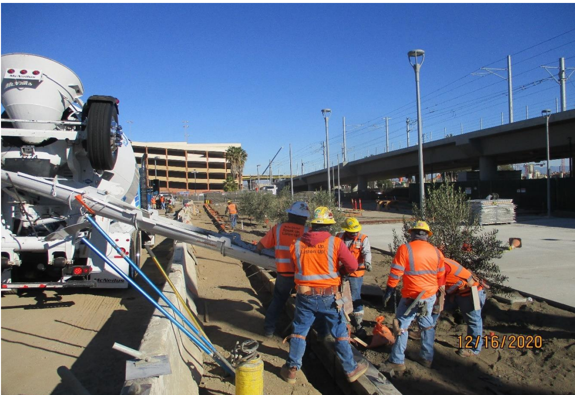
AVIATION/CENTURY- Placing concrete for the Aviation Station plaza mow strip
