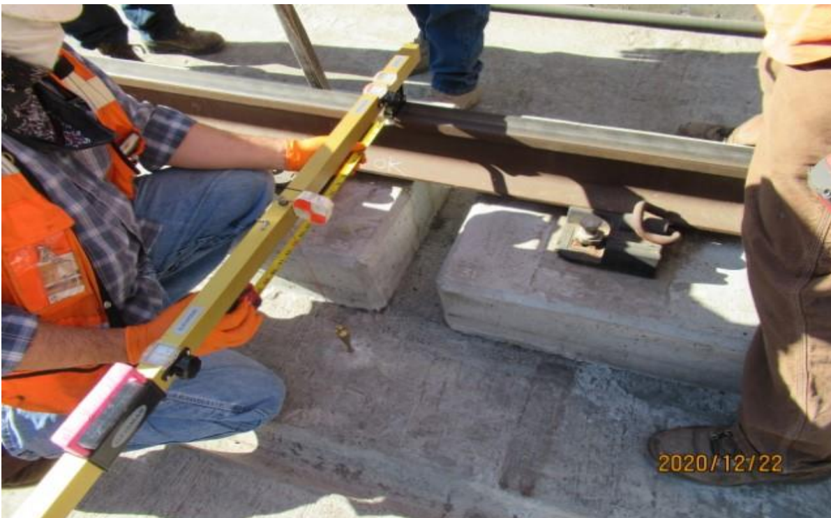
UG4 – HCC using plum bob for SB track at UG4 alignment on open issues log 000253 log status update to reflect “closed” Rework
