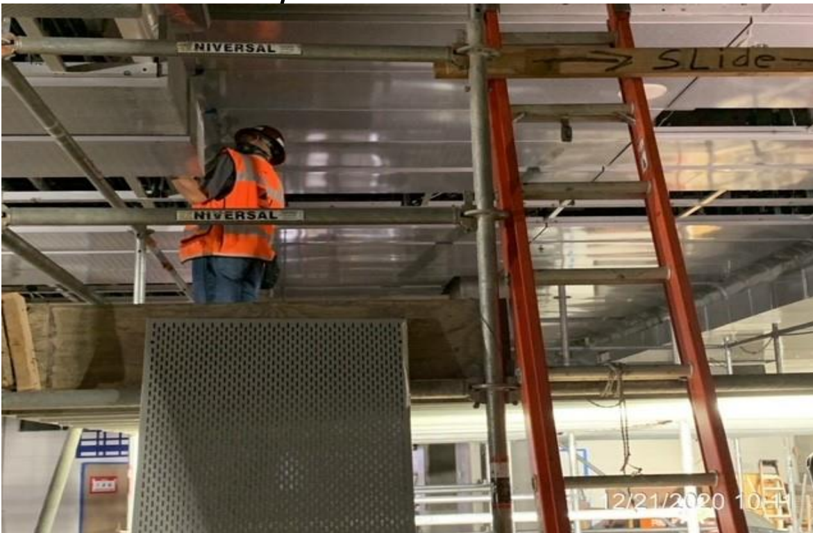
EXPO STATION – PCI installing radius and ceiling panels in paid area
