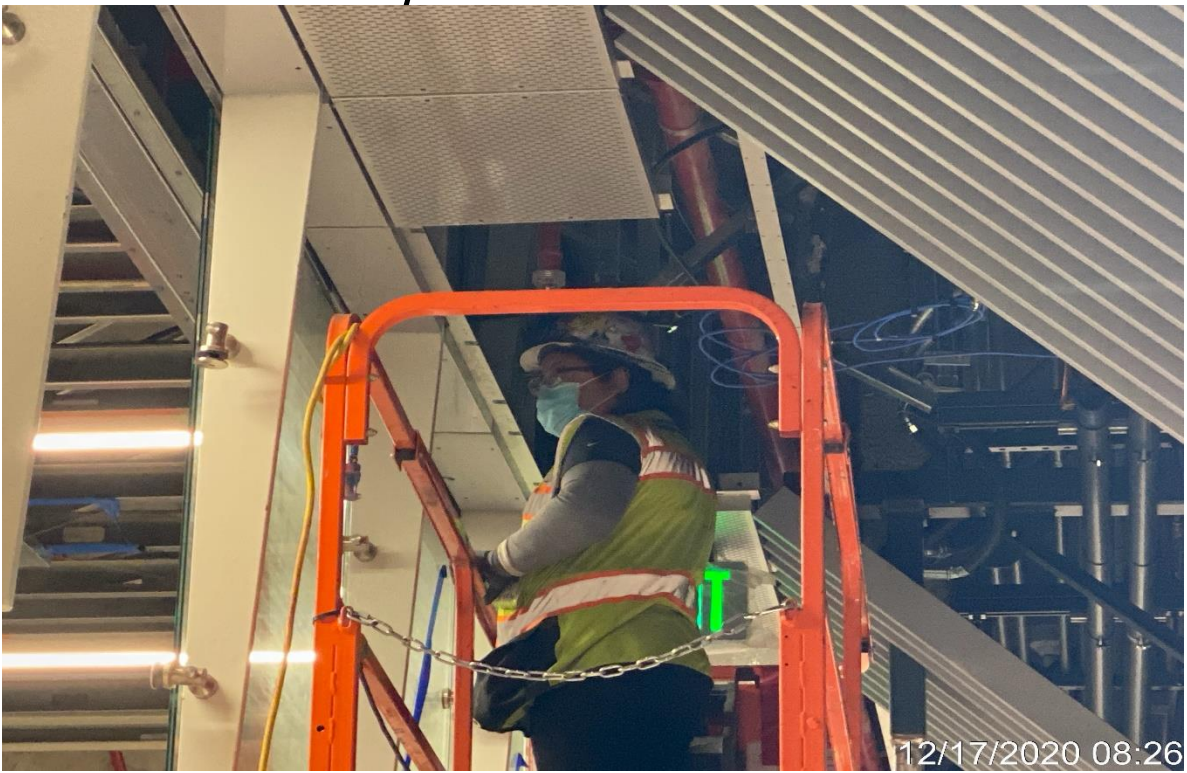
UG3 – Penhall scanning ceiling at Vernon for seismic bracing.
