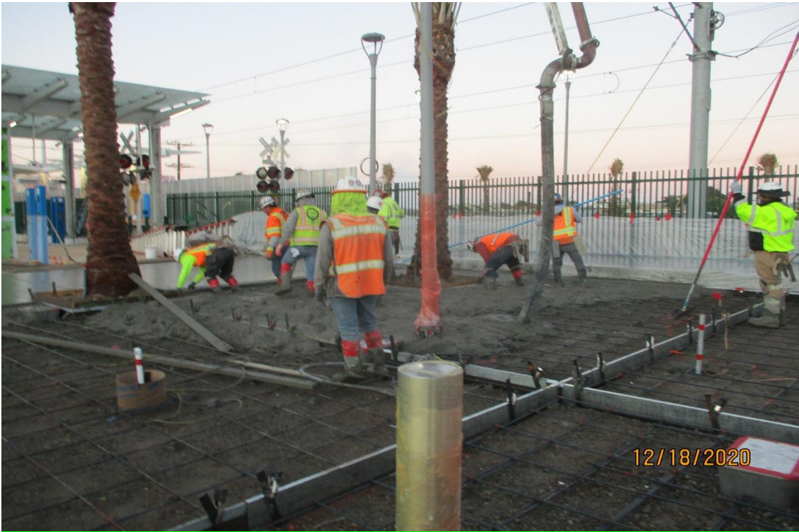
La Brea Station - Placing concrete for the La Brea Station hardscape.
