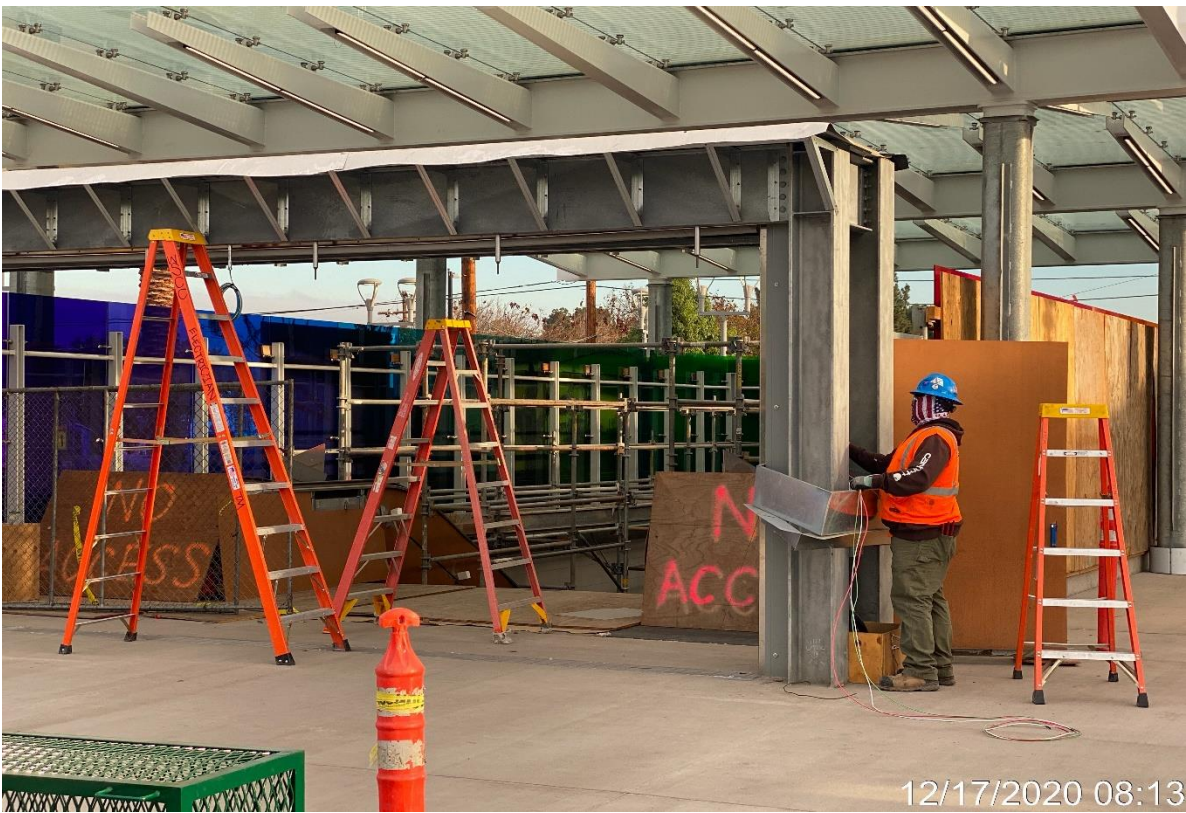
UG3 – WSCC electricians working on roll-up gate at Vernon.
