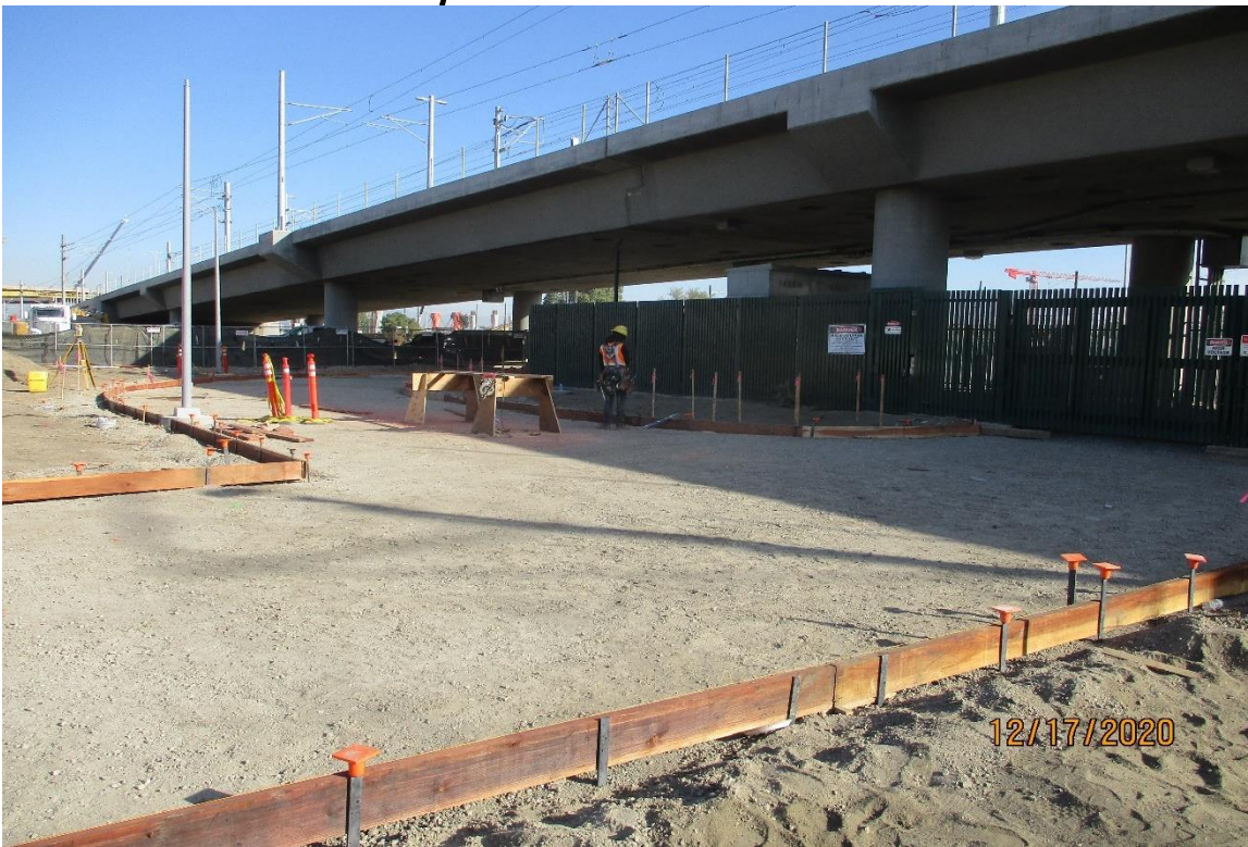
AVIATION/CENTURY- Setting header boards for the Aviation Station service road.
