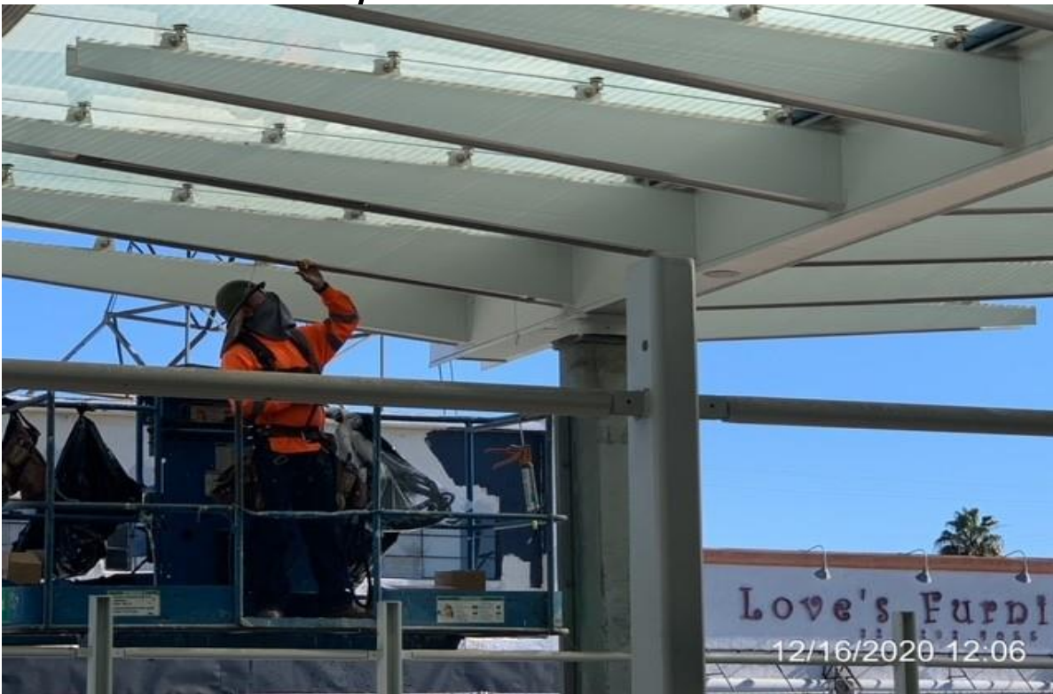
MLK STATION – VNSM caulking between Boca lights at main entrance canopy.
