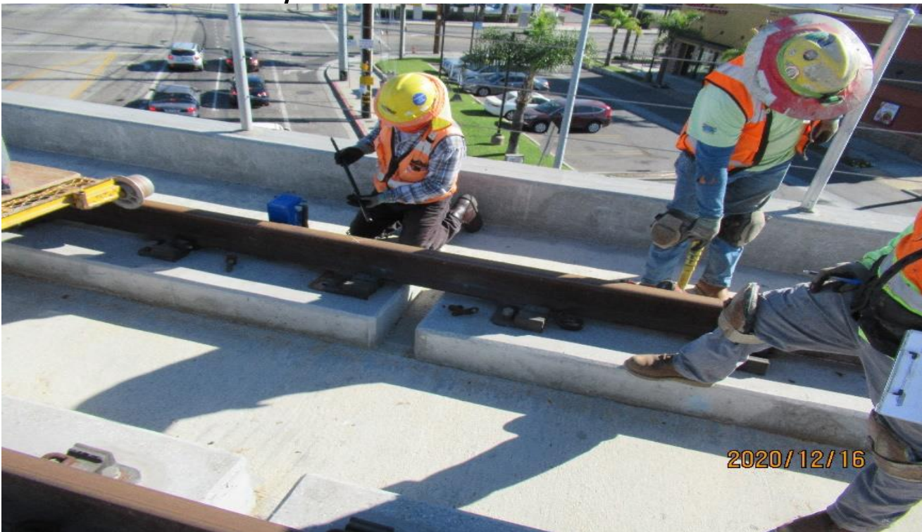
Manchester Bridge - DB Excavating conduit trench at Century and Aviation.
