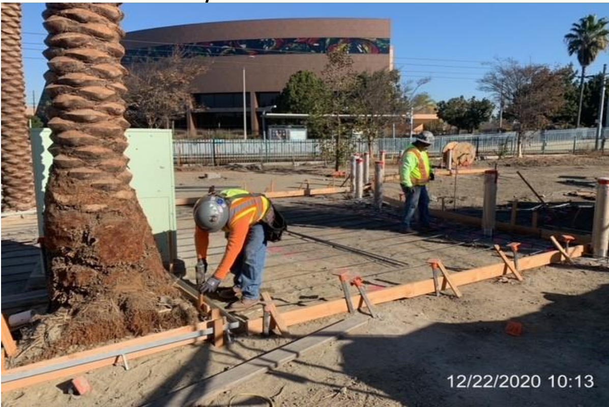
EXPO STATION – Dean Visosky forming sec. 12 for concrete slab.
