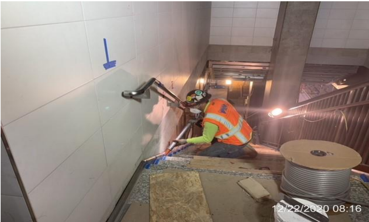
MLK STATION – Carrara Marble caulking edges of stair #2.
