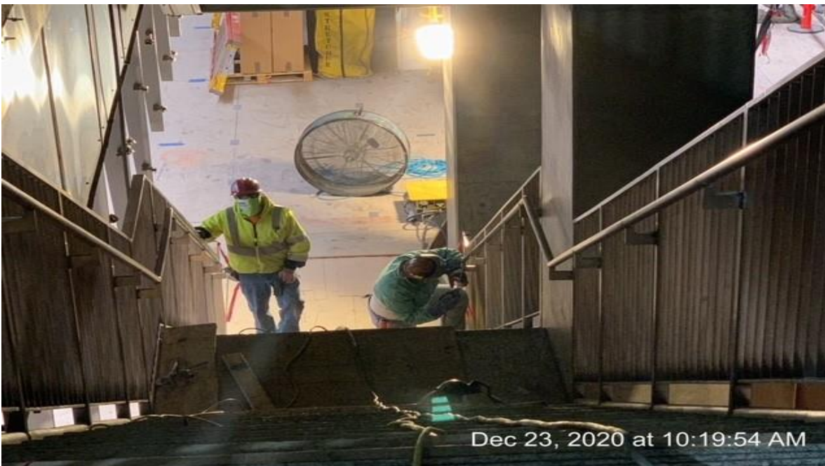
MLK STATION – McMahon setting handrails for welding at stair #3.
