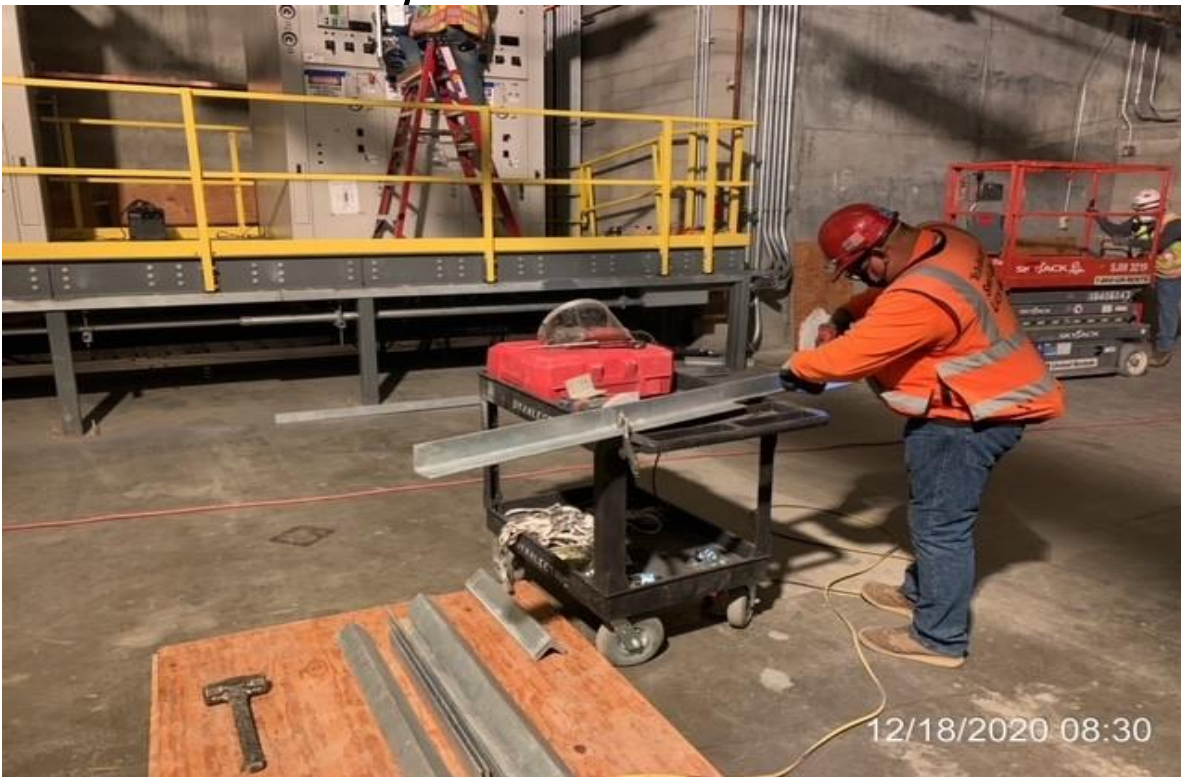
MLK STATION – WSCC ironworkers installing edge skirt for transformer platform.
