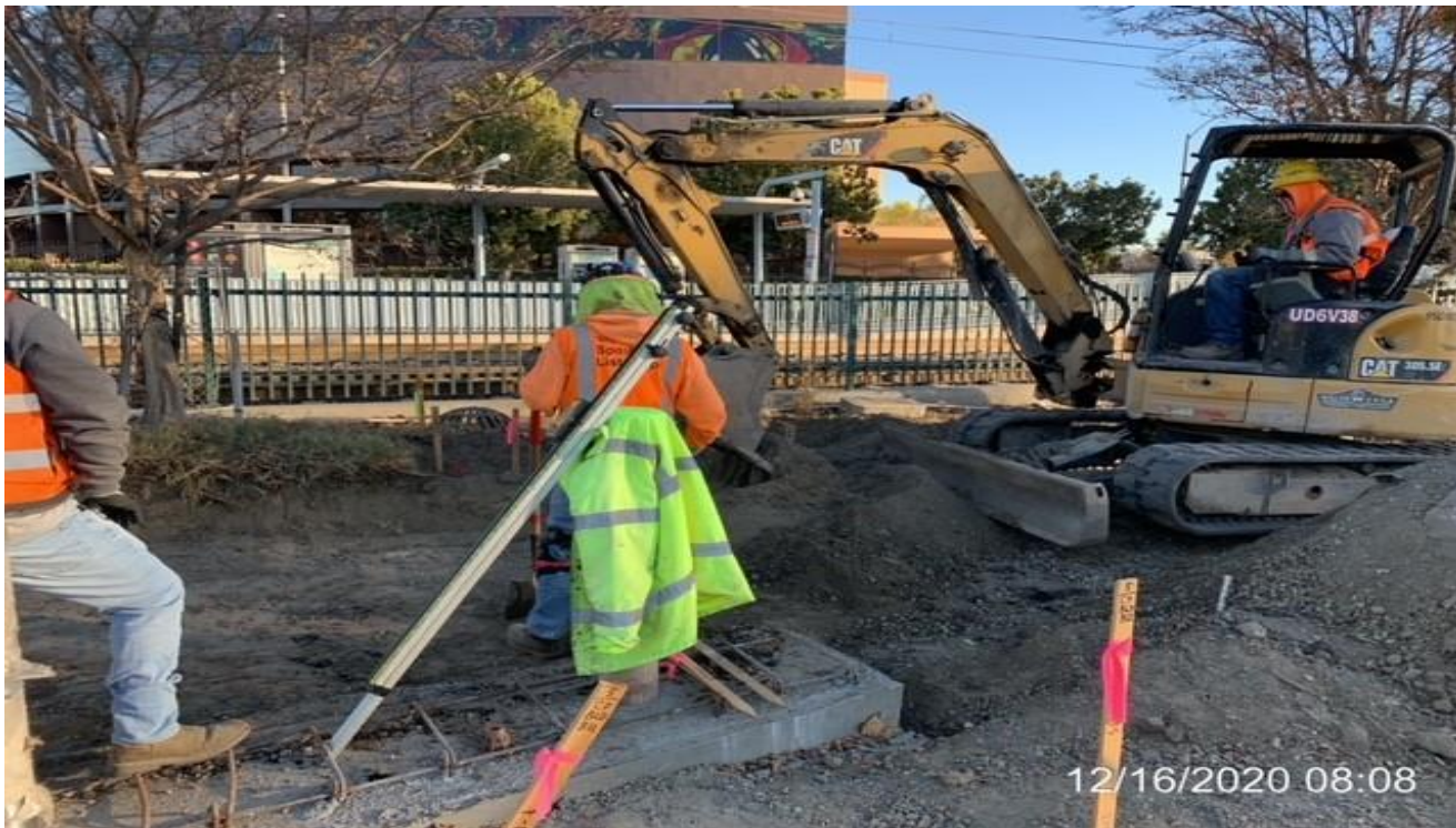
EXPO STATION – WSCC crew grading along north end of station.
