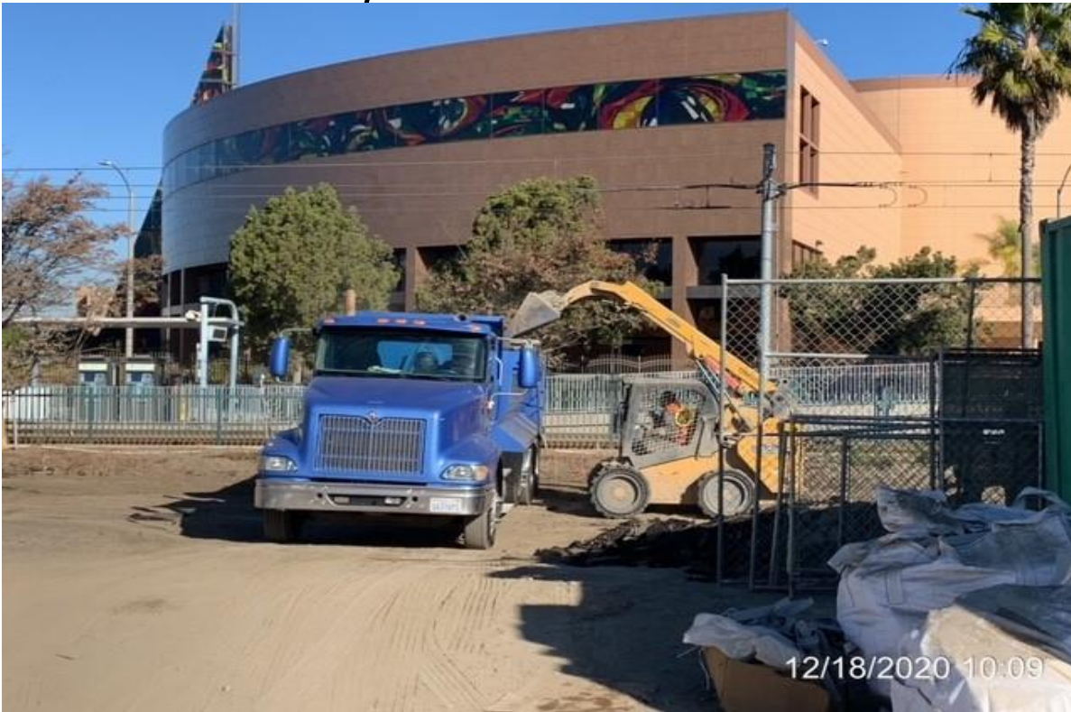
EXPO STATION - WSCC crew loading out demoed temp AC.
