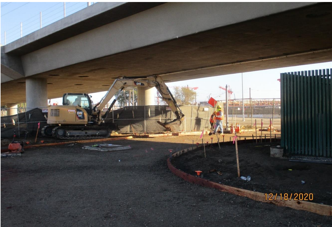
AVIATION/CENTURY- Grading for the Aviation Station service driveway.
