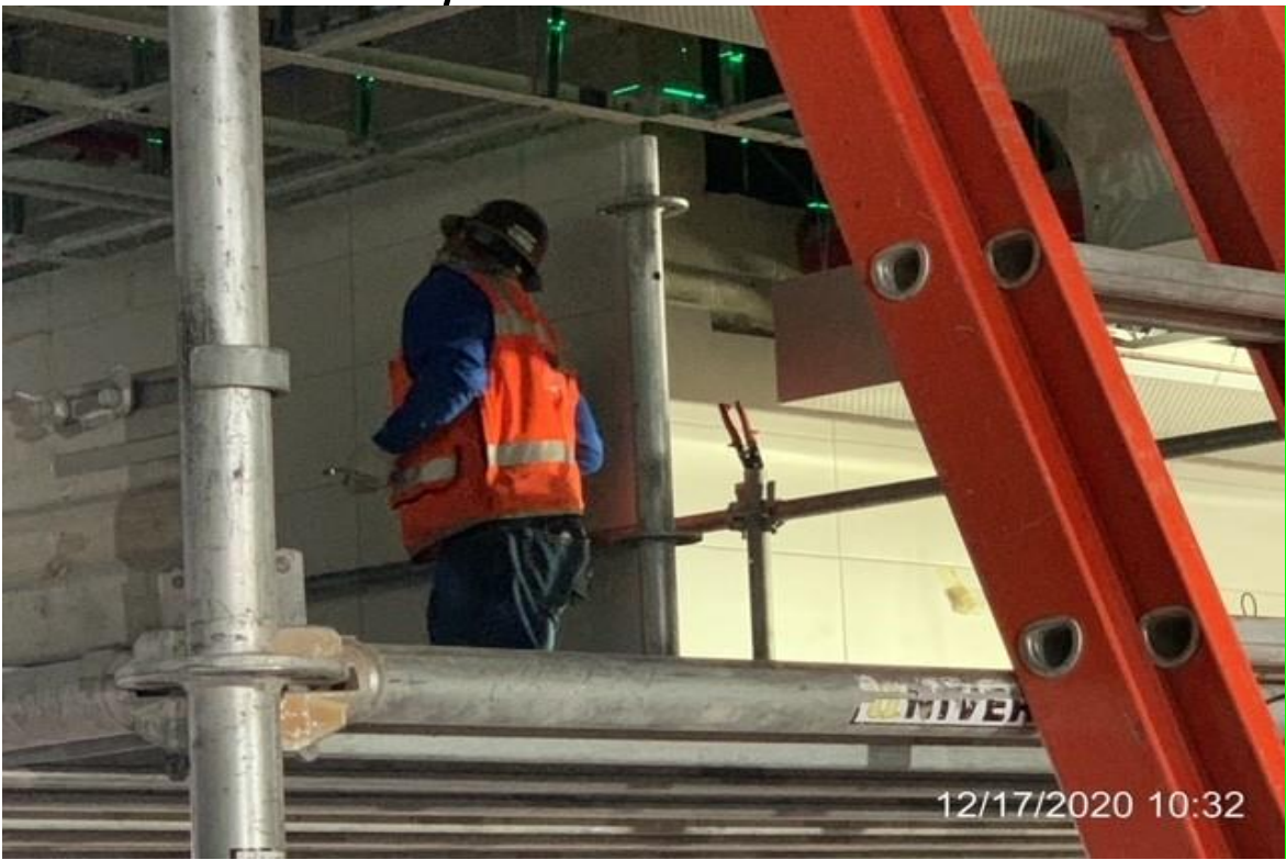
EXPO STATION – PCI installing perimeter for light cove above stair #2..
