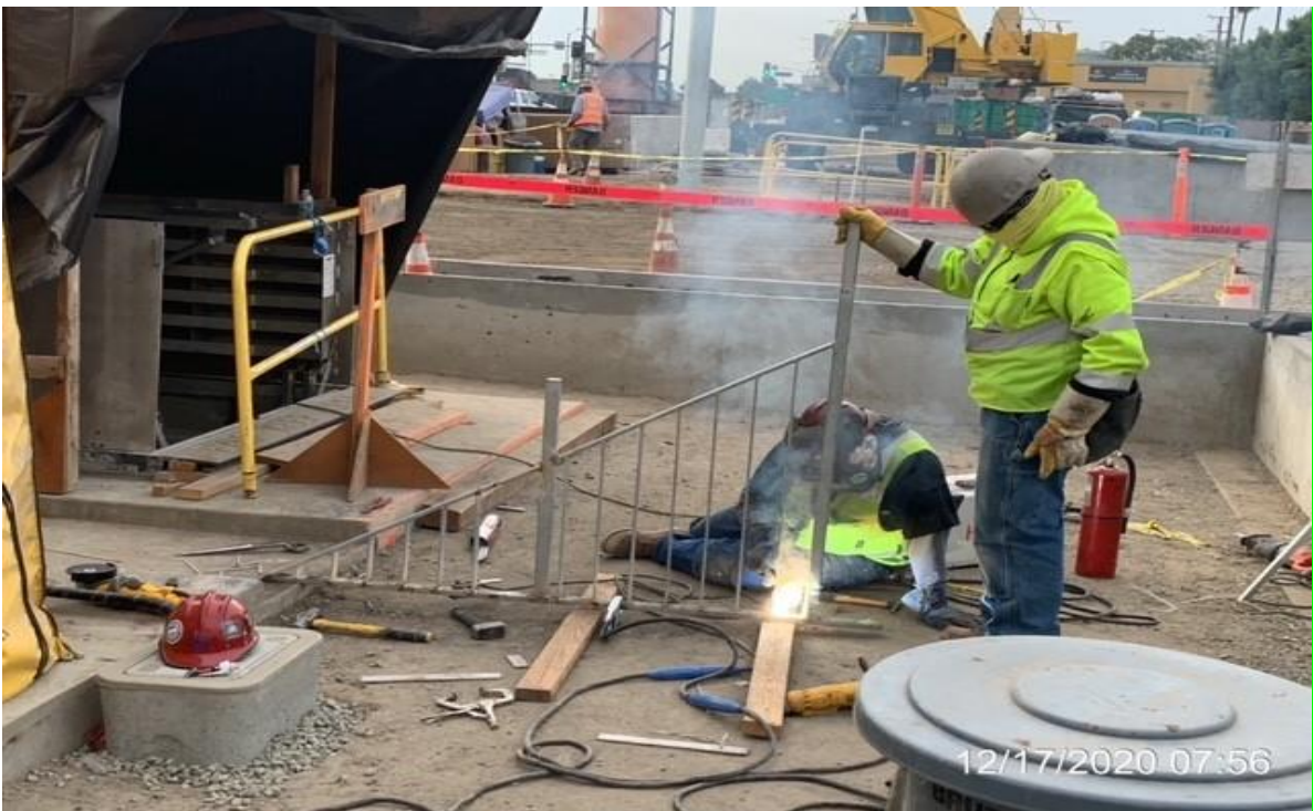
MLK STATION – McMahan prepping guardrails for installation.
