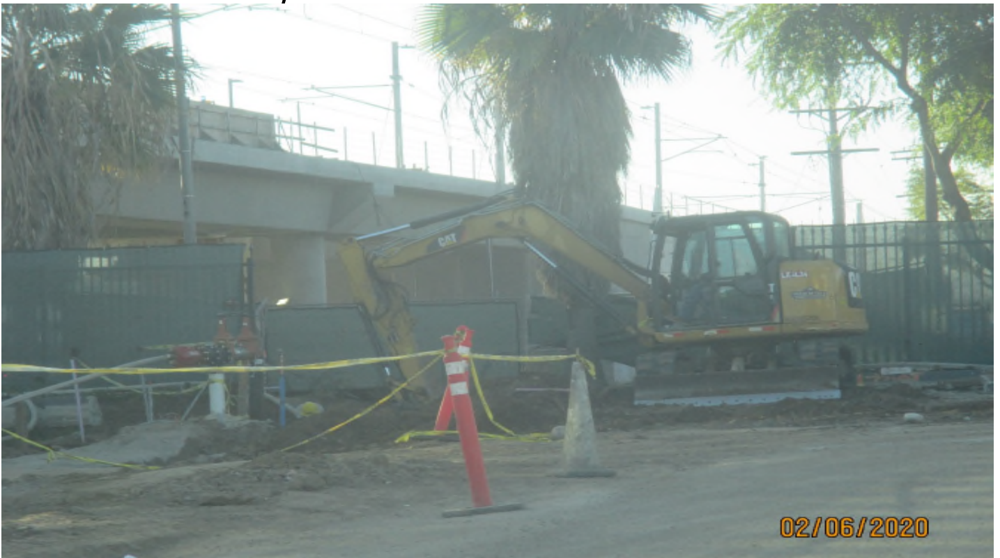
Aviation/Century – Fire line excavation at the Aviation Station.
