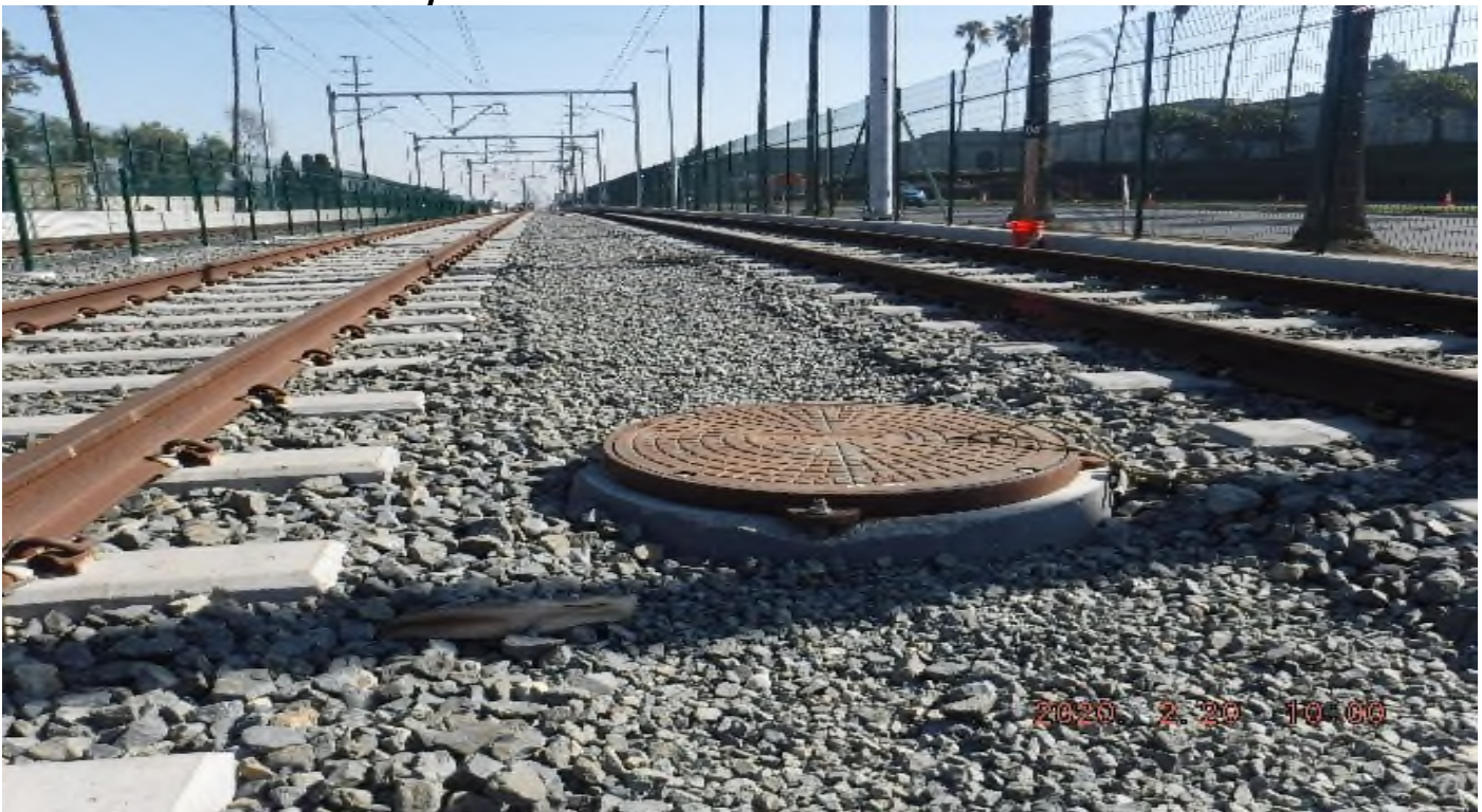
Centinela Ave. – STA 249+74 TK#4 NB looking north – MH#69 rim elevation vs. TOT, damaged cone; no track work.
