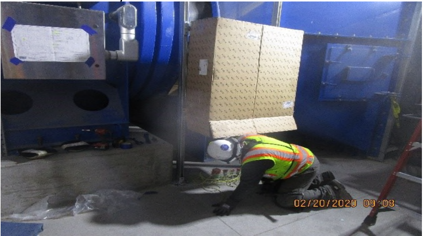
Crenshaw/MLK - MLK Emergency Fan room EVF-7-321 Continued at pull box 2 of 2 rough in supports per non approved plan
