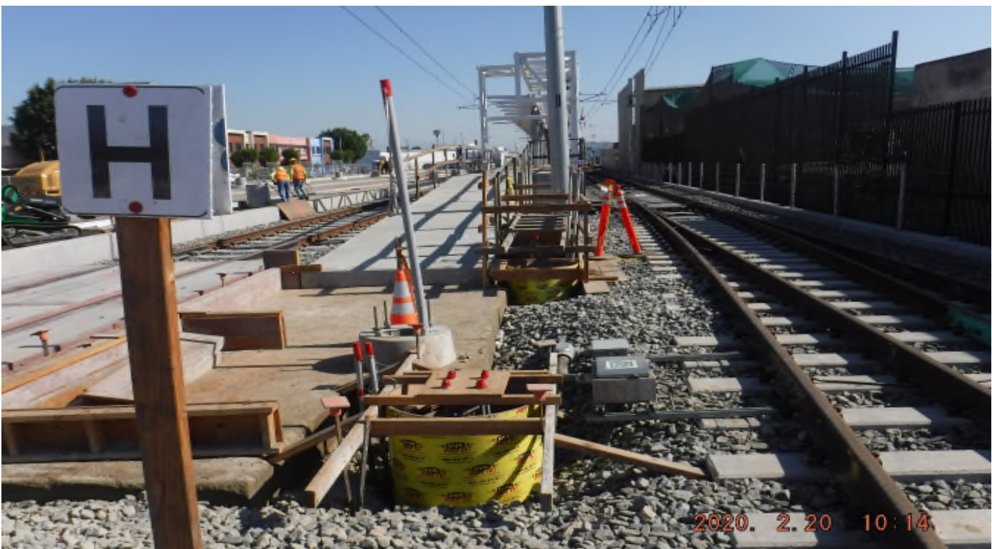
Florence/West – STA262+75_ lookN_ Landing pad & foundation vacuum excavation status_ PUNCH LIST.
