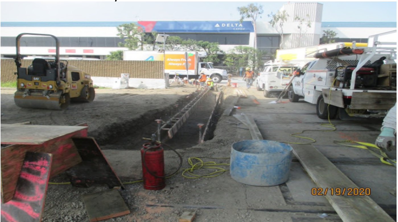
111 th Street – Forming the curb & gutter on 111th street. Facing west.
