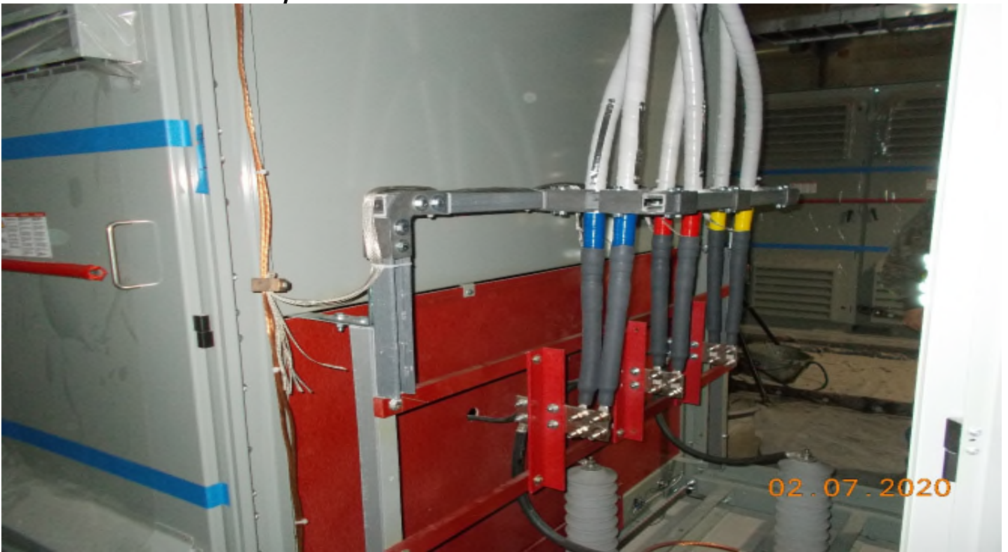
Crenshaw/Vernon - Faith Electric was landing high voltage cables in PX2S.
