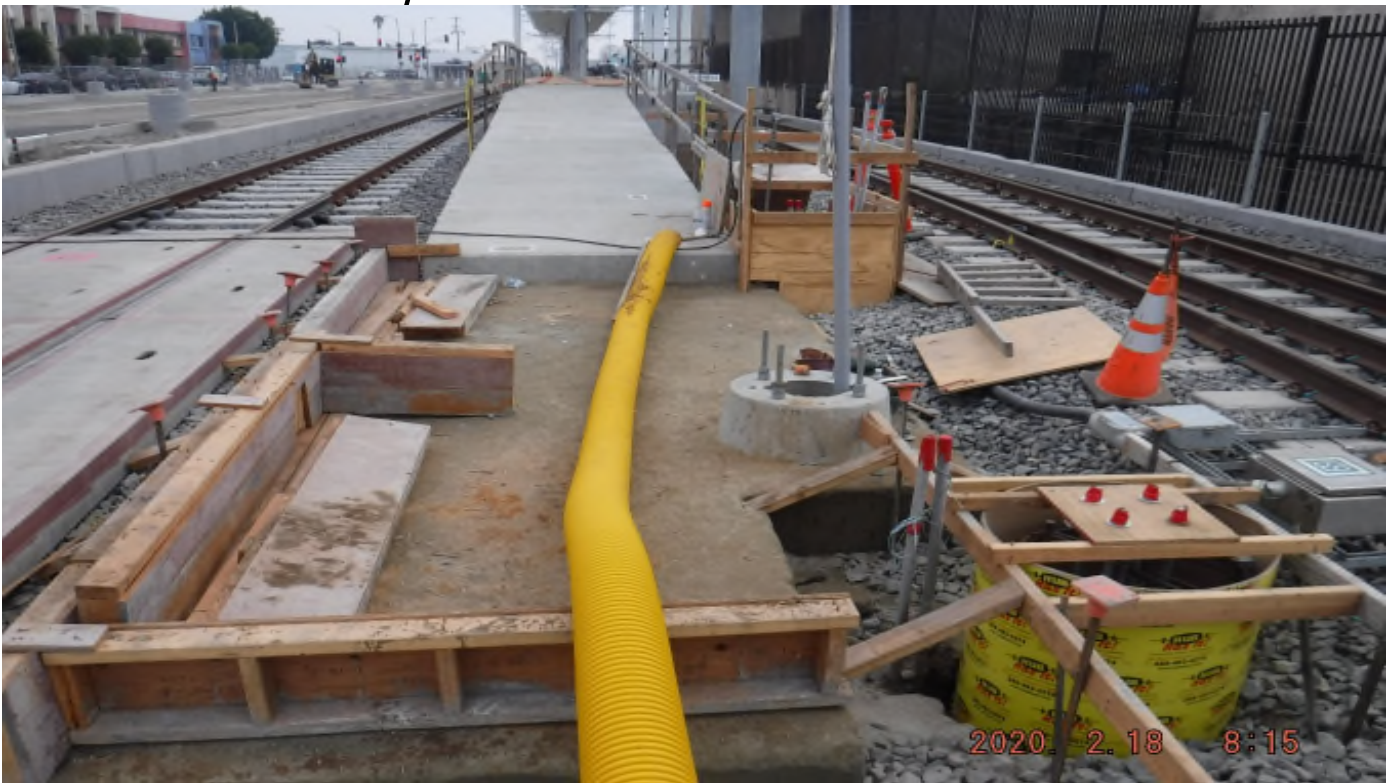
Florence/West – STA262+75_ lookN_ Landing pad & foundation vacuum excavation status_ PUNCH LIST.
