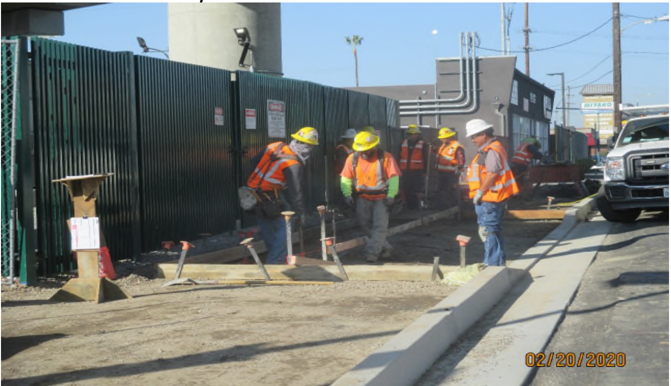
Manchester Bridge – Forming the TPSS #3 drive approach on Manchester.
