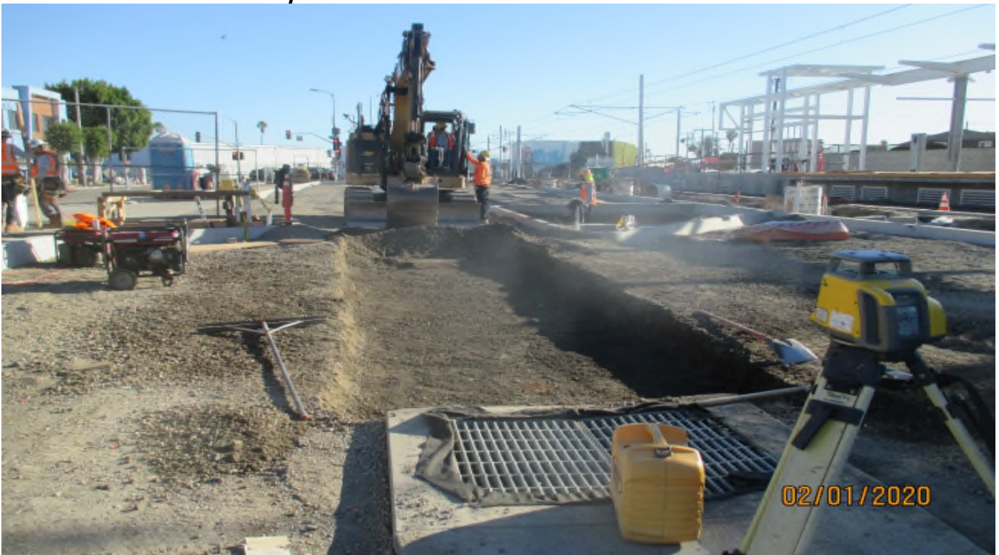
Florence/West – Cross gutter grading at the West Station park and ride.
