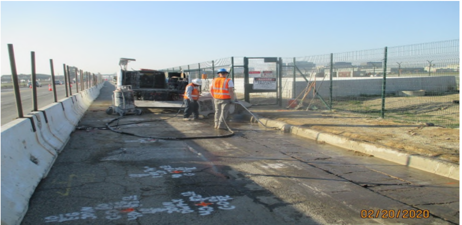
UG - 1 – Saw cutting the existing curb & gutter for demo at UG-1. Facing south.
