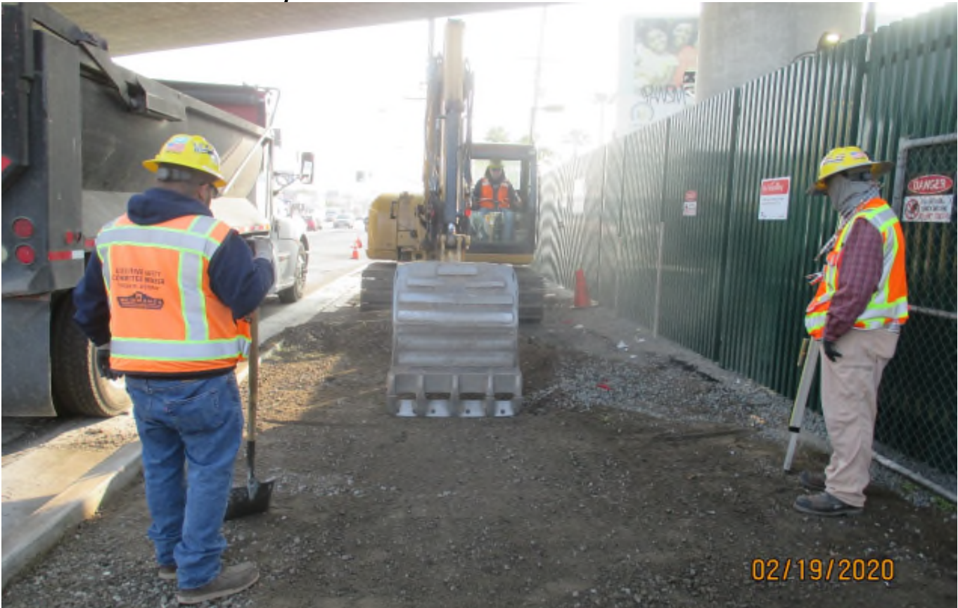
Manchester Bridge – Cutting sidewalk subgrade on Manchester.
