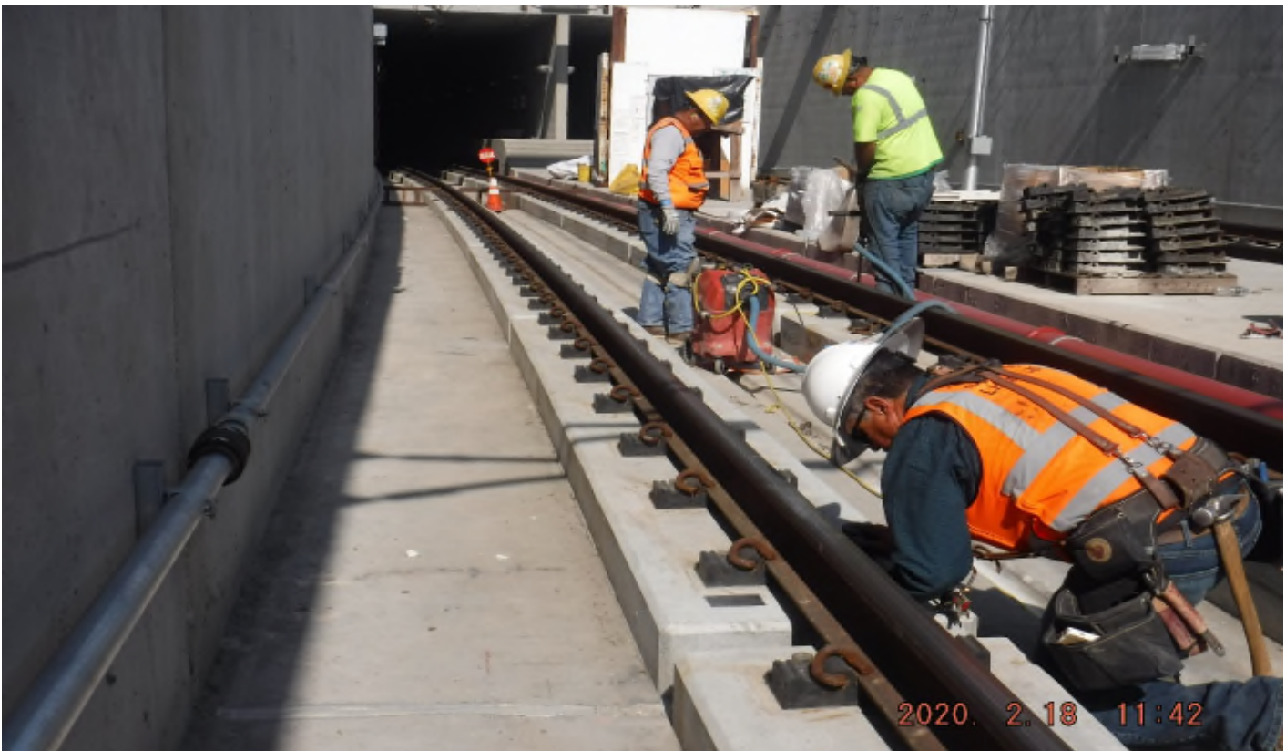
UG-4- STA366+45_ LT plinth patching_ NCR-A-111_UG4_48ST.
