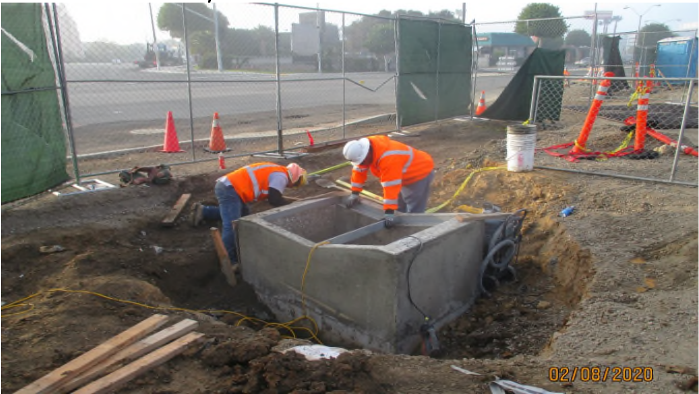
Florence/Brea – Catch basin concrete finish work at the La Brea Station.
