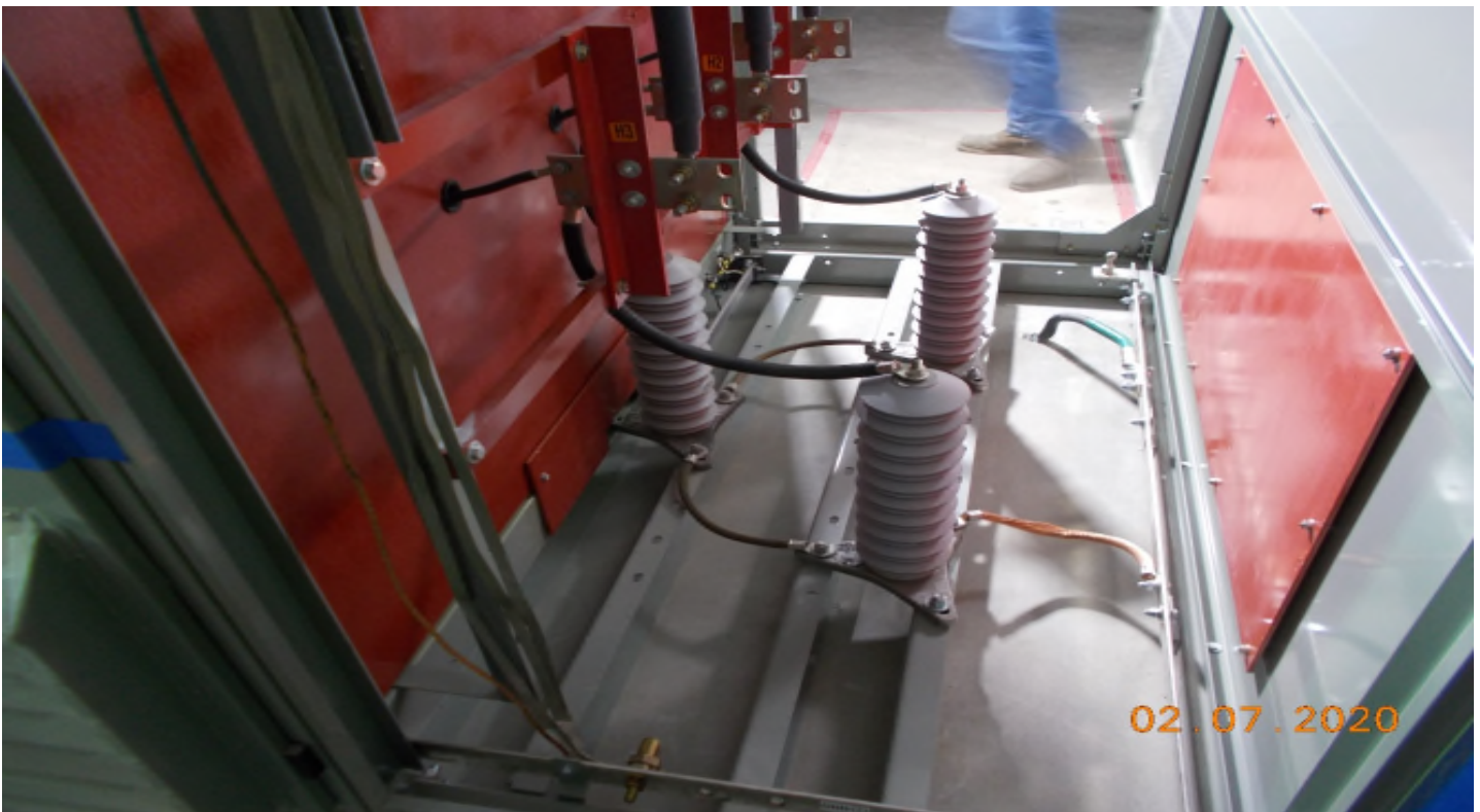
Crenshaw/Vernon - Faith Electric was cleaning surge arrestors in PX2S.
