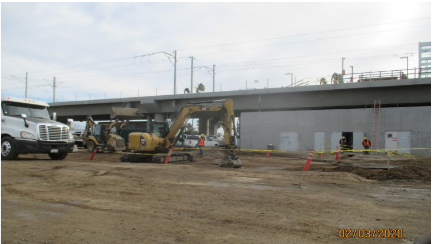
Aviation/Century – Grading and excavating at the Aviation Station plaza area.
