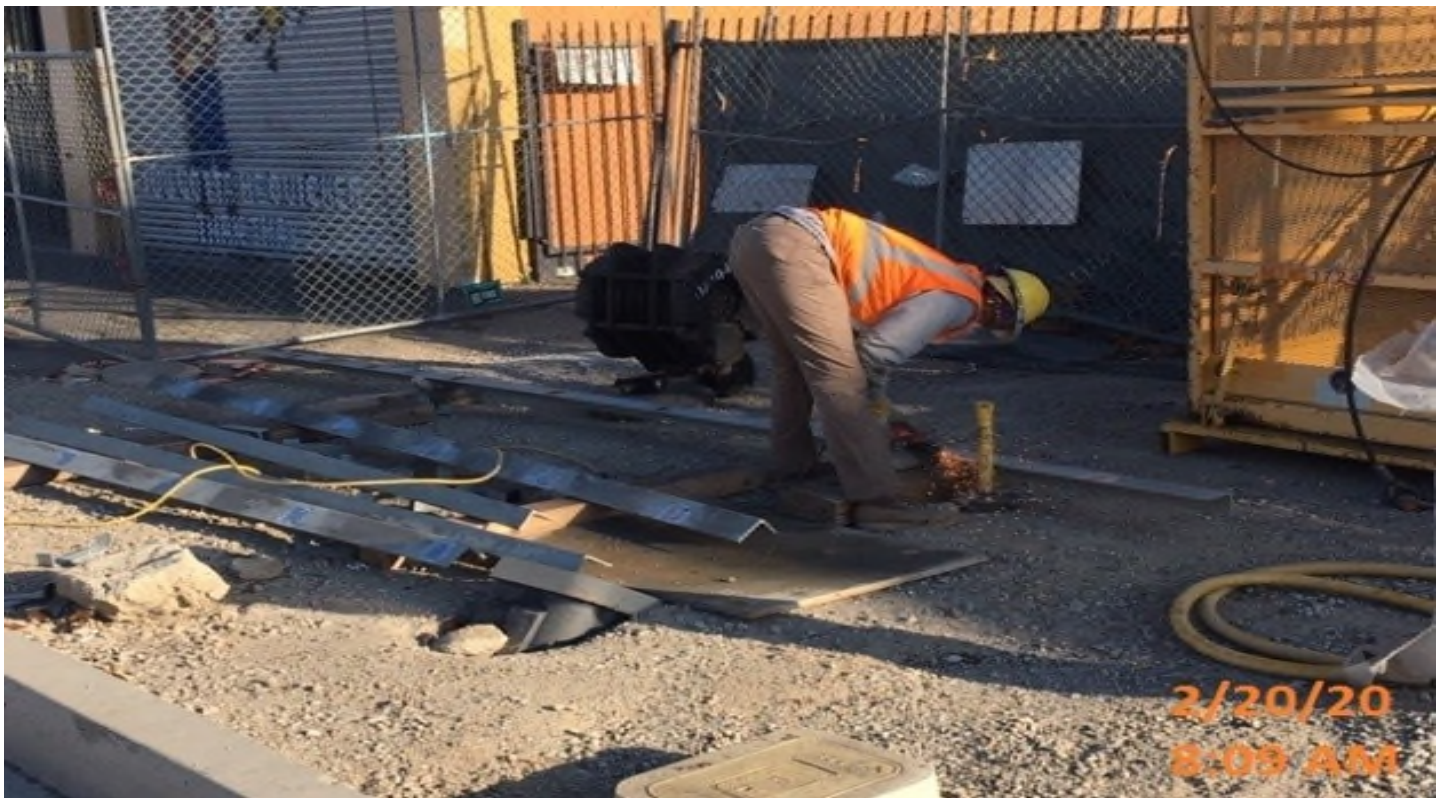
Crenshaw/Vernon - VERNON – Giroux Glass aligning and spacing canopy glass panels.
