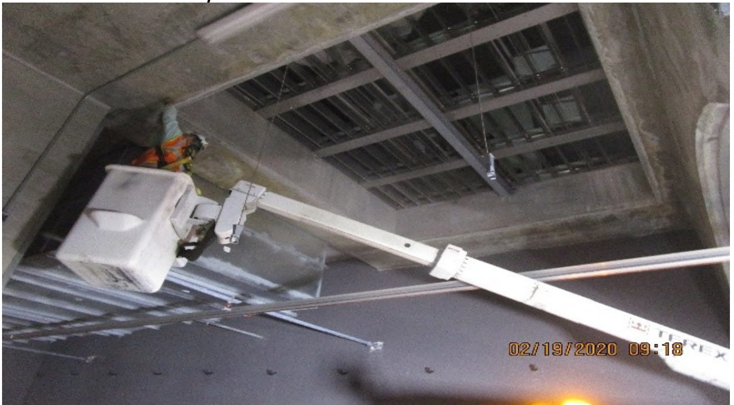
Crenshaw/MLK - Northbound track, Equipment load zone P101 continued installing Radiax cable support brackets.
