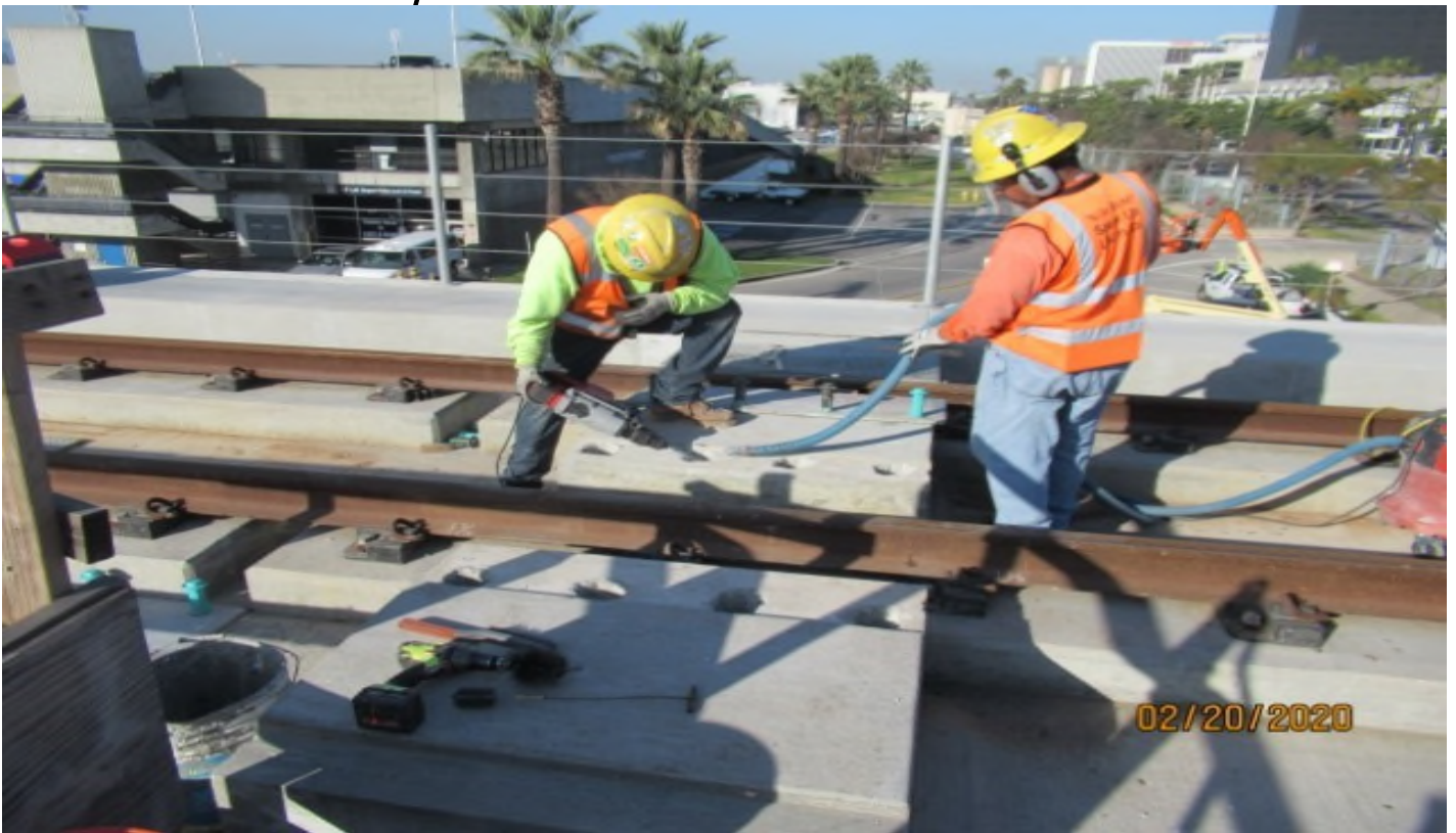
Aviation/Century – WSCC using E-hammer to chip out inserts holes on Century, Aviation bridge SB #3 track STA 66+09
