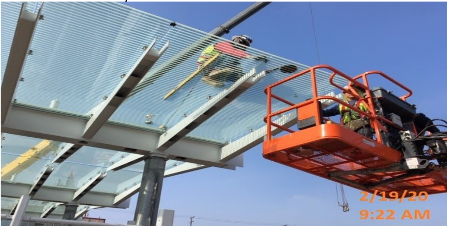
Crenshaw/Vernon - Vernon – Giroux Glass aligning canopy glass.
