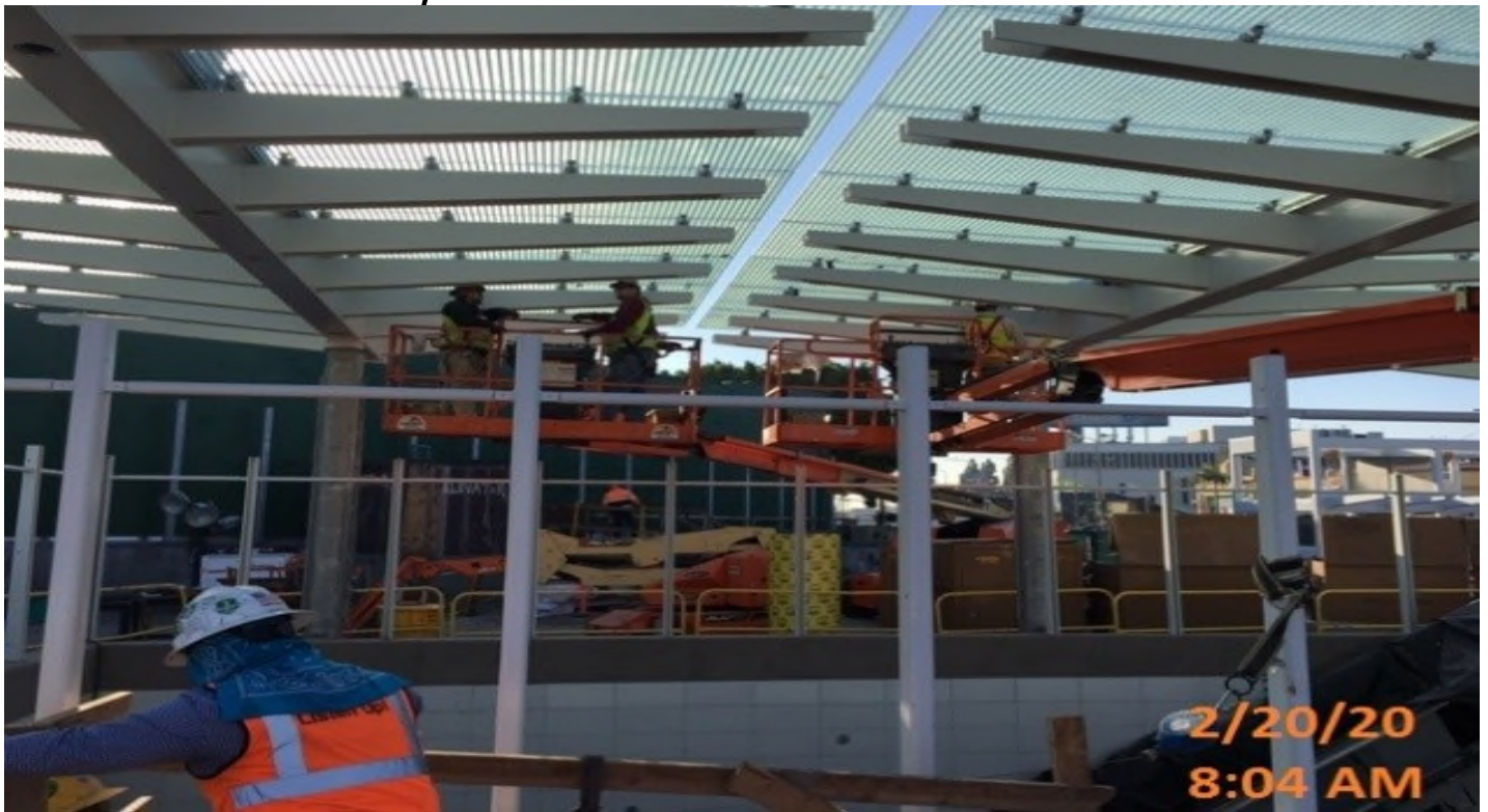
Crenshaw/Vernon - VERNON – Giroux Glass aligning and spacing canopy glass panels.
