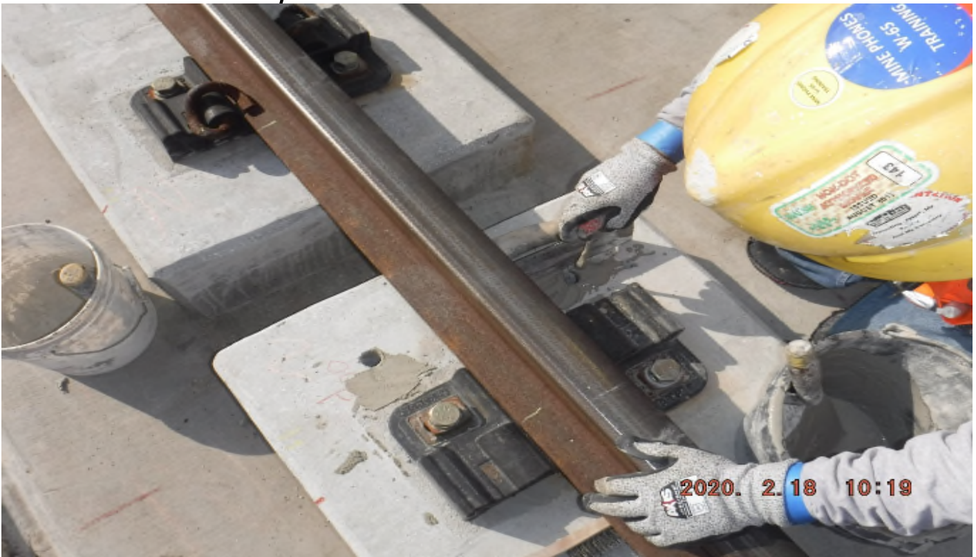
UG-4- STA366+45_ LT plinth patching_ NCR-A-111_UG4_48ST.
