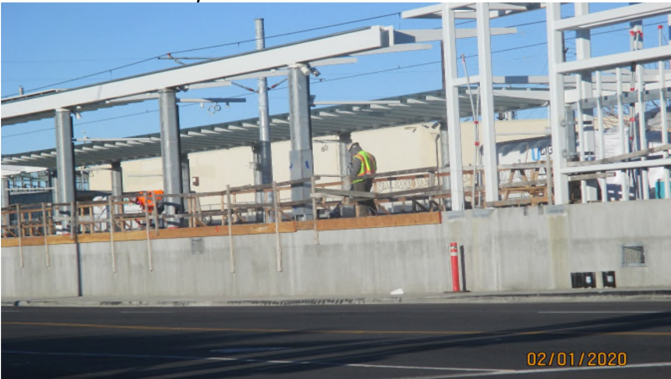
Florence/Hindry – Saw cutting expansion joints and buffing the topping slab at the NB Hindry Station platform.
