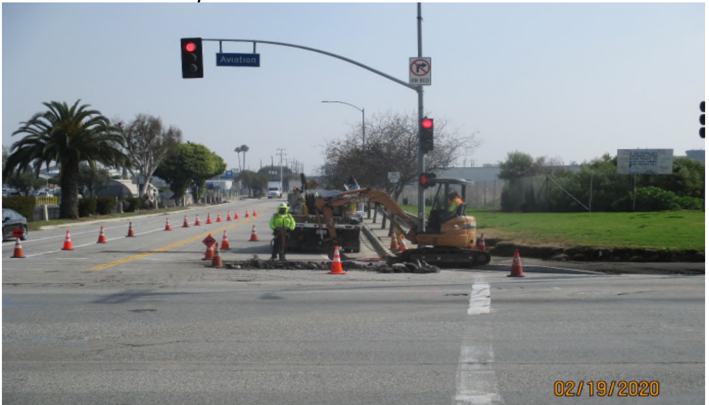
Aviation/Century – Signal conduit installation at 111th and Aviation.
