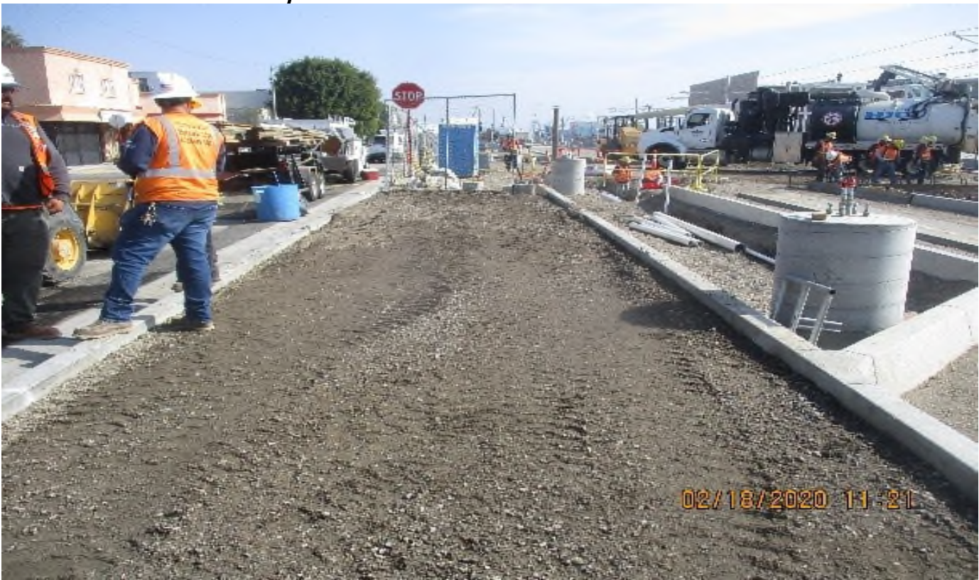
Florence/West – WSCC Making fine grade for asphalt and SWK at West Sta park and ride.
