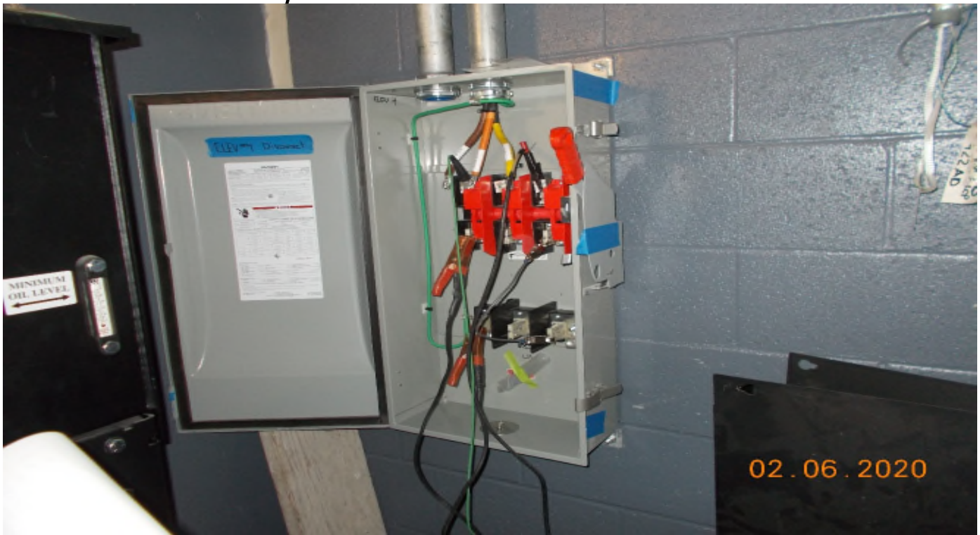
Crenshaw/Vernon - NETE was megger testing elevator disconnects.
