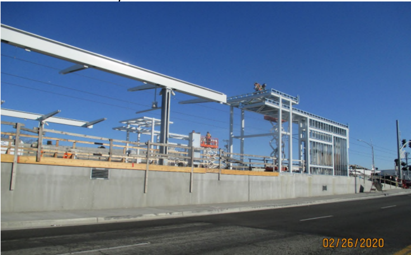
Florence/Hindry – Metal stud framing at the Hindry Station.
