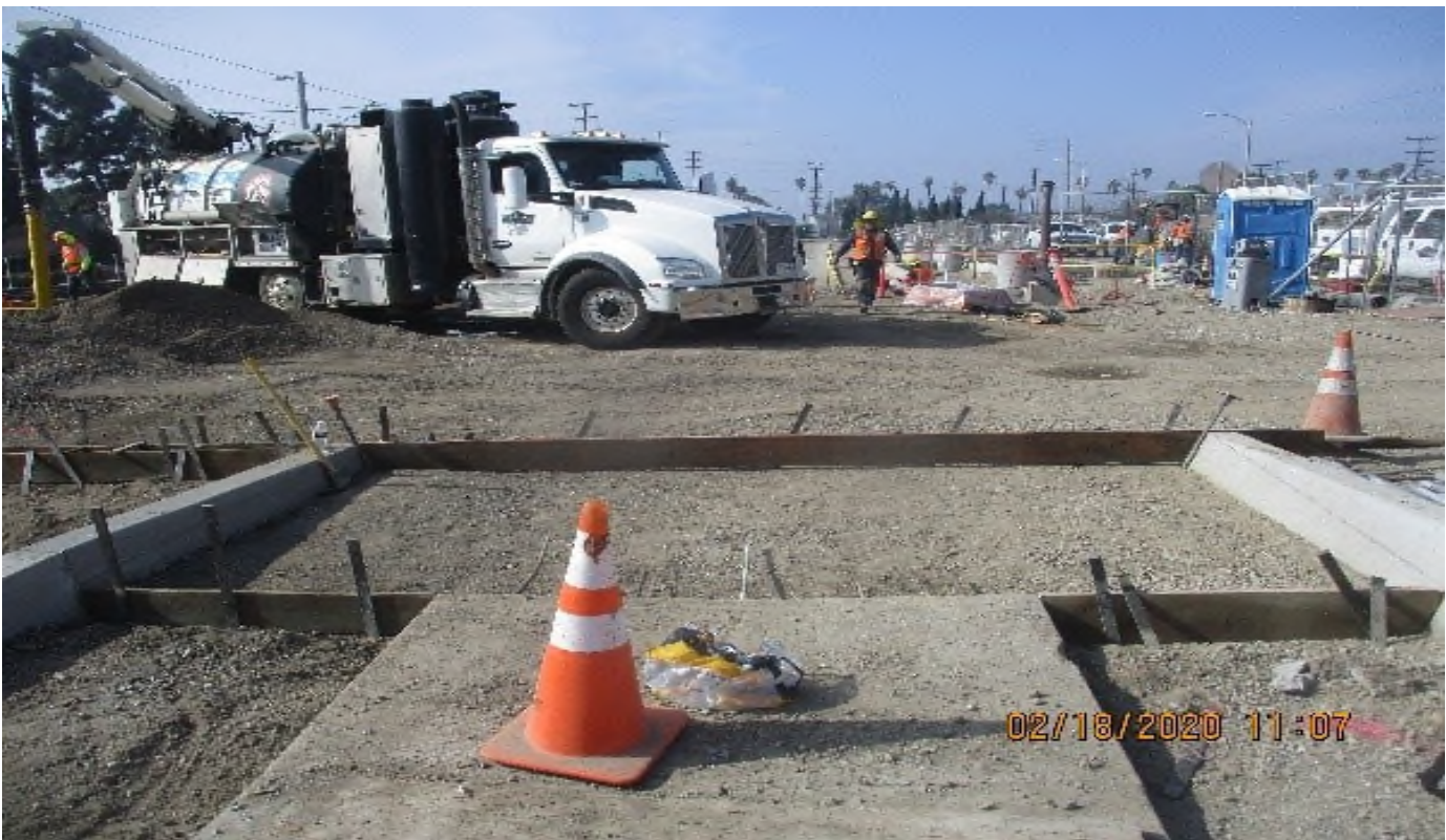
Florence/West – WSCC Making fine grade for asphalt and SWK at West Sta park and ride.
