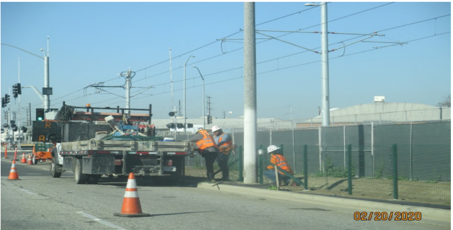
Aviation/Century – WSCC using E-hammer to chip out inserts holes on Century, Aviation bridge SB #3 track STA 66+09
