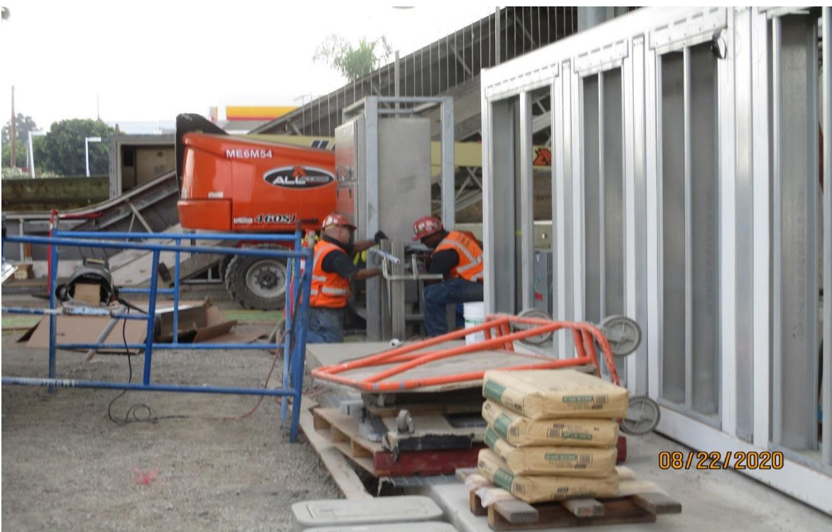
AVIATION/CENTURY- Welding and fabricating on the Aviation Station ticket vending machine.
