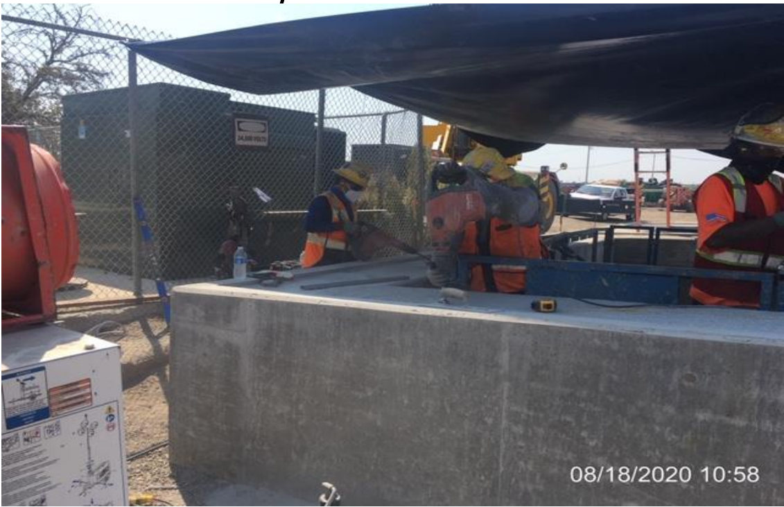
EXPO STATION– WSCC carpenters building formwork for air exhaust shaft #2.
