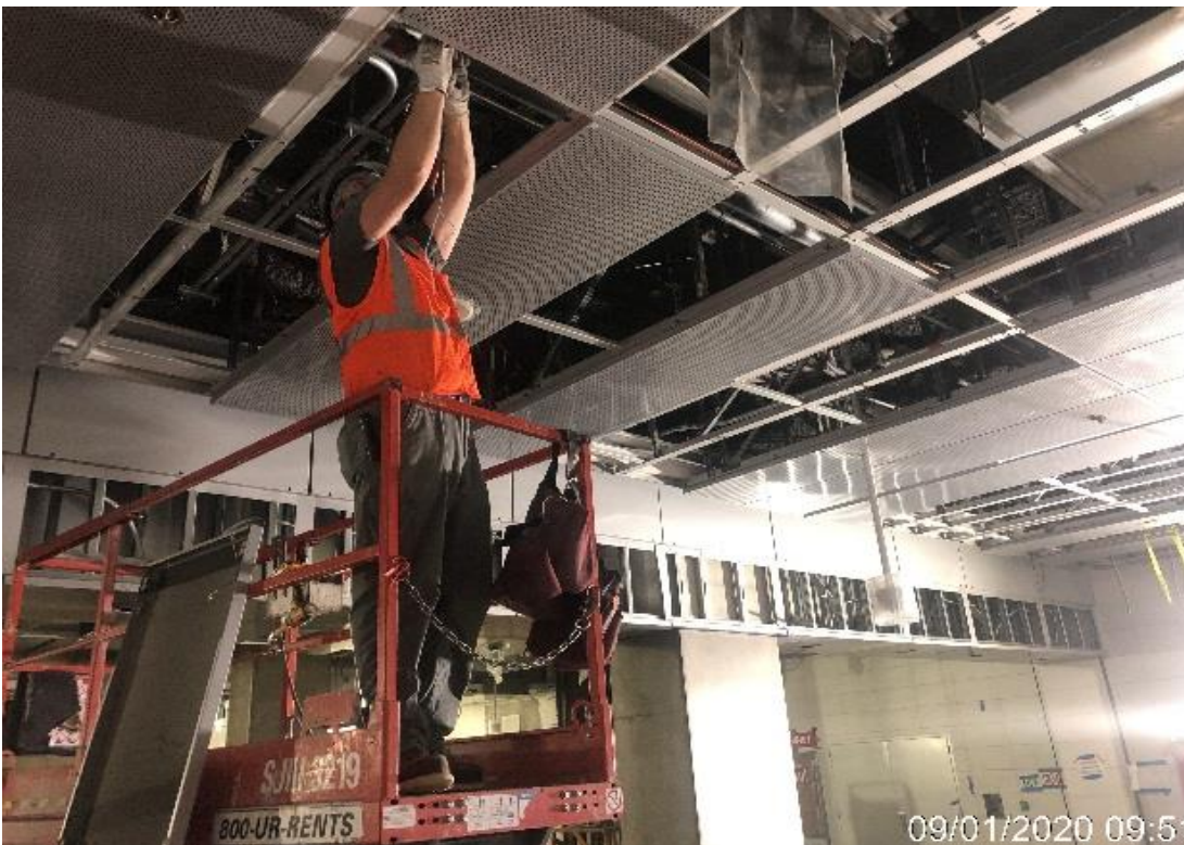
EXPO STATION – Modifying and installing ceiling panels at the concourse level.
