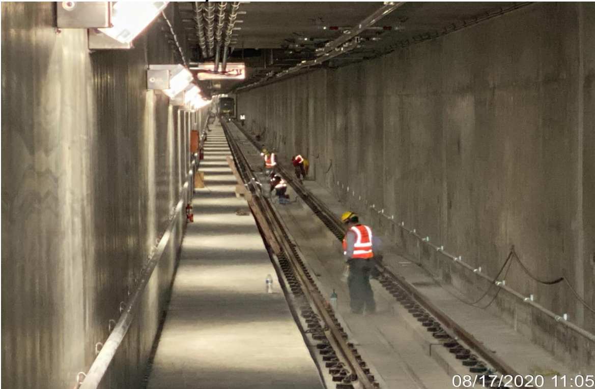
UG3 – WSCC working on plinths at UG-3.
