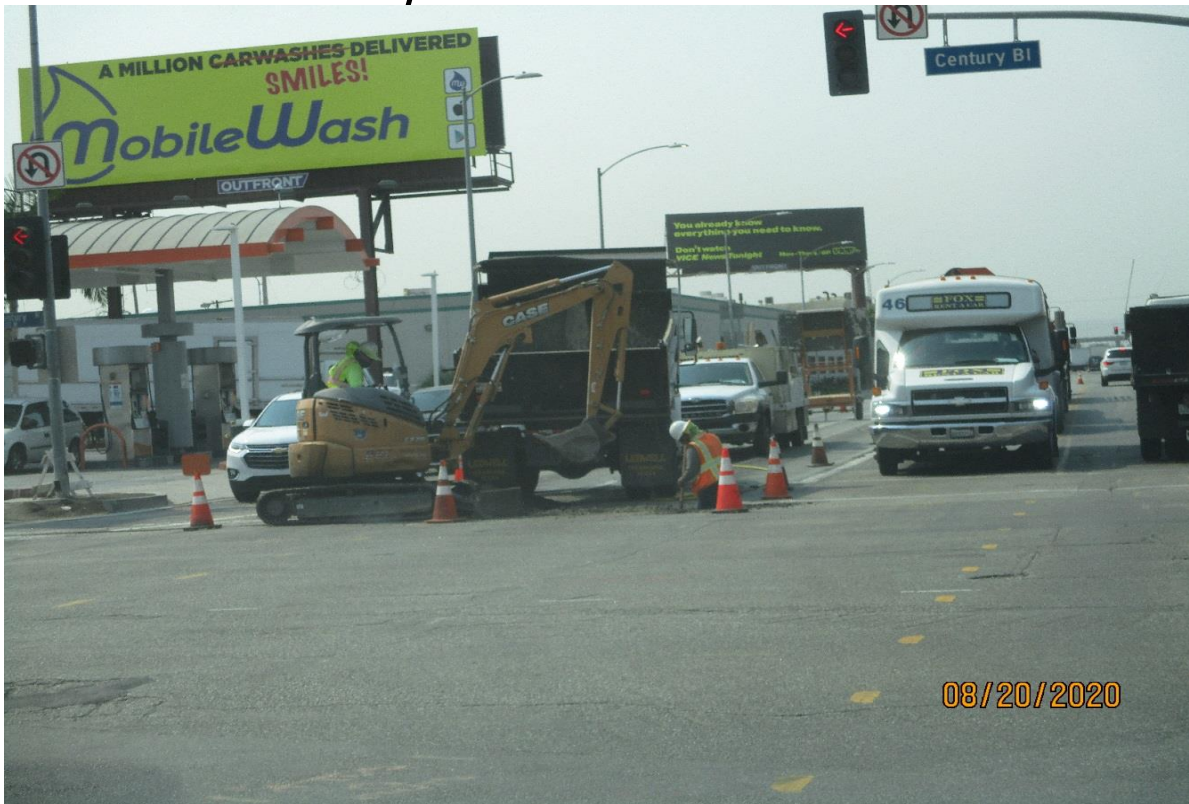
AVIATION/CENTURY- Excavating for the traffic signal conduit on Century. Facing south.
