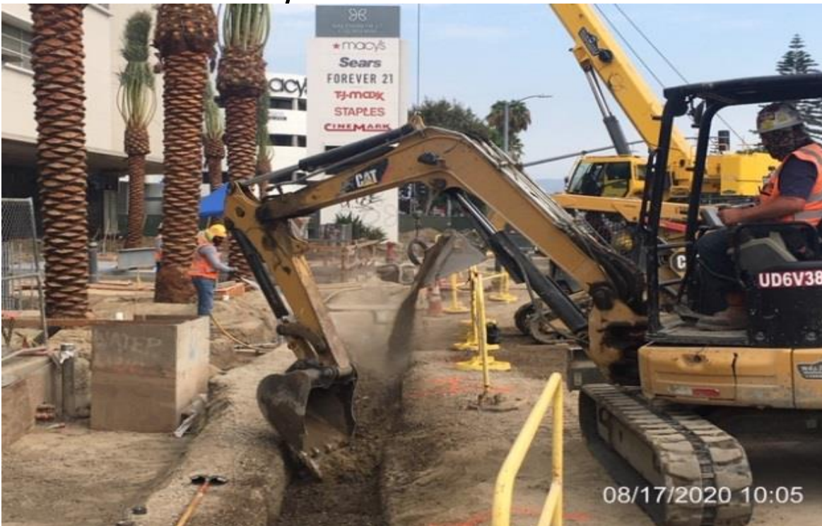
MLK STATION – WSCC crew backfilling and compacting AT&T encased trench.
