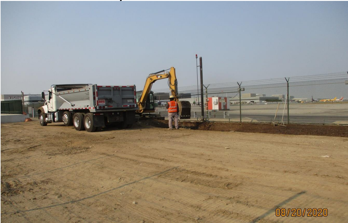
UG1- Drainage swale grading at UG-1.
