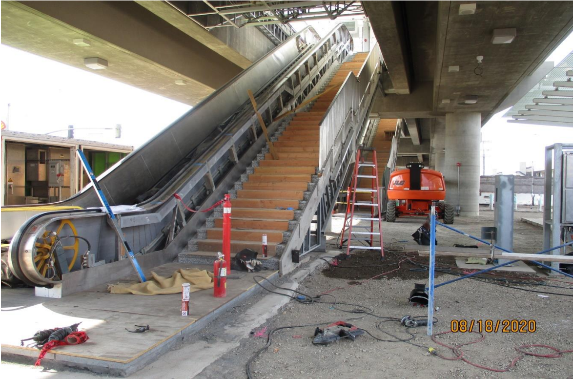
AVIATION/CENTURY- Welding stairway handrails at the Aviation station
