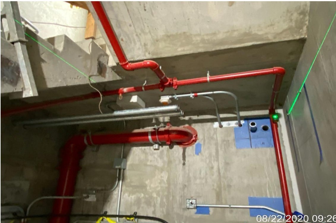
MLK STATION – Dynalectric installing 2” AT&T conduit at MLK.
