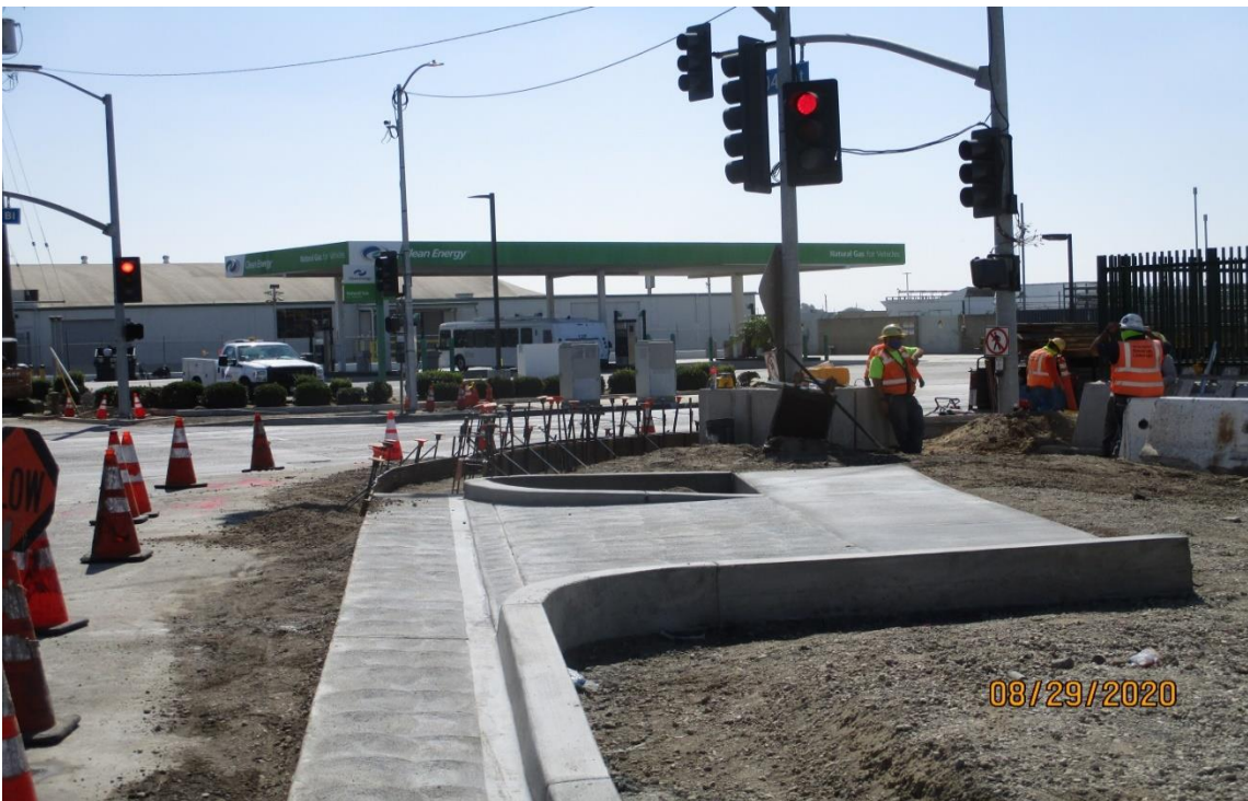
AVIATION/CENTURY- Forms set for the curb and gutter on the SW corner of Aviation and 104th.
