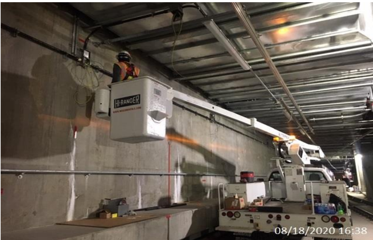
EXPO STATION – Dyna Electric terminating and splicing on SB wall.
