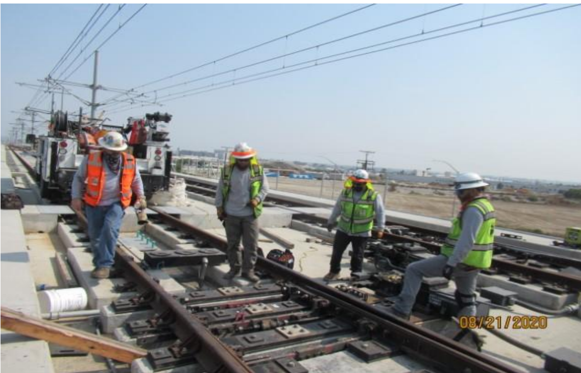
Guideway- LKC & HCC installing & adjusting connecting rods for 10ERH XO at GL Wye (switch point repair) (looking northeast) Rework
