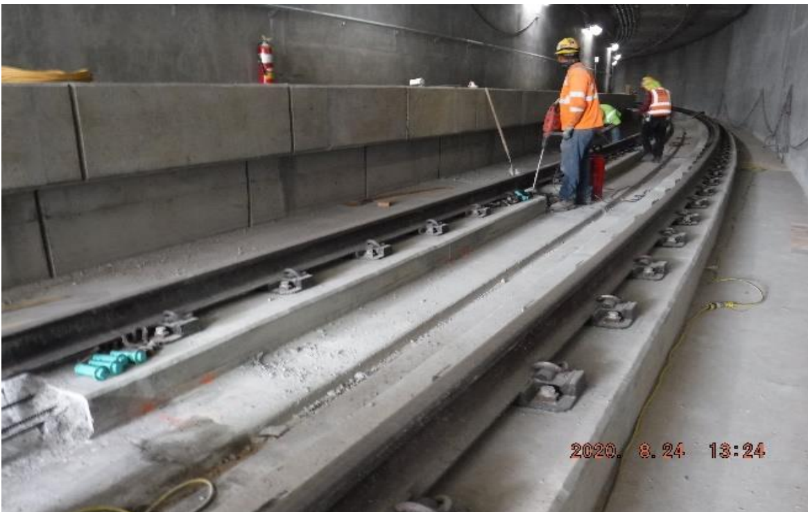
UG3 – STA 284+00 TK#4/NB looking north – NCR-A-111.B Case #4 UG3 (plinth demolition)
