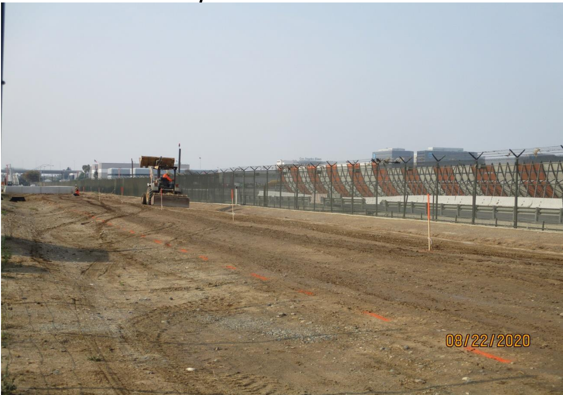
UG1- Grading for the amended soil at UG-1.
