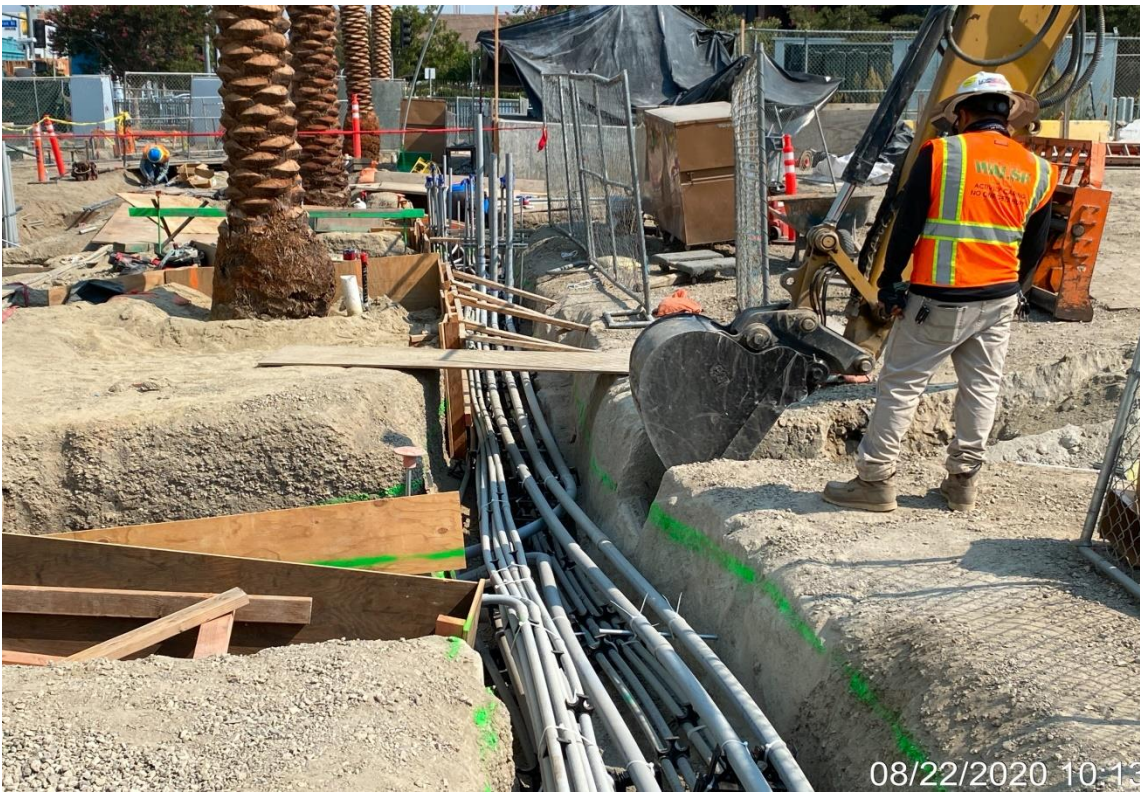
EXPO STATION SITE – WSCC excavating for conduit at Expo Yard.
