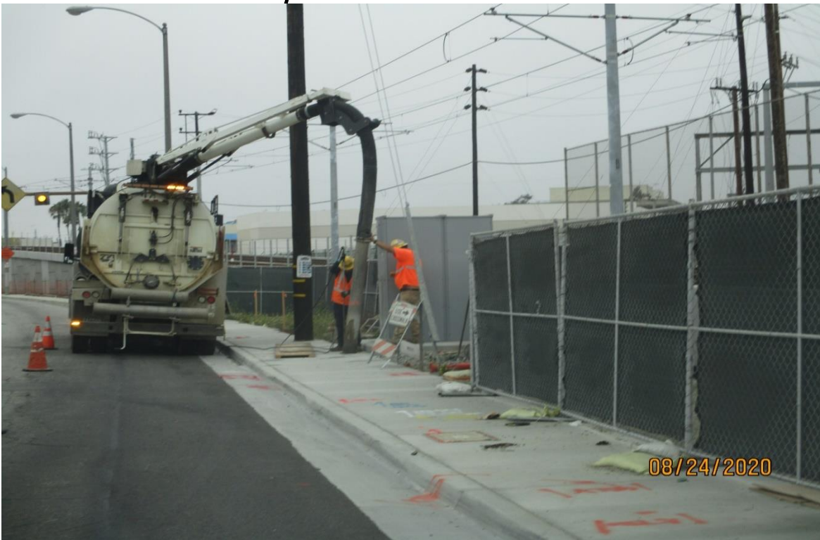
Hindry – Excavating for bollards at the Hindry Station NB platform.
