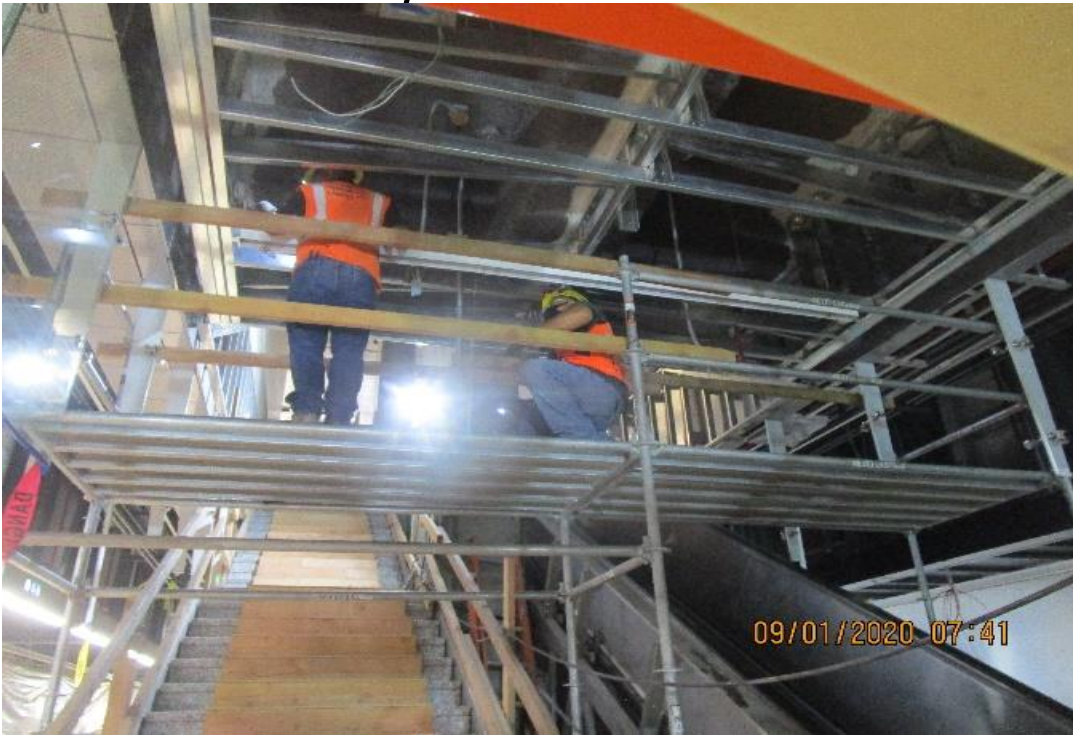
LEIMERT PARK STATION – Installing ceiling light fixtures at the platform level.
