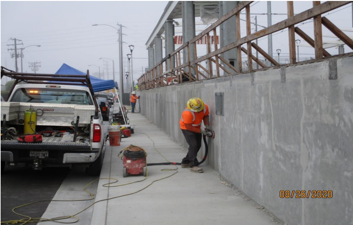
Hindry – Concrete finish work at the Hindry Station.
