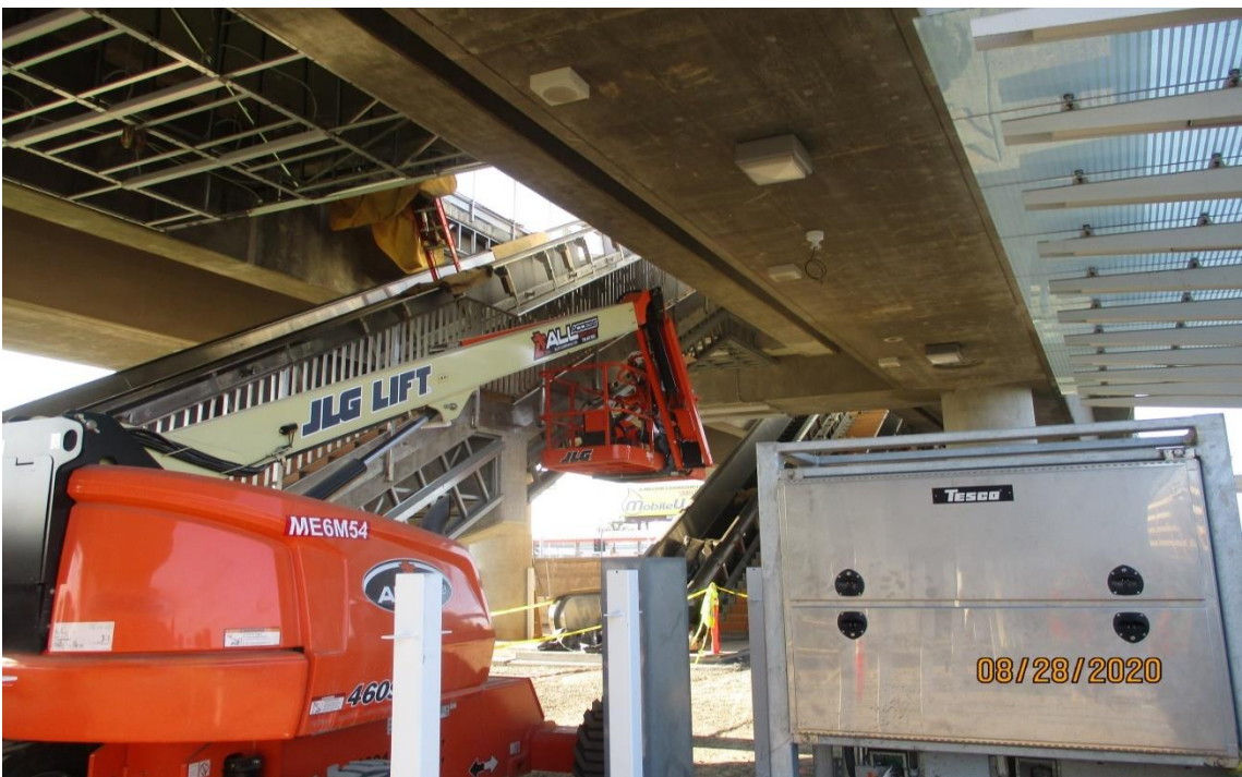
AVIATION/CENTURY- Handrail erection at the Aviation Station.
