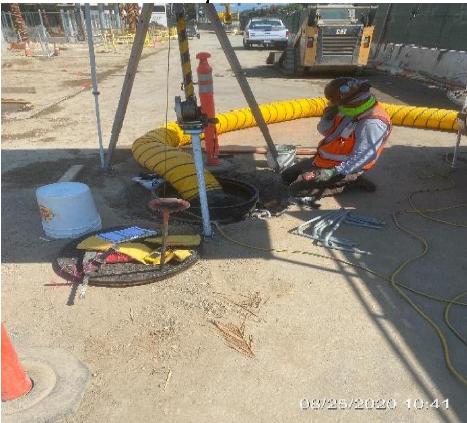
MLK STATION – Installing steel steps inside Manhole #15 at the plaza level.
