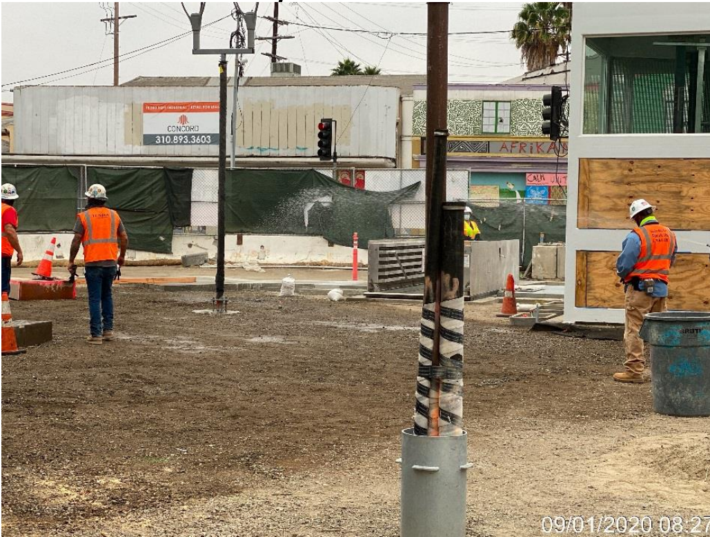
LEIMERT PARK STATION – Resume base grading/compacting throughout the plaza level.
