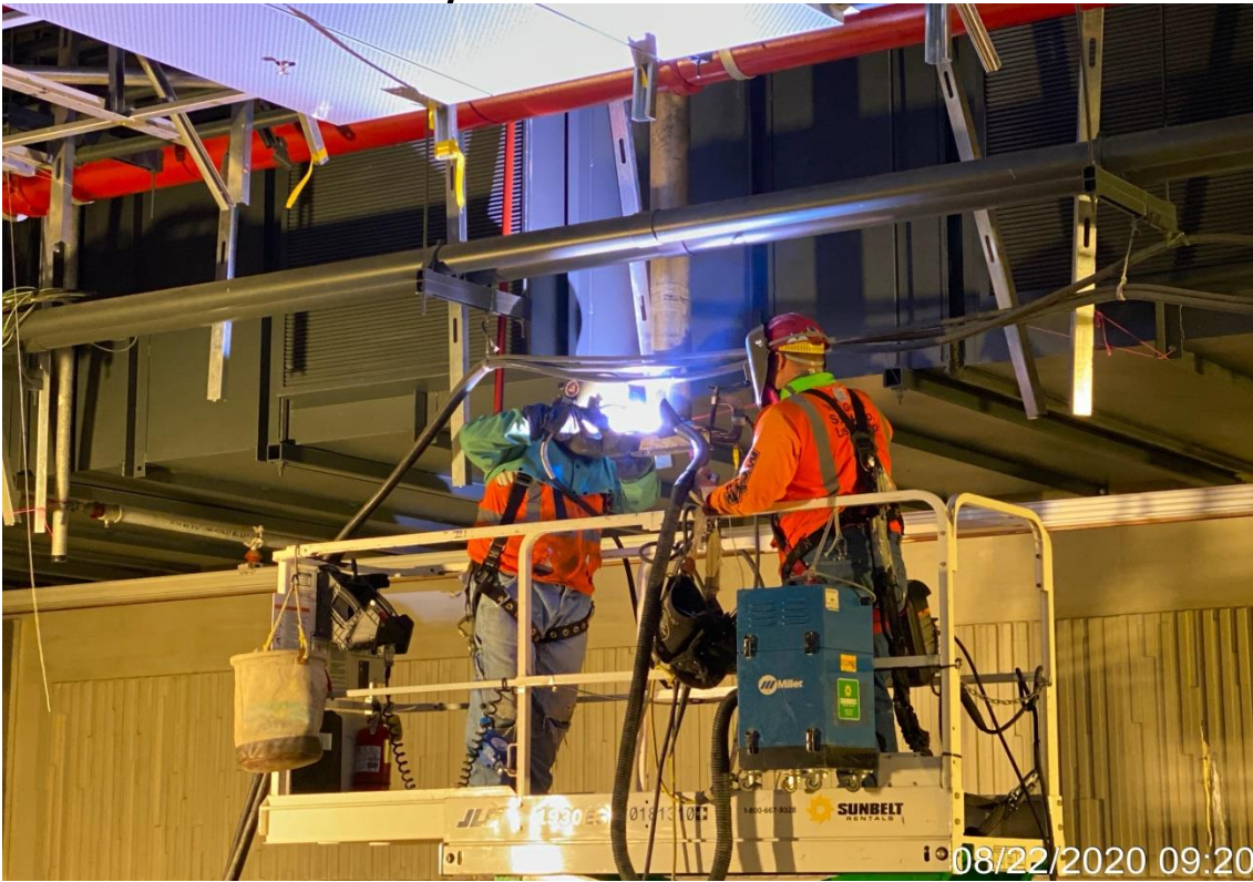
MLK STATION – WSCC welding plates onto Down Stands at MLK.
