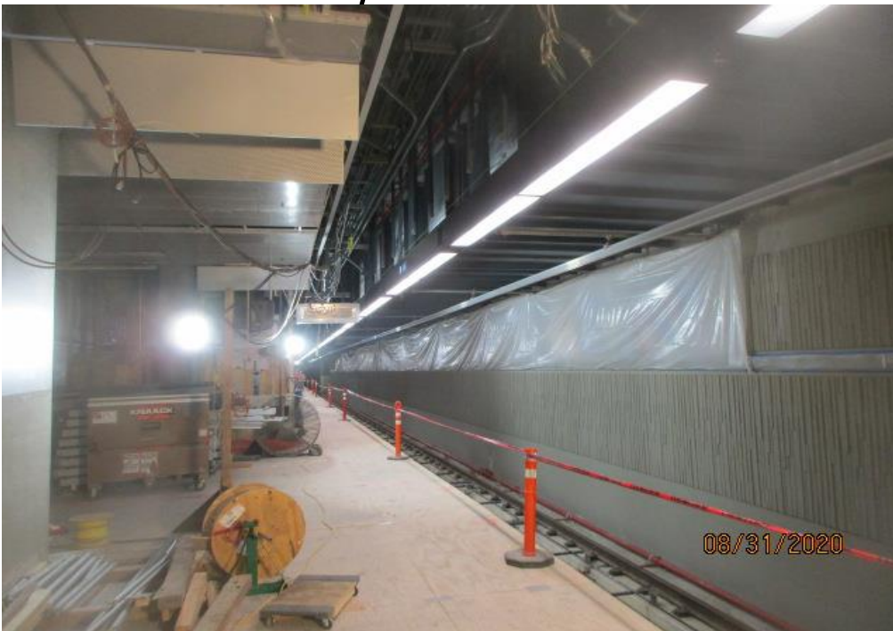
LEIMERT PARK STATION – Continue installing edge lights to the down stand support poles on the northbound side and tested lighting for the southbound at the platform level.
