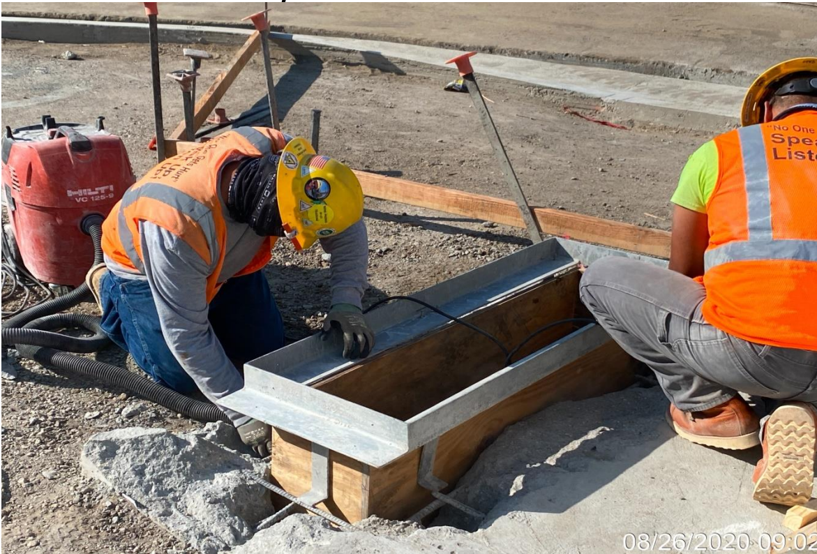
Crenshaw/Vernon – WSCC forming up Methane vent at Vernon plaza
