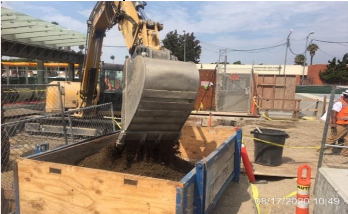
EXPO STATION SITE – WSCC crew excavating trench for electrical conduit.
