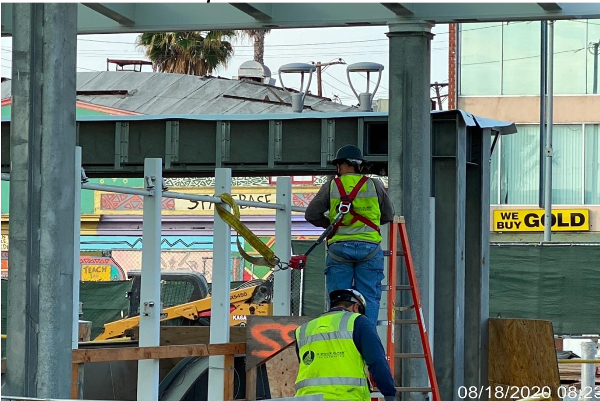
Crenshaw/Vernon – Giroux installing glass for entry structure Vernon.
