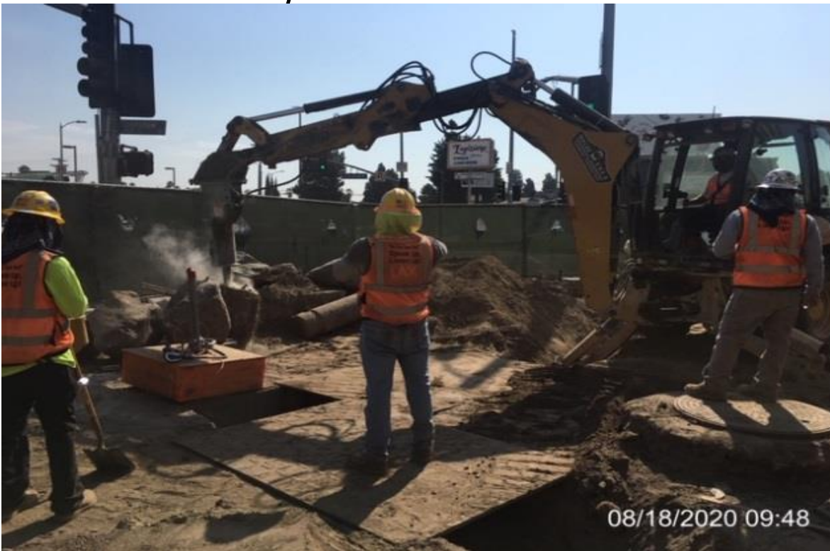
MLK STATION – WSCC crew demoing and removing concrete from walkway.
