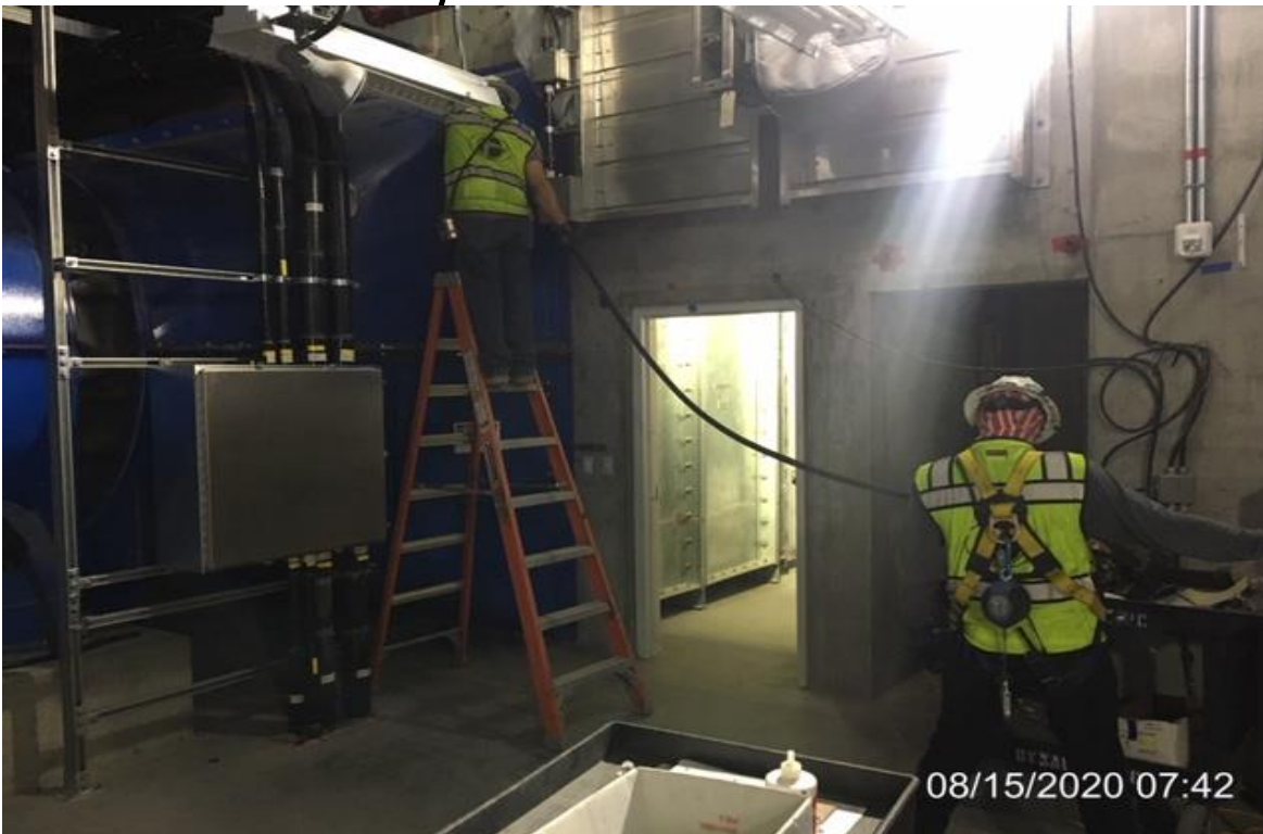
MLK STATION – LKC pulling Radiax cable and installing clicks.
