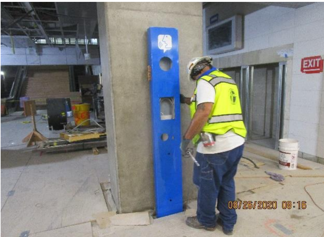
LEIMERT PARK STATION – Anchoring ETEL/PTEL podium enclosures at the concourse level.
