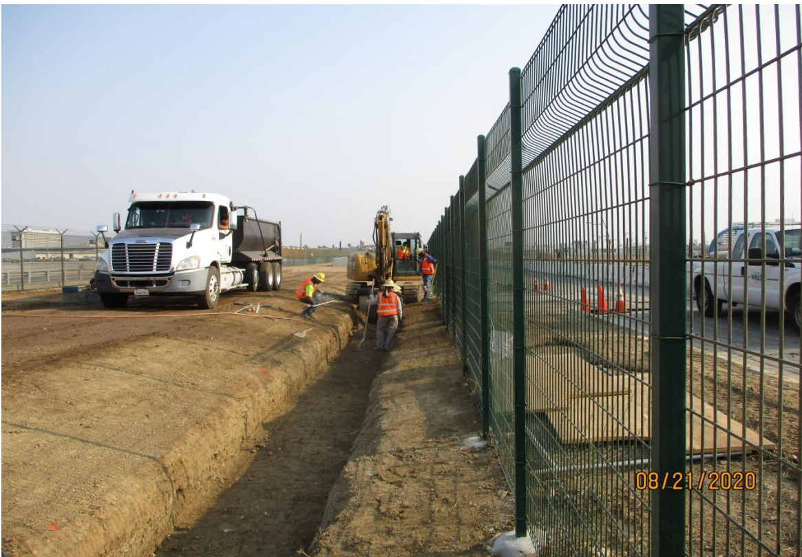
UG1- Drainage swale and amended soil grading at UG-1.
