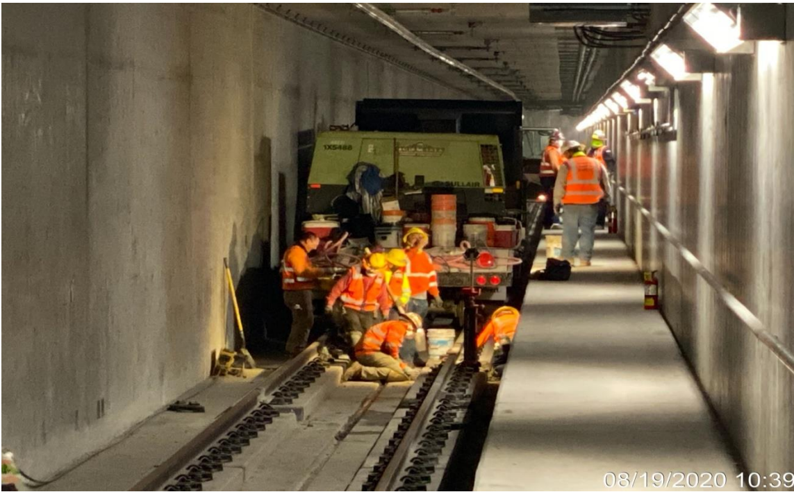
UG3 – WSCC working on plinths northbound UG-3.
