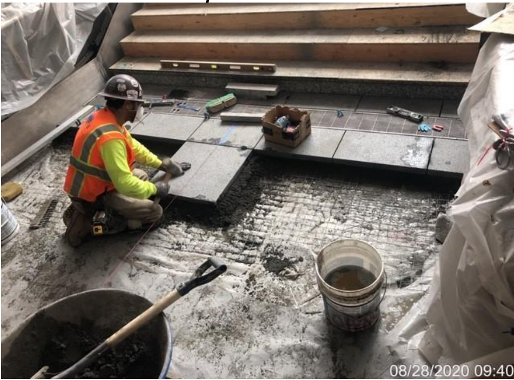
MLK STATION – Installing granite pavers to the bottom landing of Staircase 1
