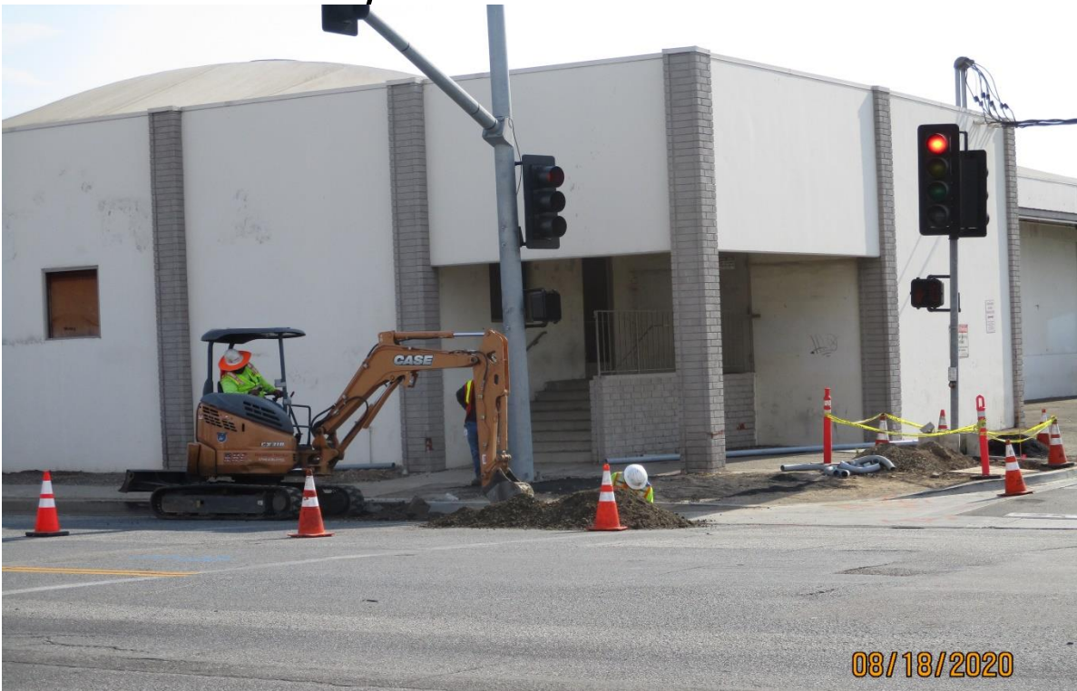
AVIATION/CENTURY- Trenching for traffic signal conduit at 104th and Aviation.
