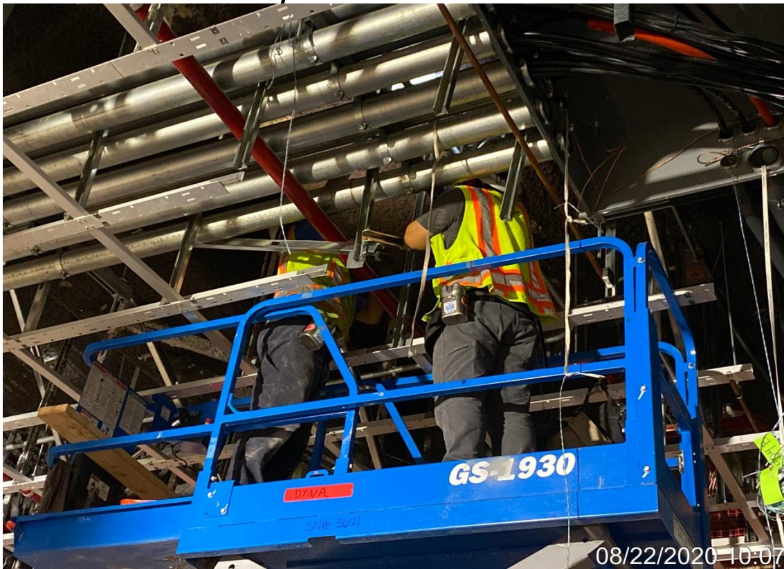
MLK STATION – Dynalectric measuring for Seismic Racks MLK.
