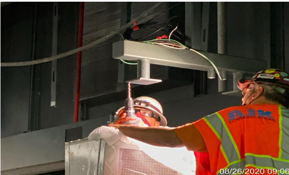
Crenshaw/Vernon – AJK installing LCD monitors at Vernon platform.
