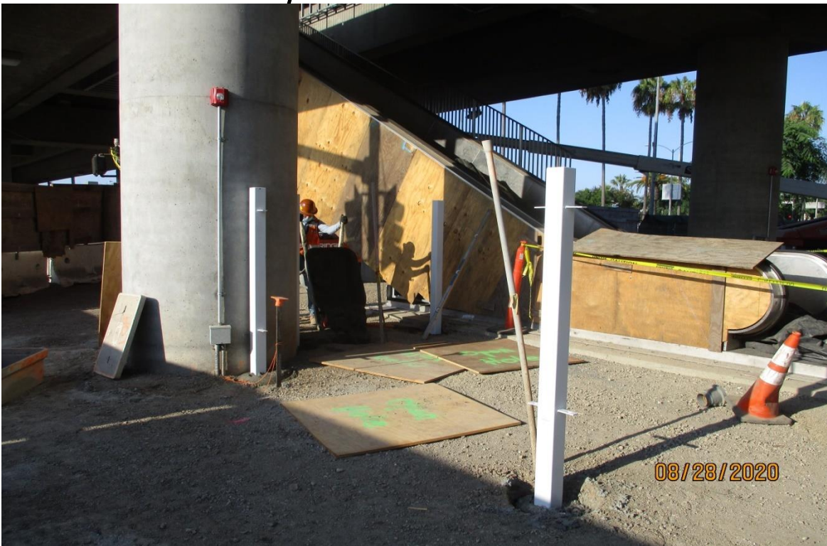
AVIATION/CENTURY- Placing concrete for the fence posts at the Aviation Station.
