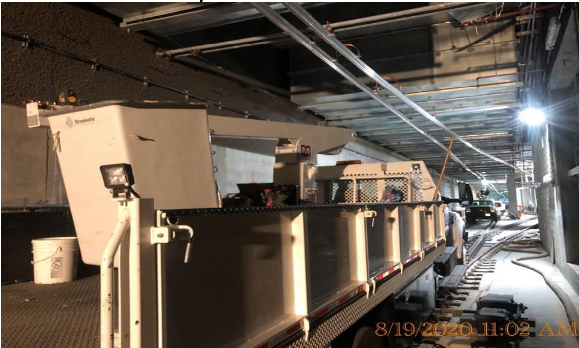
EXPO STATION – Continue installing supports and fixtures for the crossover lighting at the invert level
