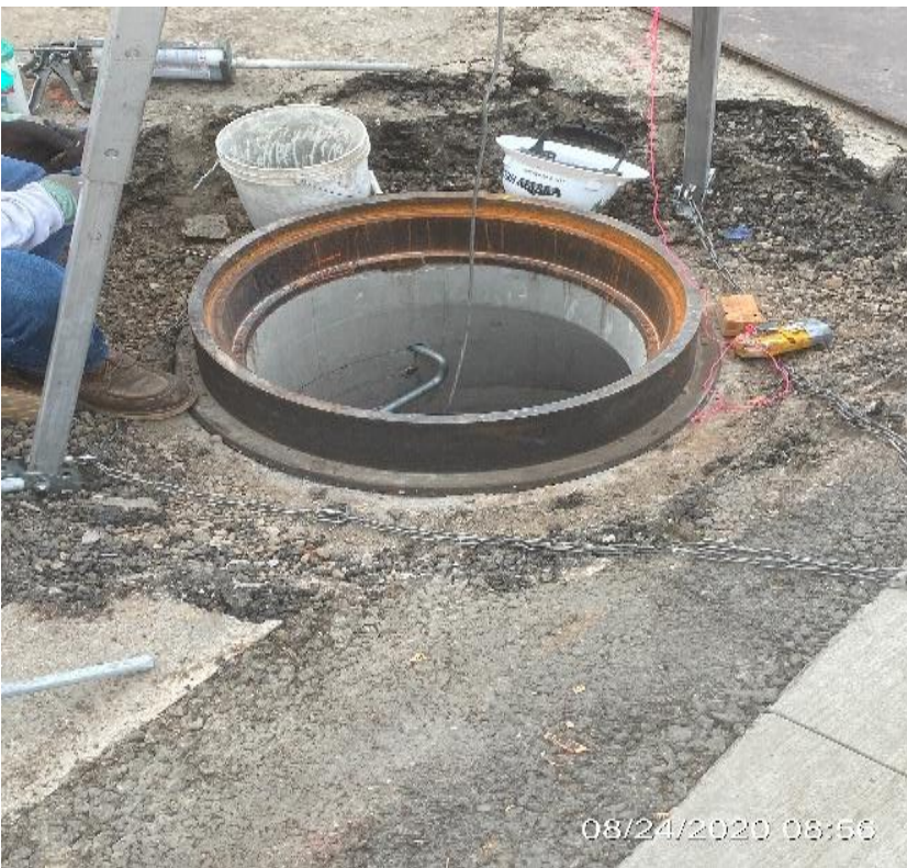
MLK STATION – Installing steel steps inside Manhole #19 at the plaza level.
