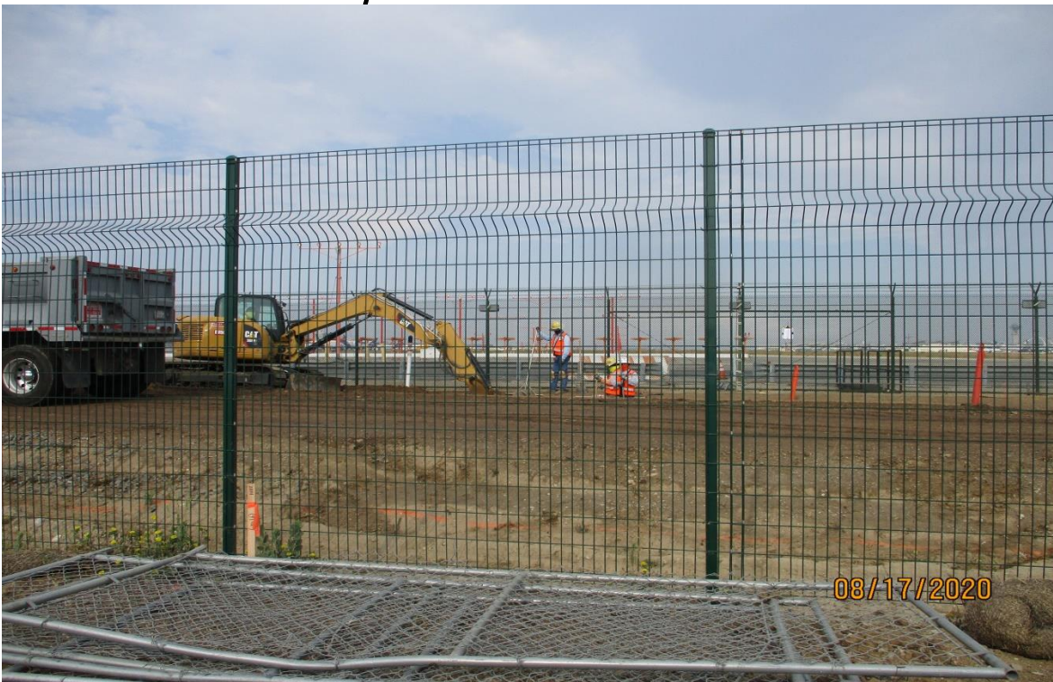
UG1- Drainage swale and amended soil grading at UG-1.
