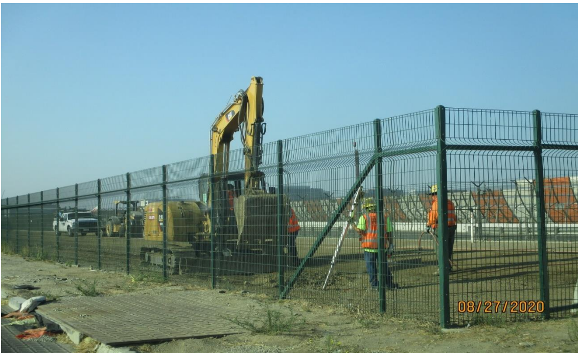
UG1- Drainage swale grading at UG-1.
