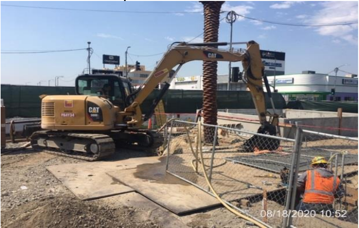
EXPO STATION SITE – WSCC crew excavating trench for AT&T conduit.
