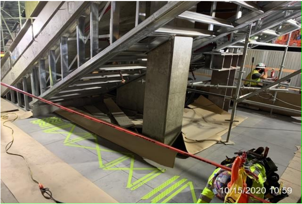
EXPO STATION– WSCC carpenter scanning platform slab for safety barrier install.
