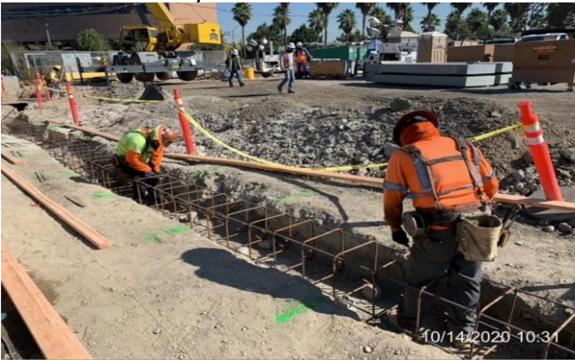
EXPO STATION – IRP installing rebar for bollard footing.
