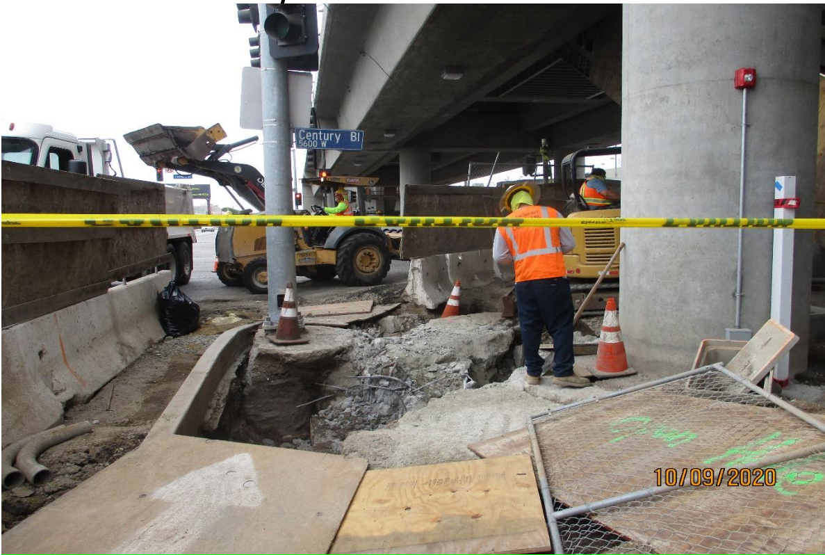
AVIATION/CENTURY- Concrete construction removal at Aviation and Century.
