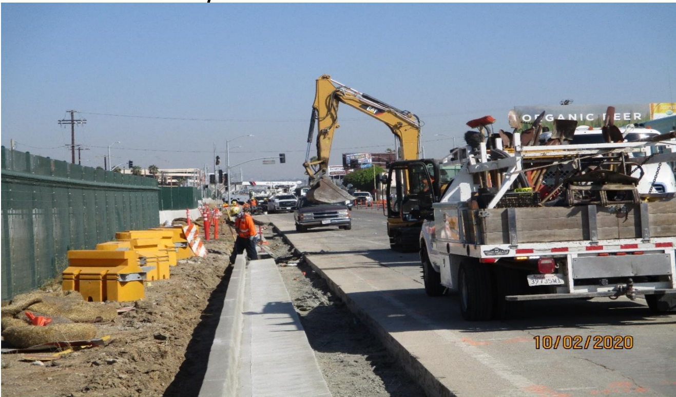
AVIATION/CENTURY- Curb and gutter removal on Aviation.
