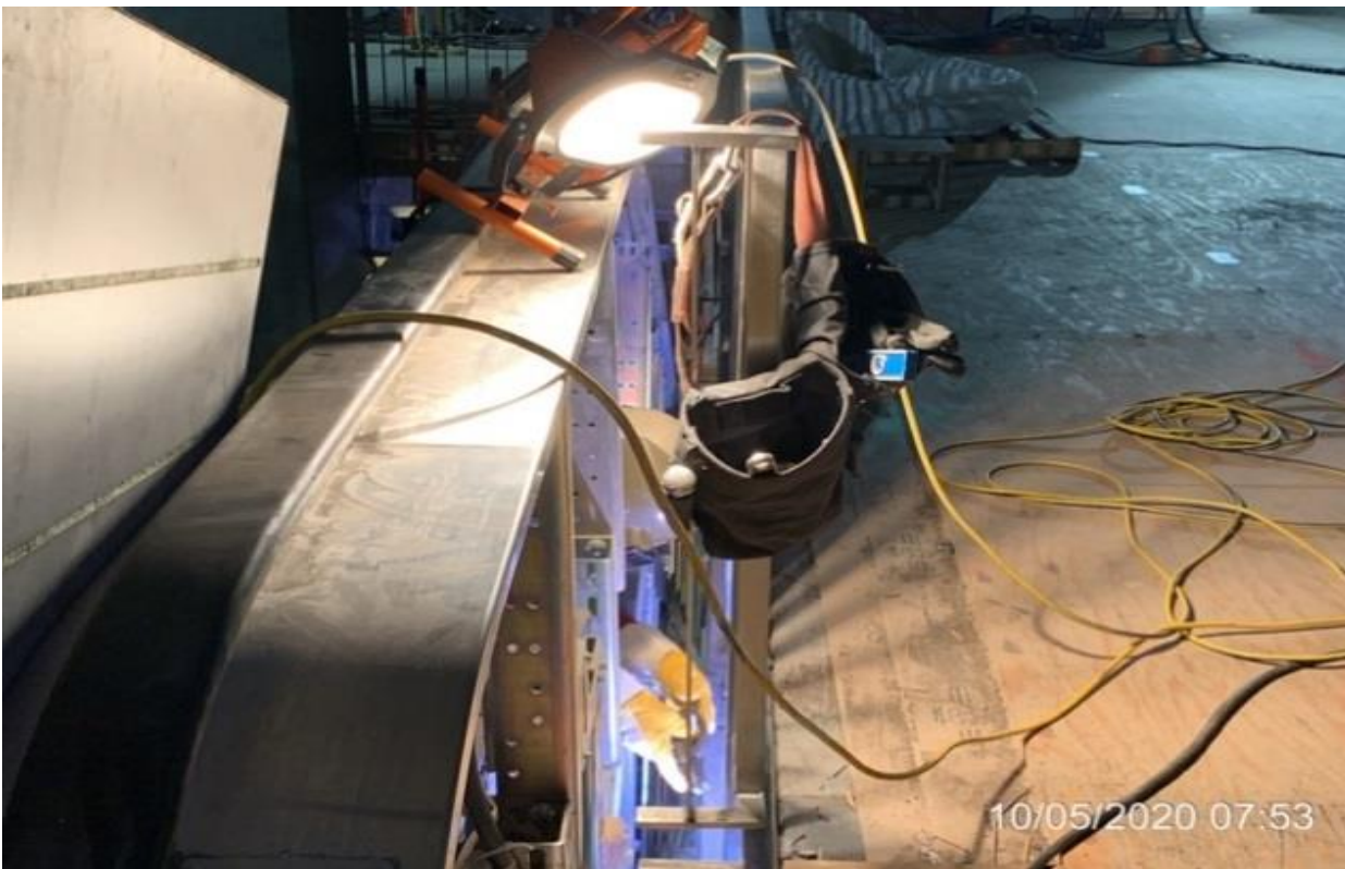
MLK STATION – McMahon cosmetic welding and grinding at stair #3.
