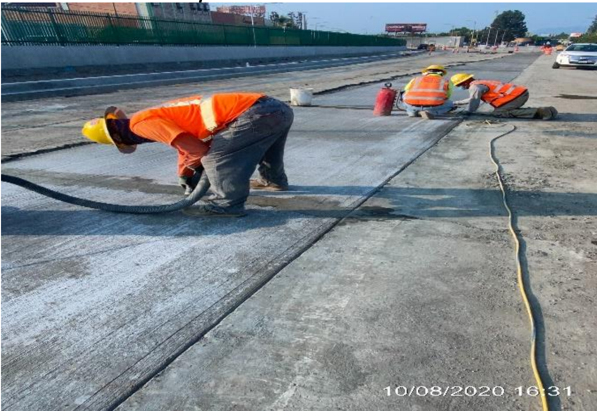
PARK MESA – Saw cutting the northbound lanes on Crenshaw Blvd from 48th St to 46th St.
