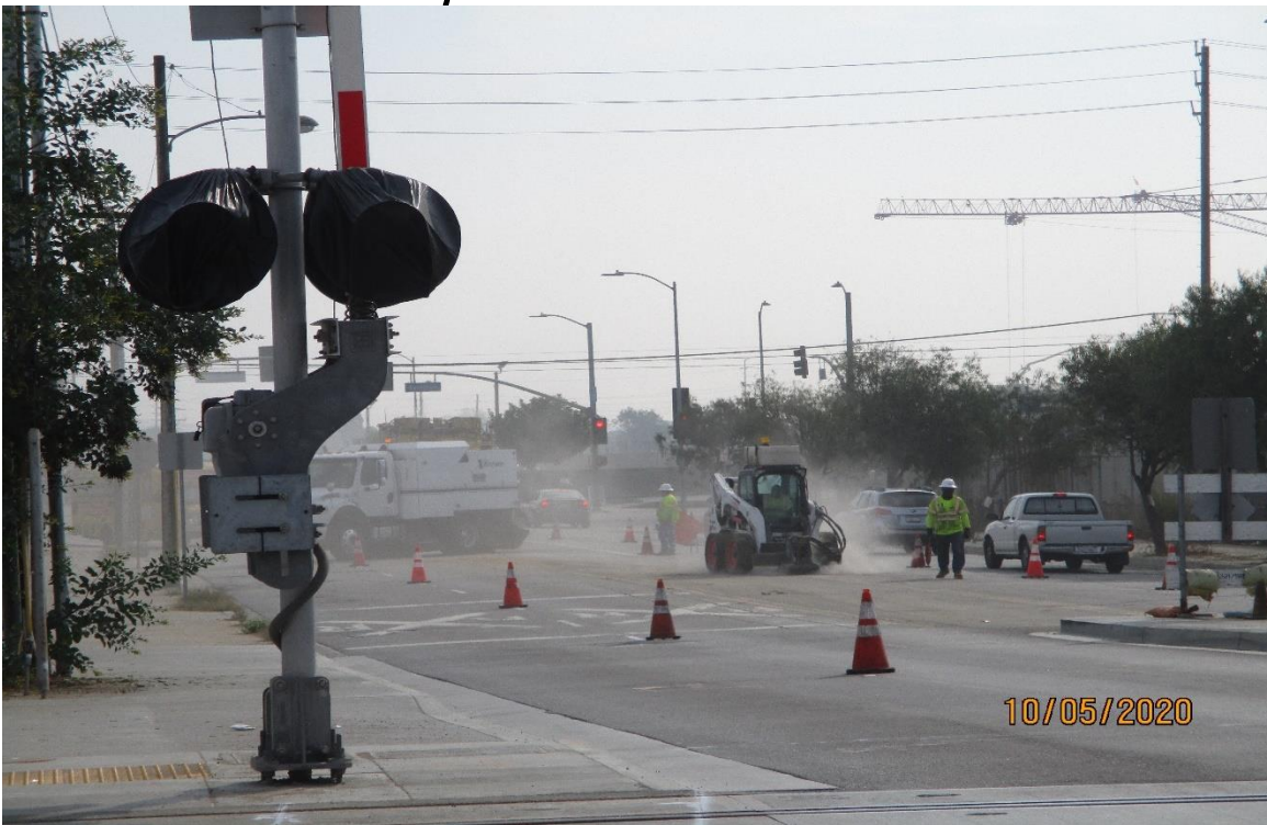
Arbor Vitae- Grinding off the temporary stripping on Arbor Vitae.
