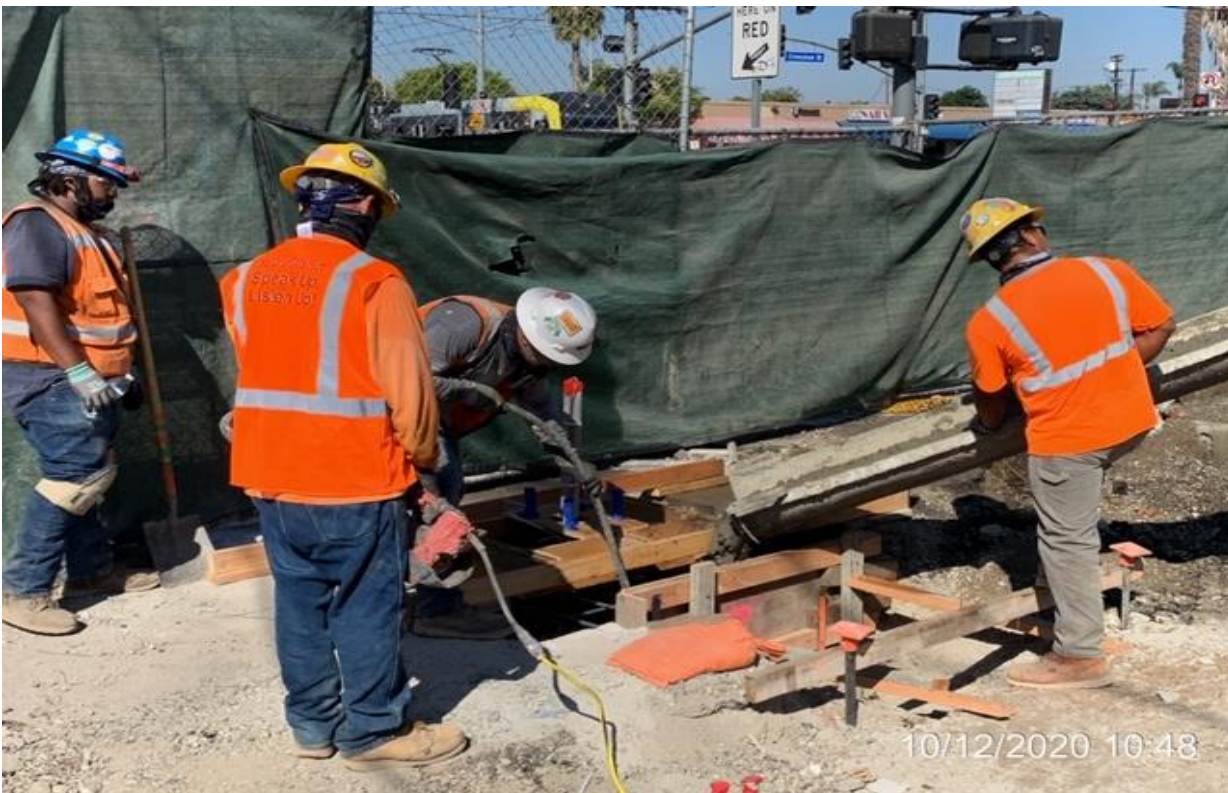
EXPO STATION – WSCC crew placing concrete footing for grand pylon signage
