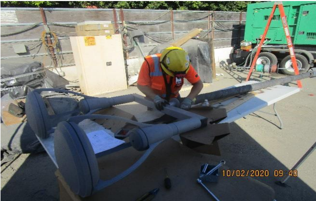
MLK STATION – Assembling pedestrian light poles for the plaza level.
