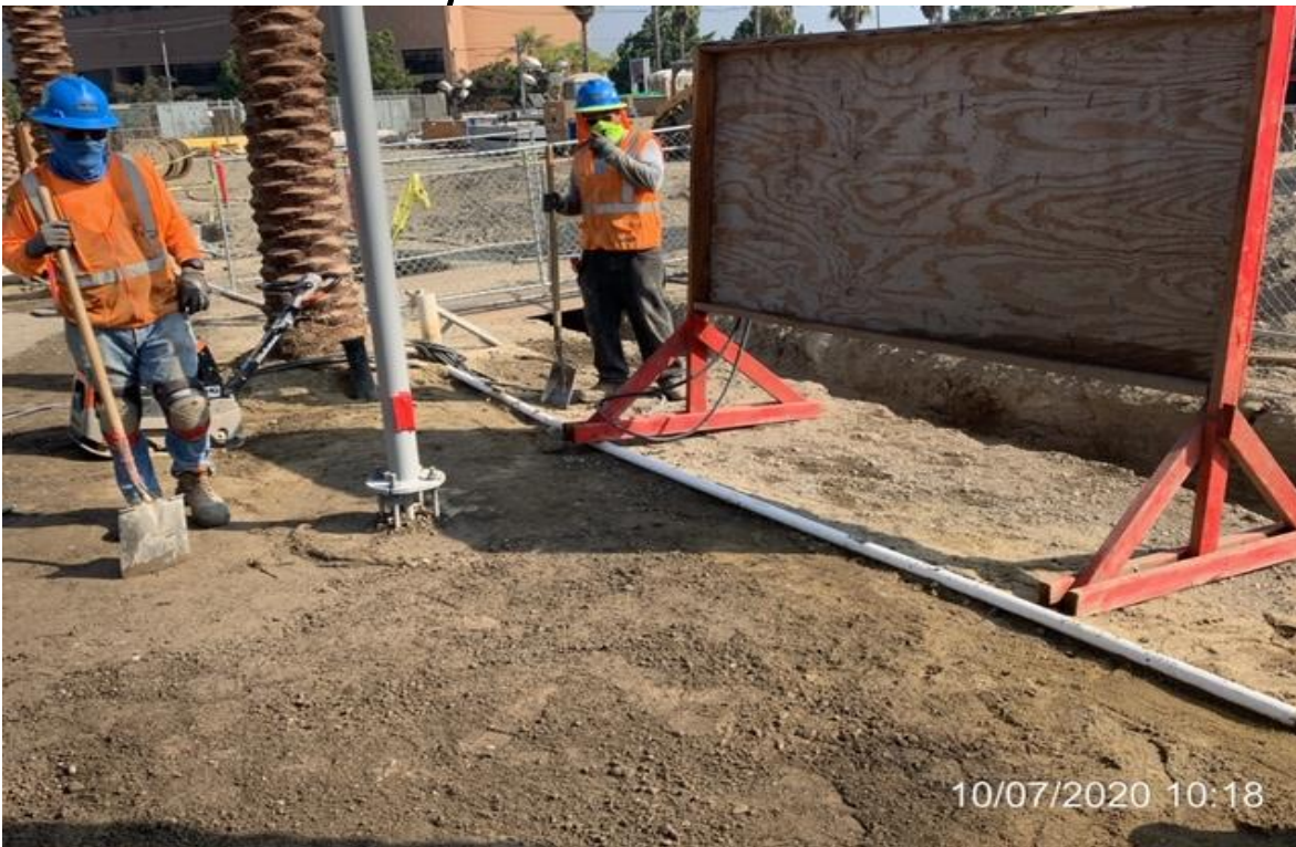
EXPO STATION– WSCC grading and compacting south end.
