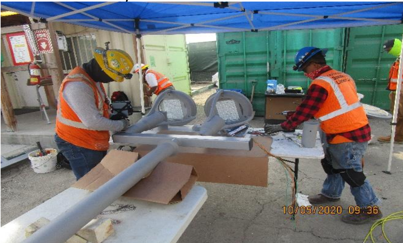
MLK STATION – Continue assembling pedestrian light poles for the plaza level.
