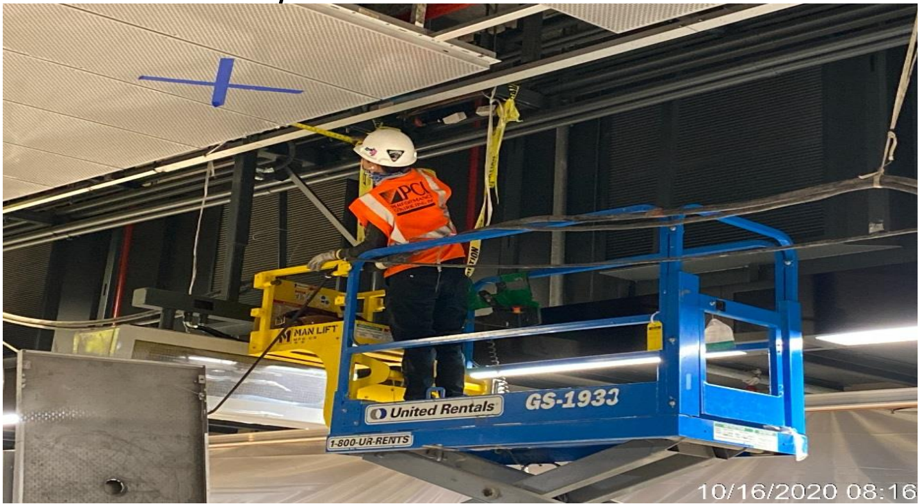
LEIMERT PARK STATION – Continue ceiling panel installation throughout the platform level.
