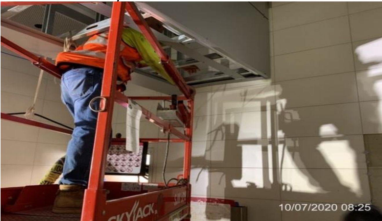
MLK STATION – WSCC ironworkers installing ambient noise sensors
