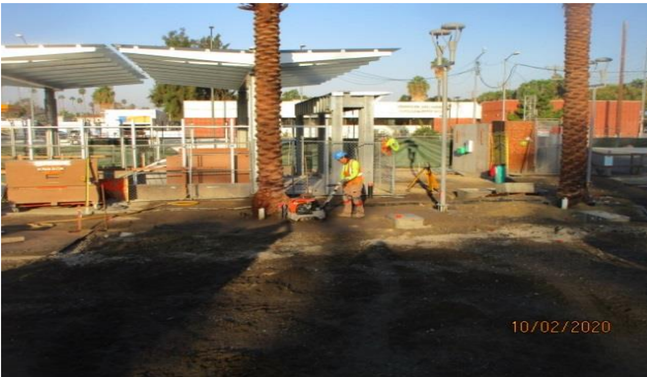
EXPO STATION SITE– Continue rough grading/compacting throughout the plaza.
