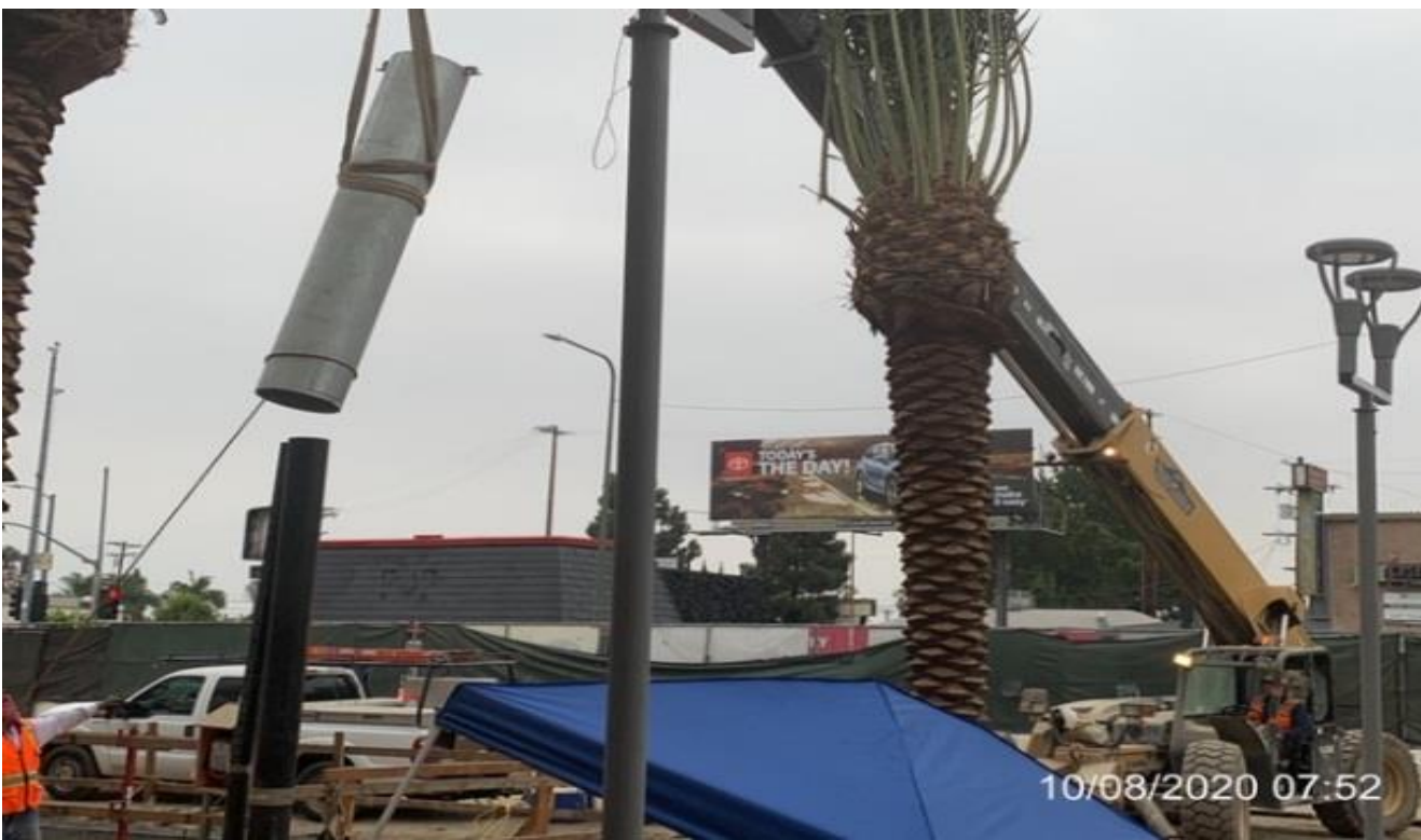
MLK STATION – WSCC ironworkers installing metal sleeve over vent stack.
