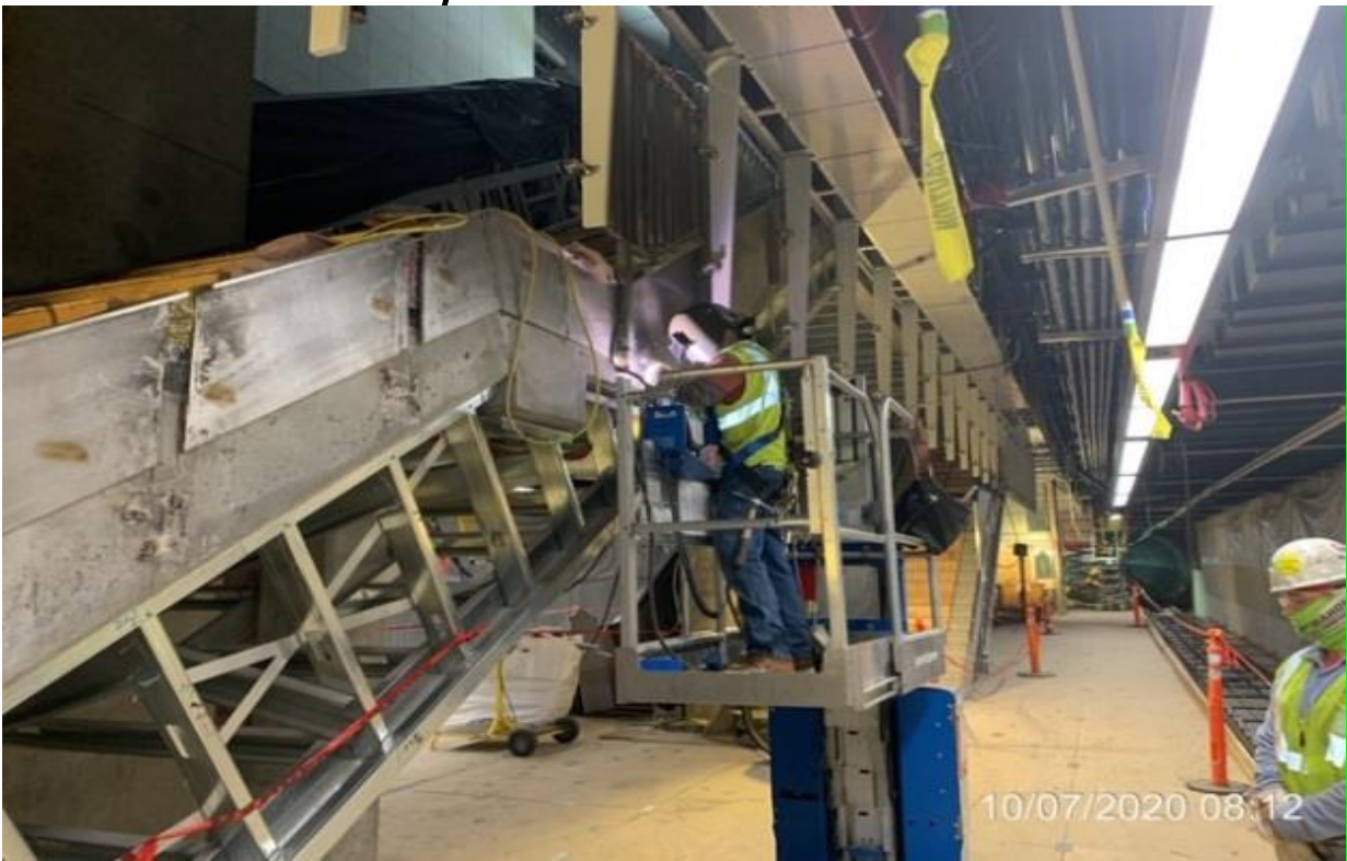
MLK STATION – McMahon cosmetic welding and grinding escalator #2.
