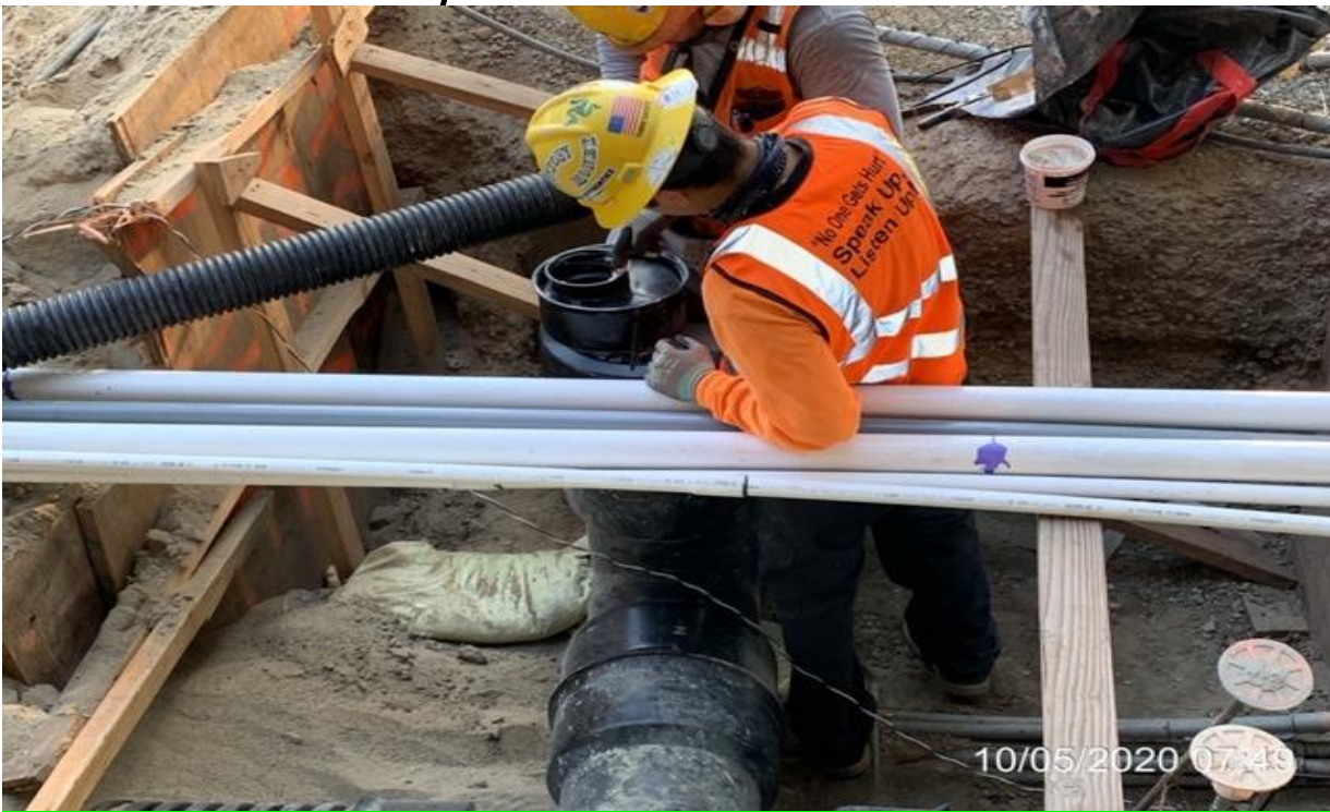
MLK STATION – WSCC crew making PVC connections for storm drain.
