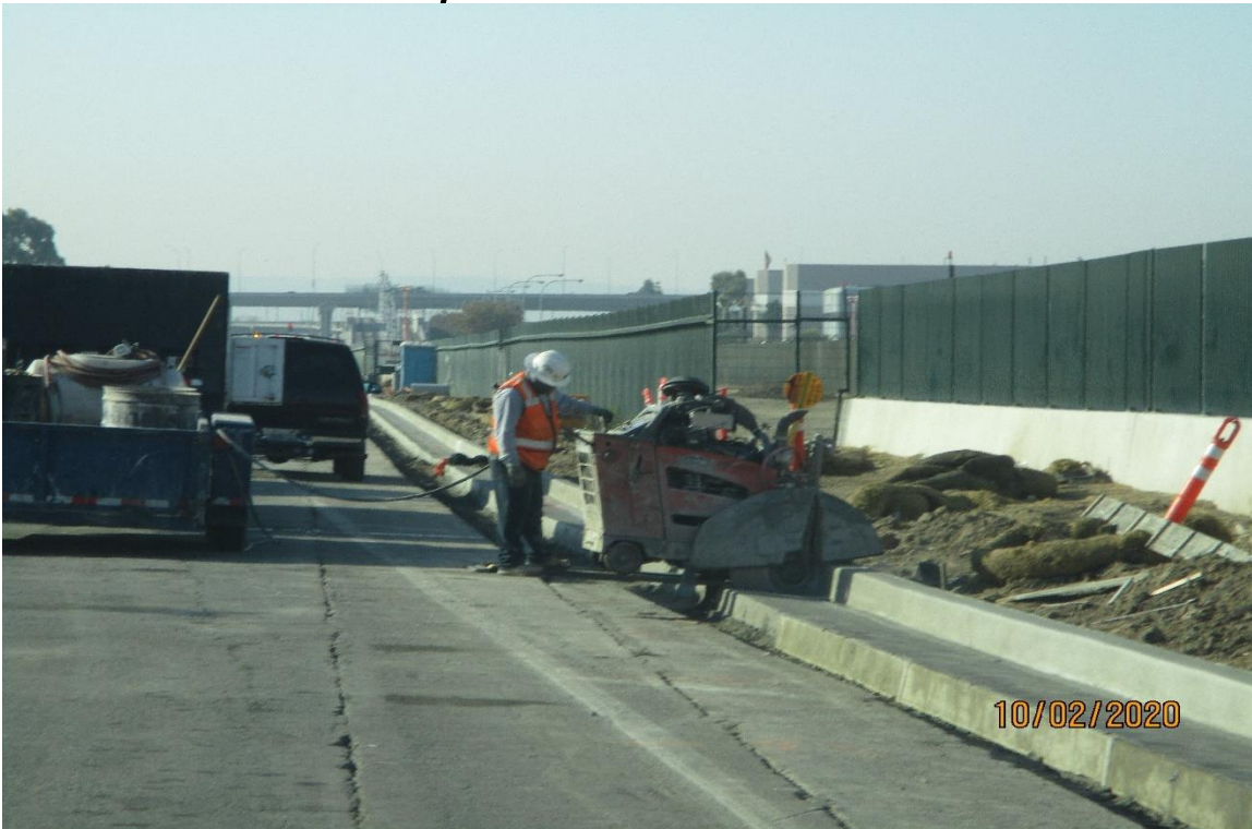
AVIATION/CENTURY - Saw cutting to remove some curb and gutter on Aviation.
