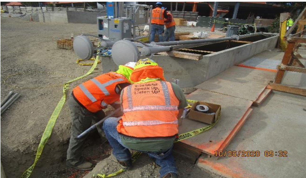
MLK STATION – Continue assembling pedestrian light poles for the plaza level.
