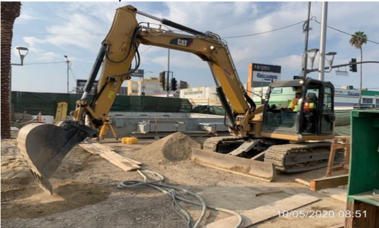
EXPO STATION – Continue rough grading/compacting throughout the plaza.
