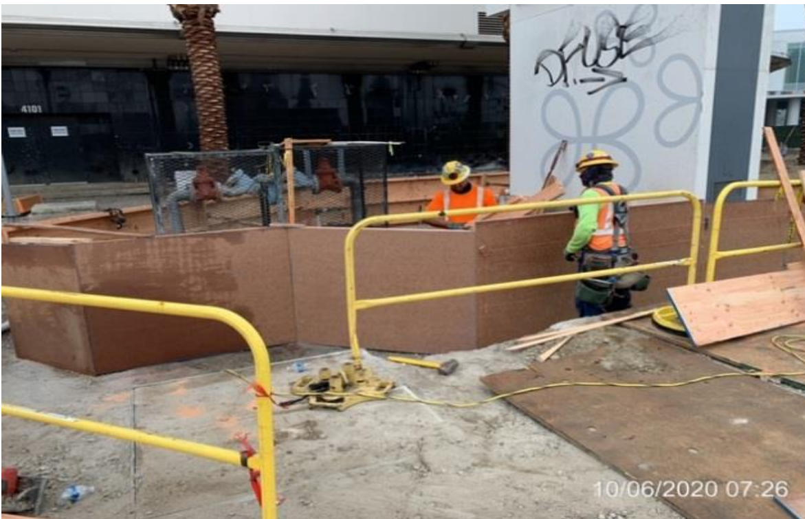
MLK STATION – WSCC carpenters building formwork for north end planter wall.
