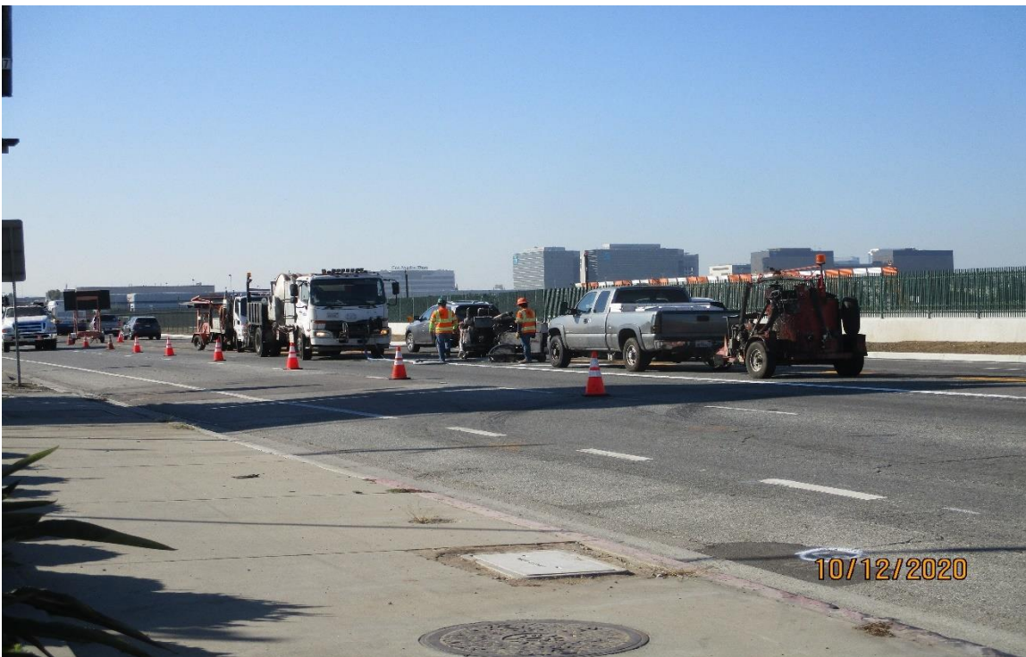
104 th street- Cutting vehicle detection loops on Aviation near 104th street.
