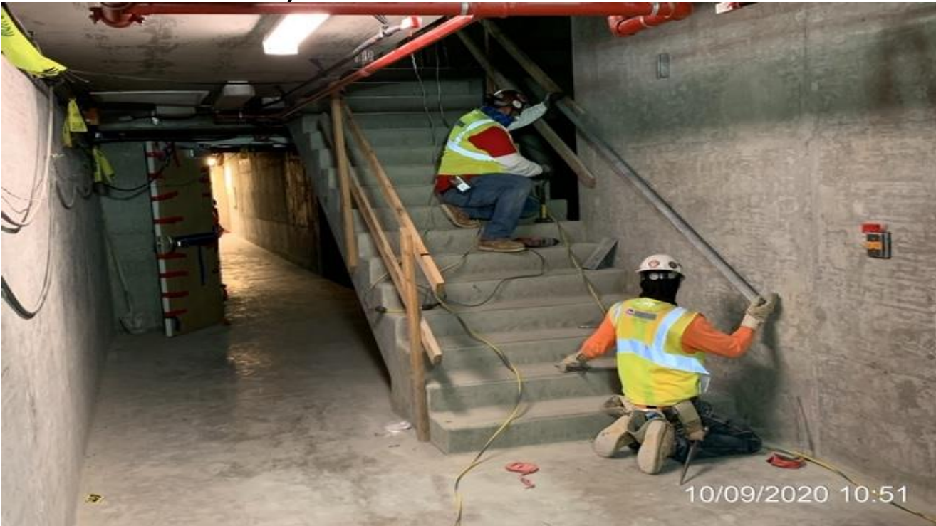
EXPO STATION – Continue installing galvanized handrails throughout Emergency Exit Stair South #2.
