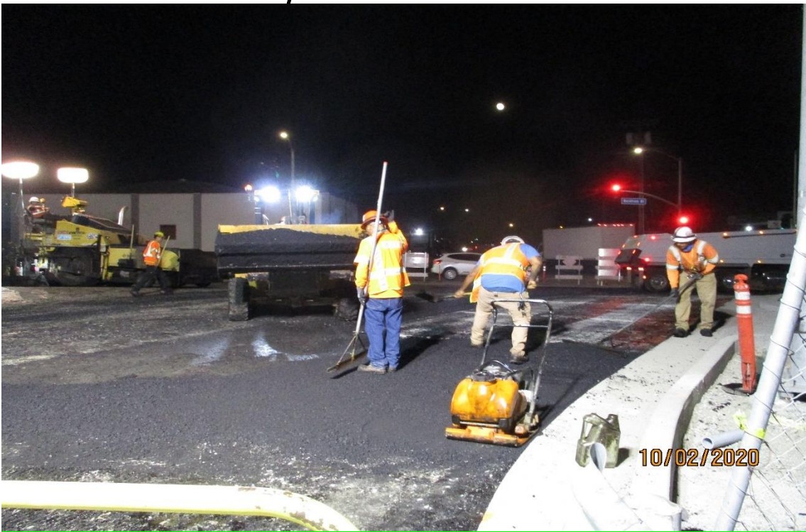
104 th street- Placing the base course of AC on 104th street.
