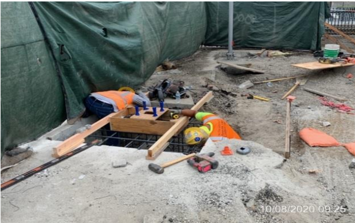
EXPO STATION – WSCC carpenters building formwork for grand pylon footing.
