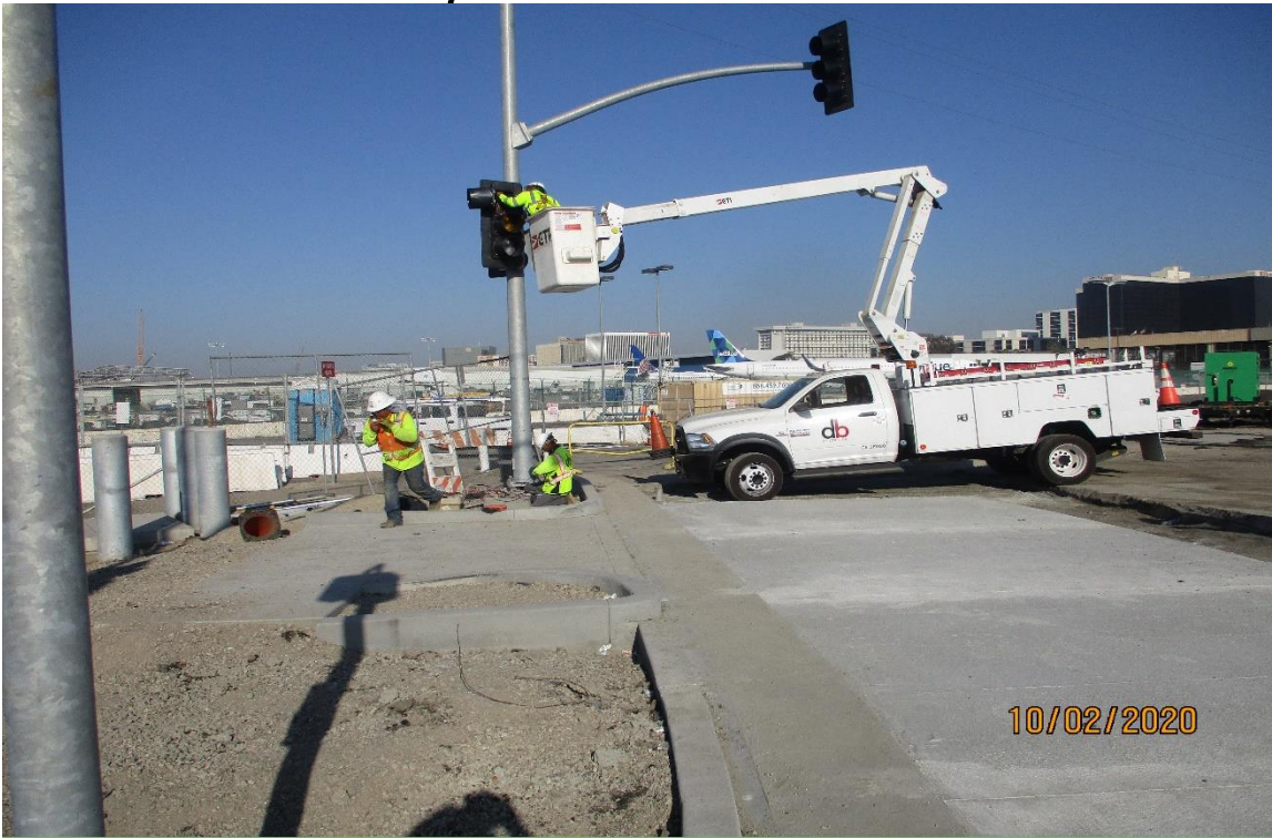
104 th street- Wiring the traffic signal lights at 104th street.
