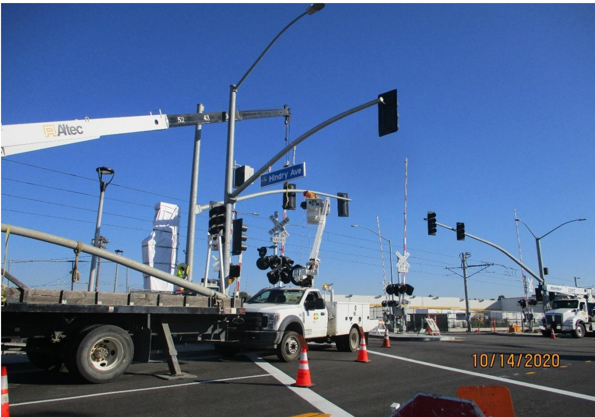
Hindry – Hanging a traffic signal mast arm at Hindry.
