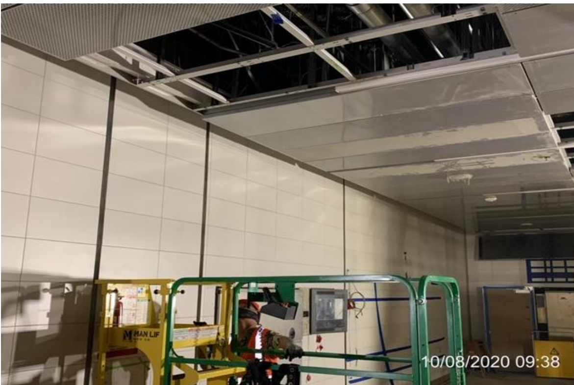
EXPO STATION – WSCC ironworkers installing ambient noise sensors.
