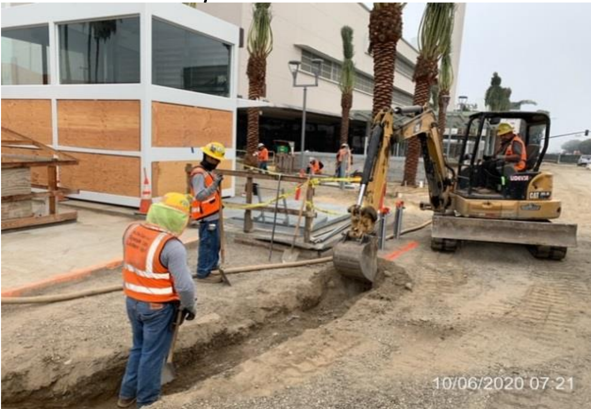
MLK STATION – crew excavating trench for CCTV conduit.
