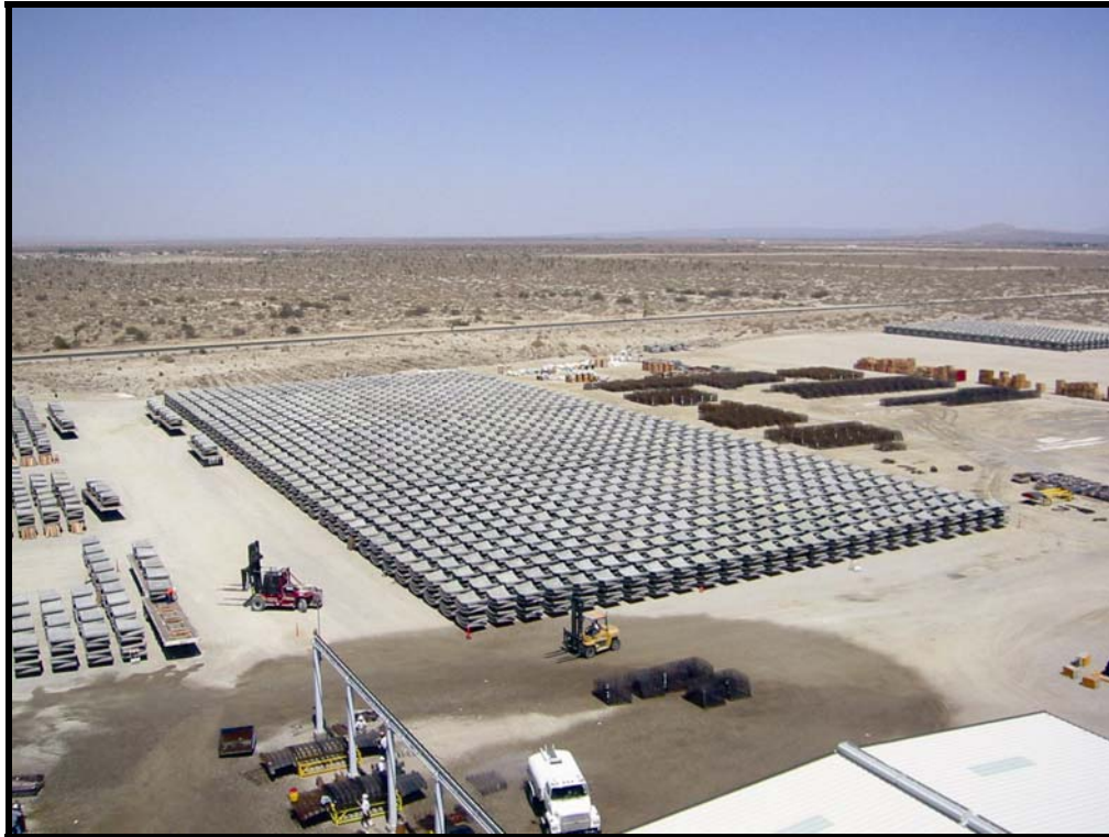
Figure 3-2 - TBM Segment Production Facility, Palmdale, CA
