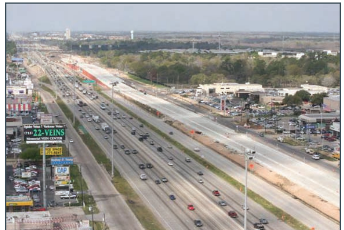
Figure 3.14 Frontage road construction
