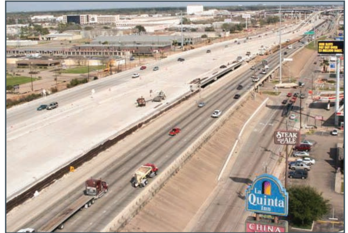
Figure 3.13 Mainline I-10 construction
