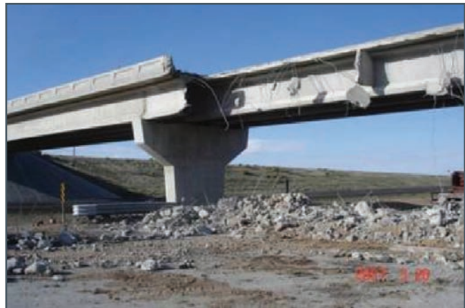
Figure 4.16 Damaged girder removed
