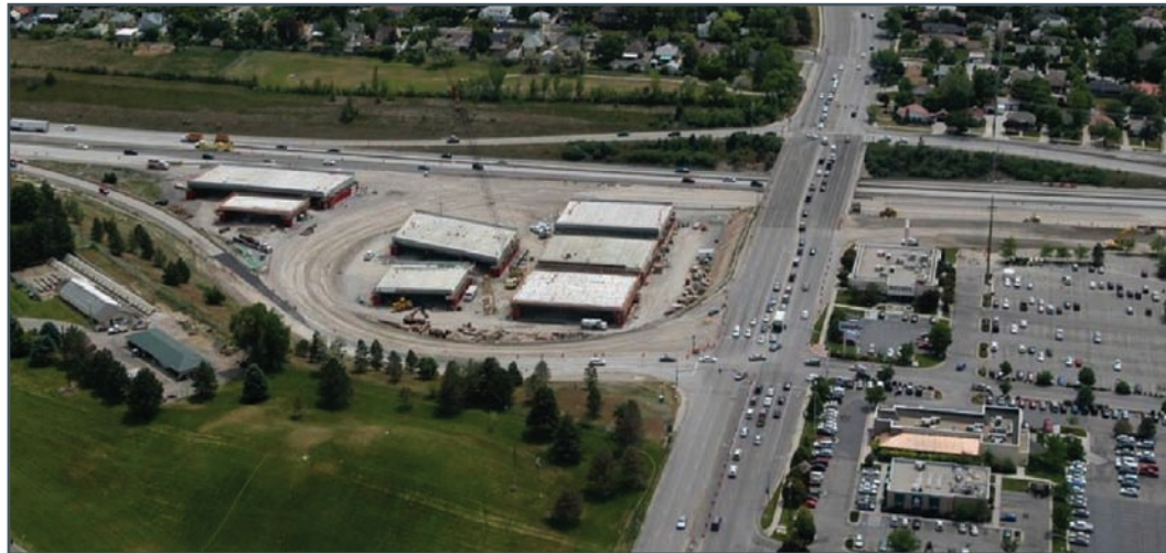
Figure 4.11 Bridge farm for the seven superstructures
