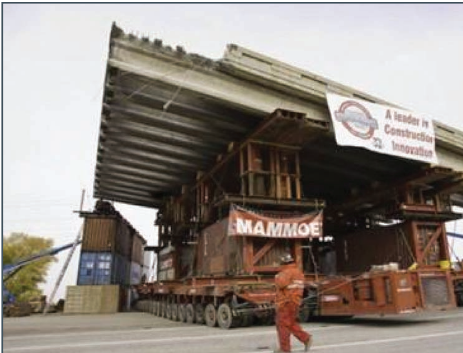
Figure 4.10 Moving existing superstructure to demolition area
