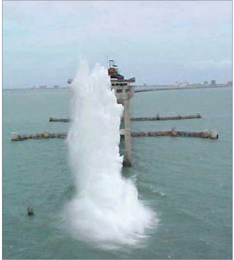
Figure 2.21 Demolition with blasting
