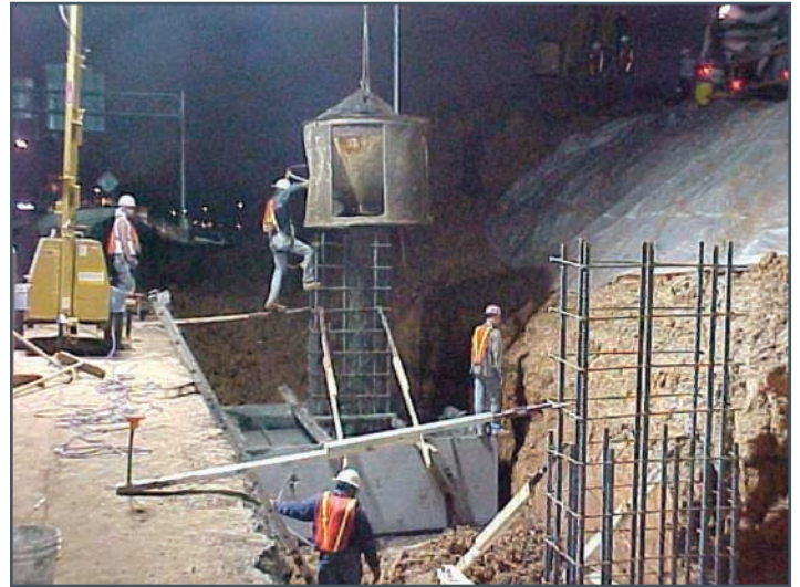
Figure 2.4 Using precast box culvert as forms
