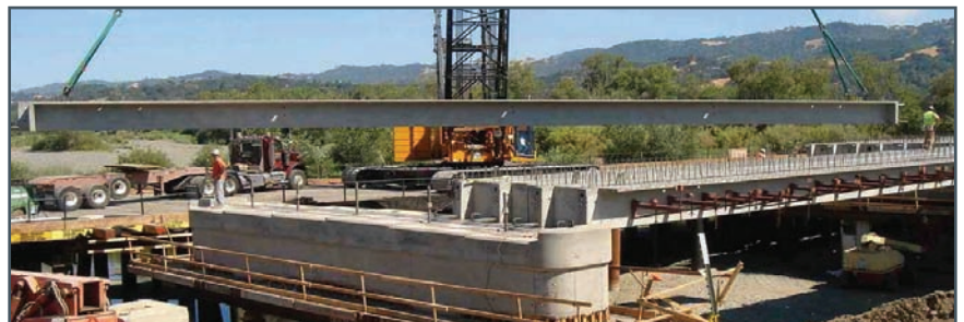
Figure 2.9 Installation of double-tee precast girders
