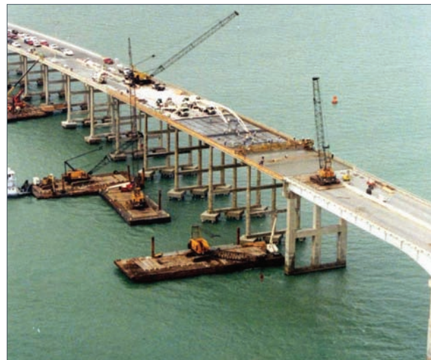
Figure 2.23 Last three spans poured on November 15
