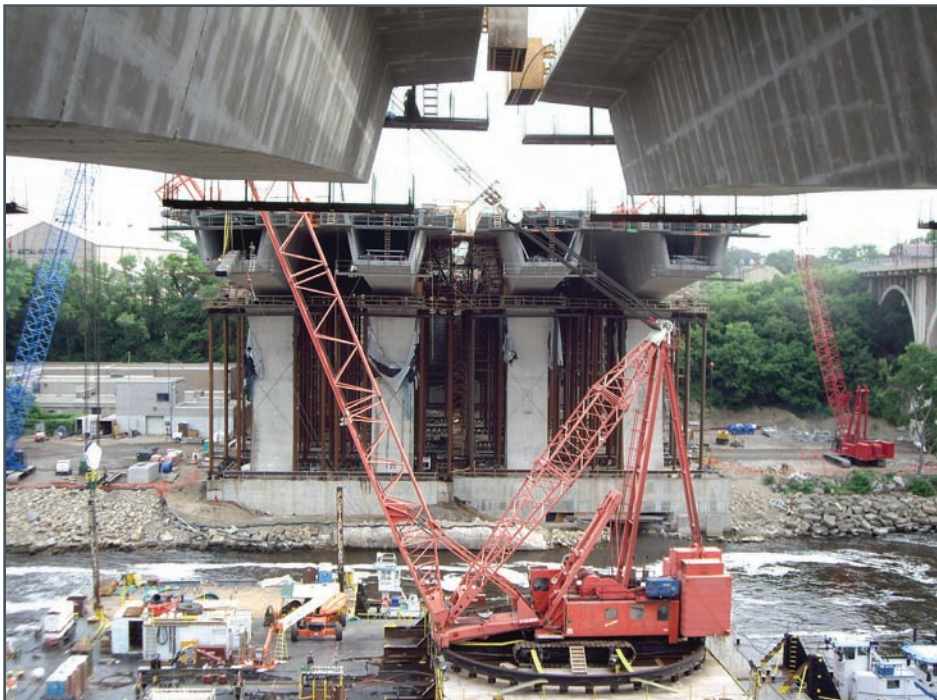
Figure 2.1 Construction of the I-35W Bridge in Minneapolis
