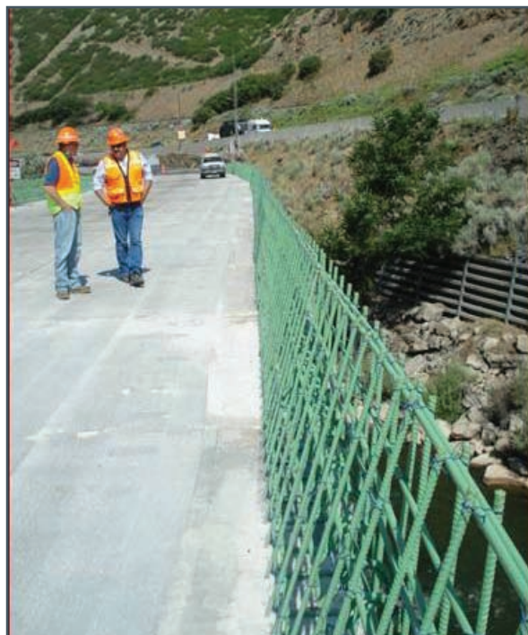
Figure 4.7 Weber Canyon precast deck panel project parapet
