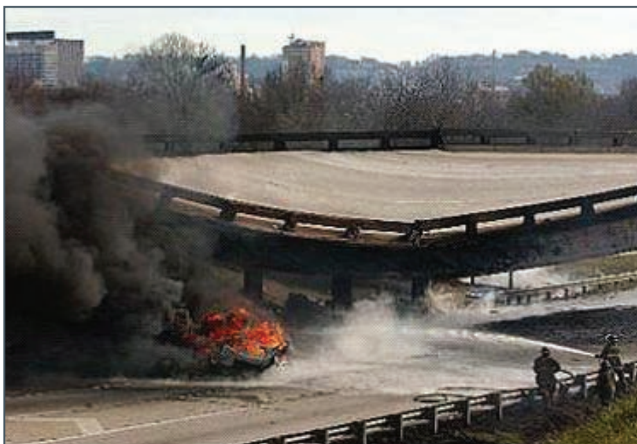
Figure 2.2 Gasoline tanker truck on fire under the bridge
