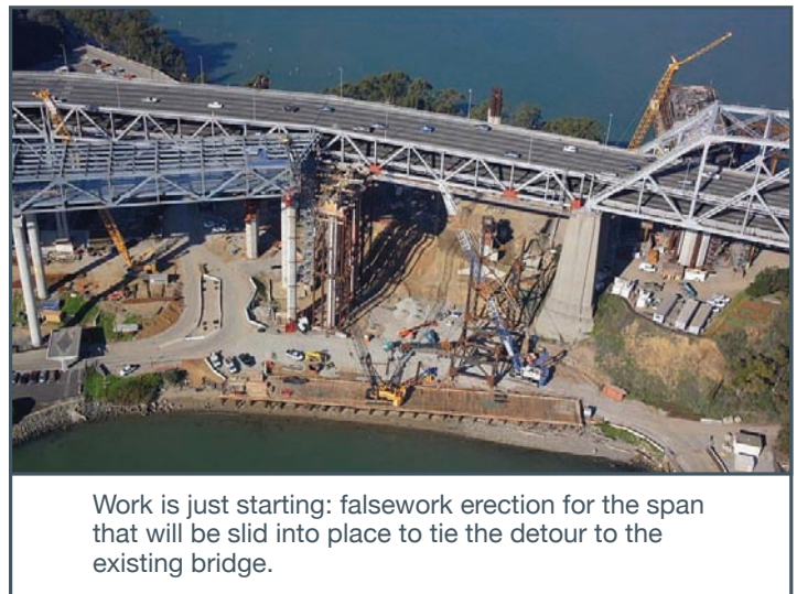
Figure 3.6 YBI detour construction
