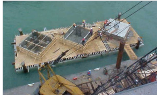
Figure 2.22 New footing construction at bent 30
