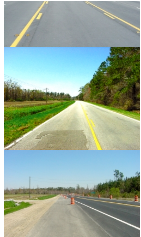
Figure 1: (left to right) McCray's Mill Road widened to a five lanes with curb and gutter section; Typical rural two-lane road that will be widened to a four-lane divided road; Typical rural two-lane road widened to a four-lane road with a striped median.
