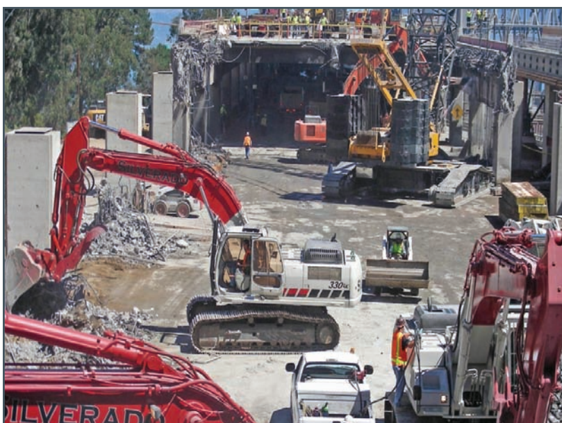
Figure 3.3 Demolition of the old YBI viaduct
