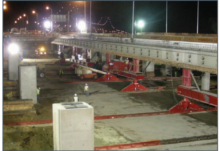
Figure 3.4 Roll-in of the new YBI viaduct
