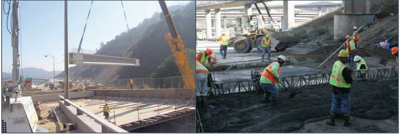
Figure 2.11 Setting girders and paving on the I-5 tunnel project
