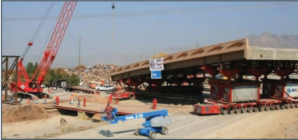
Figure 4.9 Staging area for new superstructure
