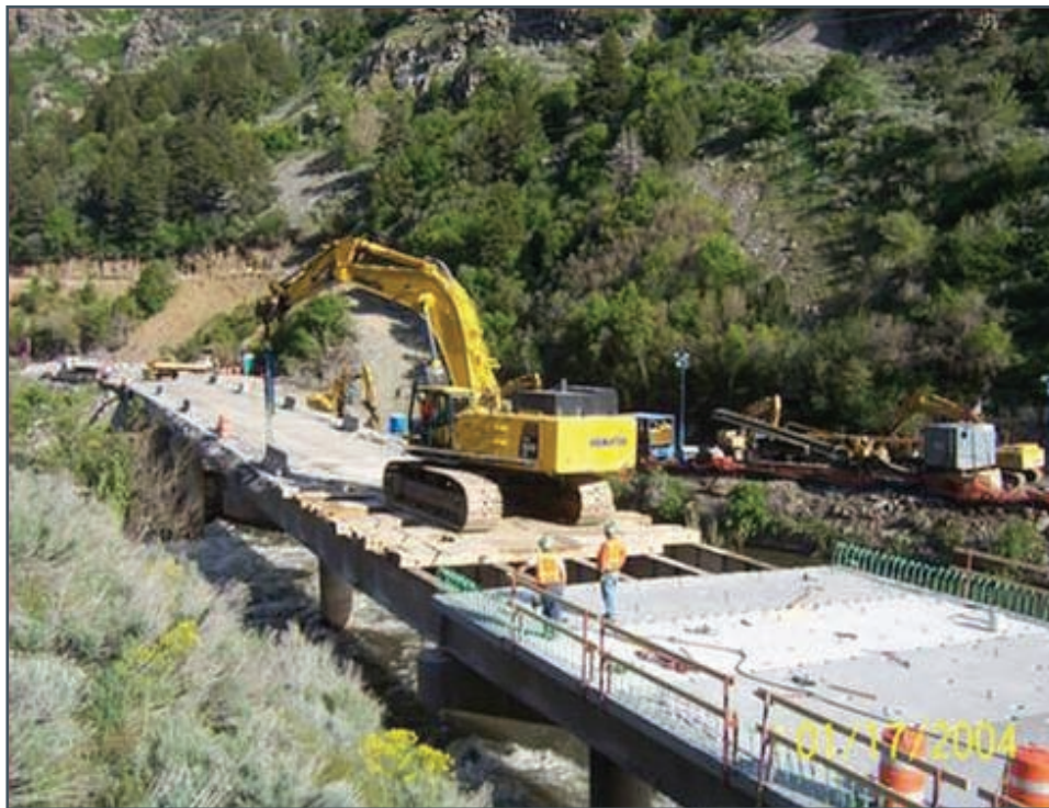
Figure 4.5 Weber Canyon precast deck panel project panel installation
