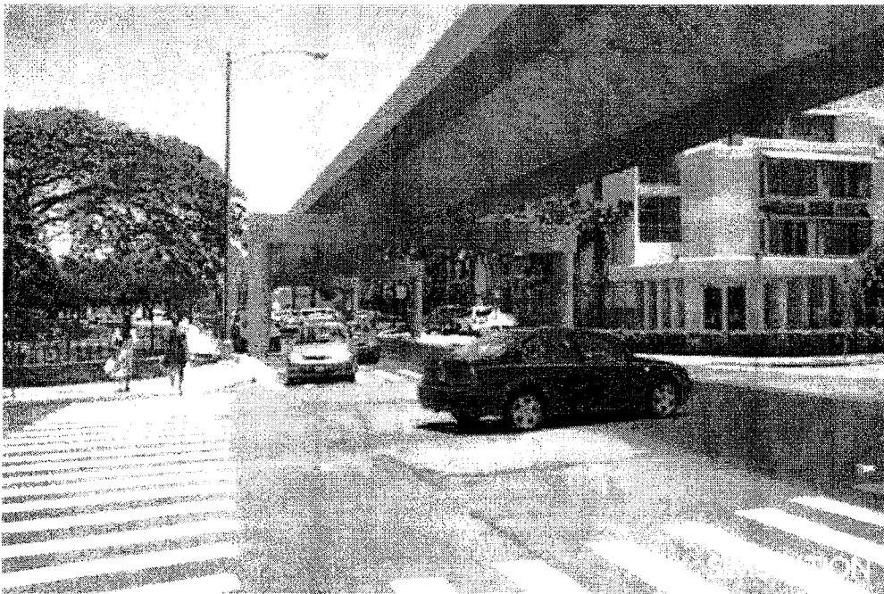
Straddle bent guideway and columns at Halekauwila Street/Cooke Street intersection
