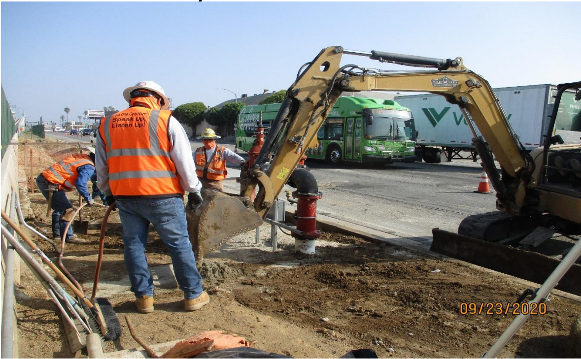
UG1- Drainage swale grading at UG-1.
