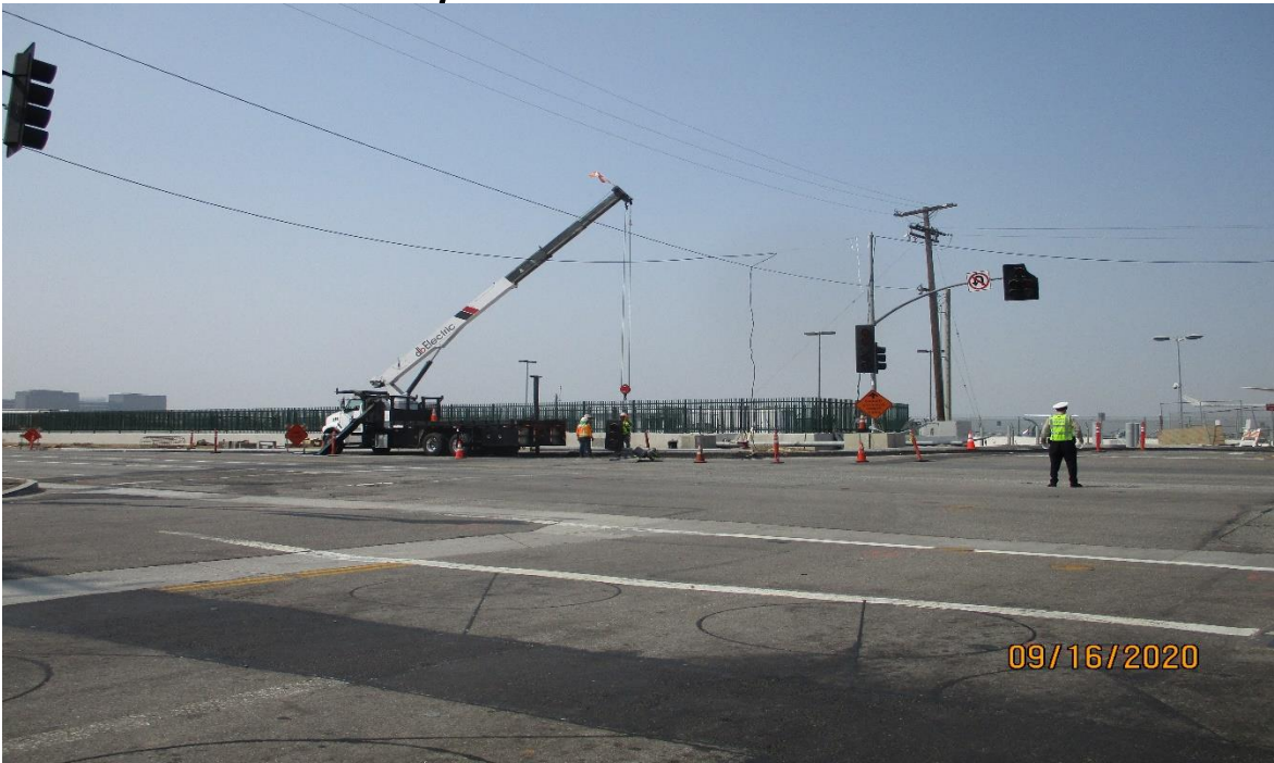
104 th street- Standing a traffic signal pole at 104th street.
