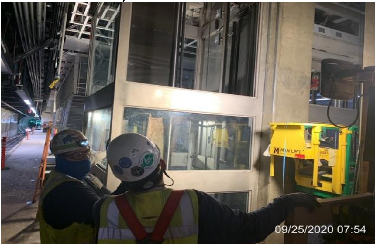
MLK STATION – Continue installing glass panels to Elevators 3&4 at platform level.
