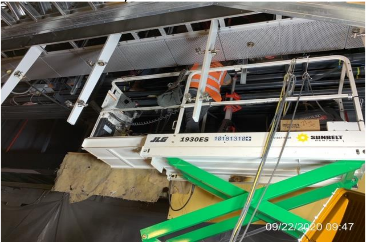
MLK STATION – WSCC ironworkers installing support arms for LCD at platform.
