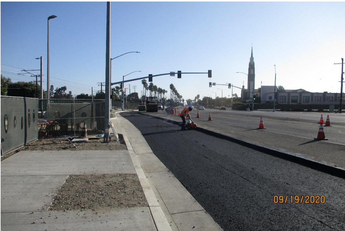
Hindry – Vibe plate compacting the AC on Florence.
