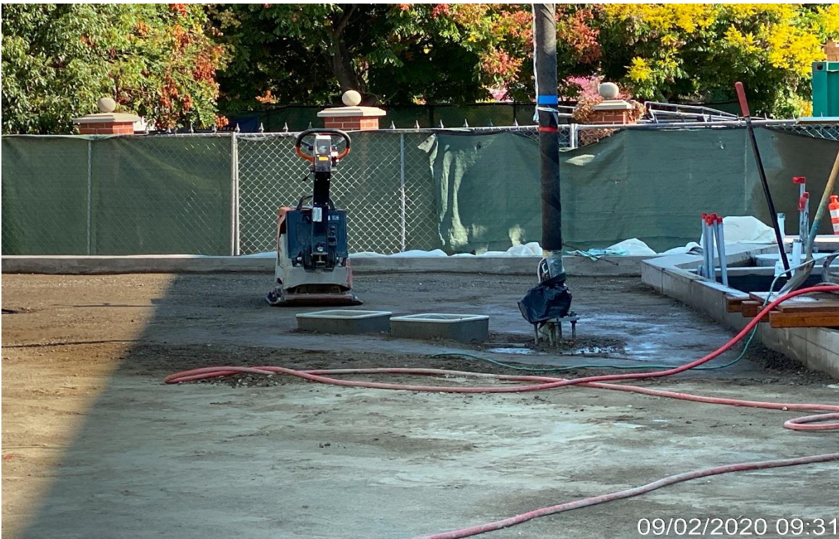
Crenshaw/Vernon – WSCC grading south end at Vernon plaza.
