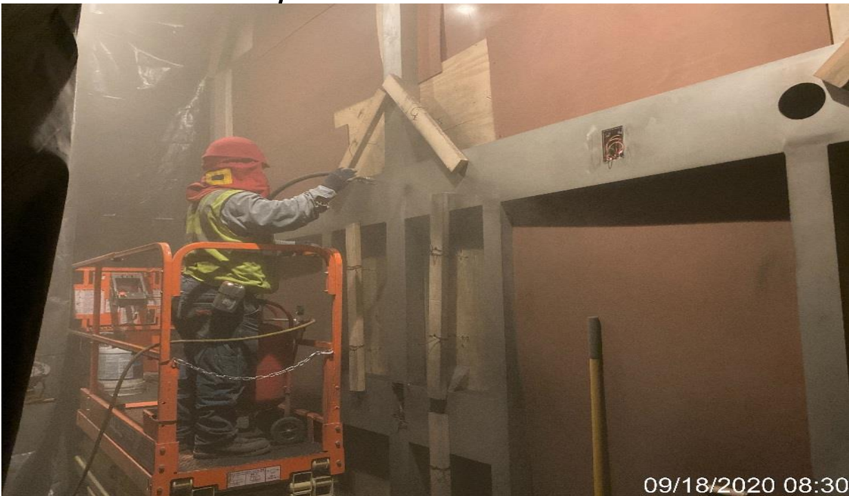
LEIMERT PARK STATION – Continue sand blasting Elevators 3&4 at the concourse level.
