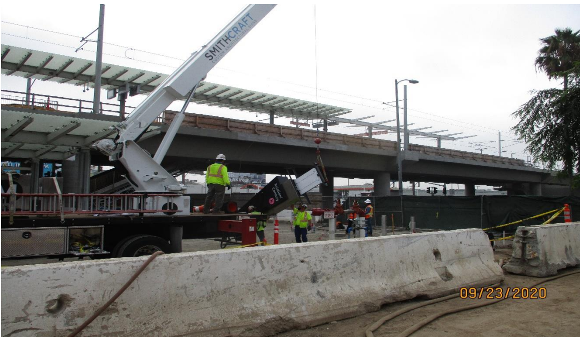
104 th street- Erecting the Grand Pylon sign at the Aviation Station.
