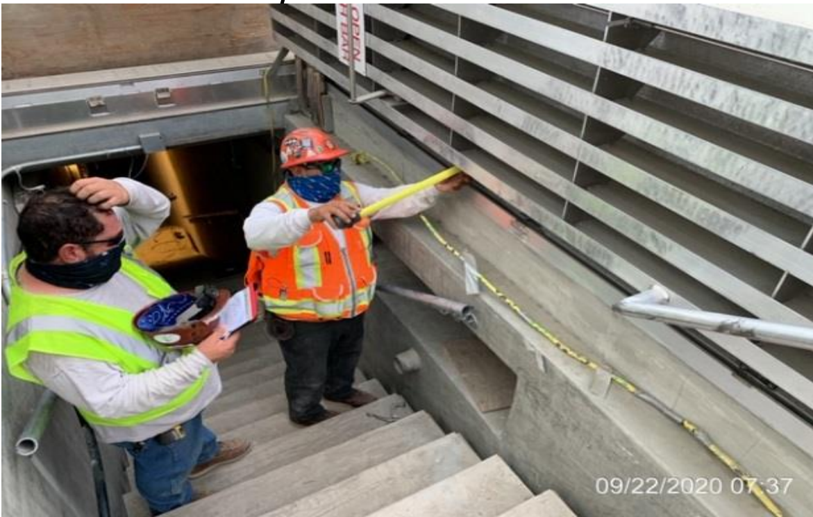
EXPO STATION – McMahon fabricating and installing galvanized handrail.
