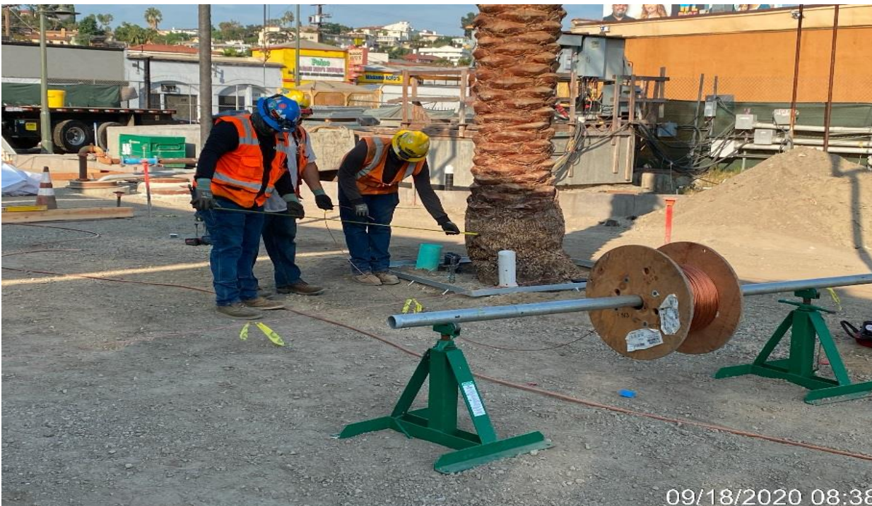
LEIMERT PARK STATION – Installing ground grid throughout the plaza level.
