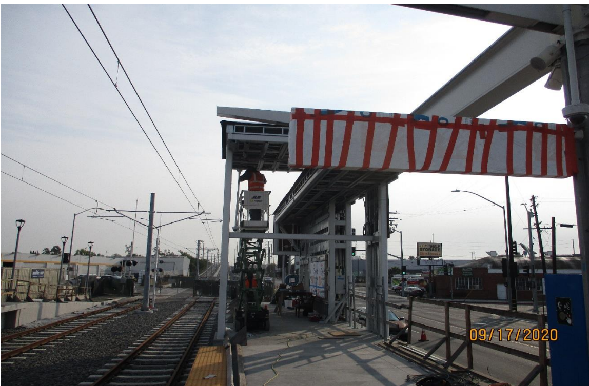
Hindry – Installing angle braces for the Hindry Station wind screen.
