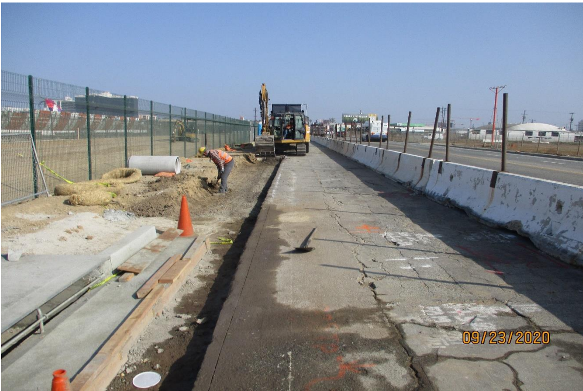
UG1- Crub and gutter removal on Aviation at UG-1.
