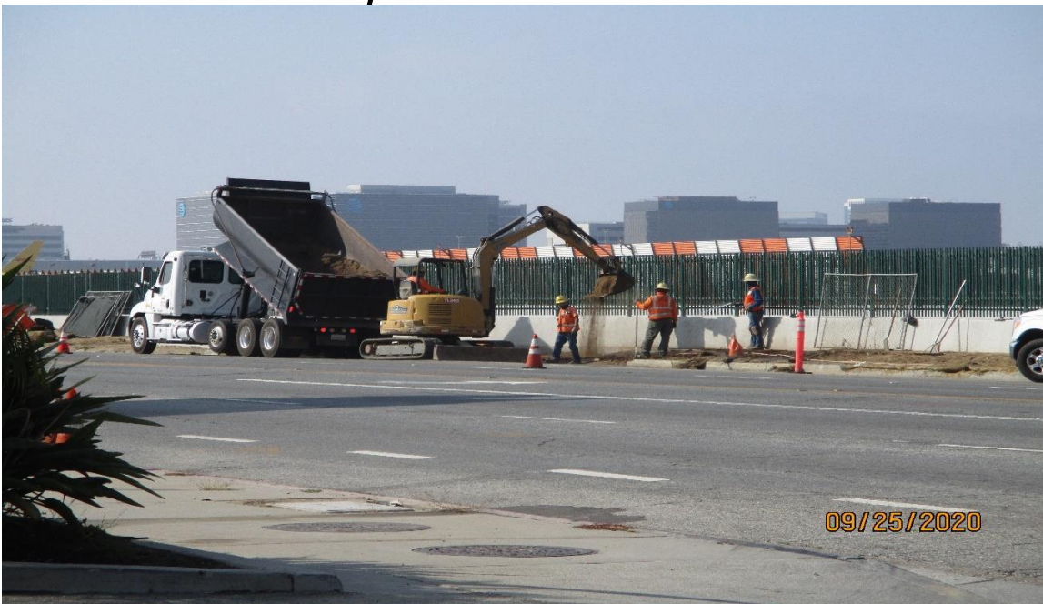
UG1- Drainage swale grading at UG-1.
