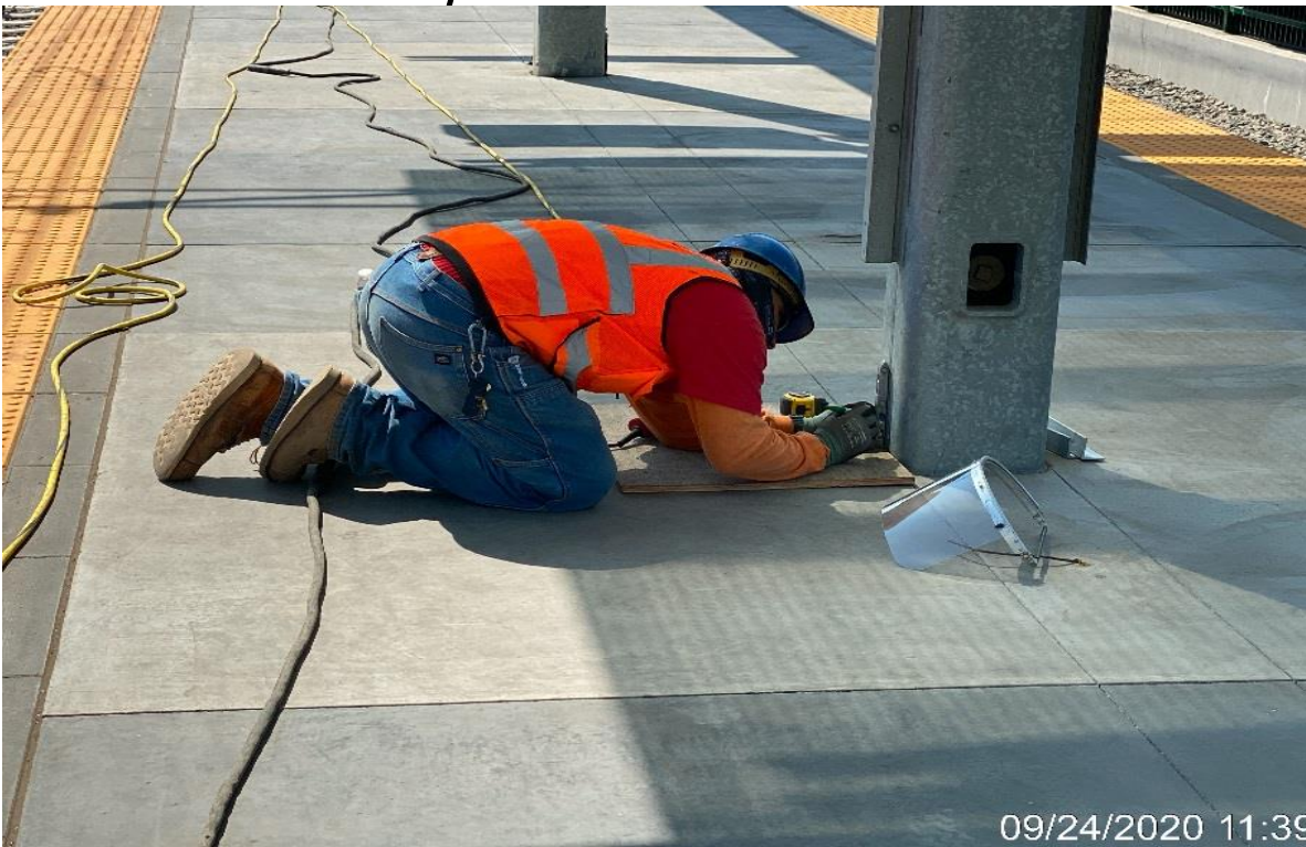
HYDE PARK STATION – Fabricating/welding mounting brackets to the platform column bases in preparation for cladding installation.
