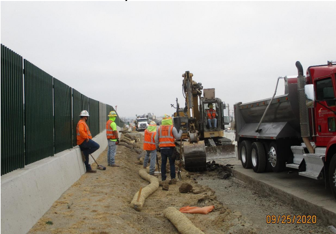
UG1- Curb and gutter removal at UG-1.
