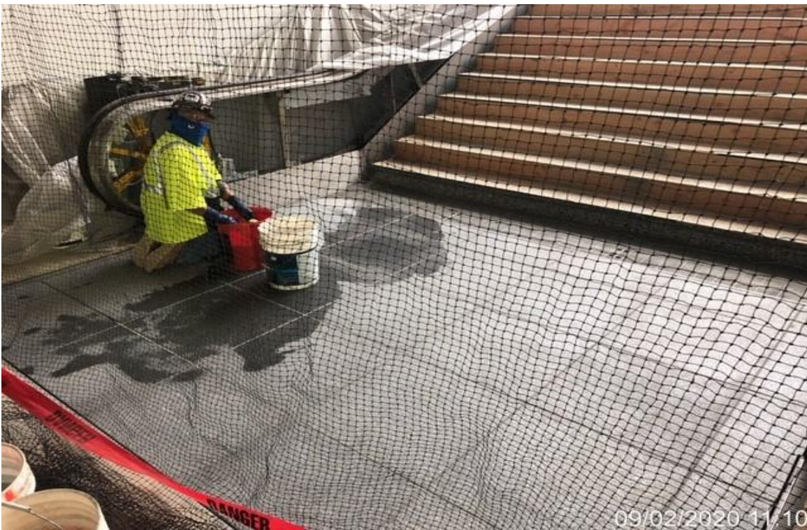
MLK STATION – Carrara Marble grouting pavers at bottom landing of staircase #1
