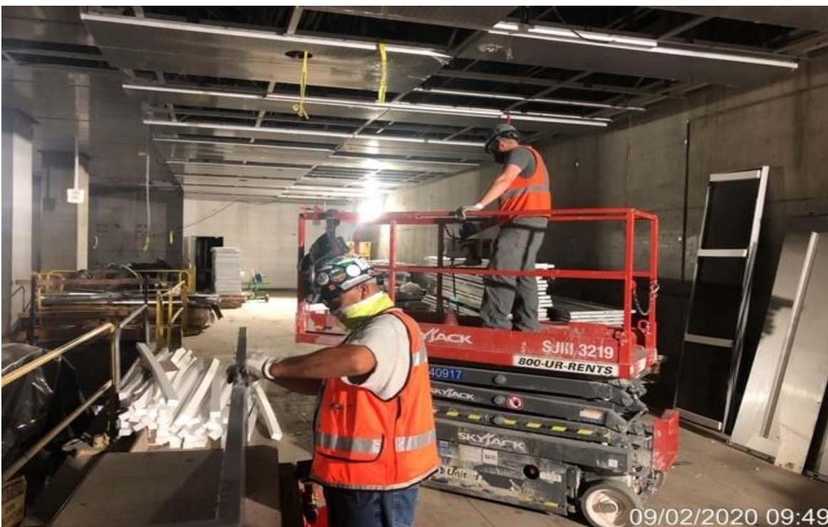
EXPO STATION – PCI installing ceiling panels at concourse level.
