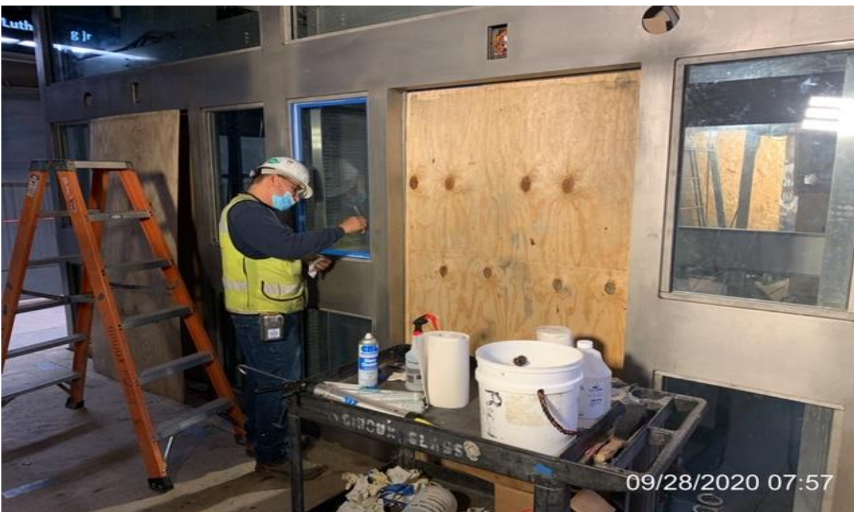
MLK STATION – Continue installing glass panels to Elevators 3&4 at platform level.
