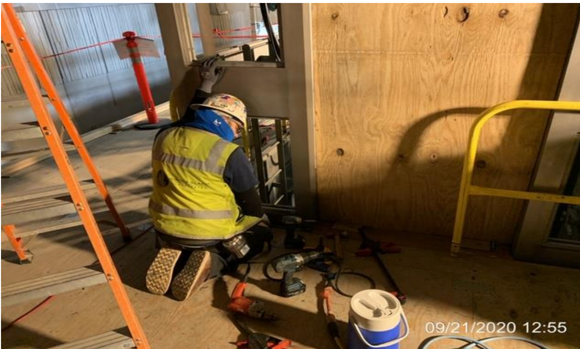
MLK STATION – Continue installing glass stops to Elevators 3&4 at platform level.
