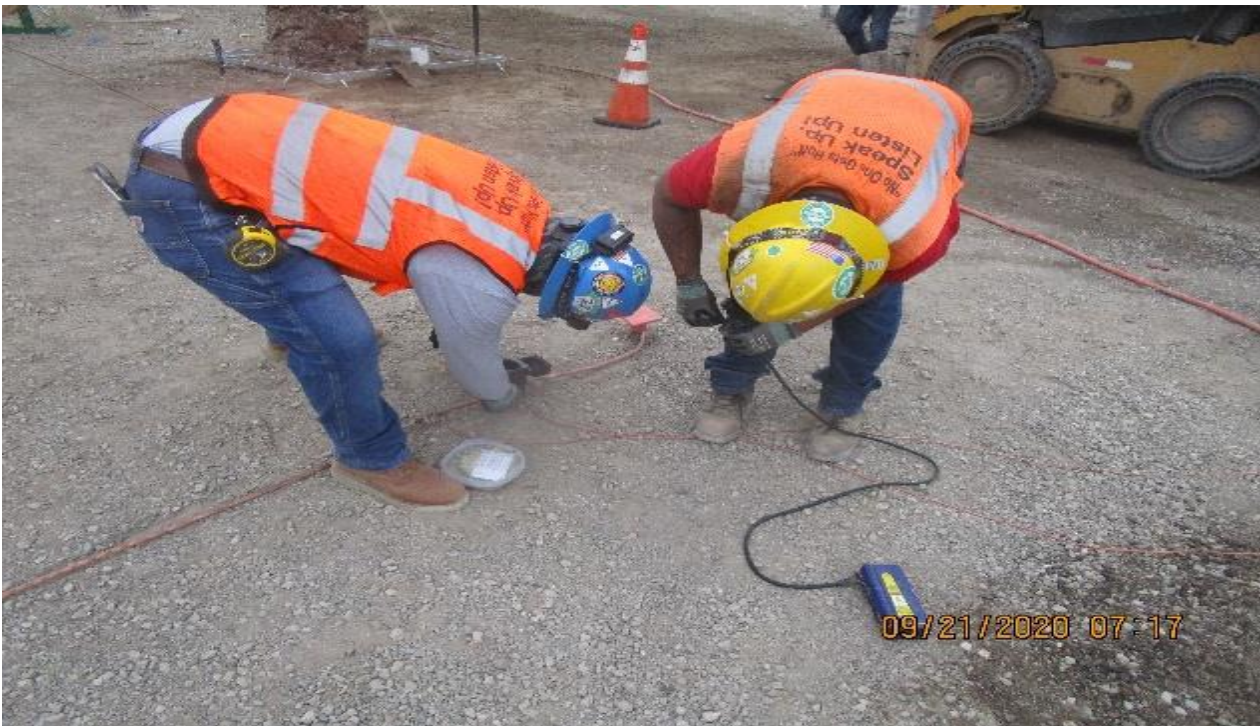
LEIMERT PARK STATION – Continue installing ground grid throughout the plaza level.
