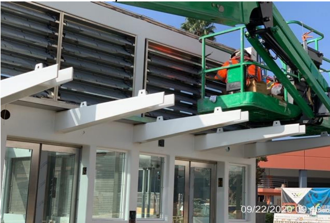
MLK STATION – VNSM installing louvers at elevator structure #1 and #2
