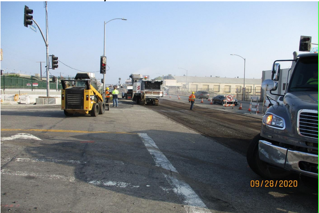
104 th street- Cold planning the existing AC at 104th street.
