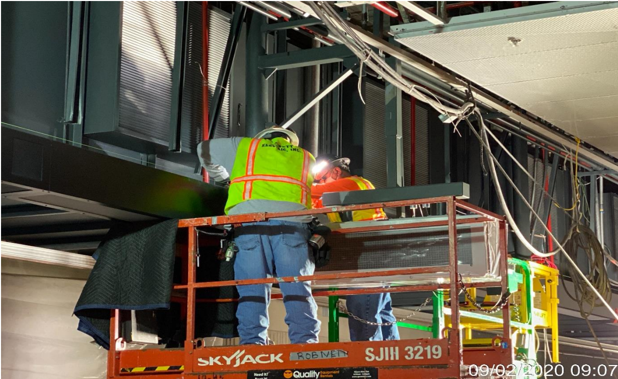
Crenshaw/Vernon – Robnett installing edge lighting at Vernon platform.
