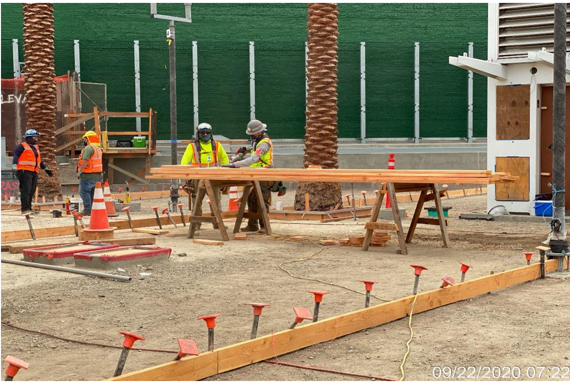
Crenshaw/Vernon – DV setting forms for concrete placement at Vernon
