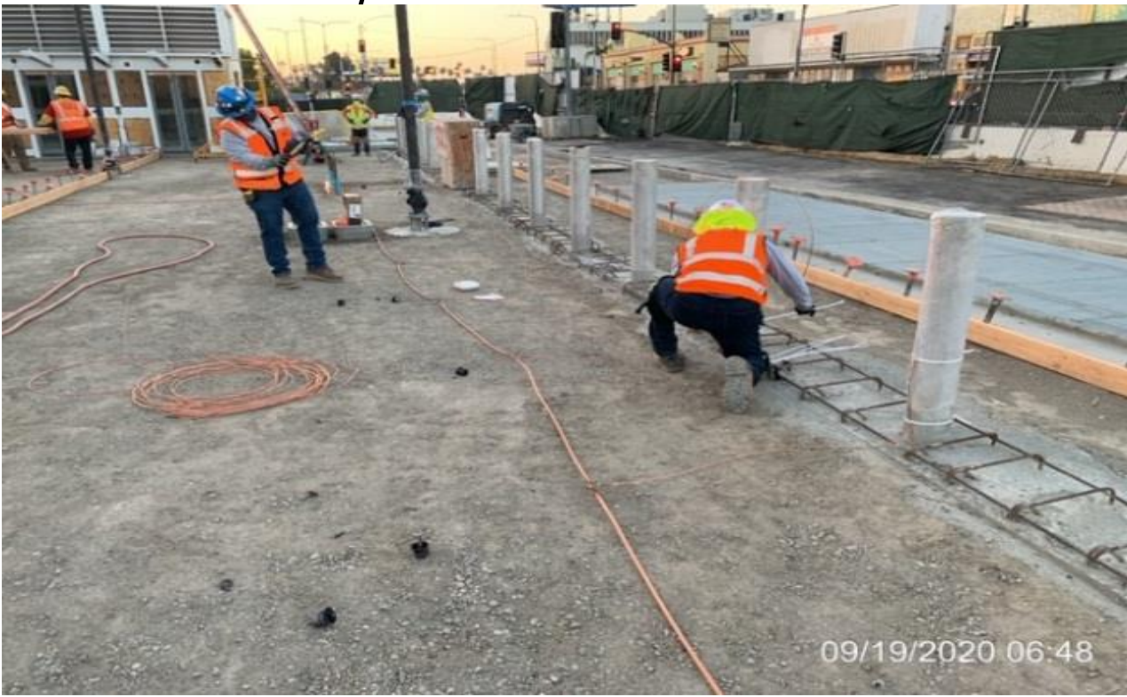
LEIMERT PARK STATION – Continue installing ground grid throughout the plaza level.
