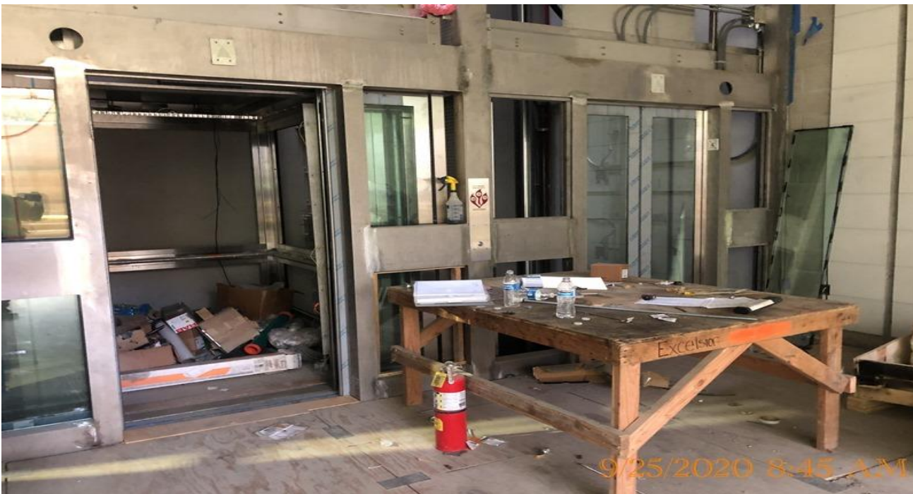
EXPO STATION – Installing glass panels to Elevators 1&2 at the concourse level.
