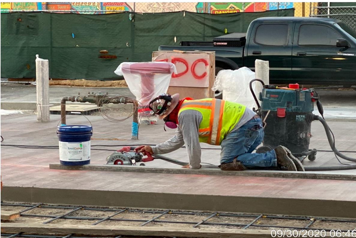
Crenshaw/Vernon – Control joint cutting for plaza slab at Vernon.
