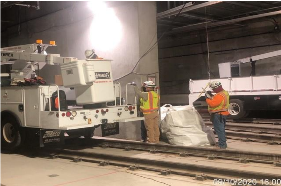
EXPO STATION – Dyna Electric crew prepping to anchor seismic supports.
