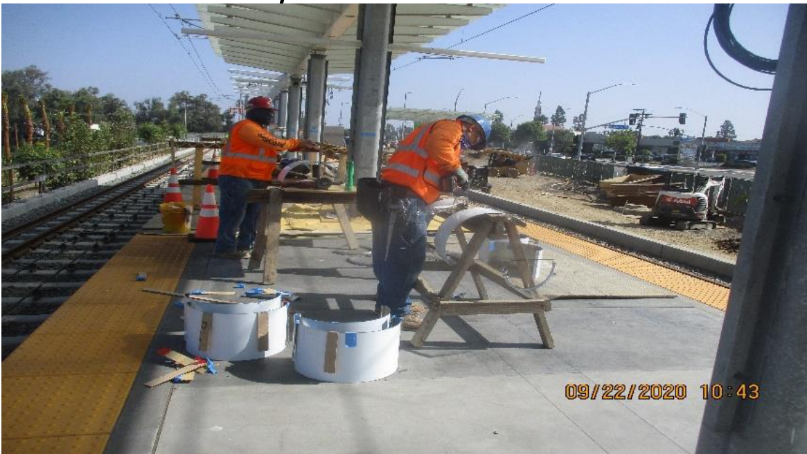
La Brea – WSCC Place padding bases at La Brea Station columns.
