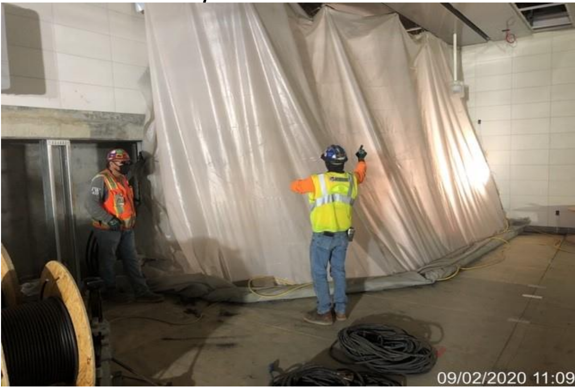
MLK STATION – McMahon sand blasting fascia of elevator #1 and #2
