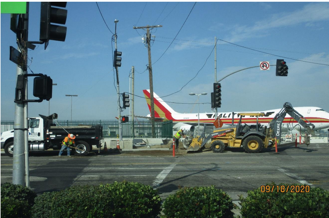
104 th street- Excavating for the traffic signal pole at 104th street.
