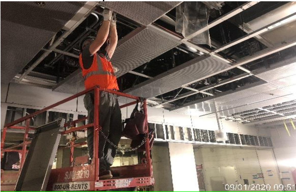
EXPO STATION – PCI modifying and installing ceiling panels.
