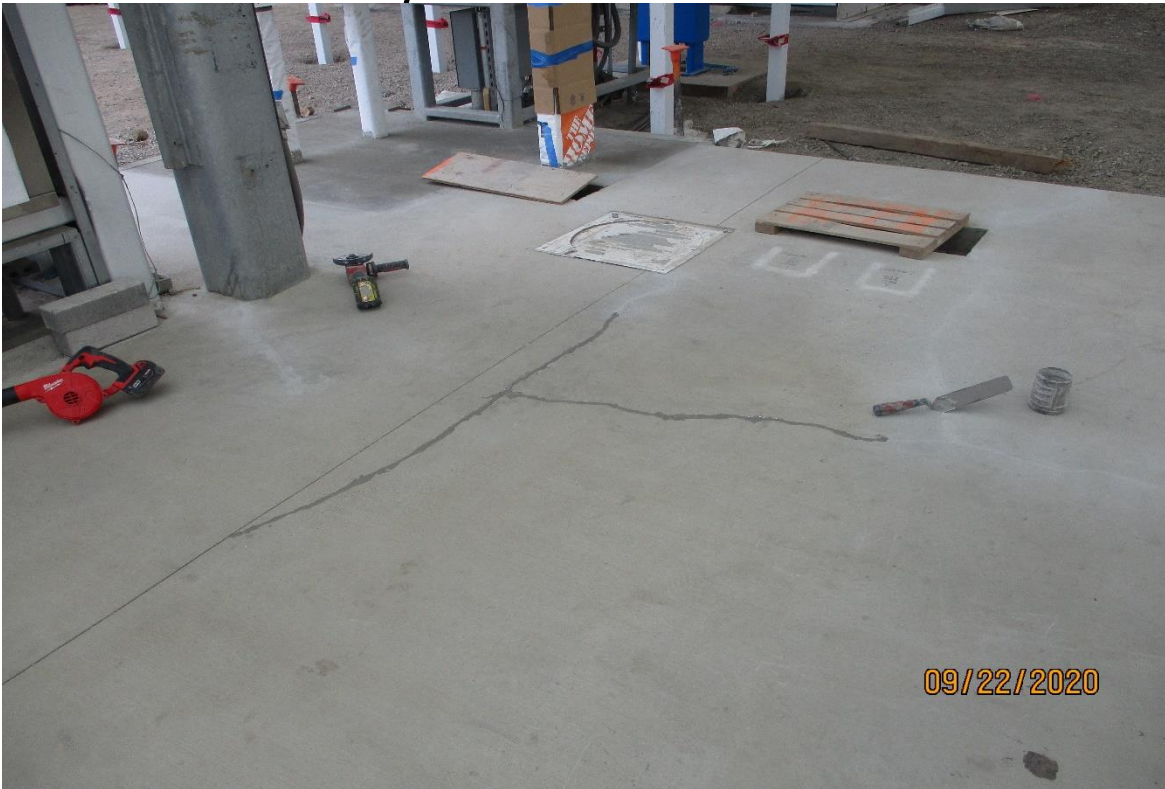
104 th street- Crack repair at the Aviation Station ticket kiosk slab.
