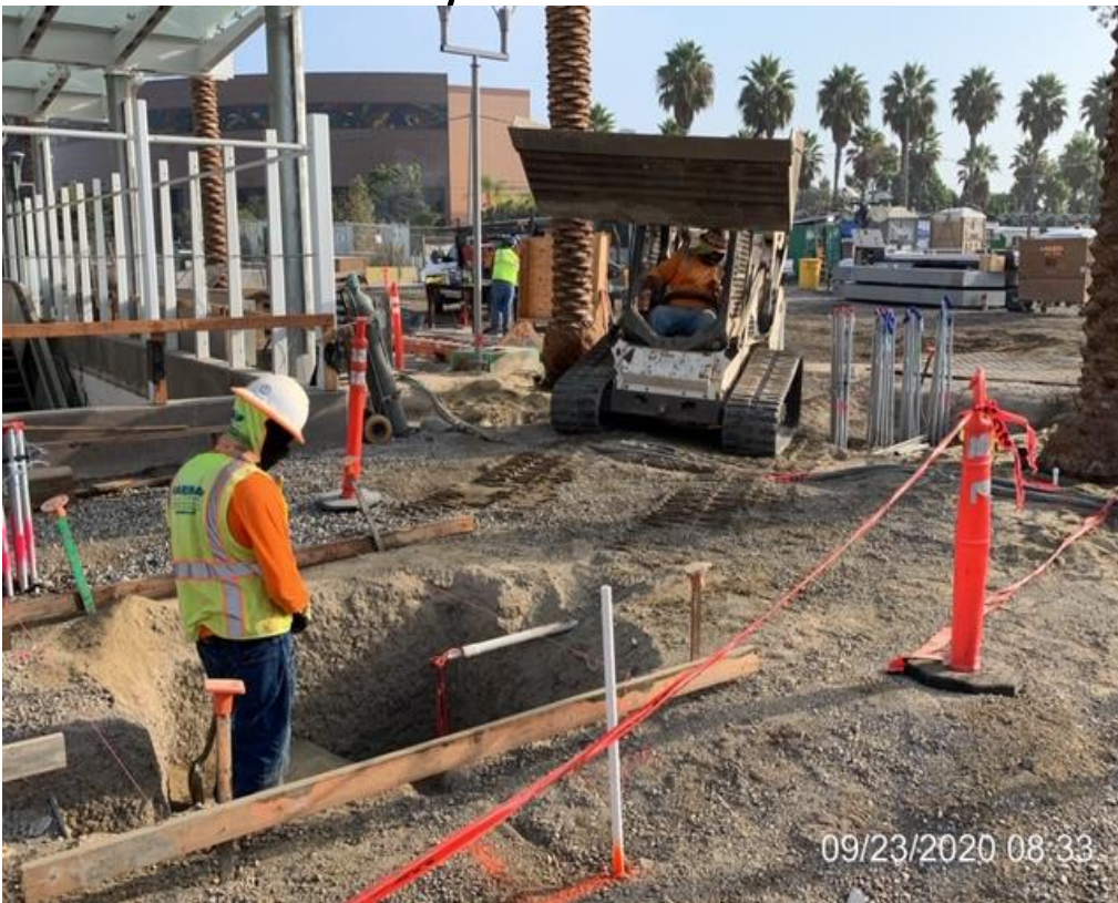
EXPO STATION – Excavating to plant Sycamore trees throughout the plaza level.
