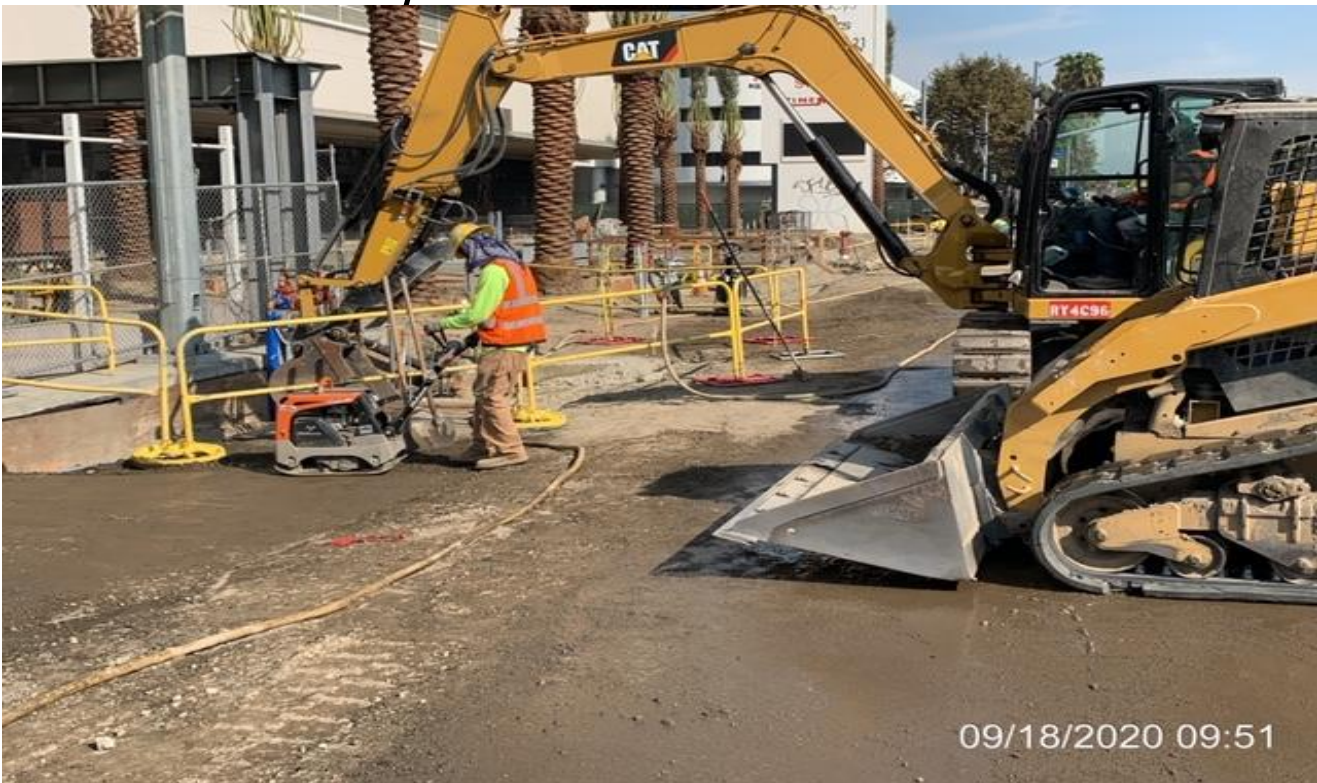
MLK STATION – Continue grading and compacting throughout the plaza level.
