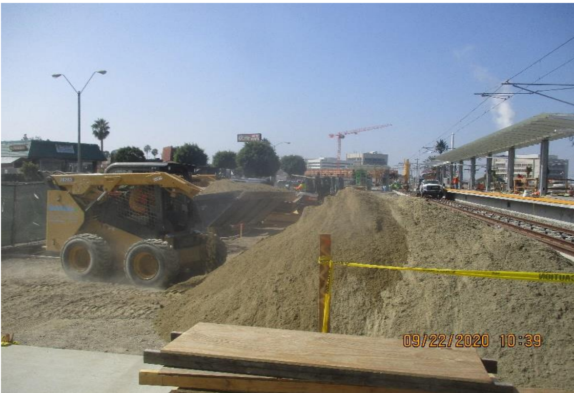
La Brea – Marina Deliver amended soil and plant trees at La Brea Sta.
