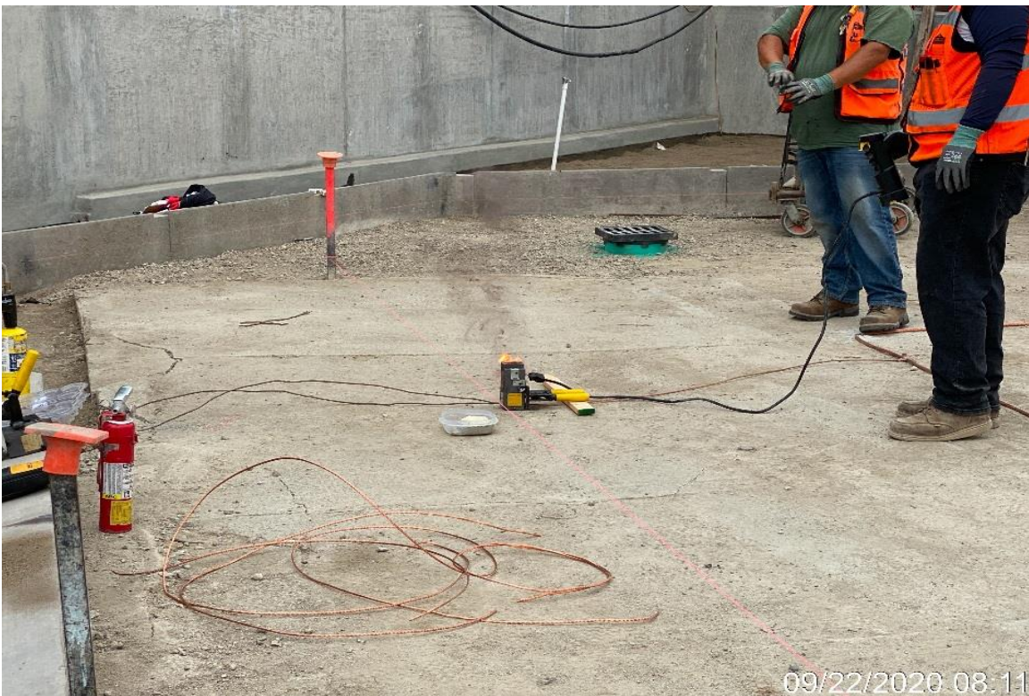
LEIMERT PARK STATION – Continue installing ground grid throughout the plaza level.
