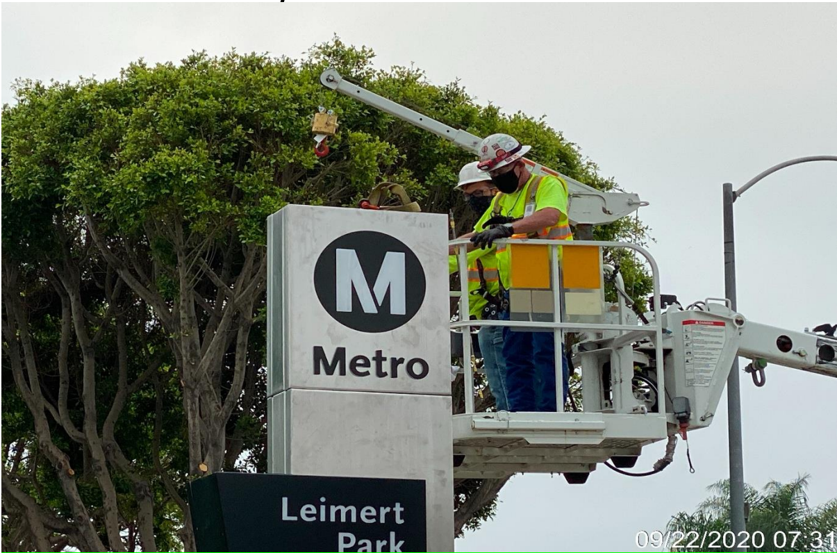
Crenshaw/Vernon – SmithCraft installing Grand Pylon at Vernon Plaza.
