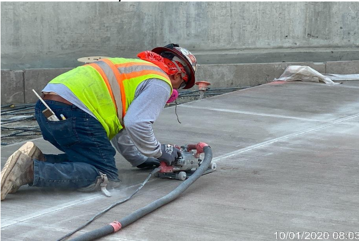
LEIMERT PARK STATION – Continue saw cutting control joints for the architectural topping slab throughout the plaza level.
