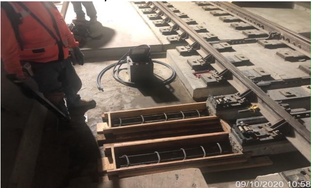
EXPO STATION – WSCC crew building formwork for re-build of plinths
