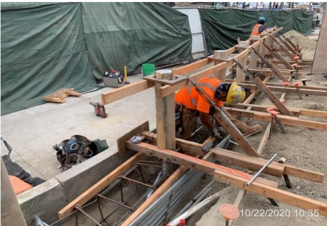
MLK STATION – WSCC carpenters setting formwork for bollard footing.
