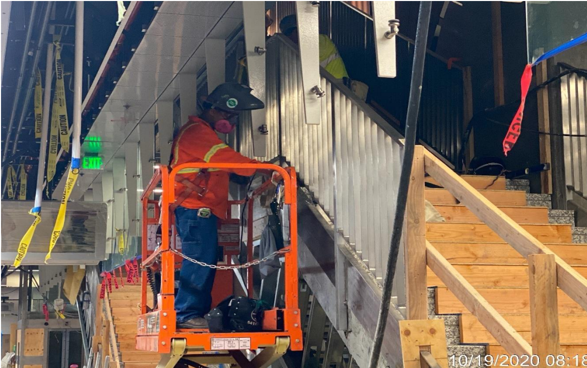
Crenshaw/Vernon – McMahon welding handrail at Vernon stairwell # 4
