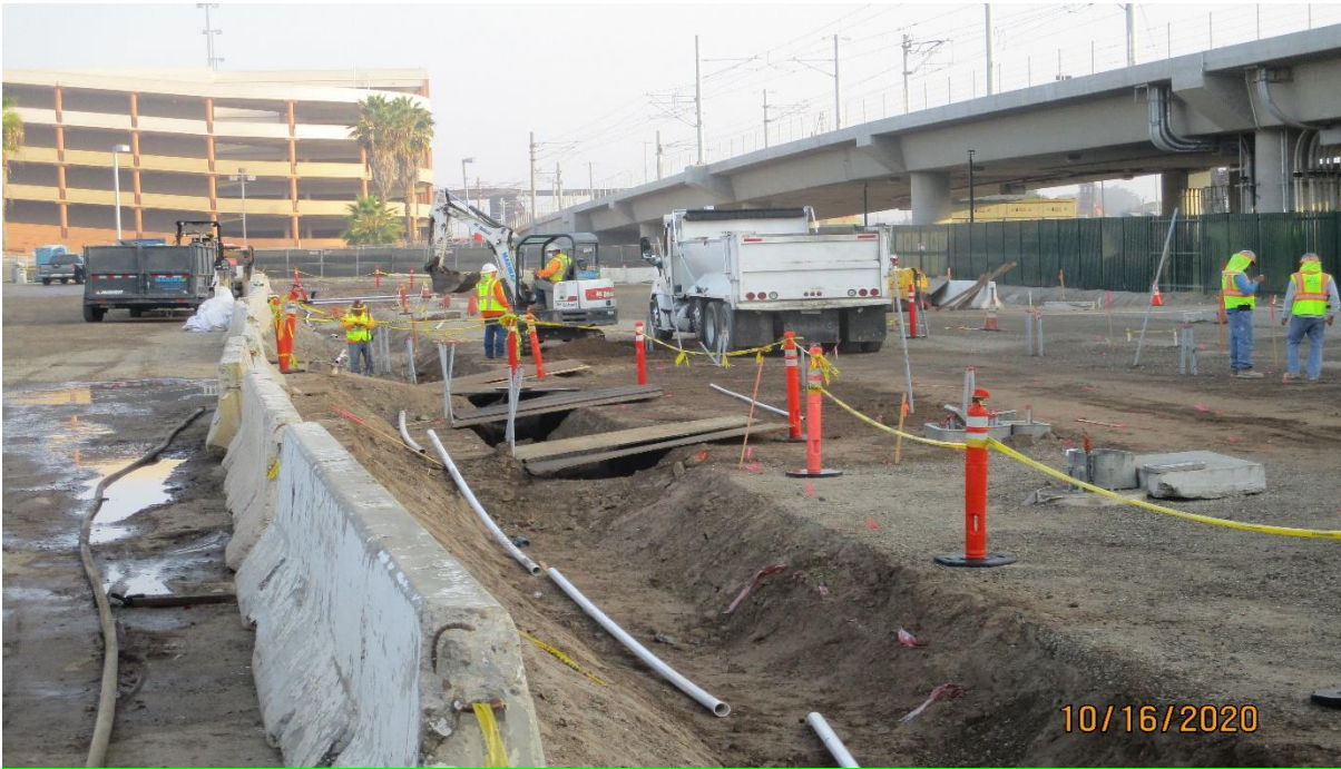
AVIATION/CENTURY - Landscape irrigation place emtn at the Aviation Station.
