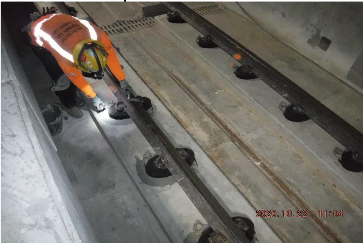
UG3 – STA 287+20 TK#4/NB looking north – UG3 patching plinth PCC (REWORK)
