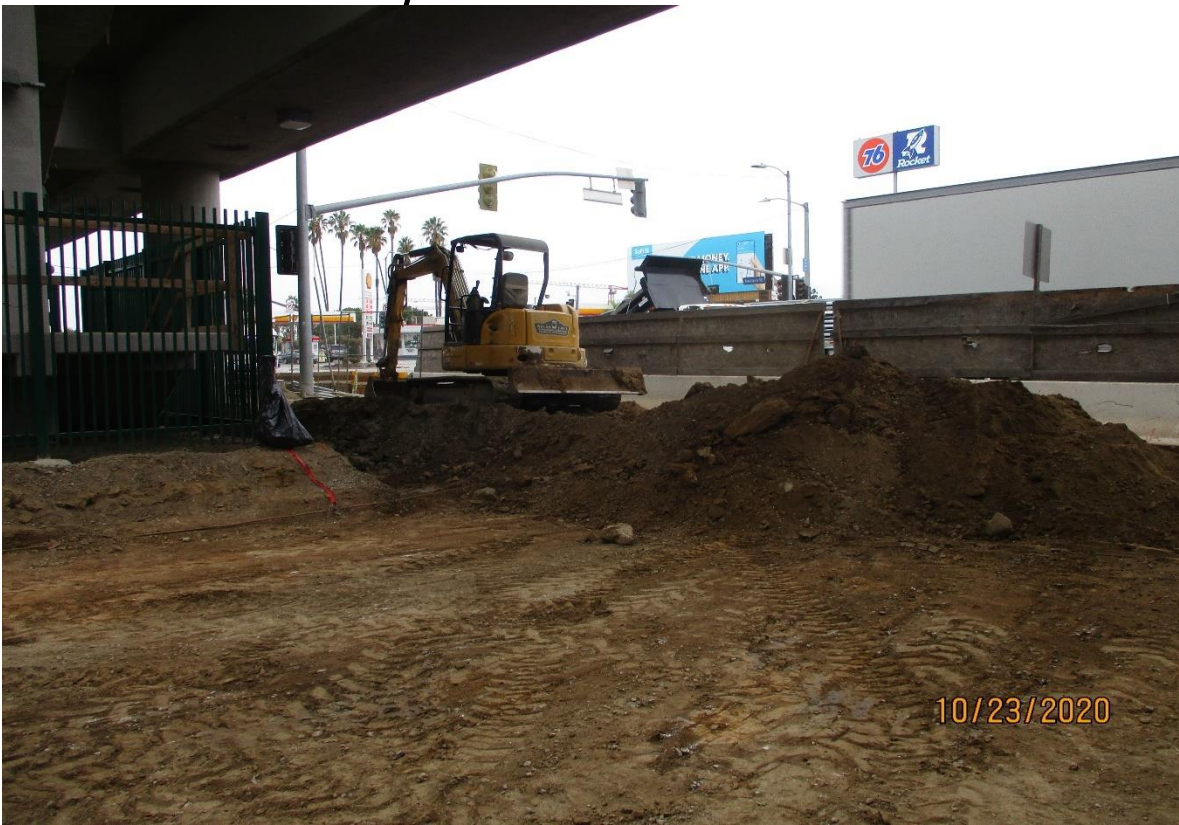
AVIATION/CENTURY- Excavating for the amended soil at Aviation and Century.
