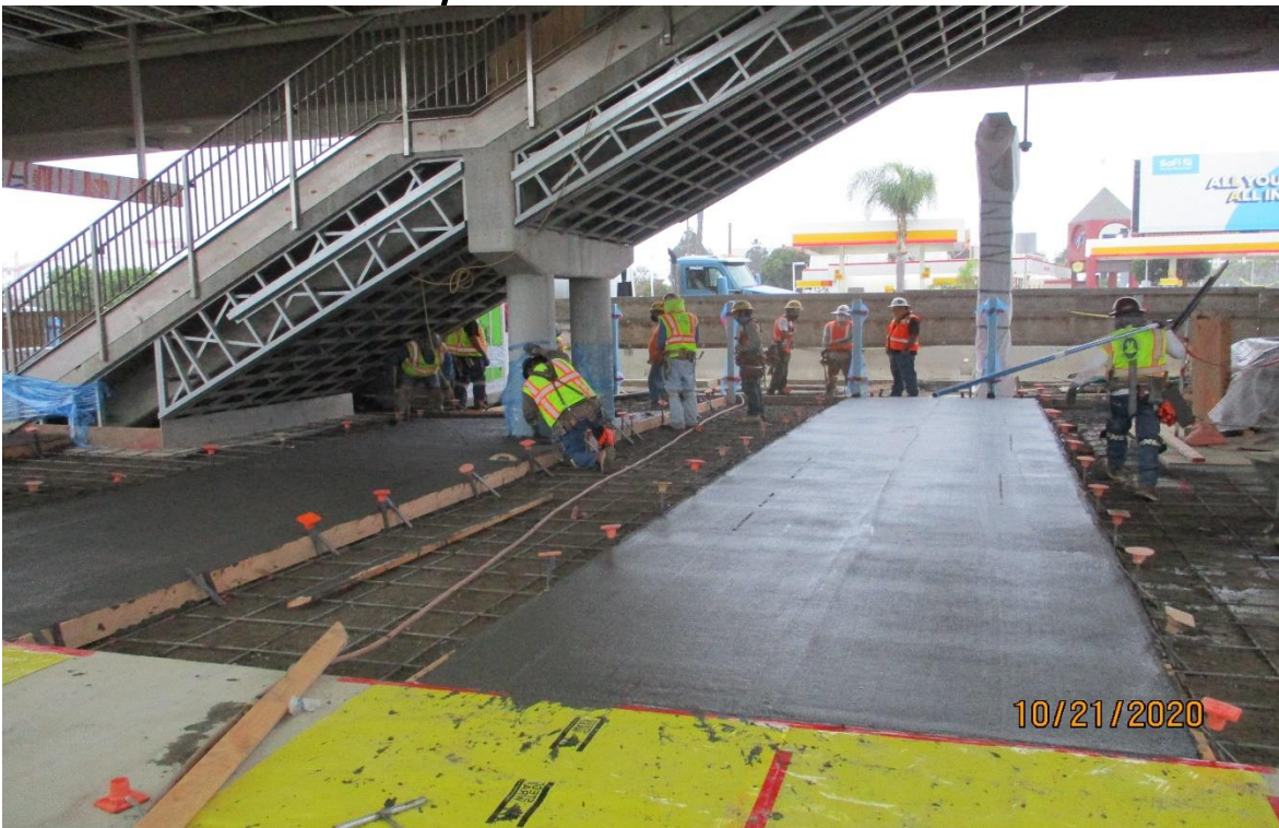
AVIATION/CENTURY- Placing concrete for the Aviation Station stairway landing.
