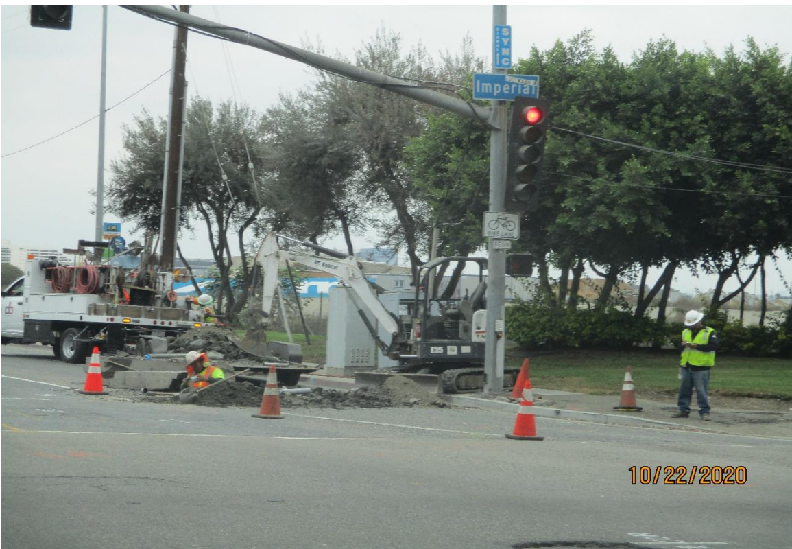
AVIATION/CENTURY- Trenching for the traffic signal conduit on Aviation at Imperial.
