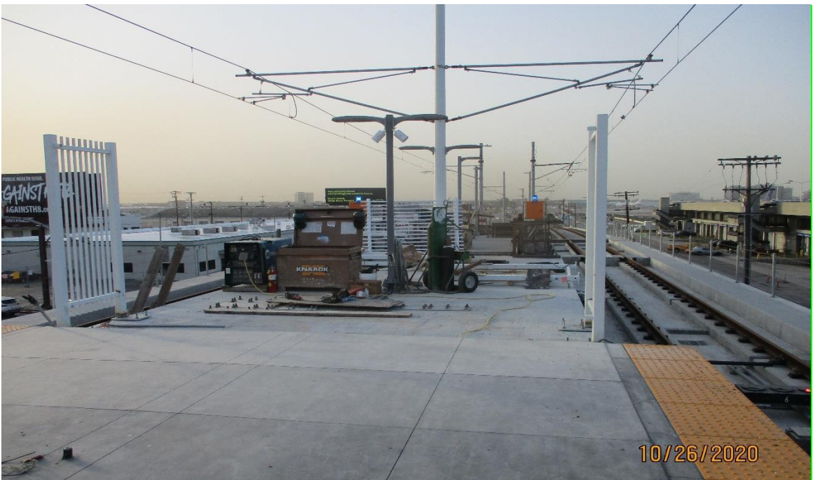
AVIATION/CENTURY- Fabricating the emergency exit fencing at the Aviation Station platform.
