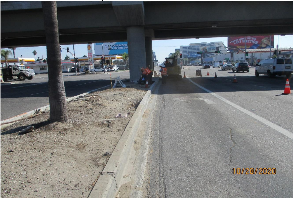
AVIATION/CENTURY- Starting to rough grade the west median at Aviation and Century.
