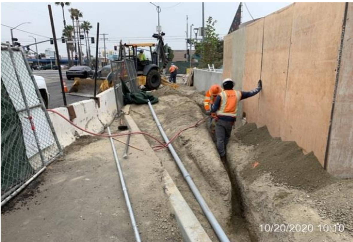
EXPO STATION - Select Electric excavating trench to extend conduits
