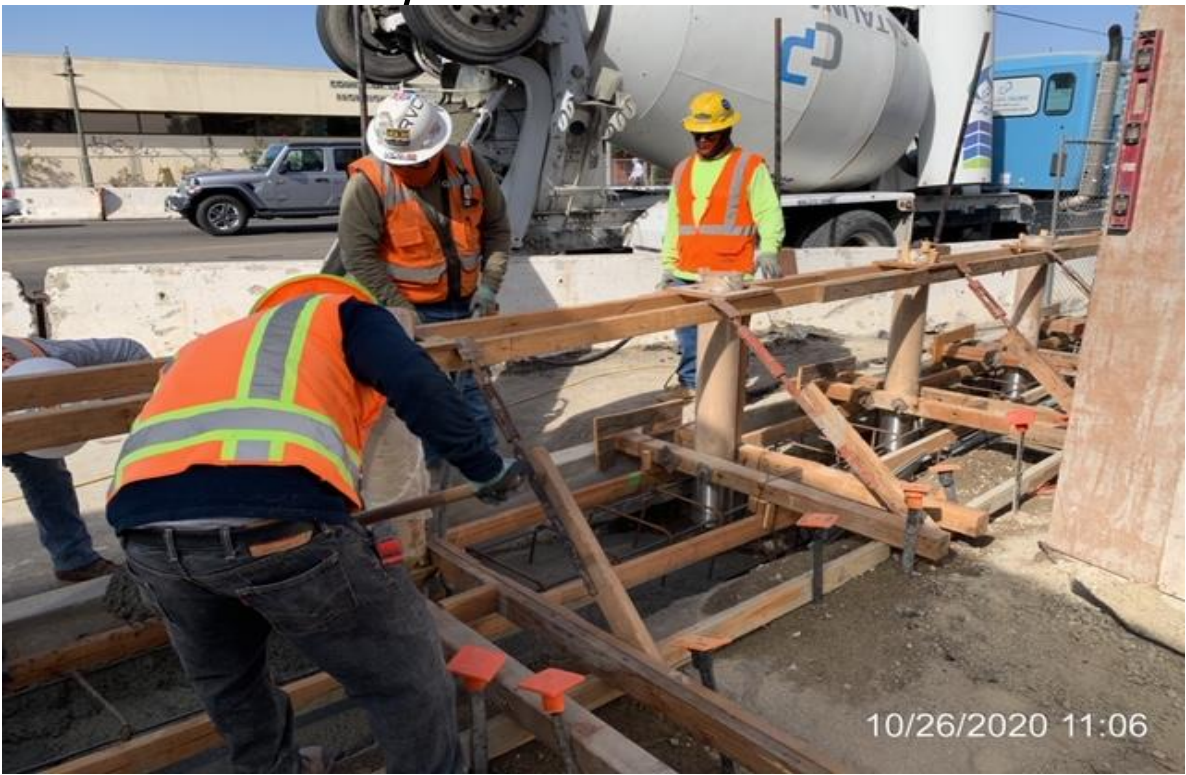
EXPO STATION – WSCC crew placing concrete for bollard footing.
