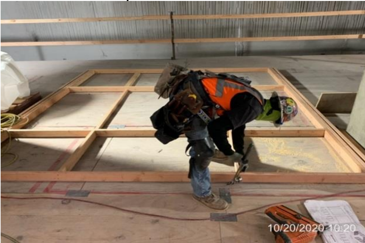
MLK STATION – WSCC carpenter building mock-up security booth.
