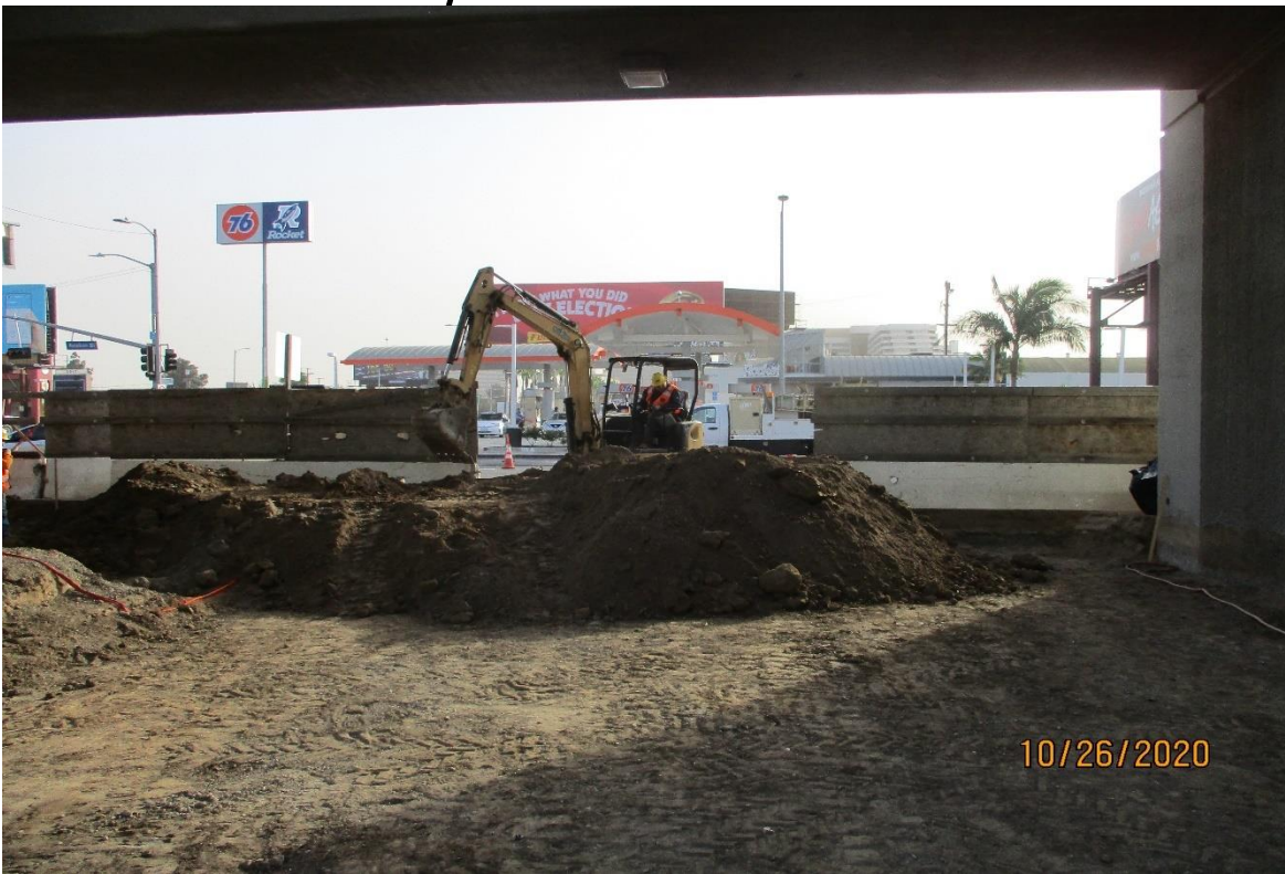
AVIATION/CENTURY- Excavating for the amended soil at Aviation and Century.
