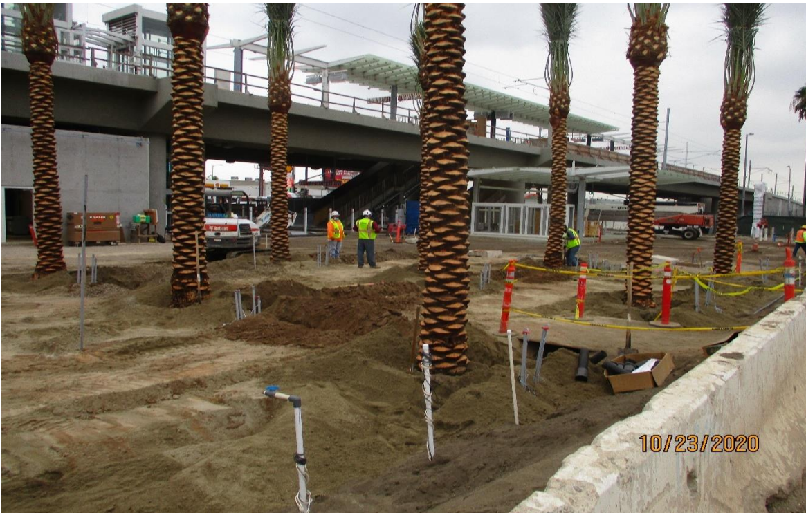
AVIATION/CENTURY- trenching for the palm tree irrigation at the Aviation Station.
