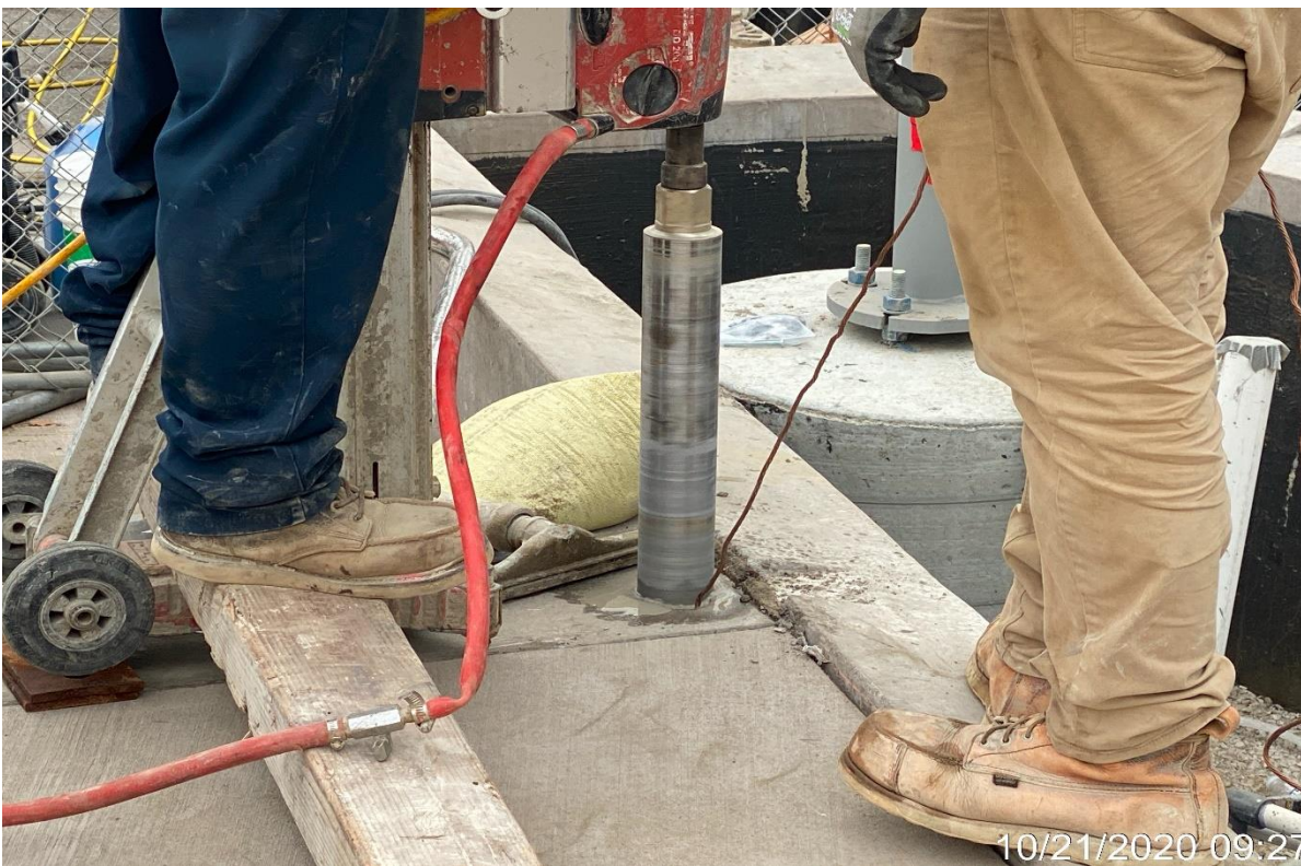
Crenshaw/Vernon – WSCC coring for handrail at Vernon plaza stairs.
