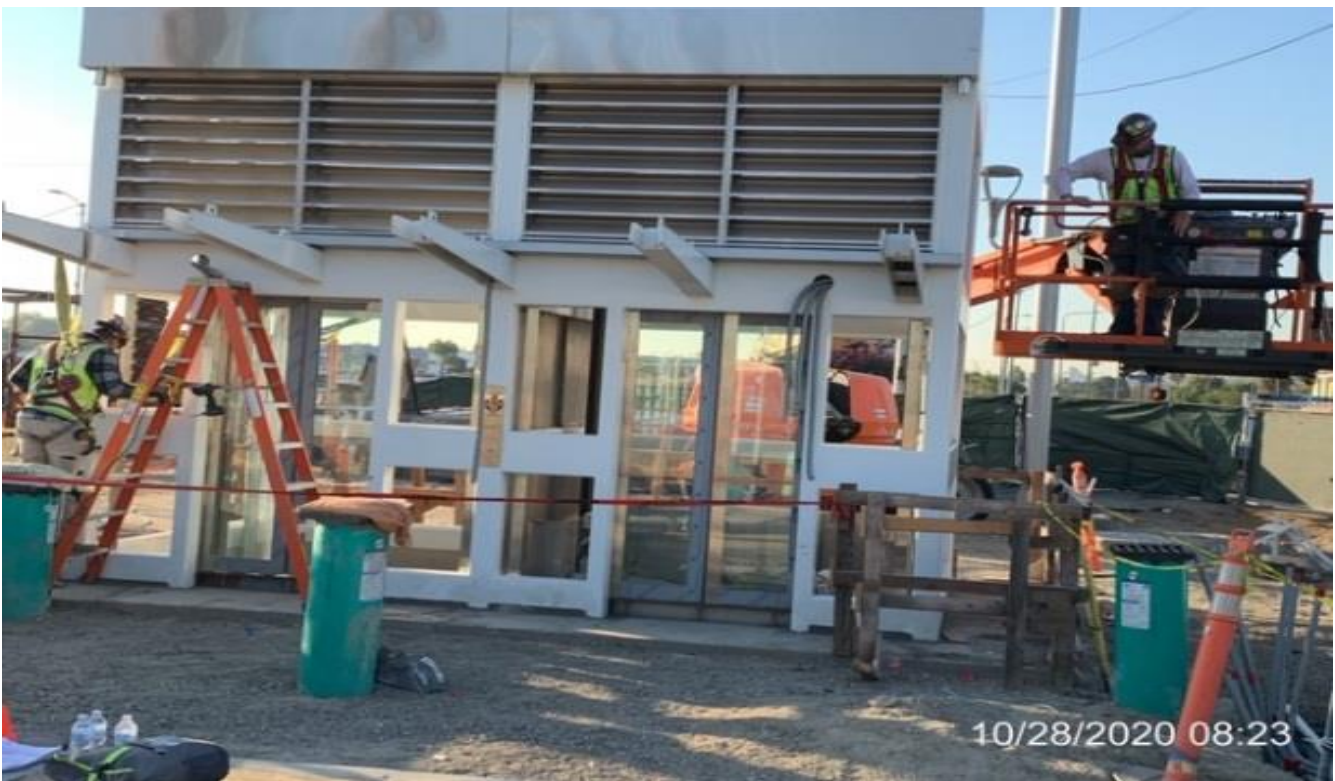
EXPO STATION – Continue installing glass stops to Elevators 1&2 at the plaza.
