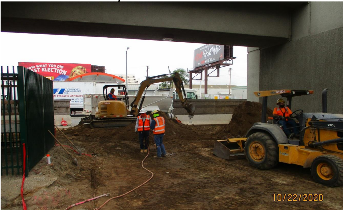
AVIATION/CENTURY- Excavating for the amended soil at Aviation and Century.
