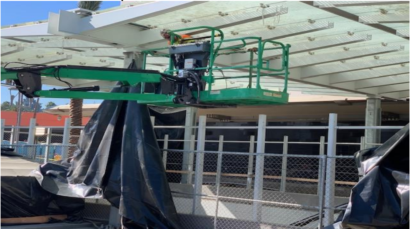
MLK STATION – WSCC ironworkers drilling for lighting at canopy.
