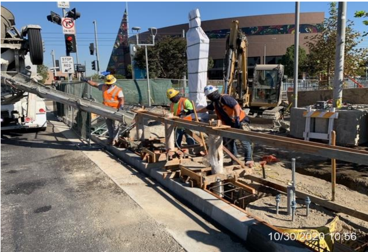
EXPO STATION – WSCC carpenters placing concrete footing for bollards.
