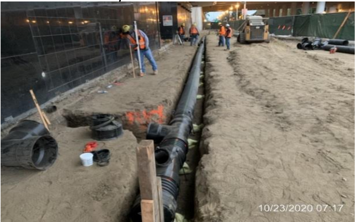
MLK STATION – WSCC crew adjusting 12” HDPE for storm drain.
