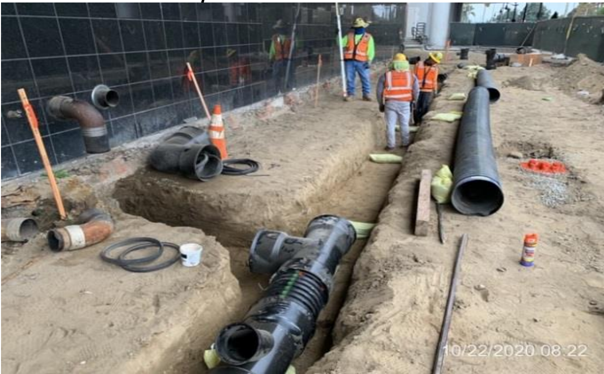
MLK STATION – WSCC crew laying 12” HDPE for storm drain.
