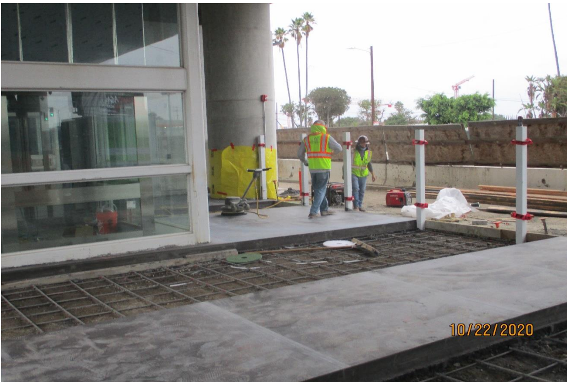
AVIATION/CENTURY- Buffing the colored concrete placed yesterday at the Aviation Station.
