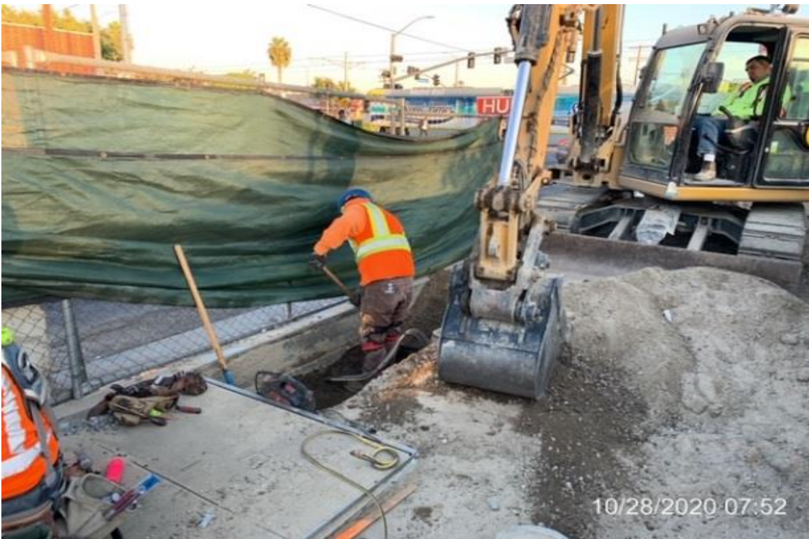
EXPO STATION SITE – WSCC crew excavating trench for bollards.
