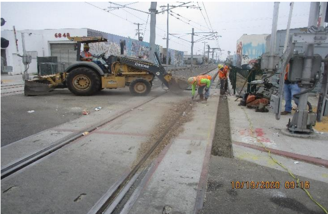
AVIATION/CENTURY- Cleanup and place Ac at West St crossing.
