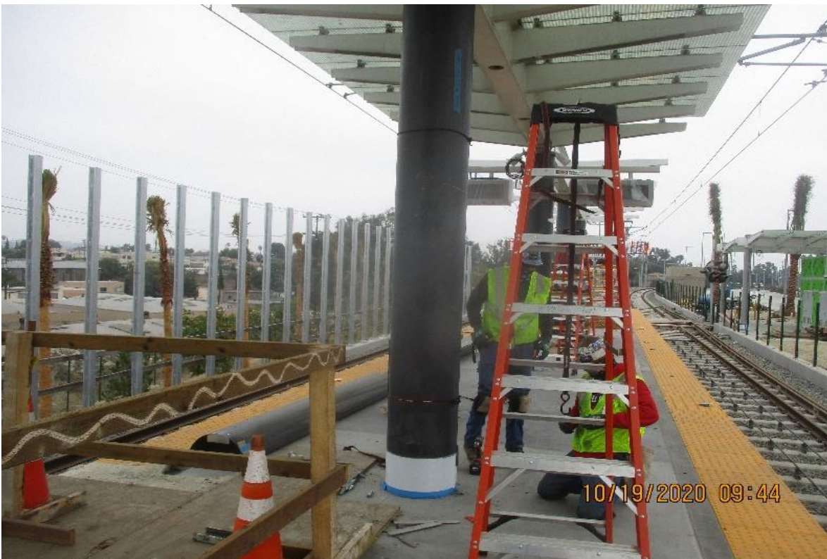
La Brea – McMahon Place cladding on columns at La Brea Sta.
