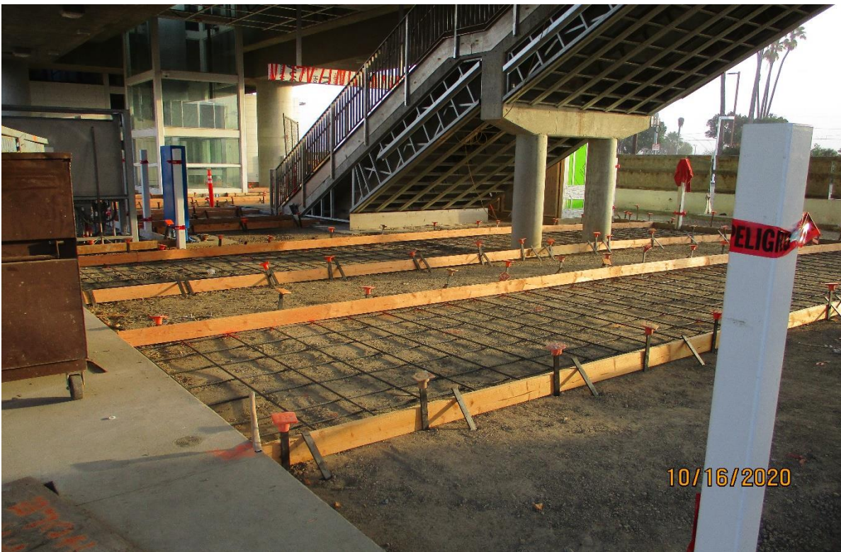
AVIATION/CENTURY- Placing rebar for the Aviation Station stairway landing area.
