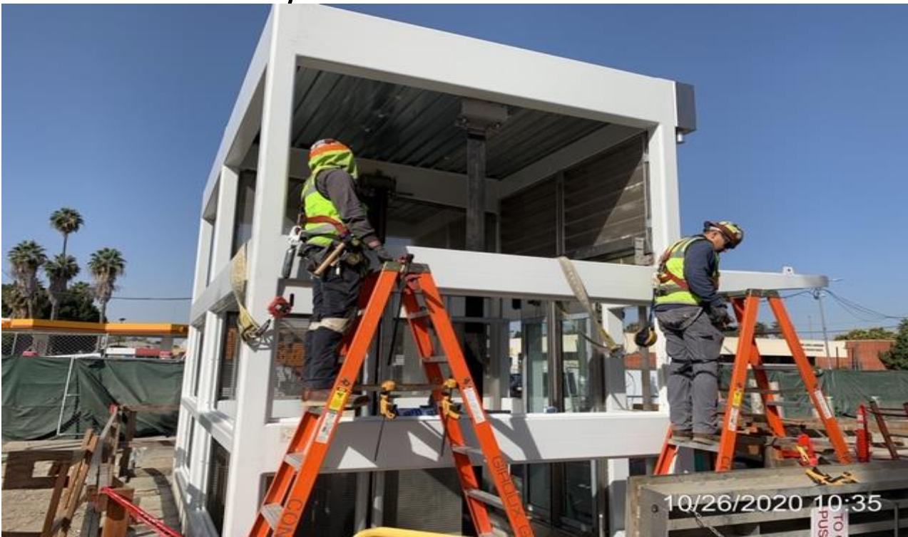
EXPO STATION – Continue installing glass stops to Elevators 1&2 at the plaza.
