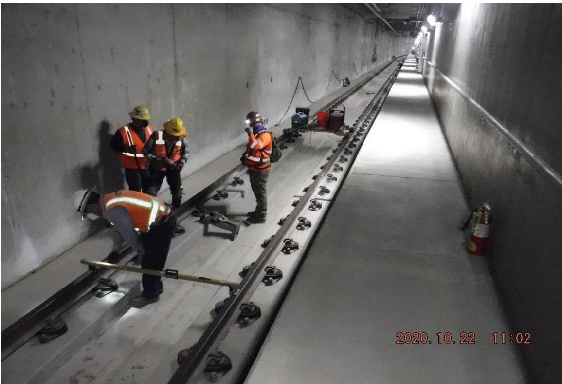
UG3 – STA 288+75 TK#4/NB looking south – adjusting gage (track geometry) in UG3
