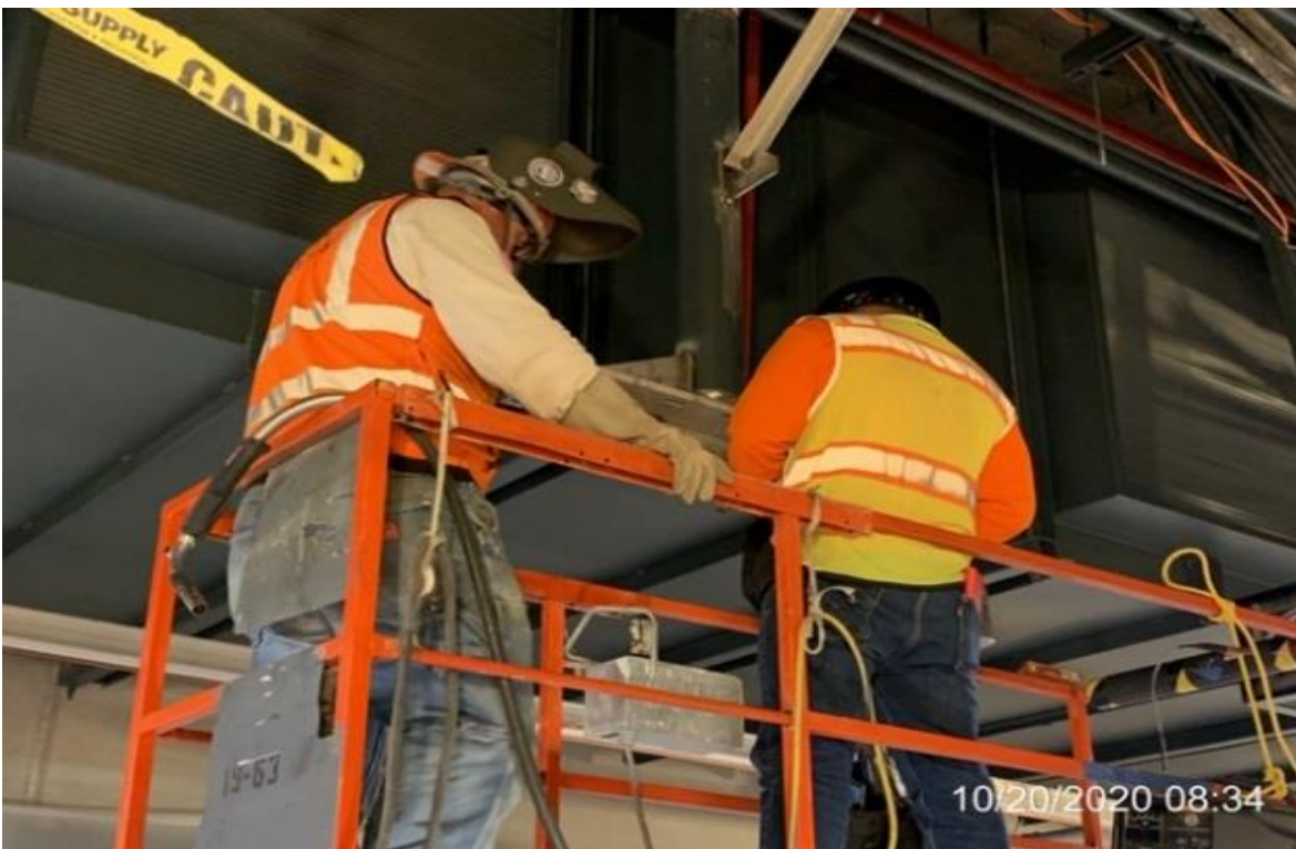
MLK STATION – WSCC ironworkers correcting placement of down stand bottom plates.
