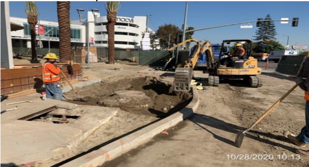
MLK STATION – Excavating/grading the northeast corner of the plaza.
