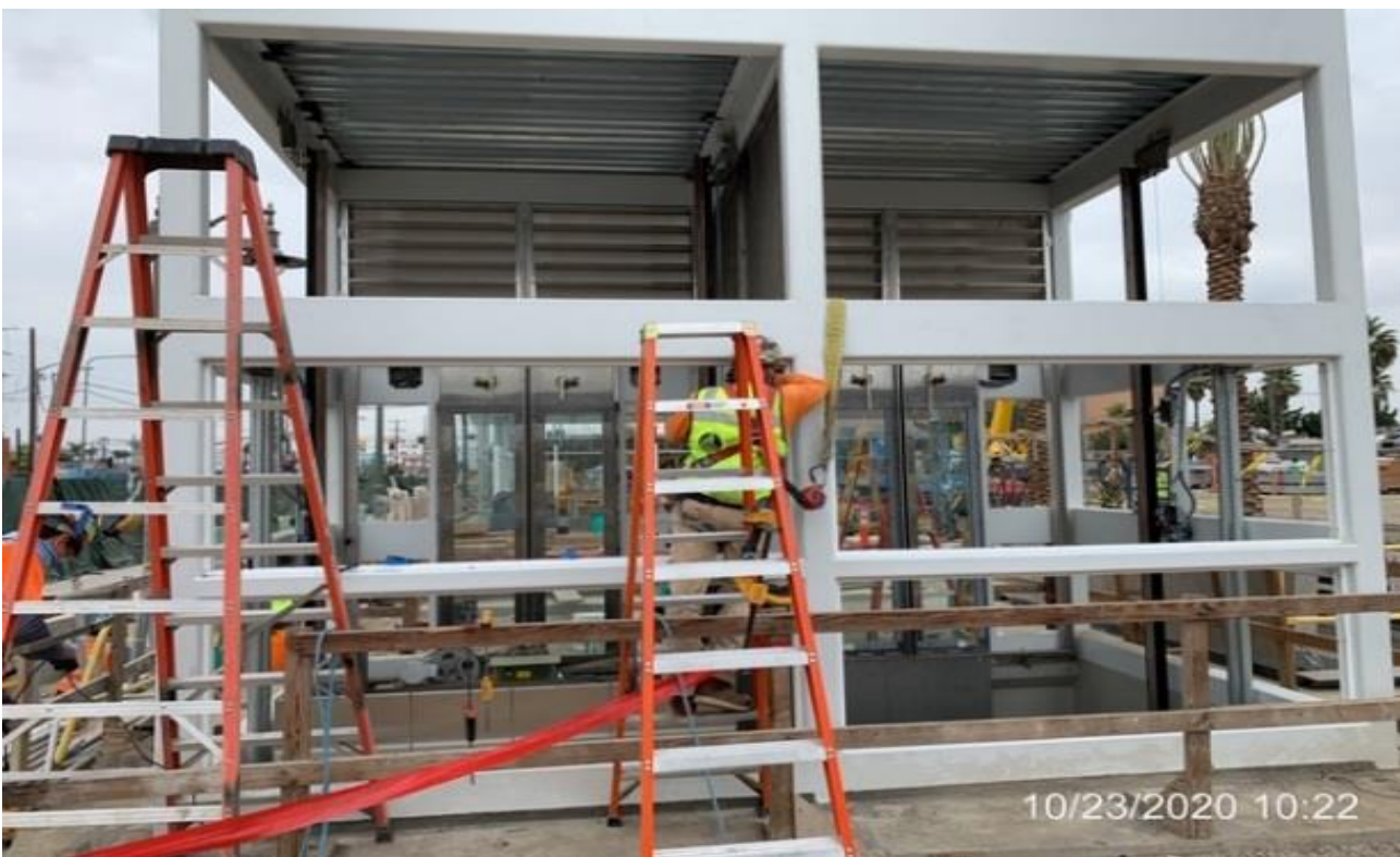
EXPO STATION - Installing glass stops to Elevators 1&2 at the plaza.
