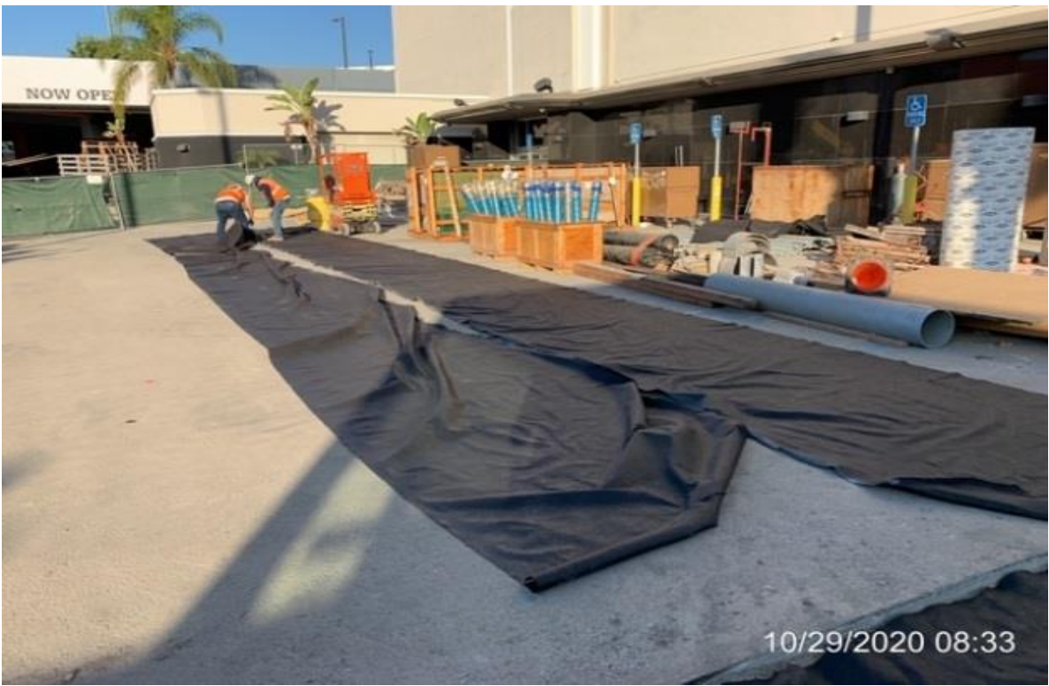
MLK STATION – WSCC installing soil liner inside south planter.
