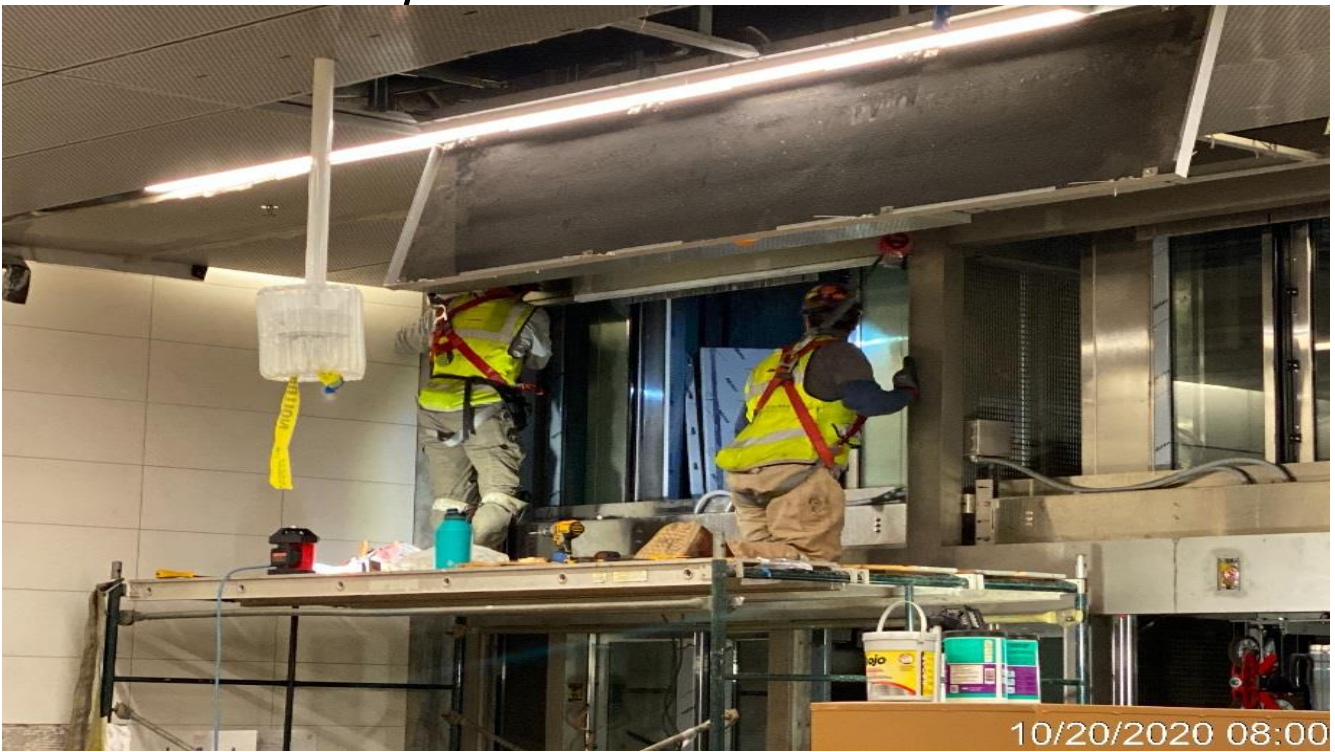
LEIMERT PARK STATION – Continue installing perforated ceiling panels throughout the concourse.
