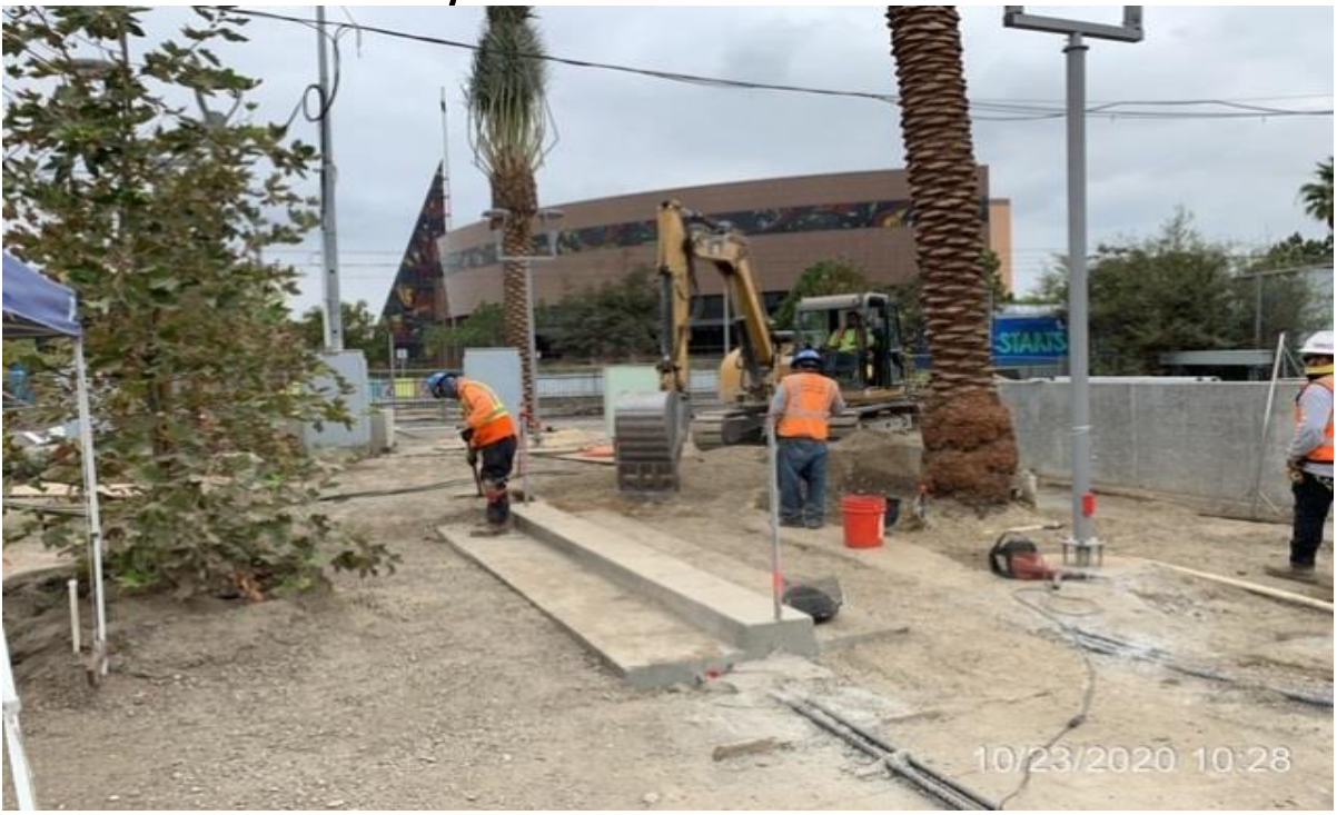
EXPO STATION– WSCC crew grading at north east end of station.
