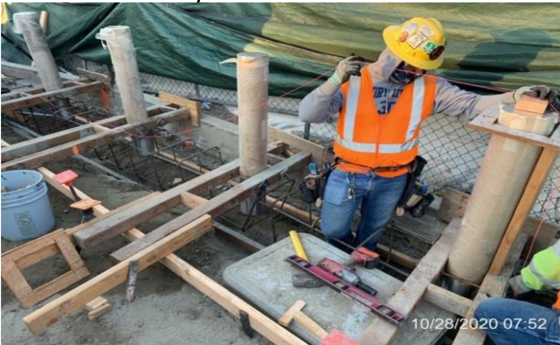
EXPO STATION SITE – WSCC carpenters setting bollards and formwork for footing.
