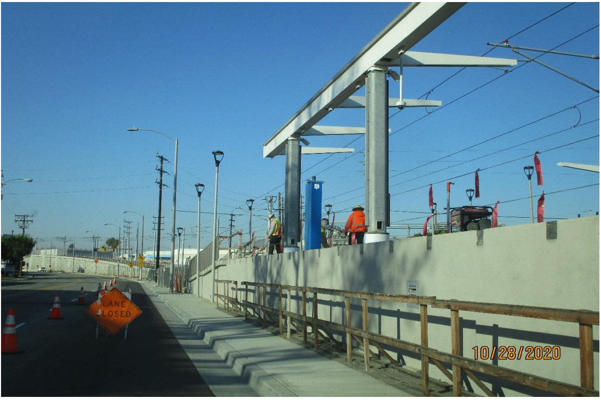
Hindry – Buffing the topping slabs for the NB Hindry platform.
