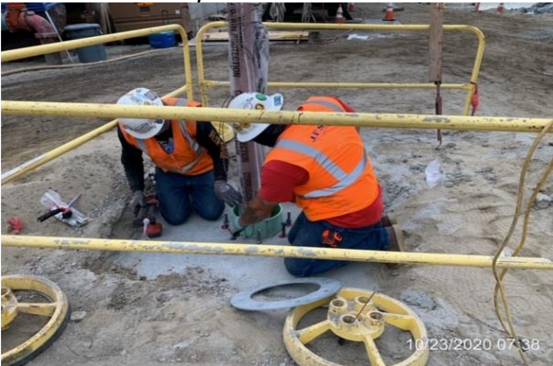
MLK STATION – WSCC crew epoxying bolts for vent stack base
