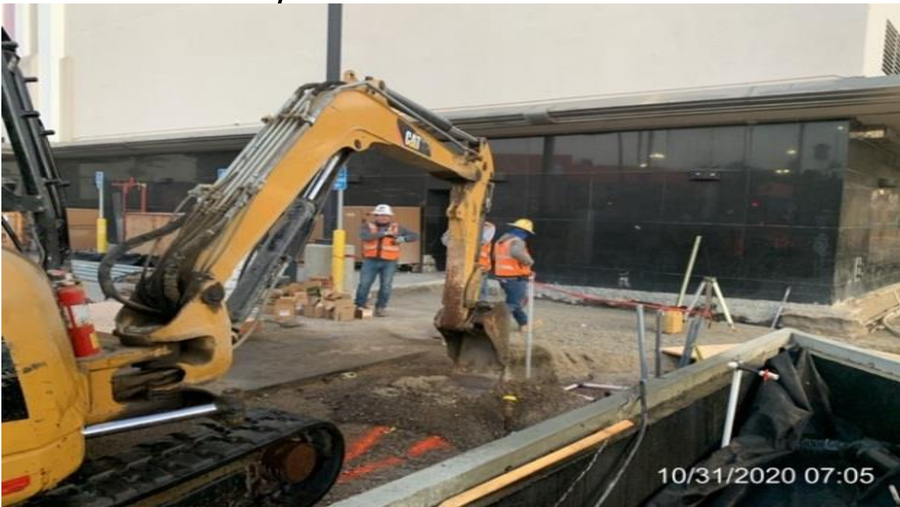
MLK STATION – Excavating/trenching for irrigation and landscape conduit at the plaza.
