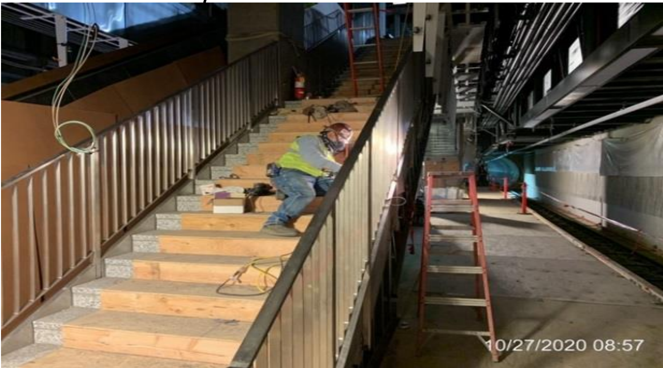
MLK STATION – Continue welding guardrails to Staircase 2 from concourse to platform.
