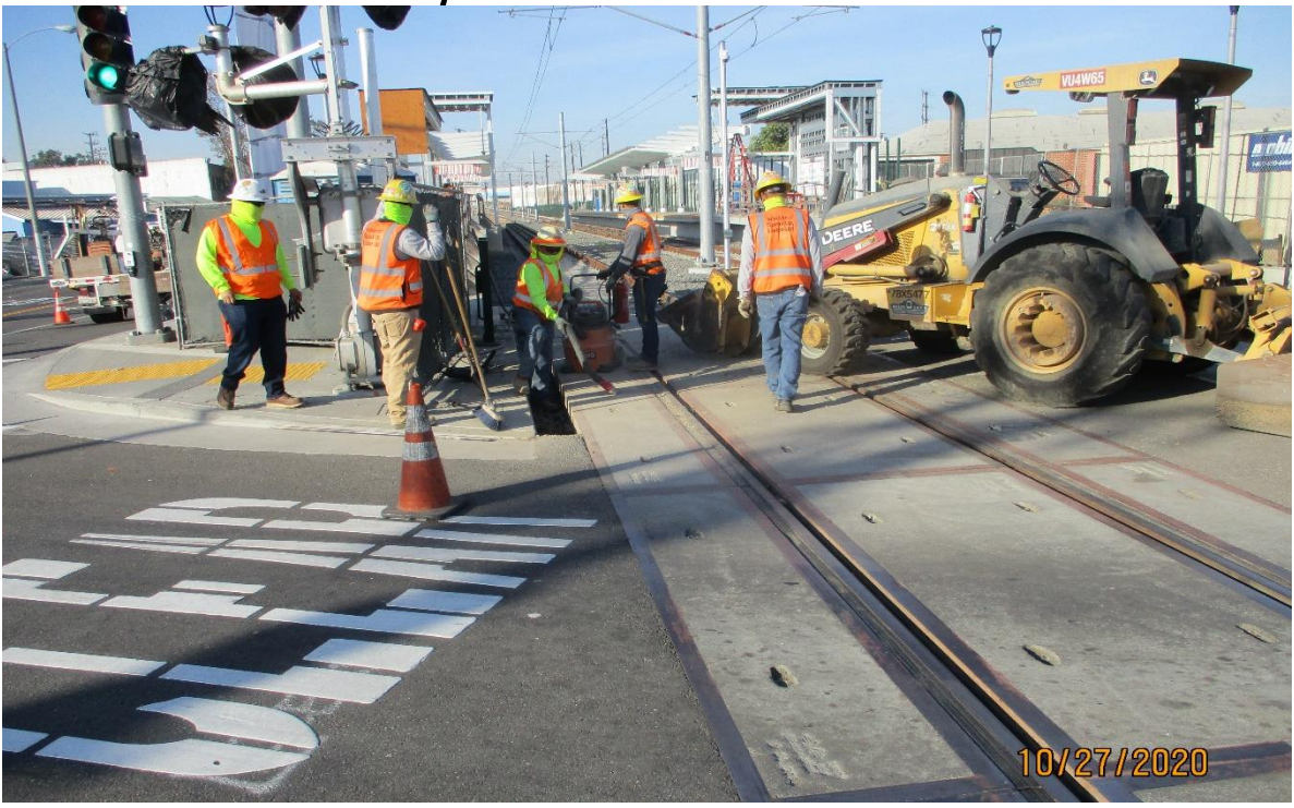
Hindry – Prep to slot pave at the Hindry crossing.
