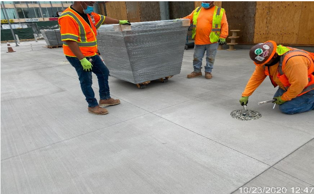
LEIMERT PARK STATION – Setting and installing planter pots throughout the plaza.
