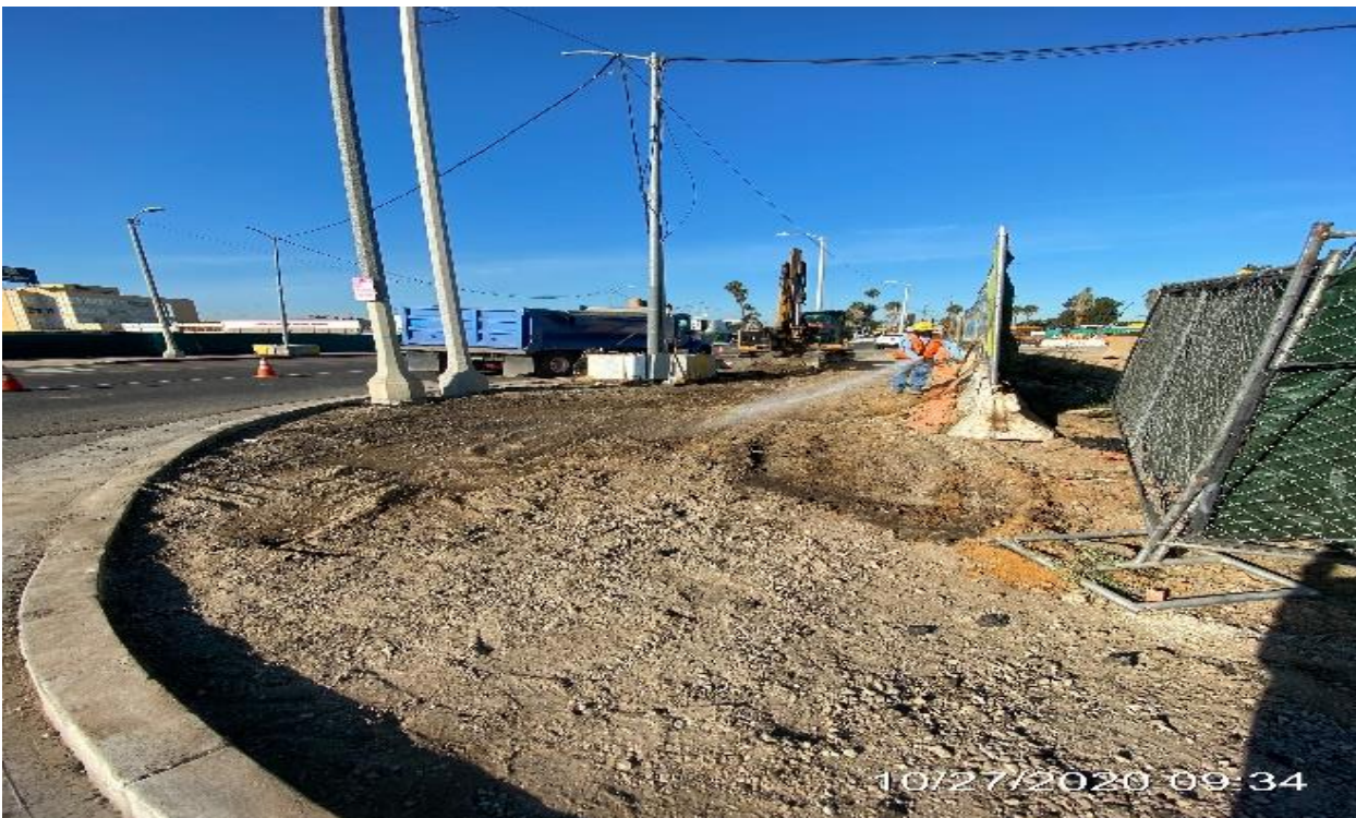
EXPO STATION – Excavating/grading sidewalk on westbound Obama Blvd and Crenshaw Blvd.
