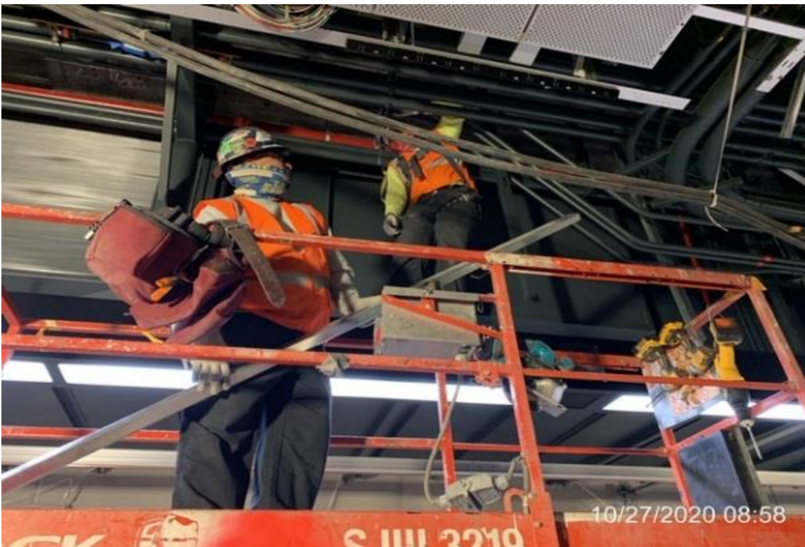
MLK STATION – PCI re-installing supports for angles ceiling panels.
