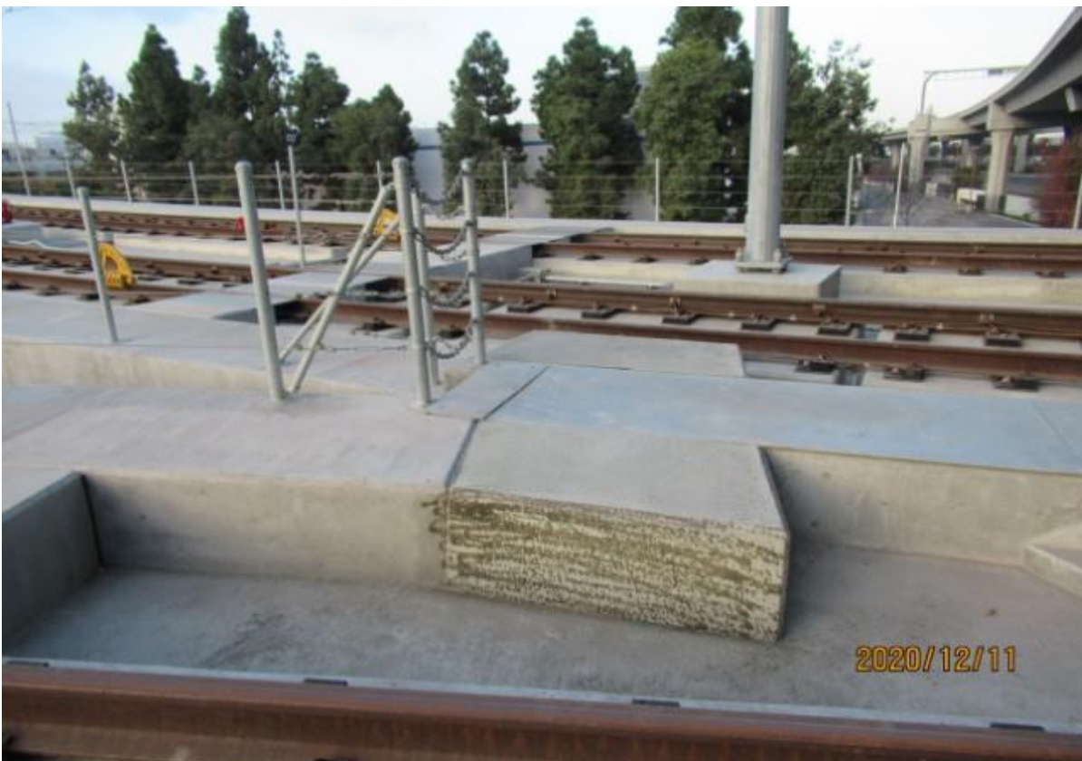
AVIATION/CENTURY- GL Wye STA 13+14 Emergency Walkway extension platform
