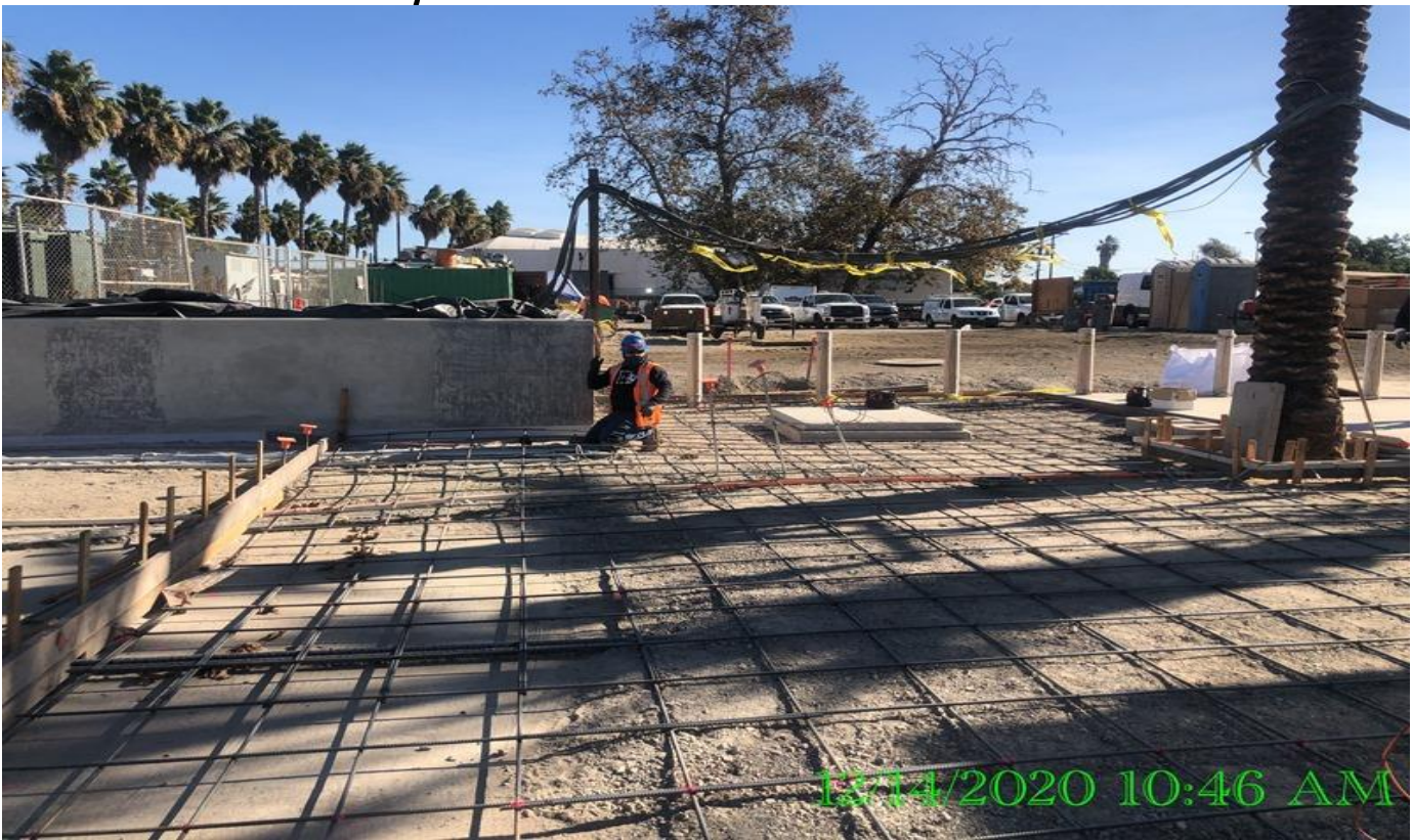
EXPO STATION – Continue ground grid system installation at the plaza.
