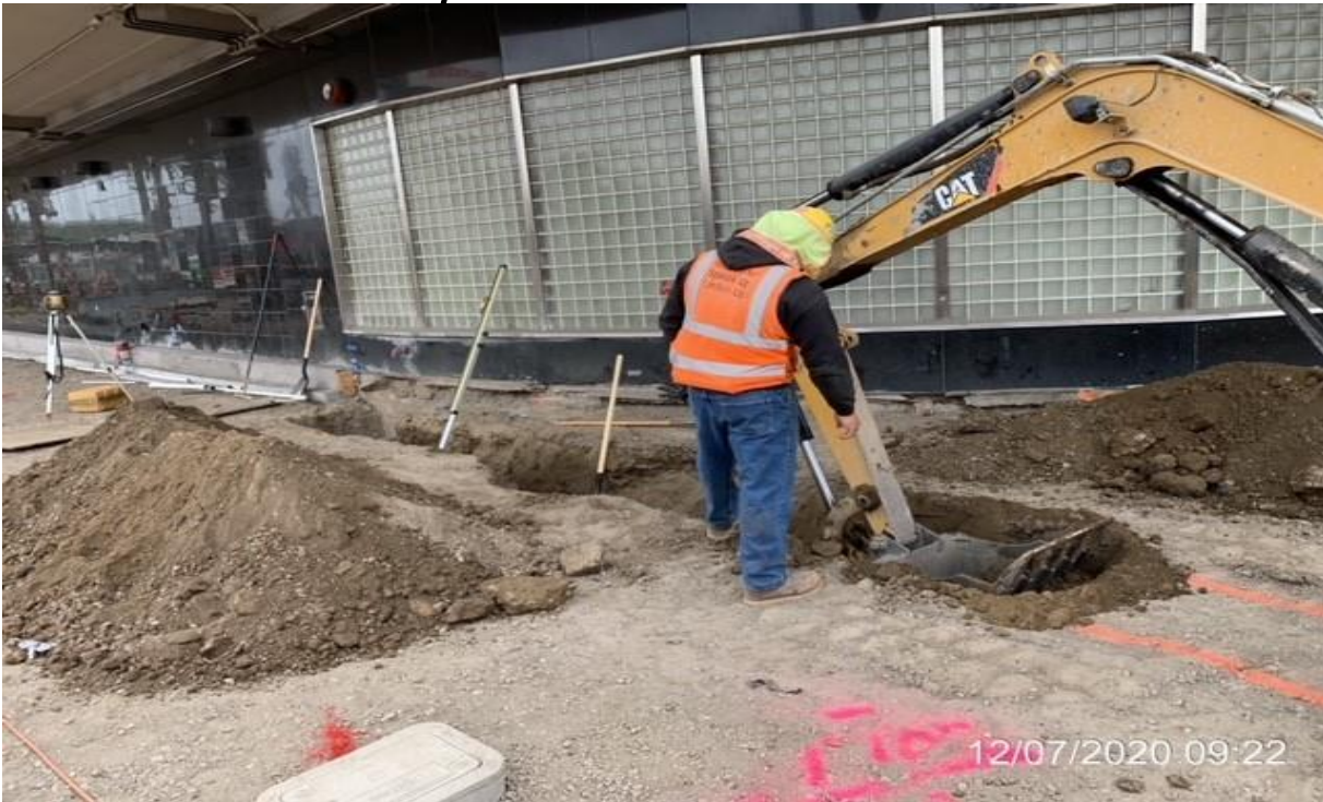
MLK STATION – WSCC excavating trench for gas line.
