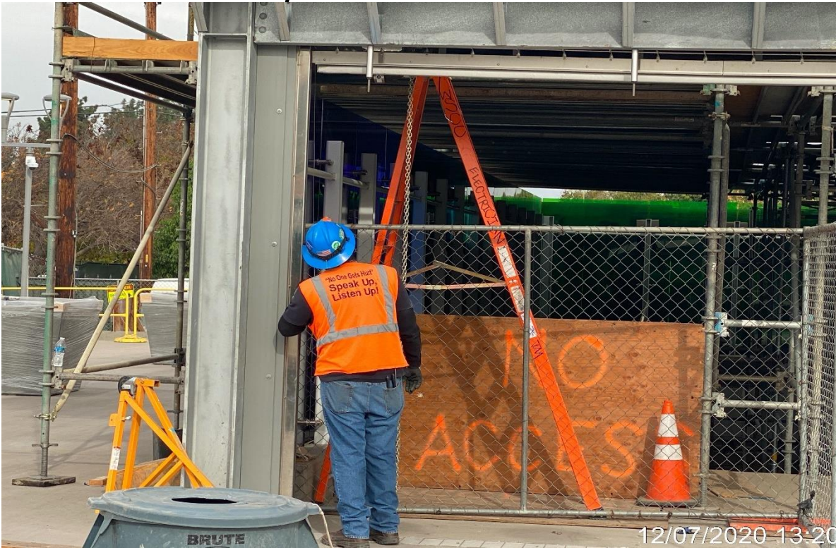
UG3 – WSCC working on roll up gate at Vernon plaza.
