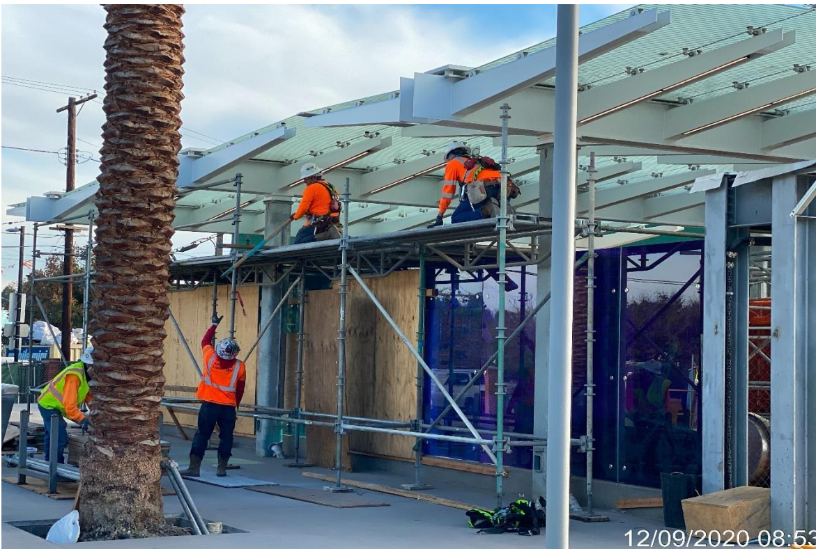
UG3 – Scaffolding being removed at entry portal of Vernon.
