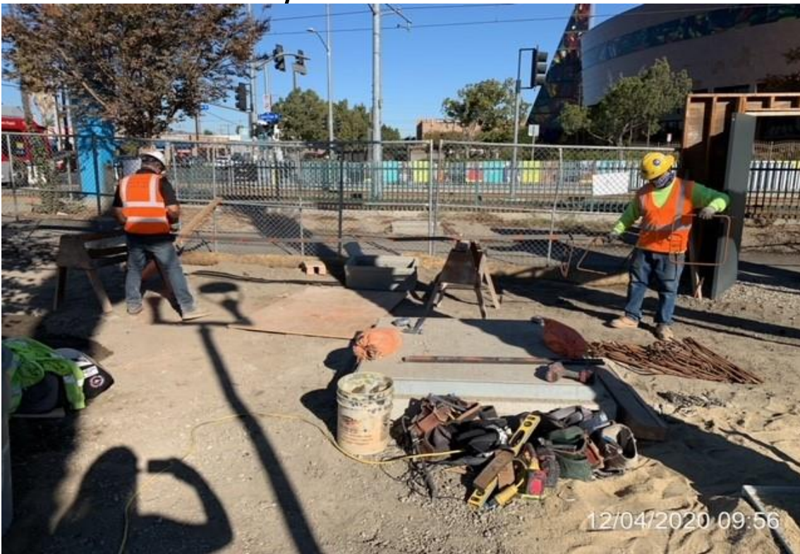
EXPO STATION – WSCC carpenters building formwork for bollards.
