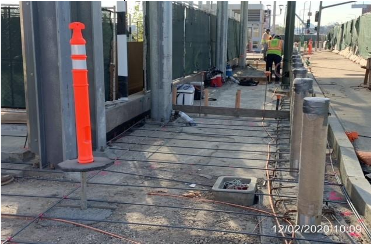
EXPO STATION– Dean Visosky setting rebar reinforcement for concrete slab.
