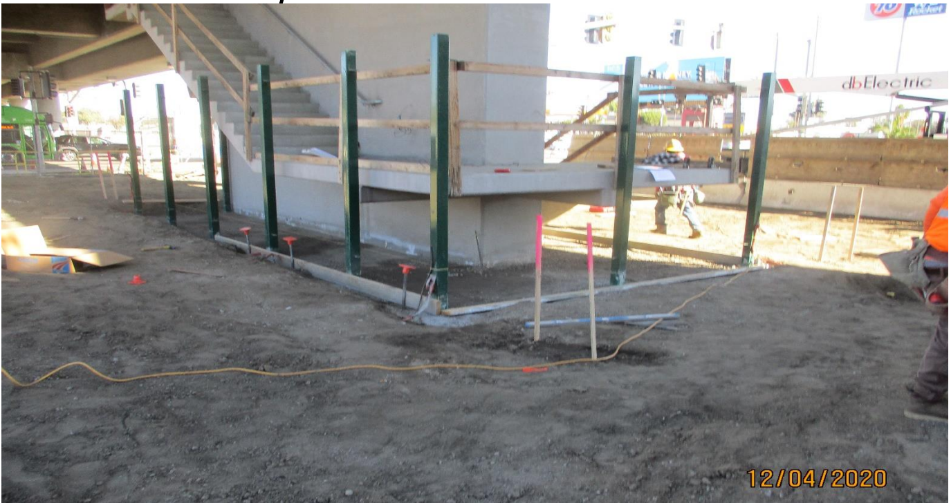
AVIATION/CENTURY- Setting forms for the hardscape concrete at the SW corner of Aviation and Century.
