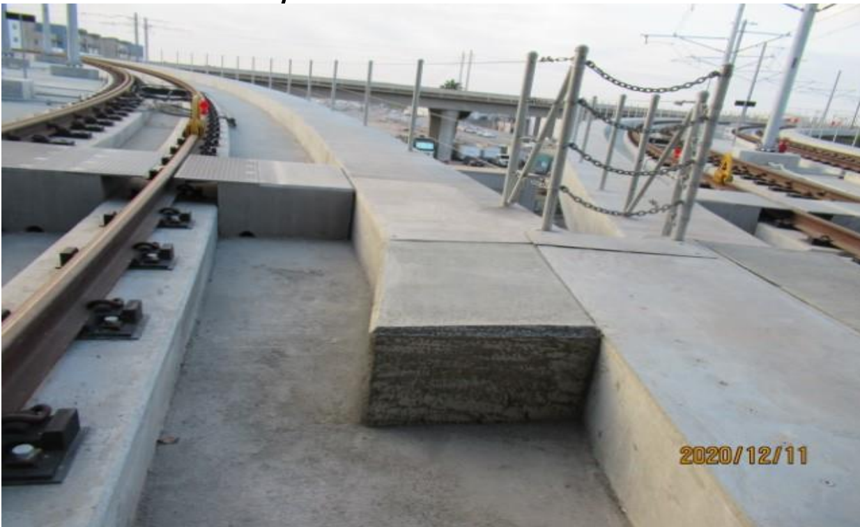
AVIATION/CENTURY - East leg of Wye WSCC placed extension on Emergency Walkway.
