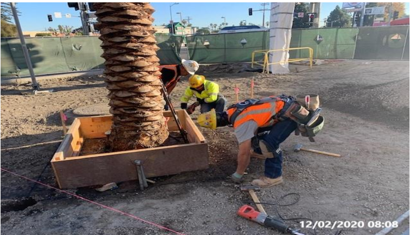
MLK STATION – WSCC carpenters building formwork for tree frames.
