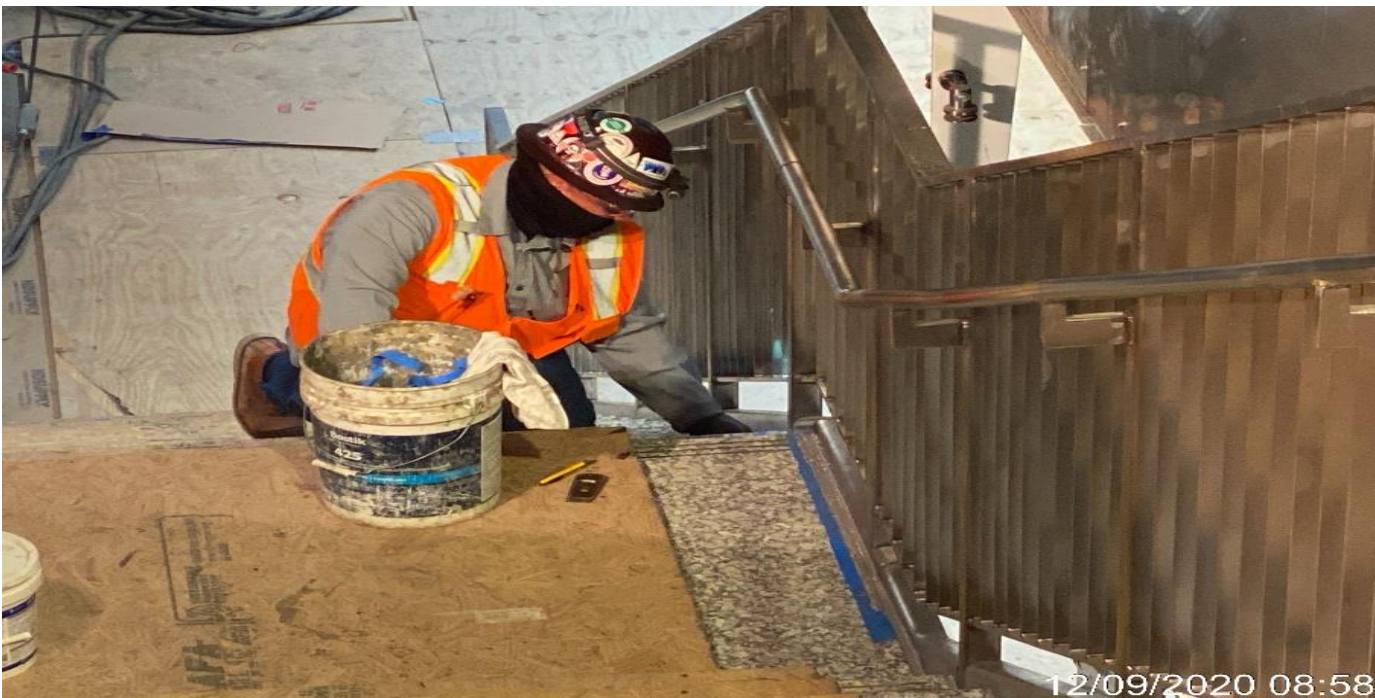
LEIMERT PARK STATION – Continue caulking and grouting the edges of Staircases 3 from concourse to platform.
