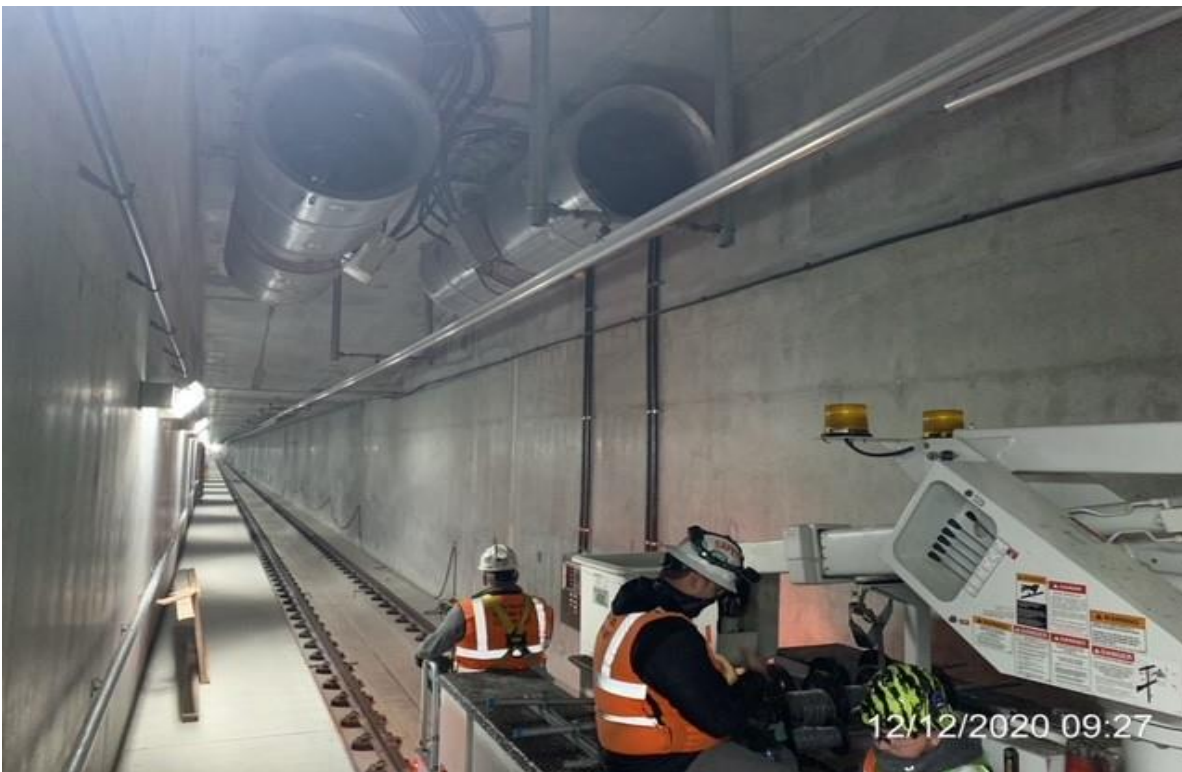
UG3 – Start-up crew running mechanical tests on booster fan.
