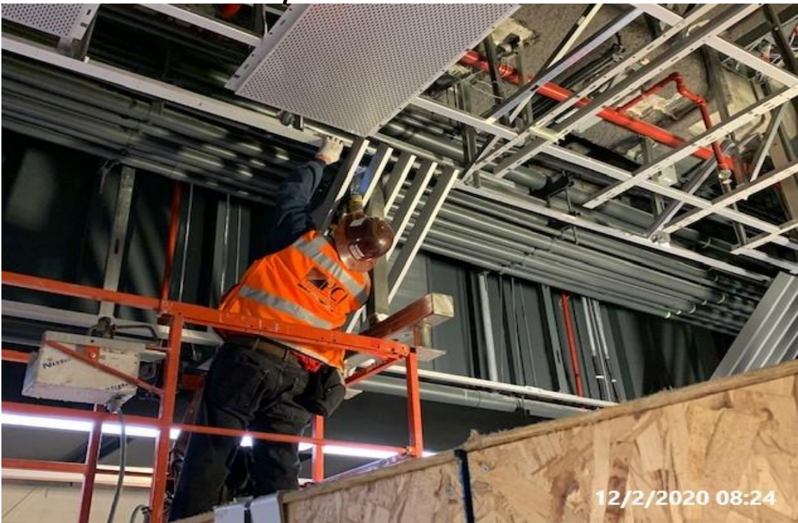
MLK STATION – PCI re-installing “Barz” angle panels
