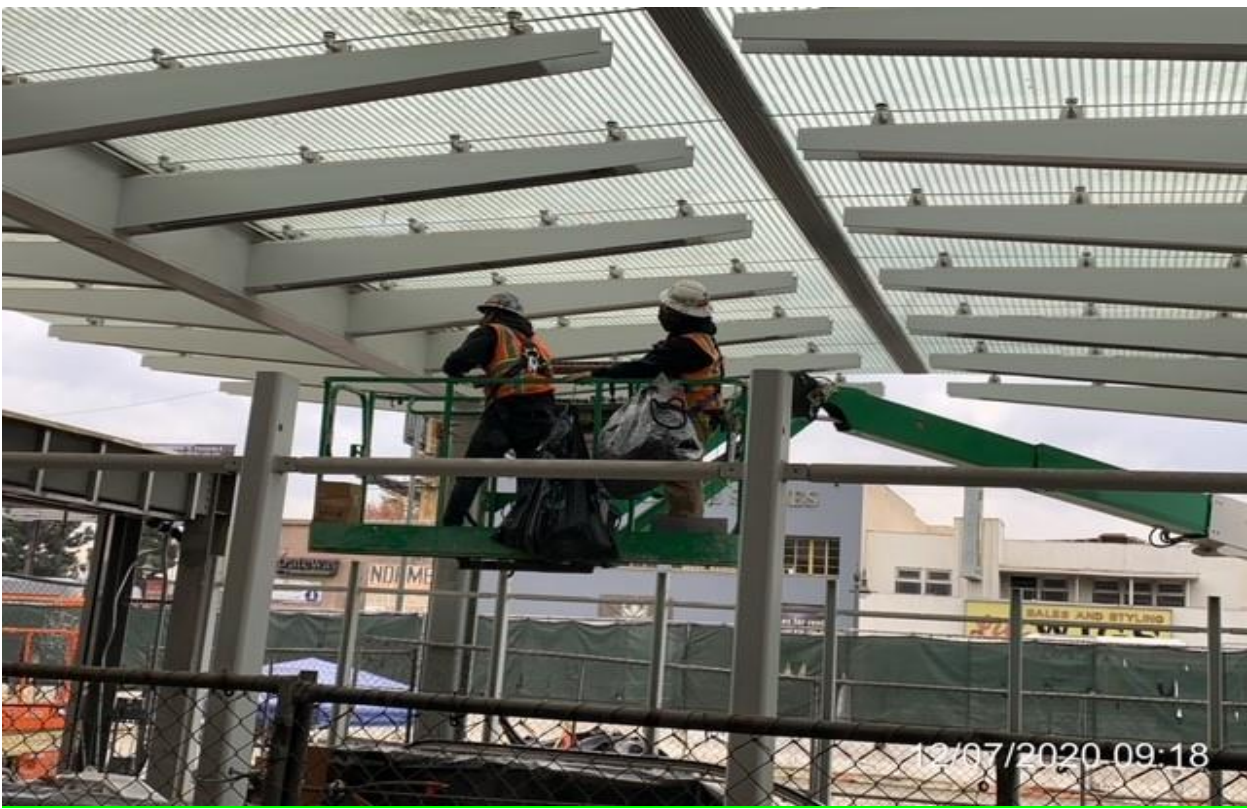
MLK STATION – VNSM applying caulking to Boca light fixtures.
