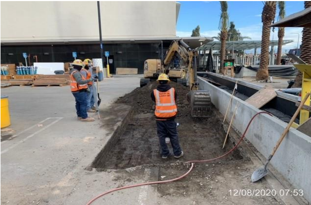
MLK STATION – WSCC crew excavating for curb and gutter.
