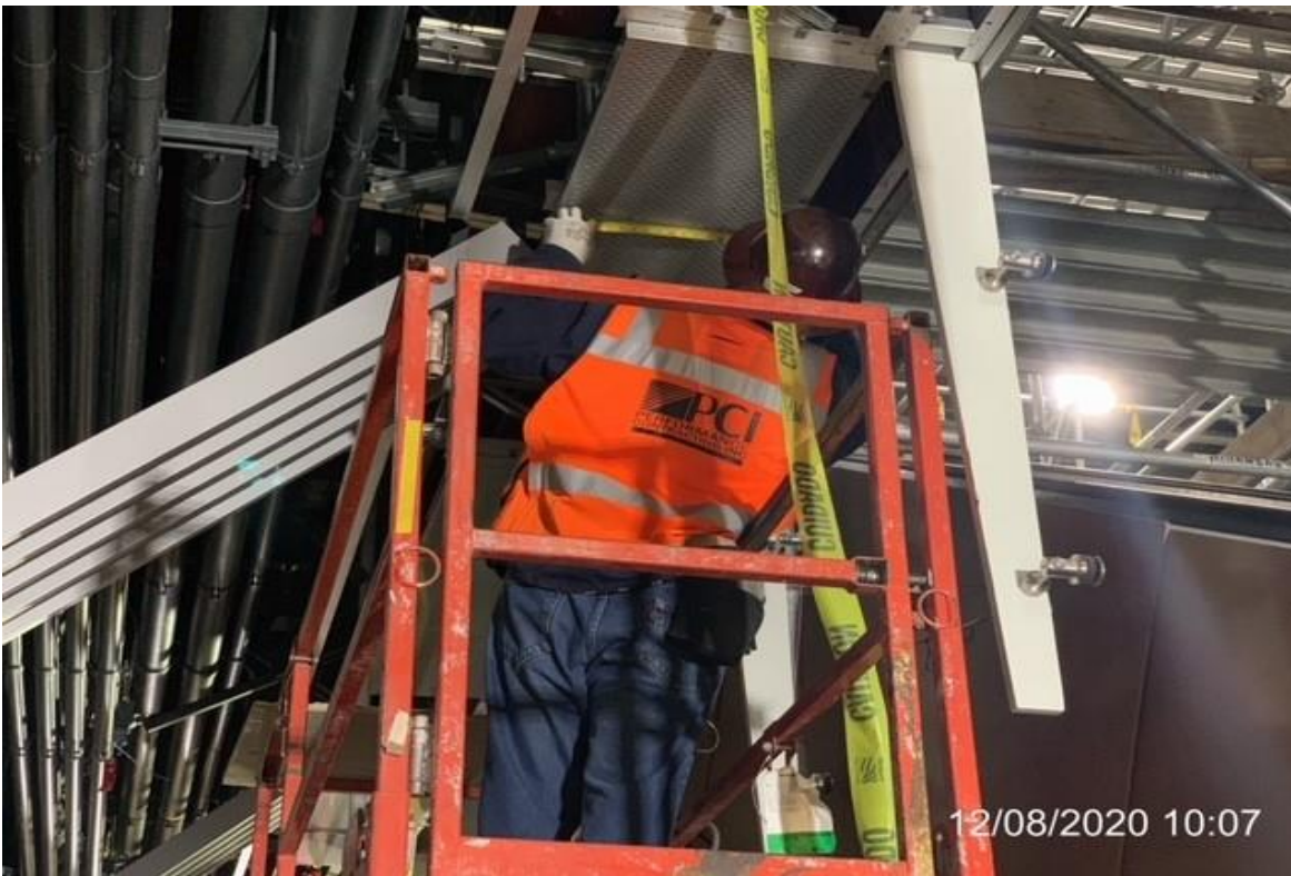
EXPO STATION– PCI taking field dimensions for custom ceiling panels.
