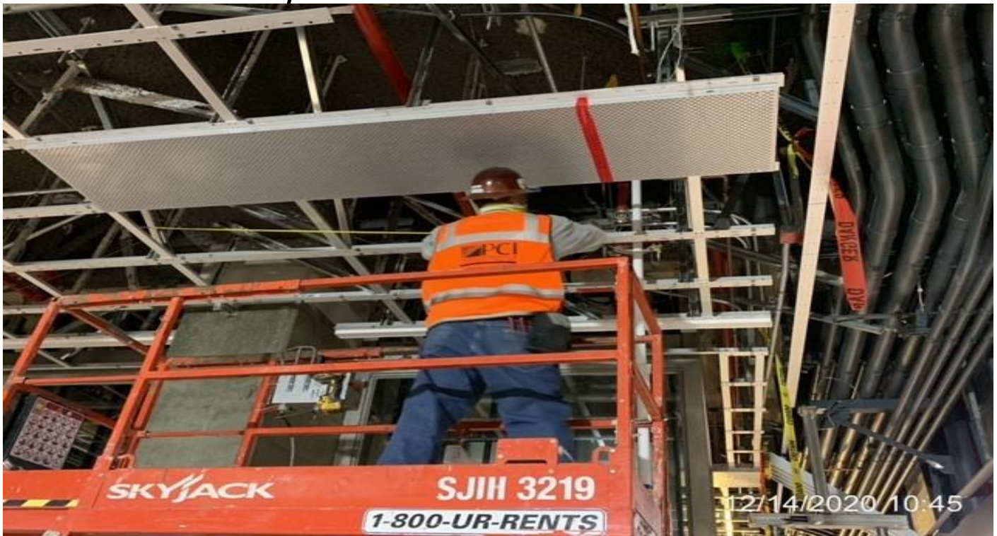
EXPO STATION – Resume perforated ceiling panel installation throughout the platform.
