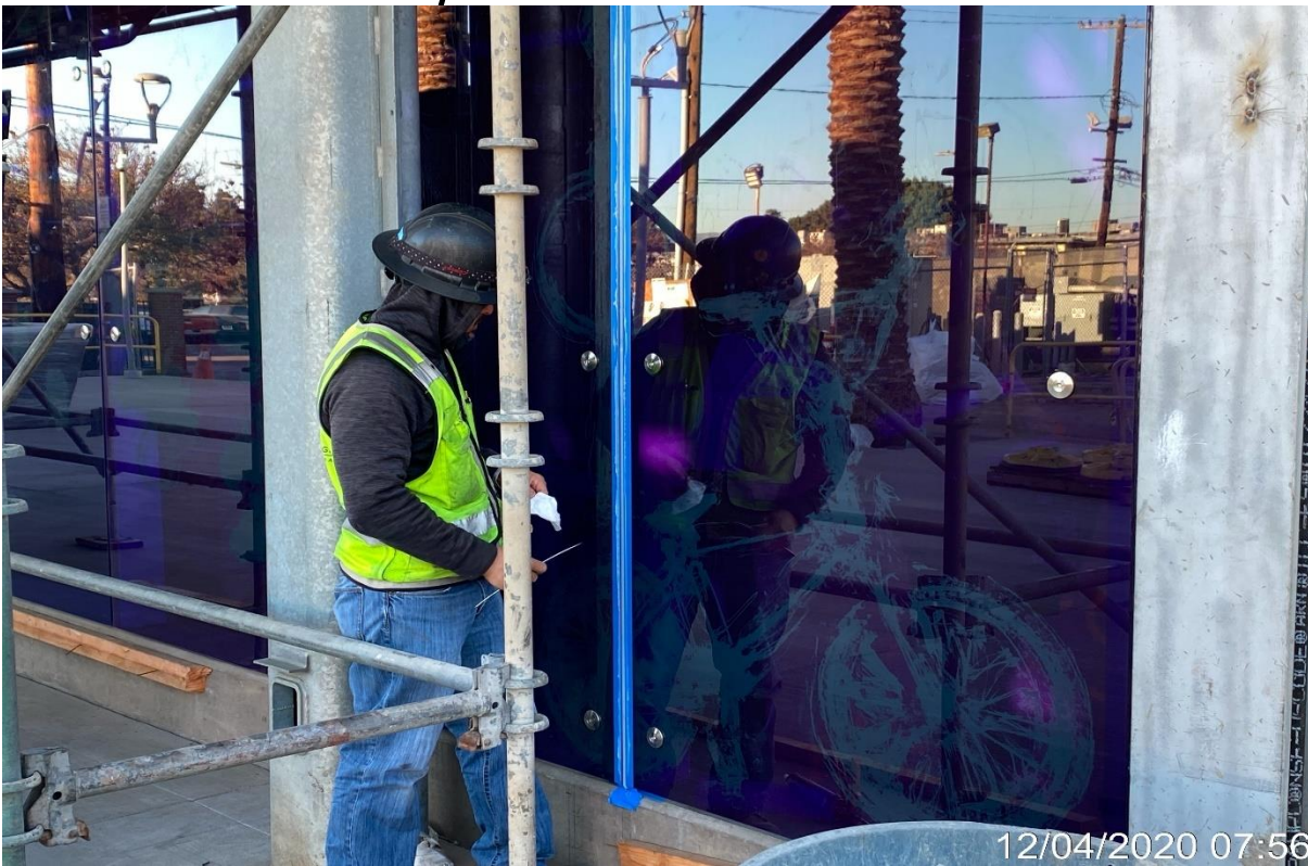
UG3 – Giroux caulking the art glass at Vernon plaza.
