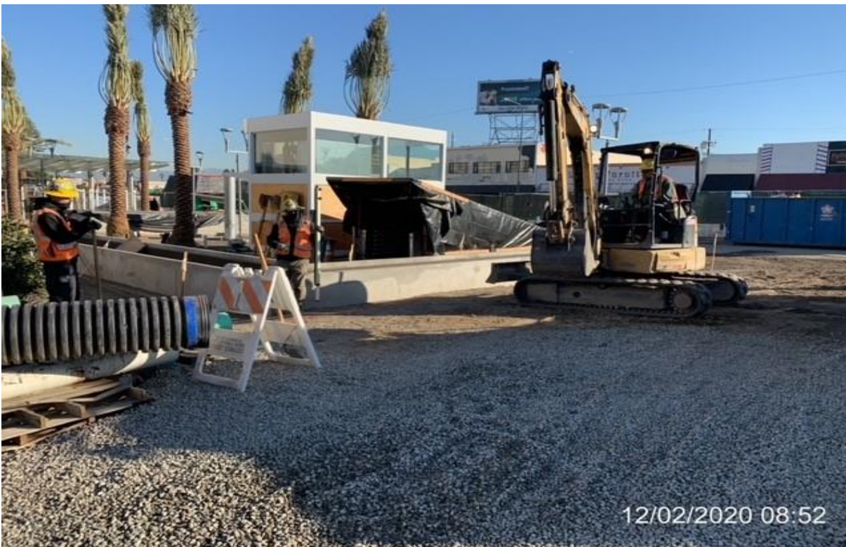
MLK STATION – WSCC crew excavating trench for curb.
