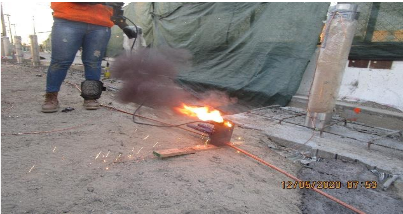
EXPO STATION – Continue ground grid system installation at the plaza.
