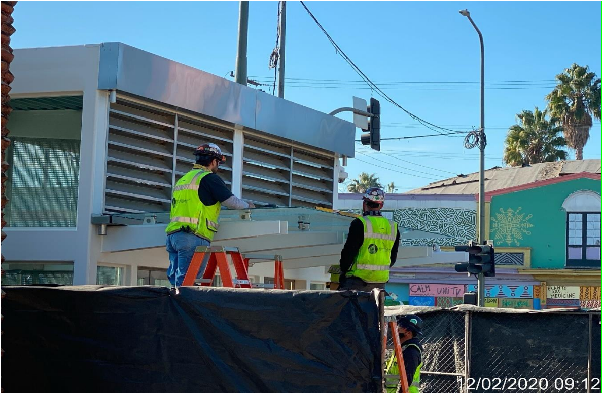
UG3 – Giroux installing Elevator glass at Vernon plaza.
