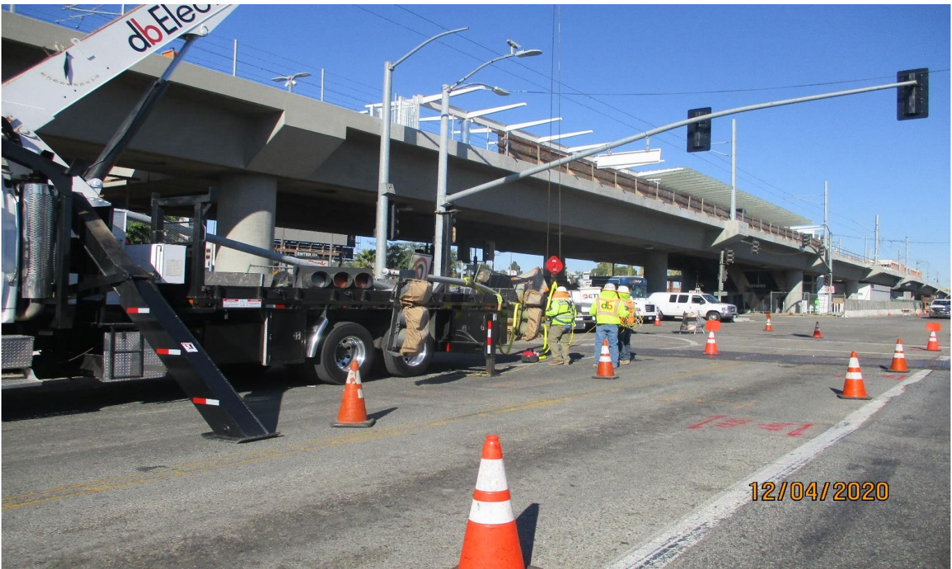
AVIATION/CENTURY- Traffic signal pole removal at Aviation and Century.
