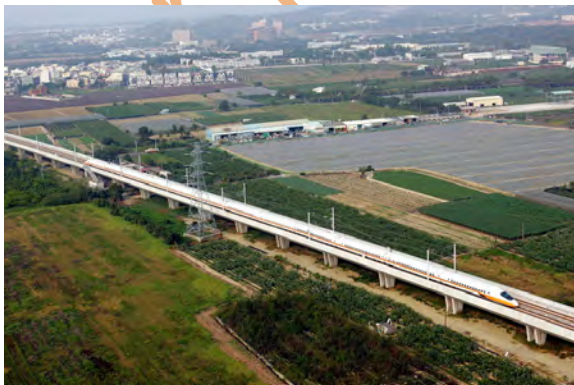
Taiwan's high-speed rail system operates on elevated structure to accommodate land use.
