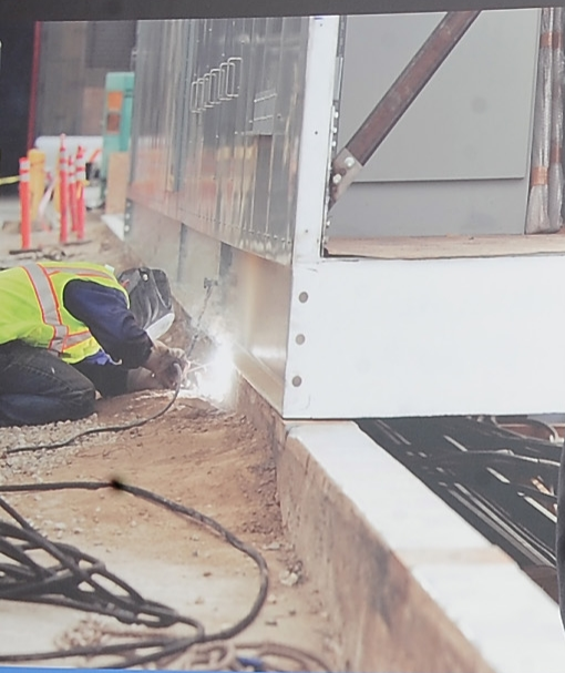
Welding of New Traction Power Substation.
