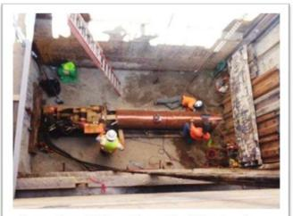
Bore pit on Victory Pl. north of Empire Ave. The pit is about 30' deep and 20' wide. It will be used to install a 24" steel casing and plastic conduits that will house communication lines.
