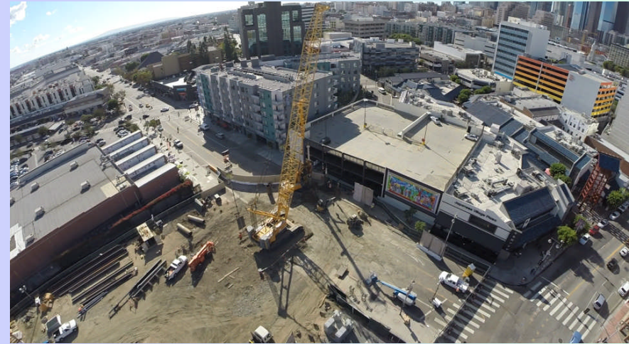
Construction Activities at 1 st /Central Station yard
