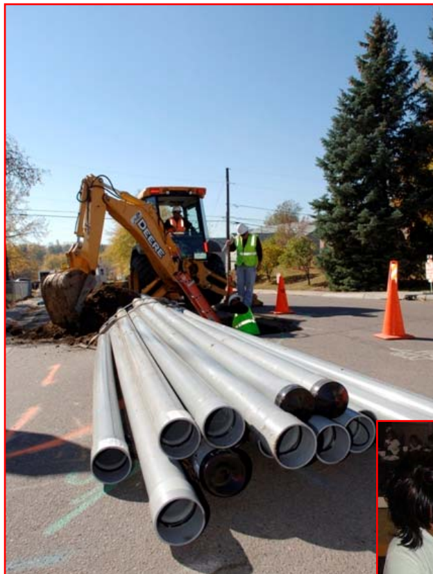
West Corridor construction crews prepare to relocate utilities – November 2007
