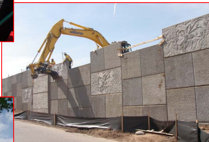
West Corridor retaining walls being erected along Kipling Street – May 2009
