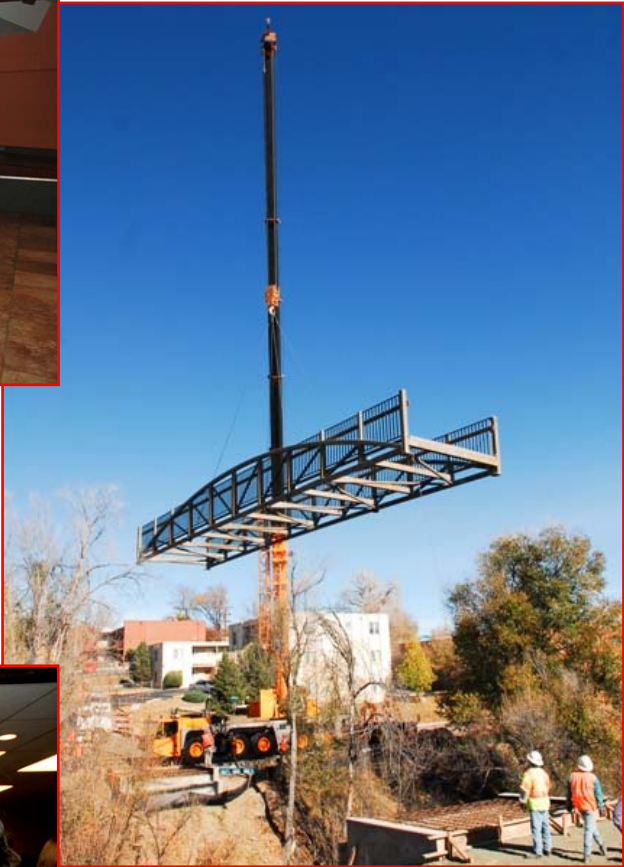
Placing a pedestrian bridge on the West Corridor – November 2008
