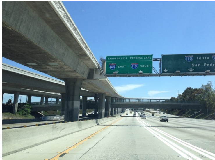
Figure 12: Photo of Existing I-110/I-105 HOV/HOT Direct Connectors
