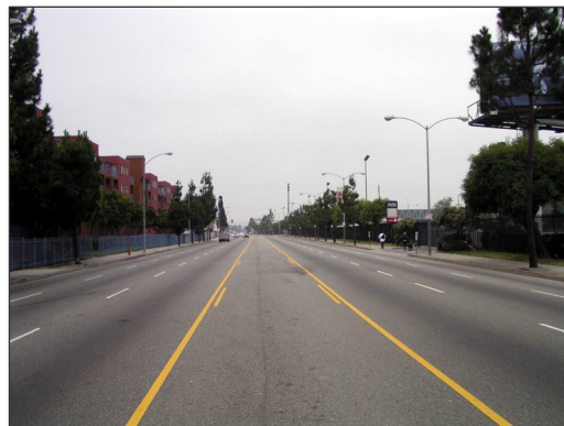
Martin Luther King Boulevard, facing west
