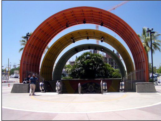
North Hollywood Metro Red Line station
