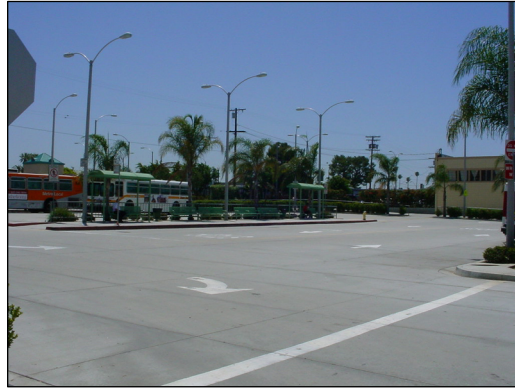
Inglewood Bus Center bus turnaround
