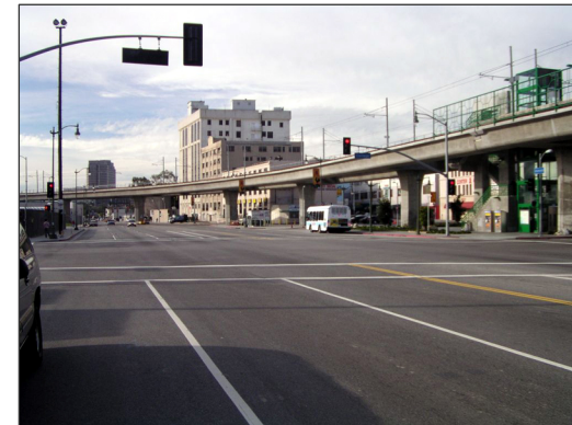
Alameda Street facing south across College Avenue
