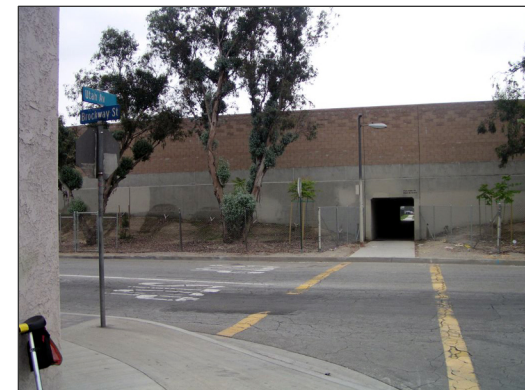
Pedestrian undercrossing at Utah Avenue and the 10 freeway
