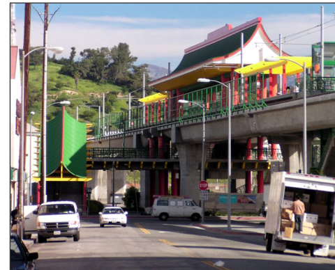
Spring Street facing north towards station
