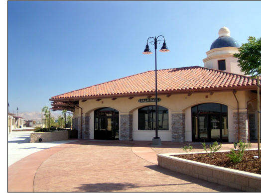
Palmdale Transportation Center
