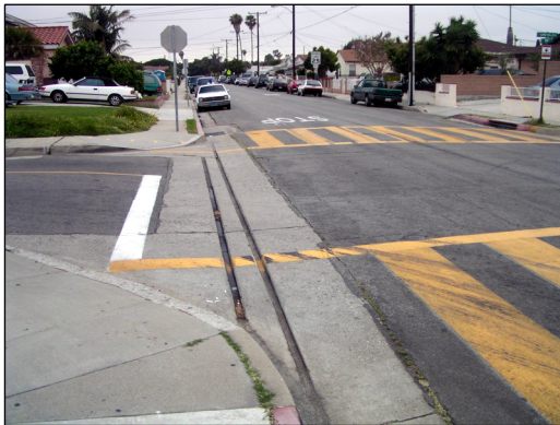
Slots in the valley gutters at Grevillea Avenue and 166 th Street
