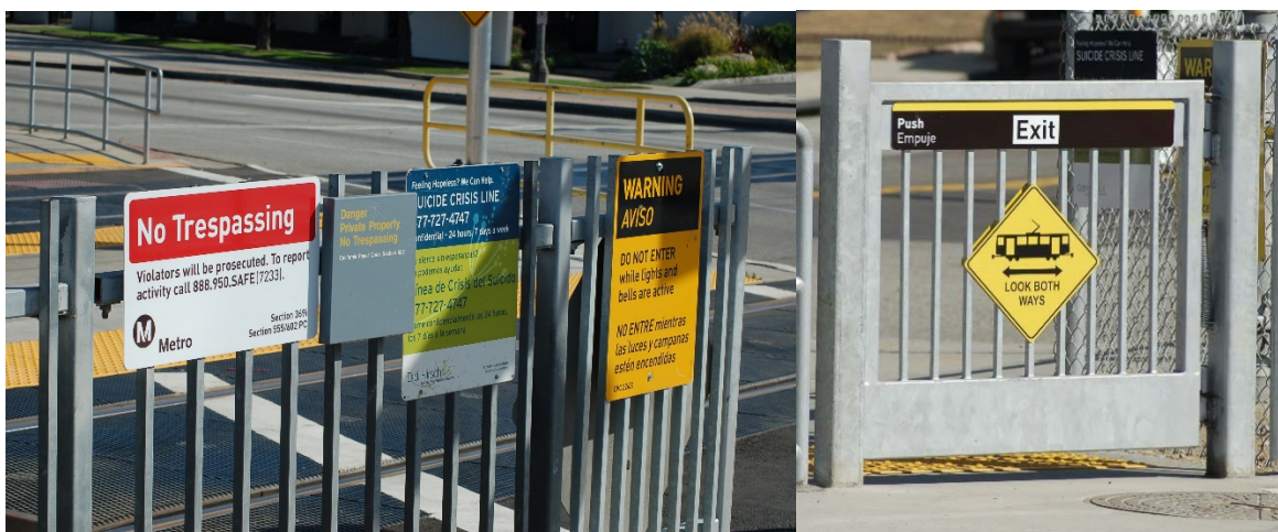
Figure 5. - Wardlow pedestrian gates and signs.
