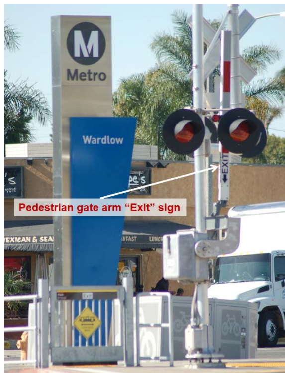
Figure 4. - Pedestrian gate arm "Exit" sign pointing to the pedestrian exit gate.
