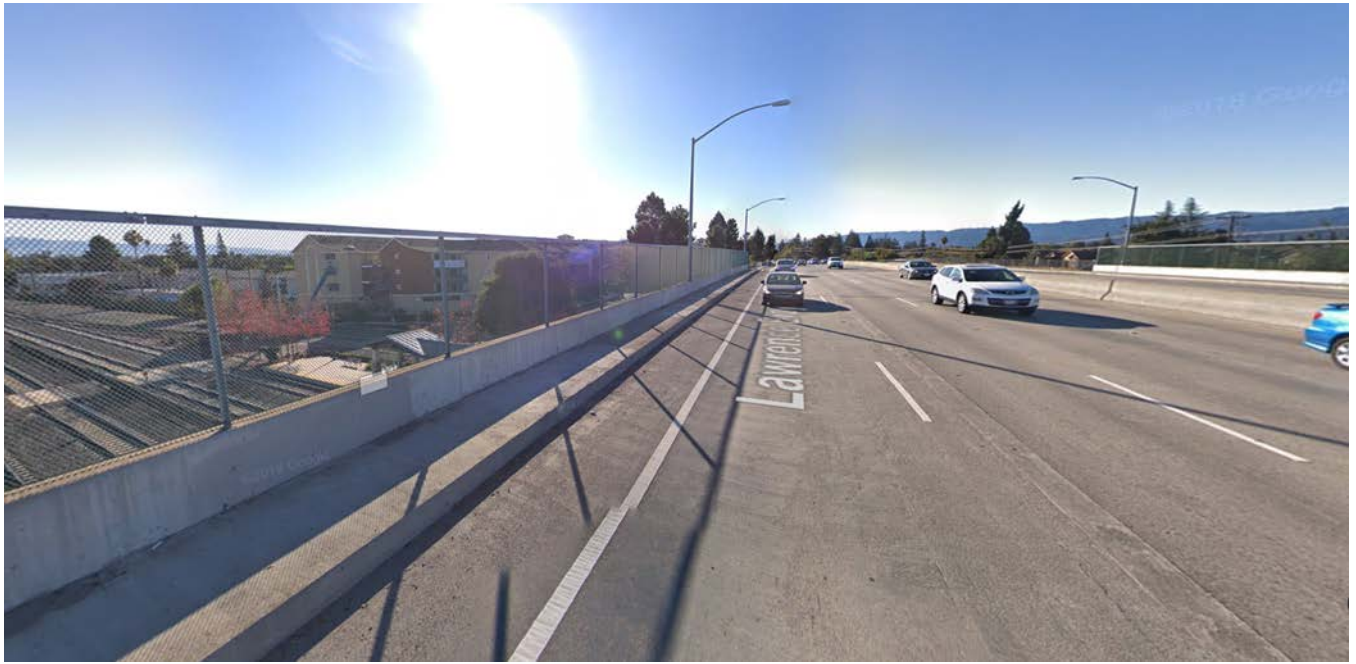
Figure 5. - The long climbing sidewalk along Lawrence Expwy Overhead Structure City of San Jose, CA
