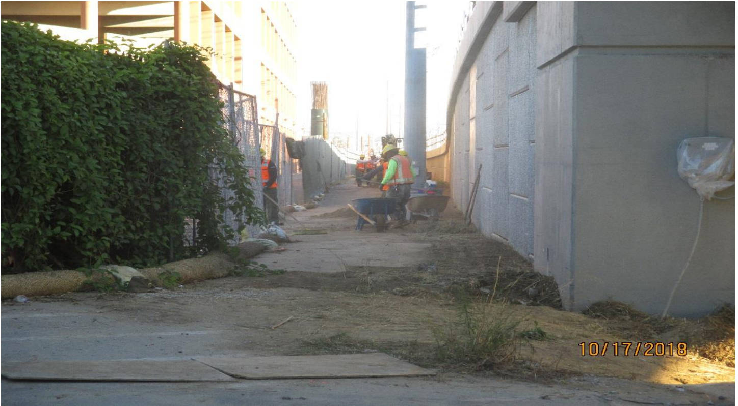
MSE 75L&R- Grading along the SB side of RW #75.
