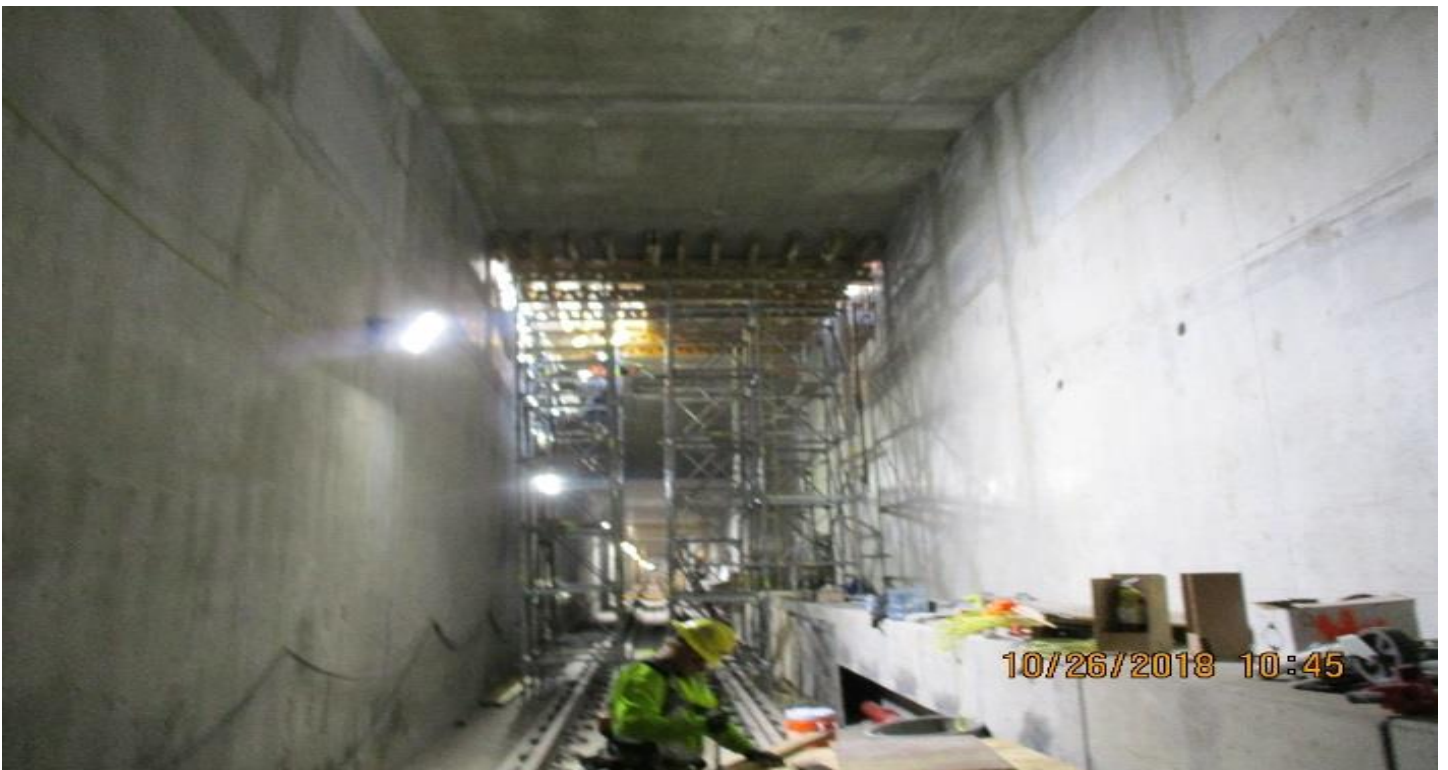
UG3 - Installation of falsework for the roof at section 69.
