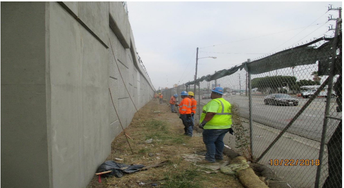
MSE 75L&R- Grubbing and grading at the NB side of RW #75.
