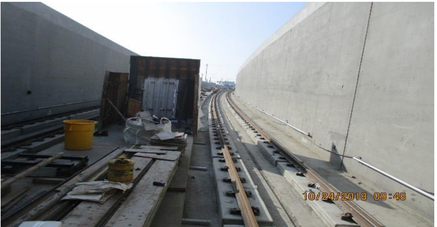
UG4 – Tracks at the south portal looking south.
