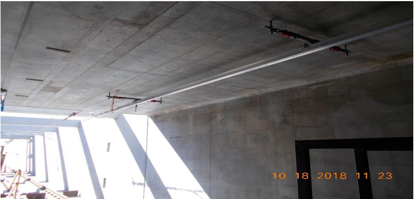
UG1- Installing OCR on track 3.
