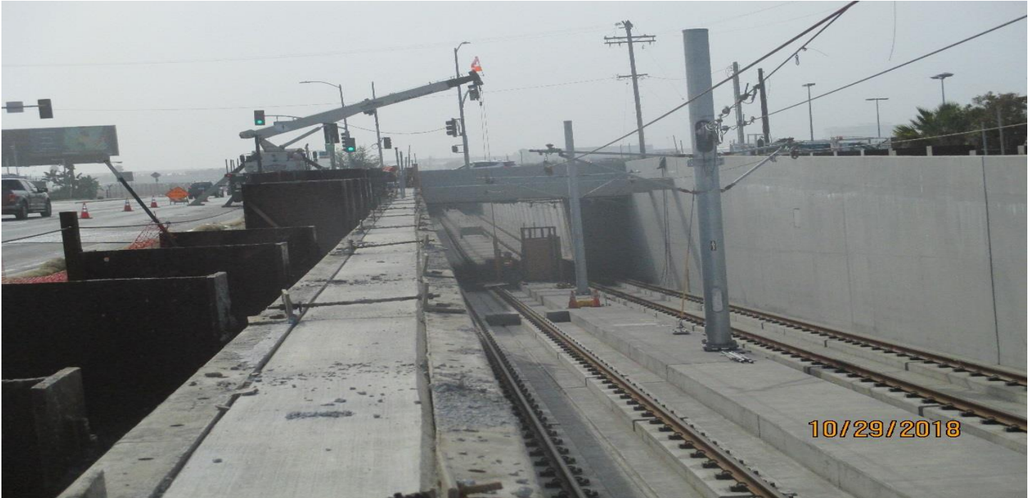
UG1- Installation of the security gates at UG-1
