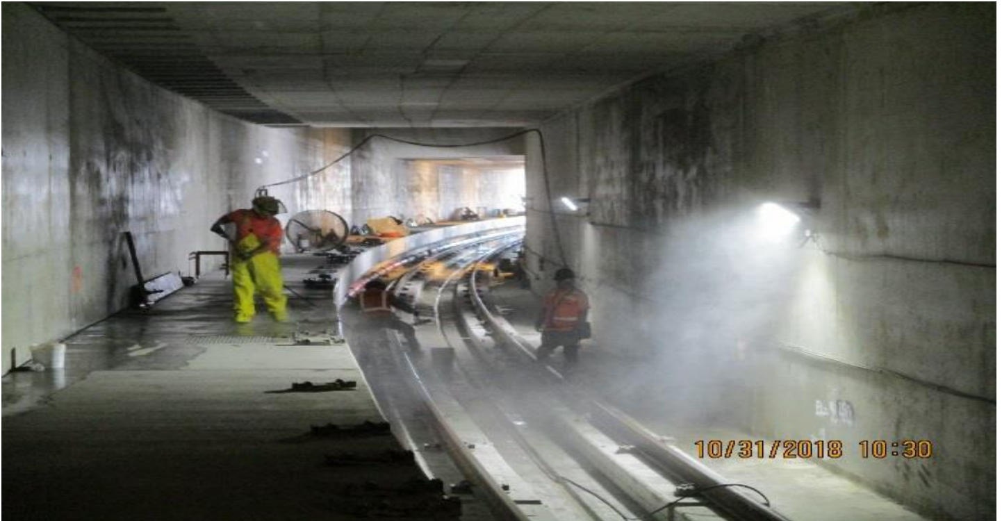
UG4 – Pressure washing plinths and emergency walkway in the SB tunnel.
