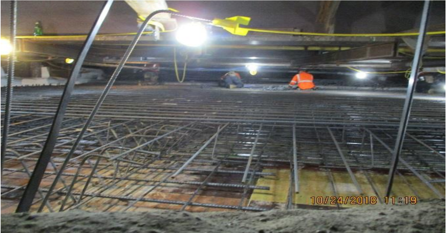
UG3 - Installation of rebar at the roof deck at section P-69.
