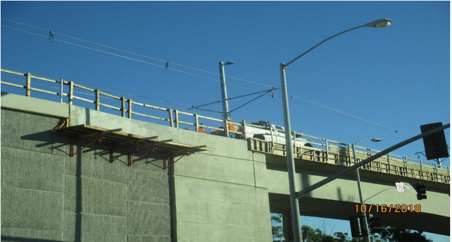
MSE 140L&R- Cable railing installation at RW #140.
