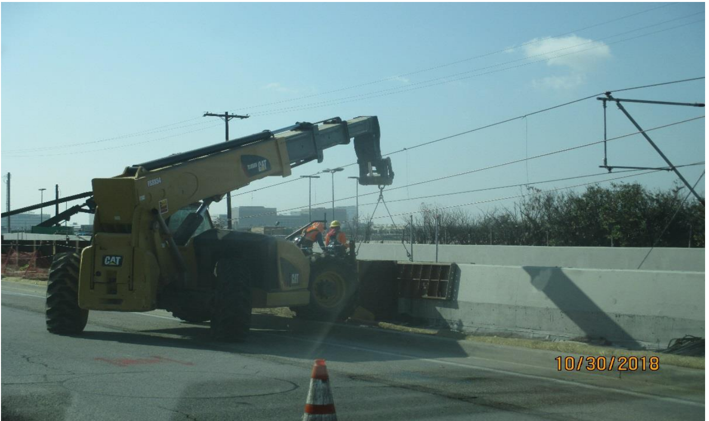
UG1- Stripping barrier wall forms at UG-1.
