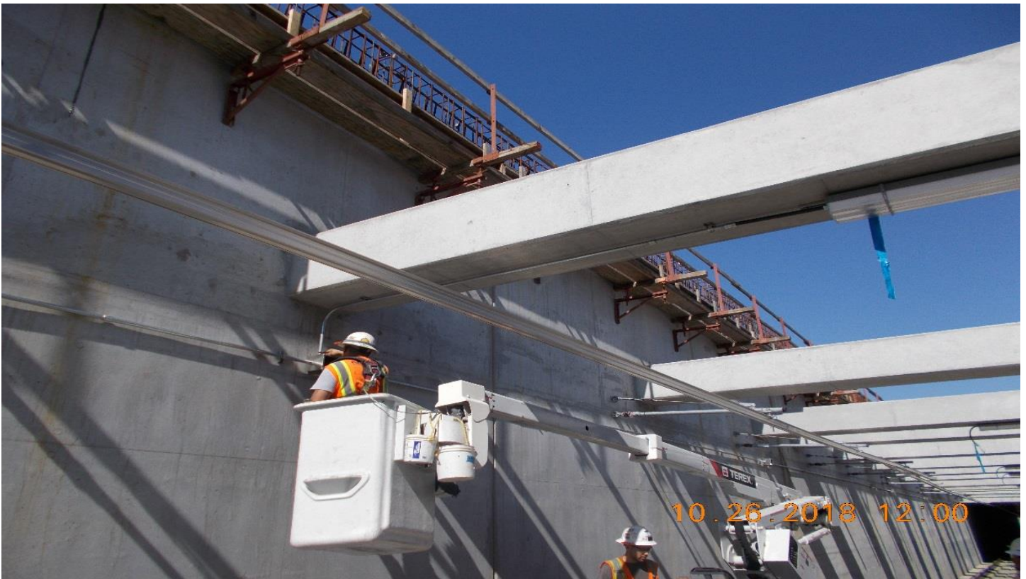
UG1- Running 1 inch IMC branch conduit.
