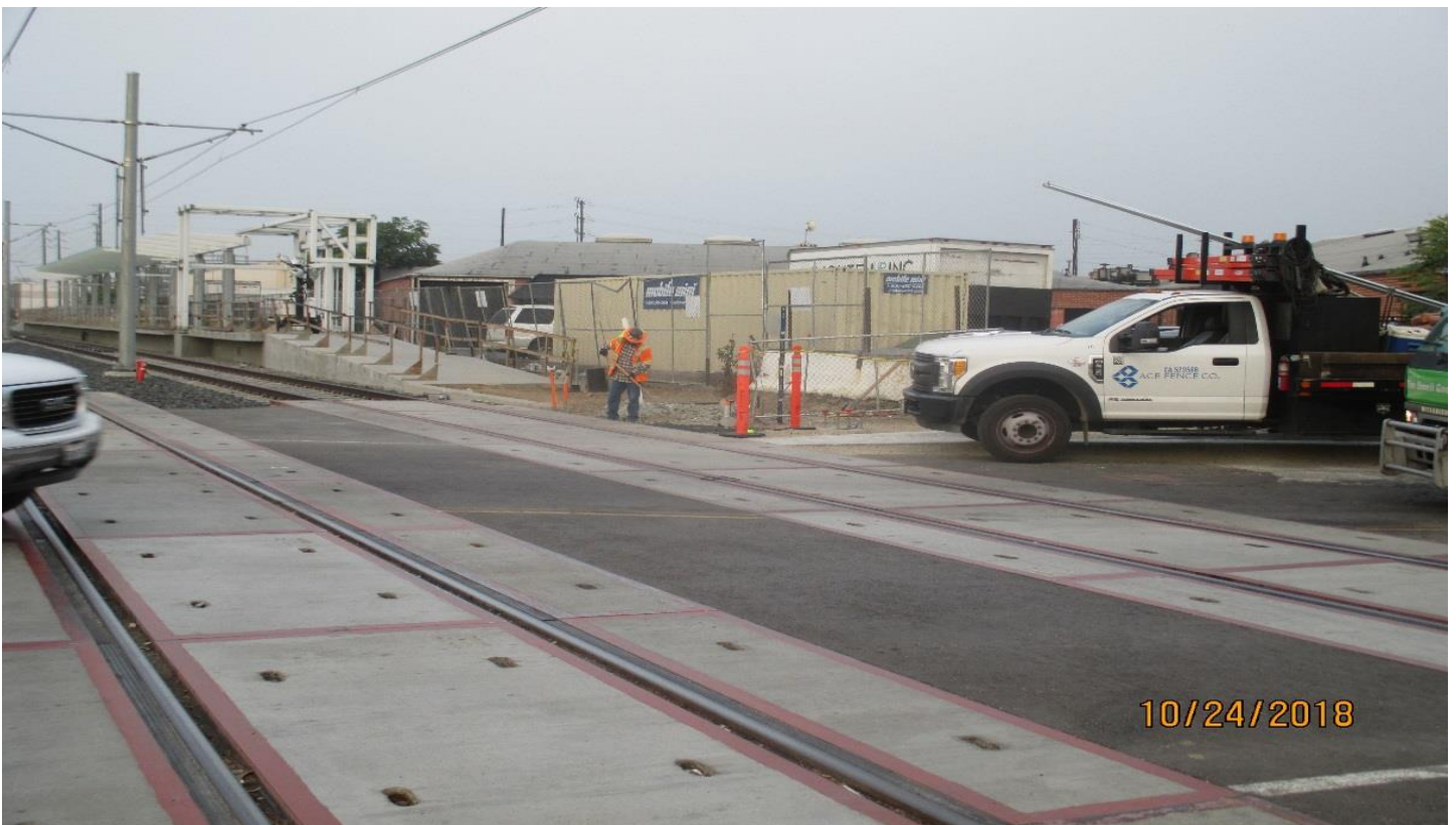
B1 GUIDEWAY - Setting crossing gate posts at Hindry.
