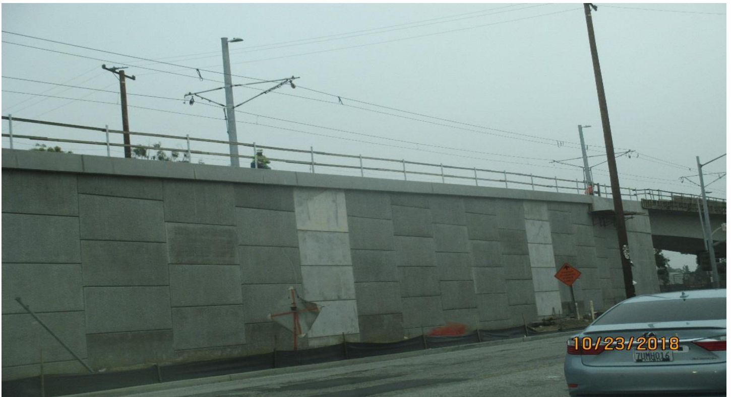
MSE 140L&R- Stringing cable for the cable railing fence on RW #140.
