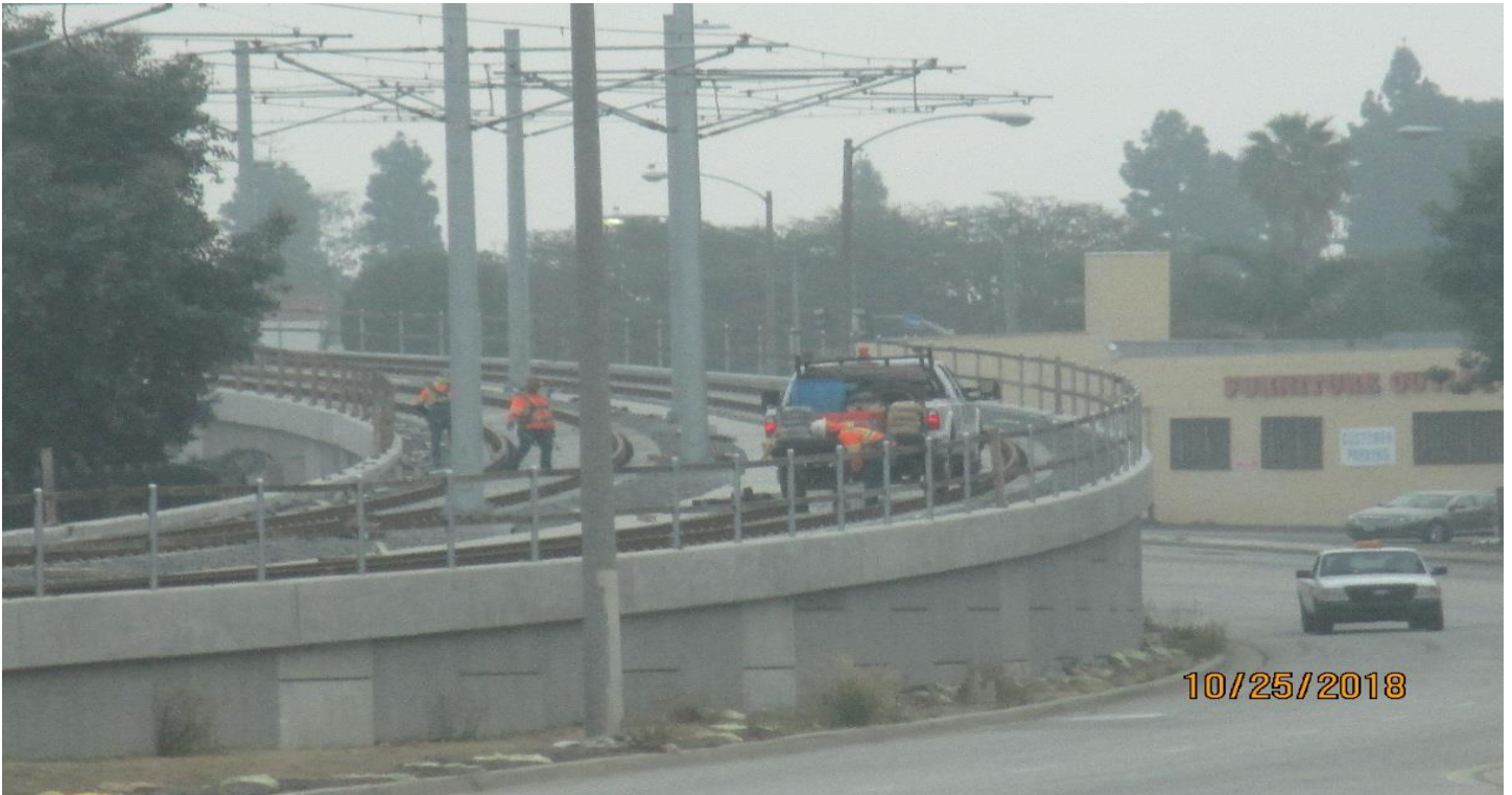
MSE 192L&R- Cable railing installation at RW #192.
