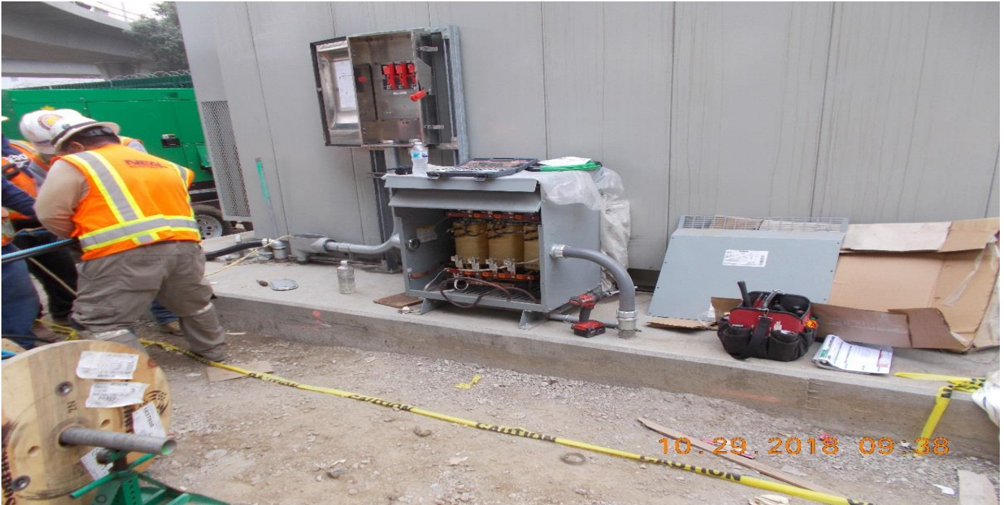
TPSS- TPSS #1- Pulling 3 - 250's + a ground to feed the TC&C bungalow.
