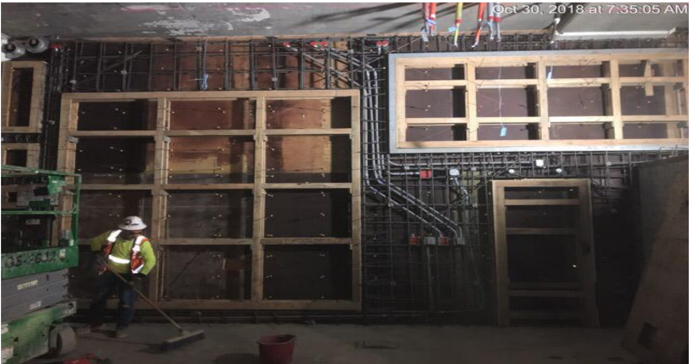
EXPOSITION/CRENSHAW STATION – Installation of blockout formwork at wall G60.
