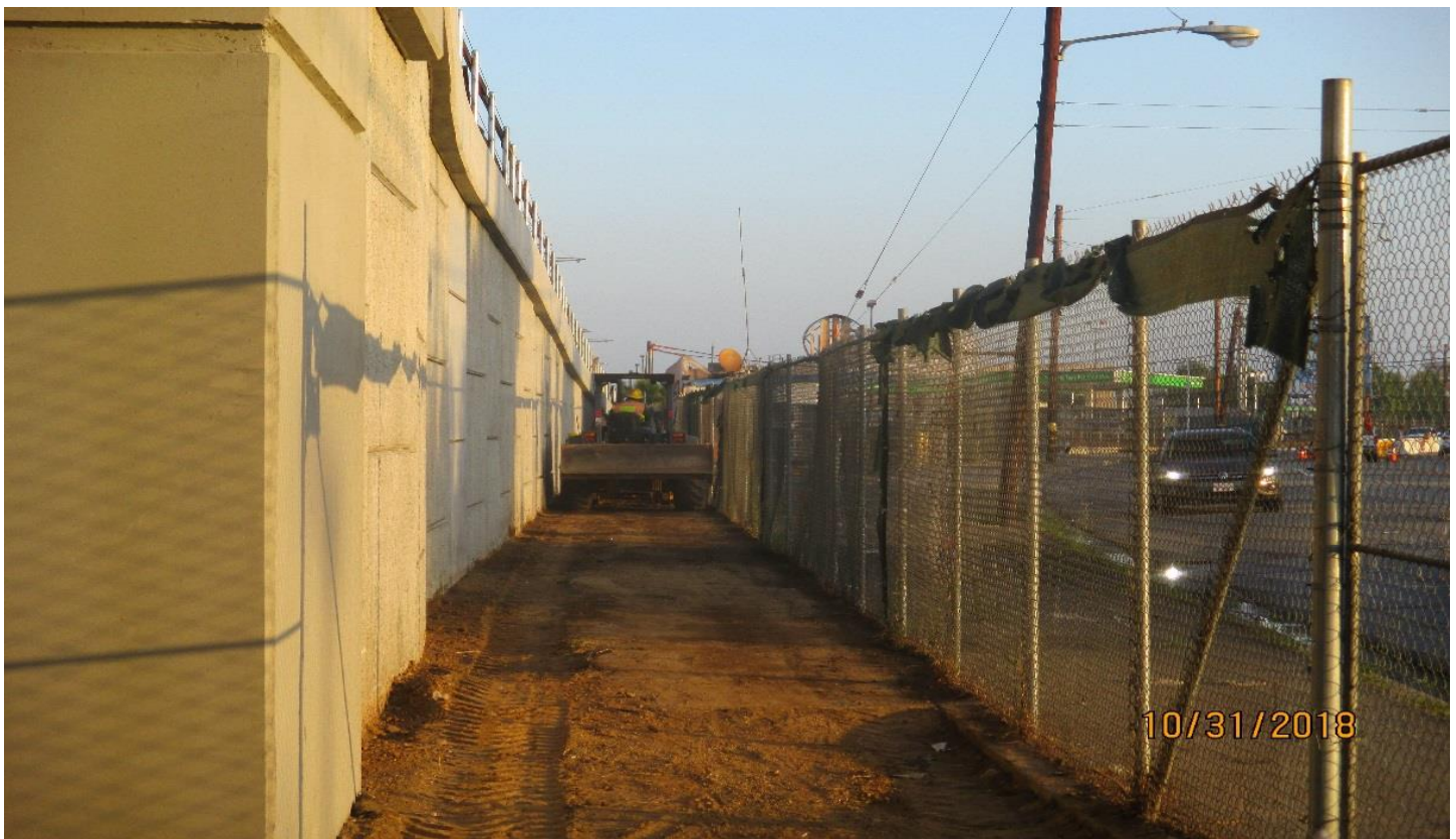
MSE 75L&R- Rough grading on the NB side of RW #75.
