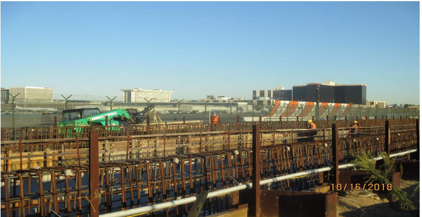
UG1- Setting barrier wall forms for UG-1.
