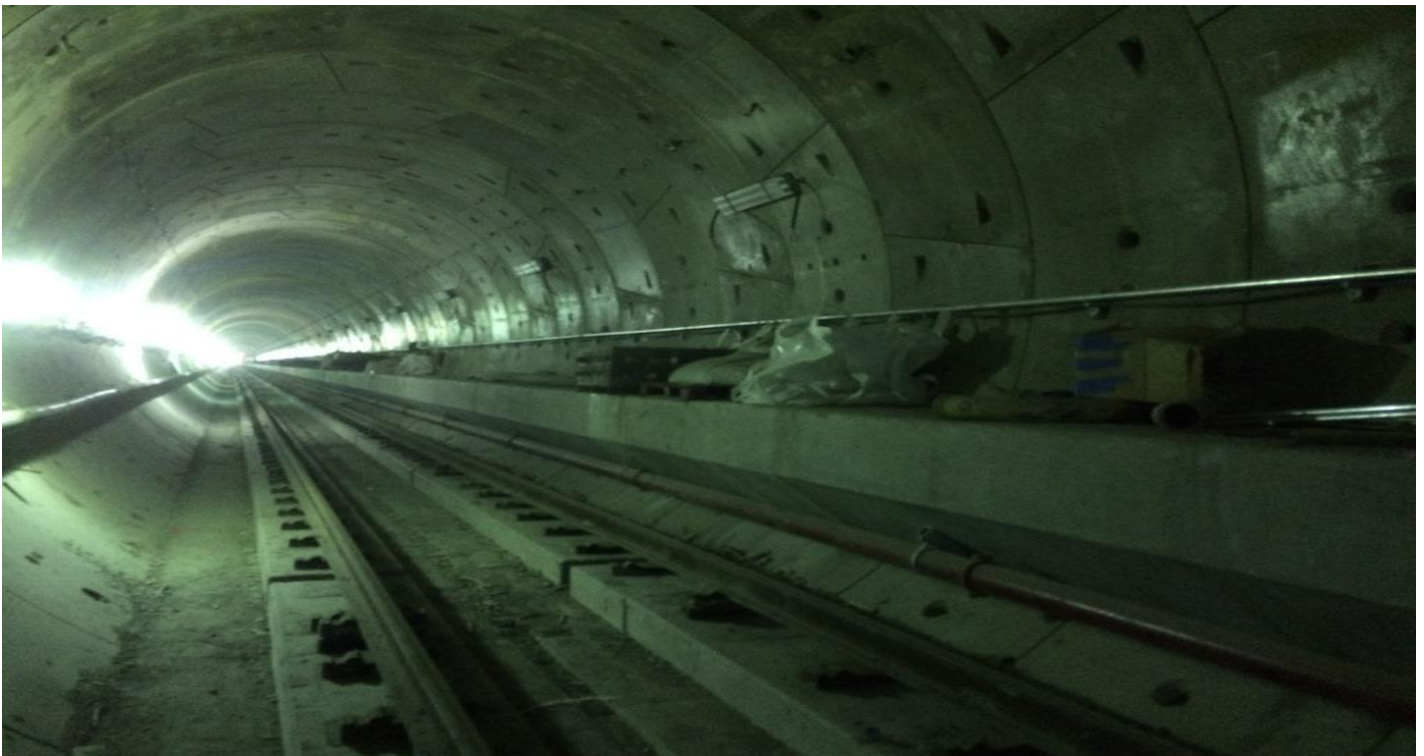
TUNNEL – SB tunnel between Expo and MLK station.
