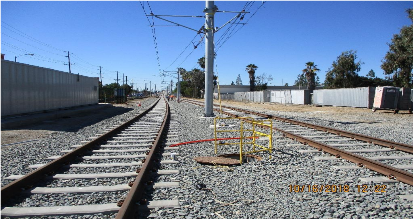
B1 GUIDEWAY - Pulling 144 fiber optic cable East of Cedar Ave.
