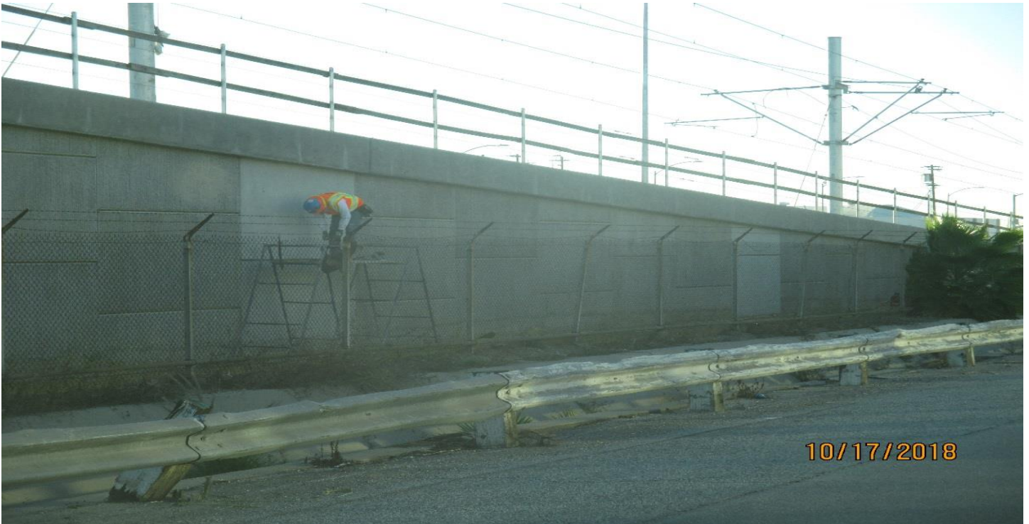
MSE 60L&R - Concrete finish work at RW #60.
