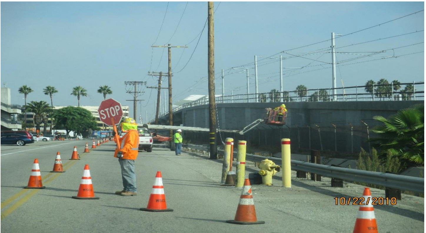
MSE 60L&R - Concrete finish work for the SB side of RW #60.
