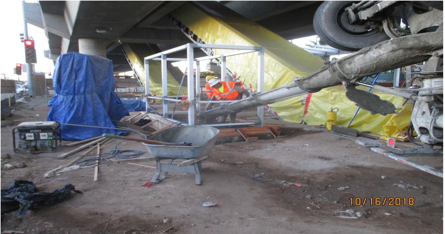
AVIATION/CENTURY STATION- Erection of the Aviation Station ticket booth.
