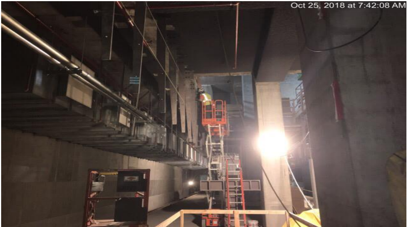
MARTIN LUTHER KING JR. STATION- Installation of downstands above the platform.
