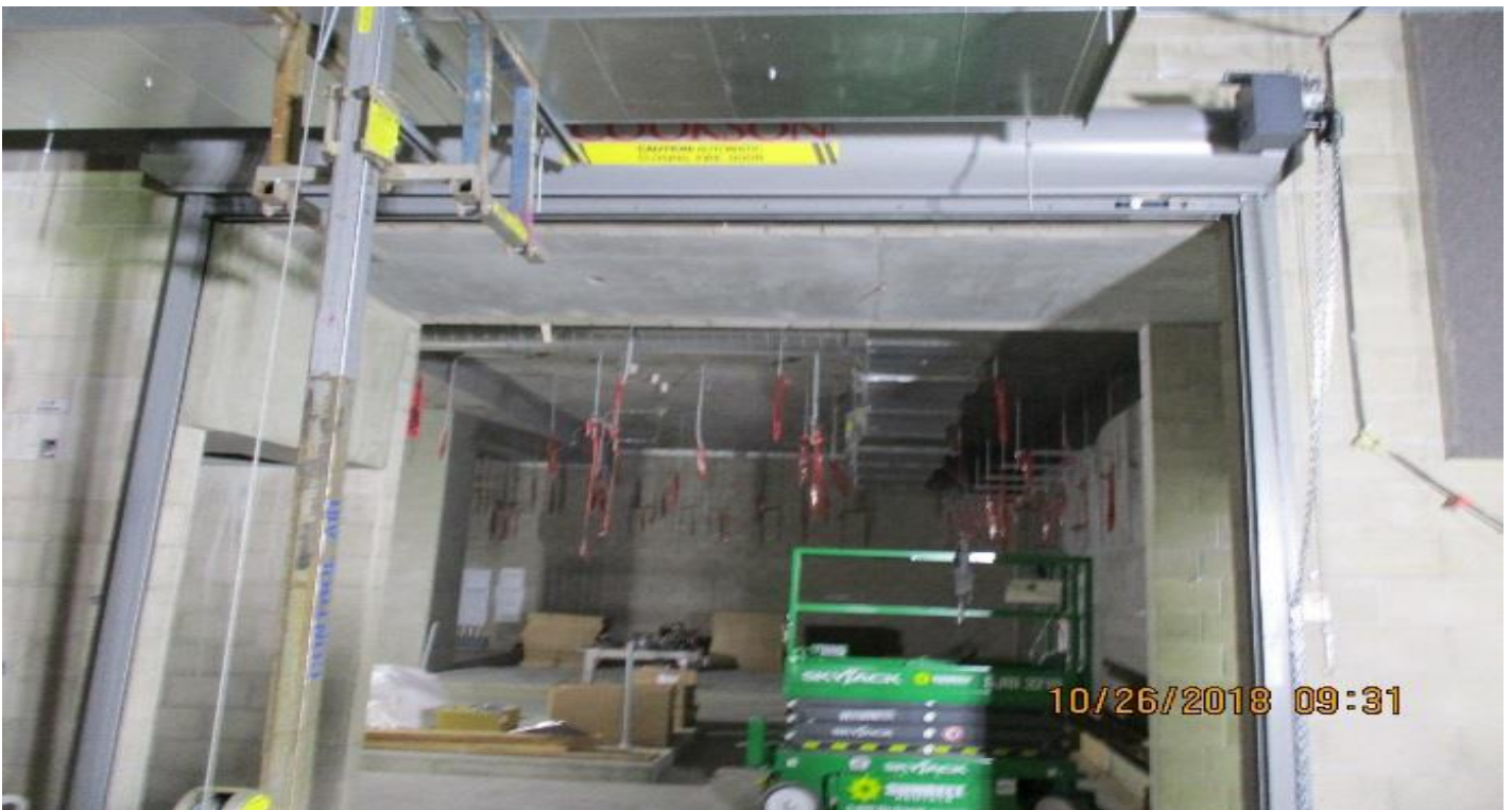
LEIMERT PARK STATION – Installation of overhead coiling doors at the concourse.
