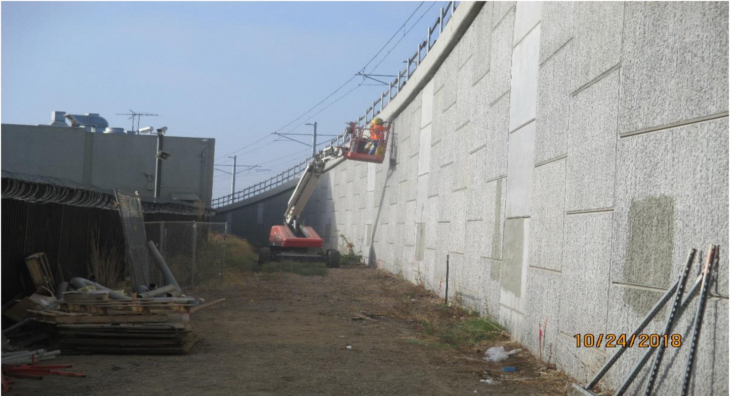
MSE 111L&R- Concrete finish work at RW #111.
