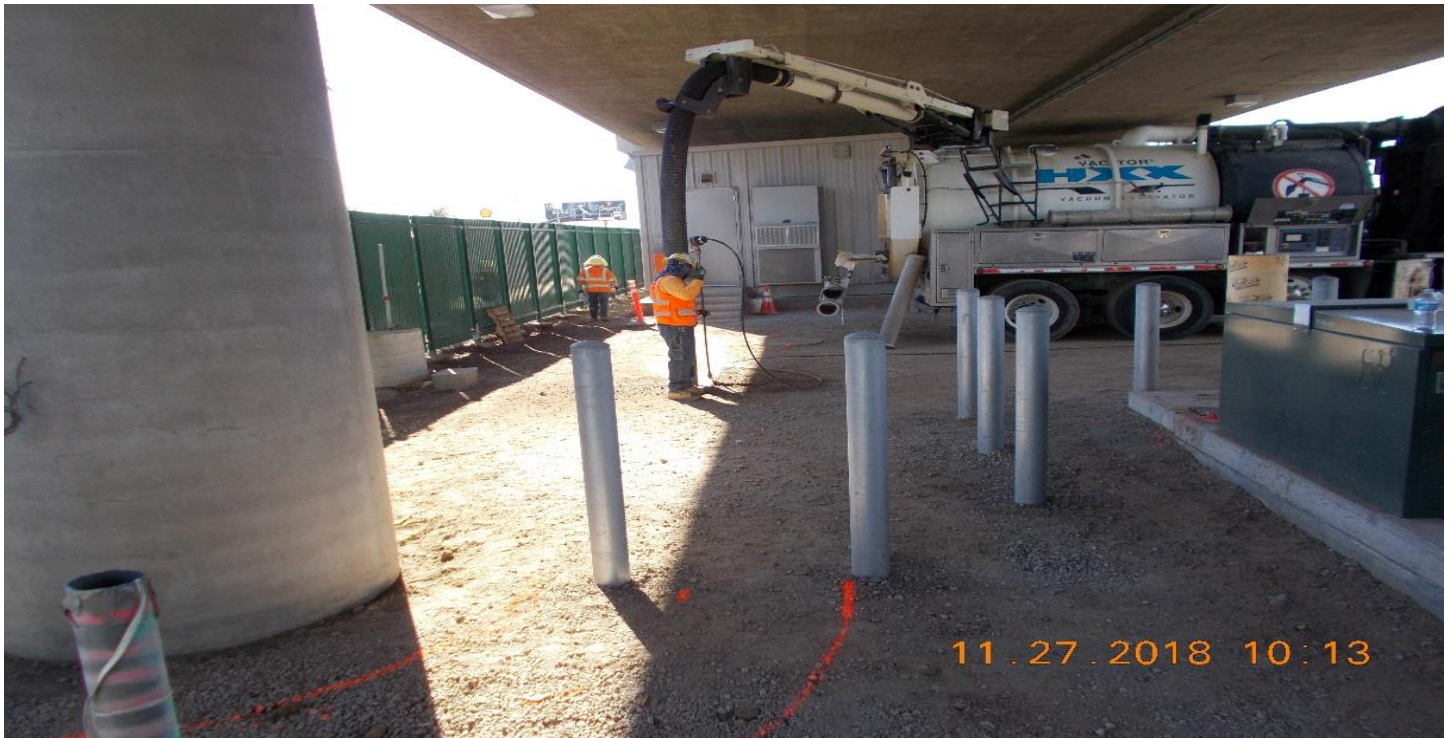
TPSS- TPSS #2. WSCC potholing for negative returns adjustment design change.
