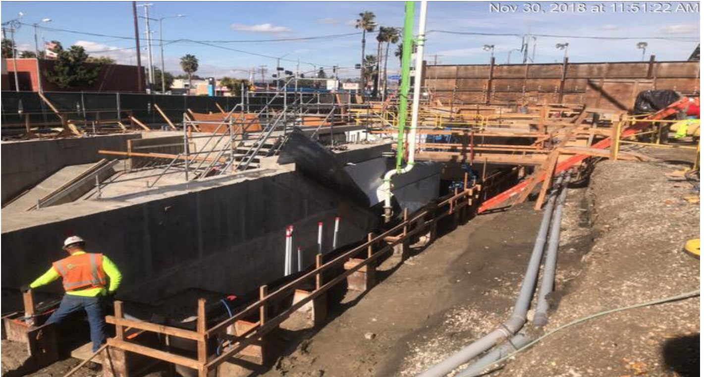
EXPOSITION/CRENSHAW STATION – Concrete placement for Emergency Exit Stairs #3
