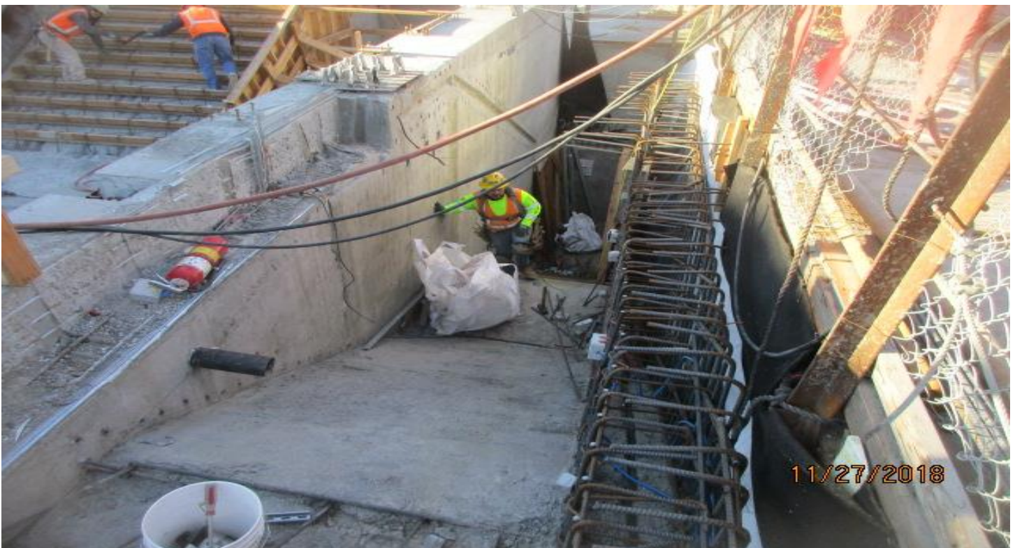
LEIMERT PARK STATION – Construction of wall at North Emergency Exit #2.
