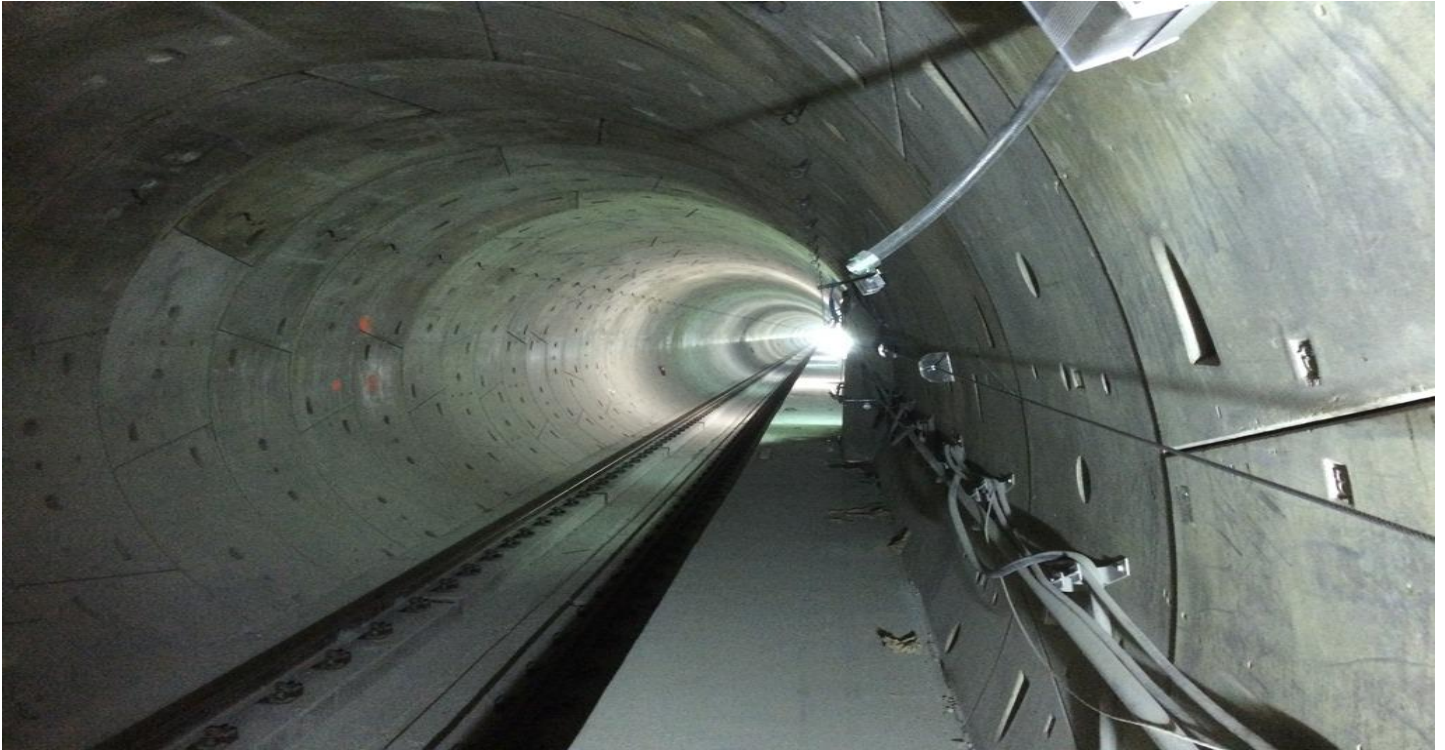
TUNNEL – Northbound tunnel between Expo and MLK Station.
