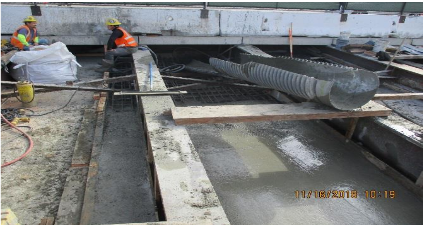
UG3 - Concrete placement for roof section P63.
