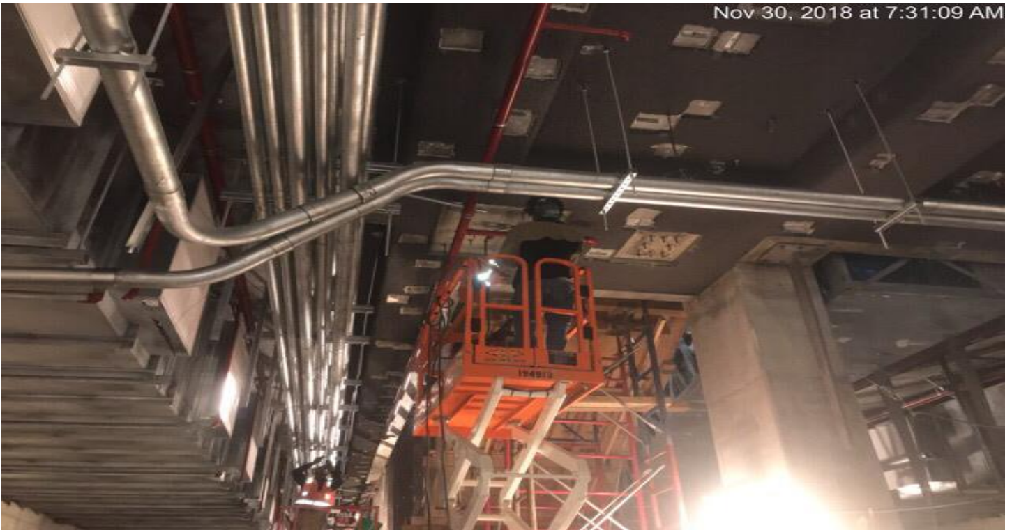
MARTIN LUTHER KING JR. STATION Installation of downstands above the platform.
