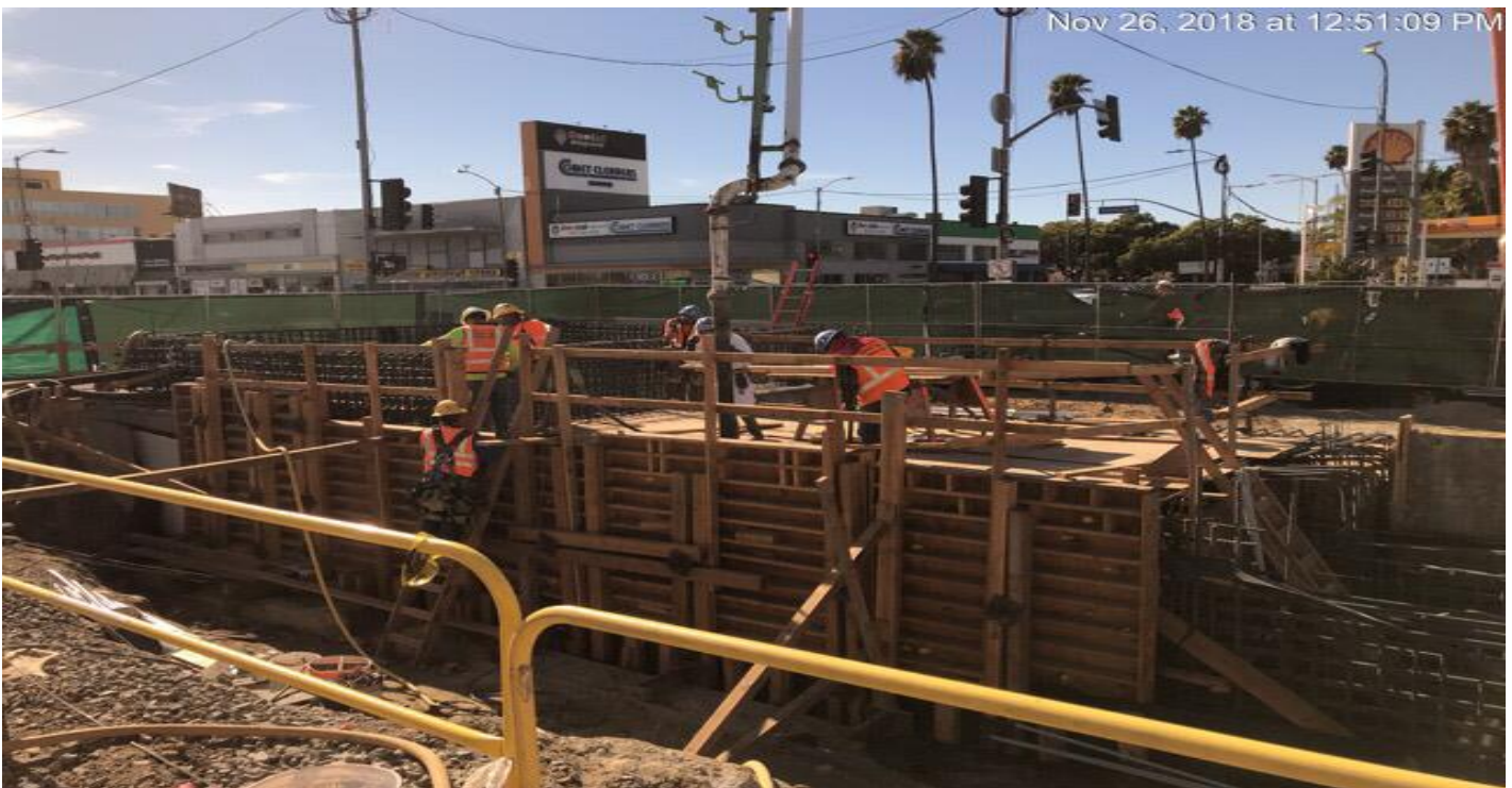
EXPOSITION/CRENSHAW STATION – Installation of formwork for plaza wall R9.
