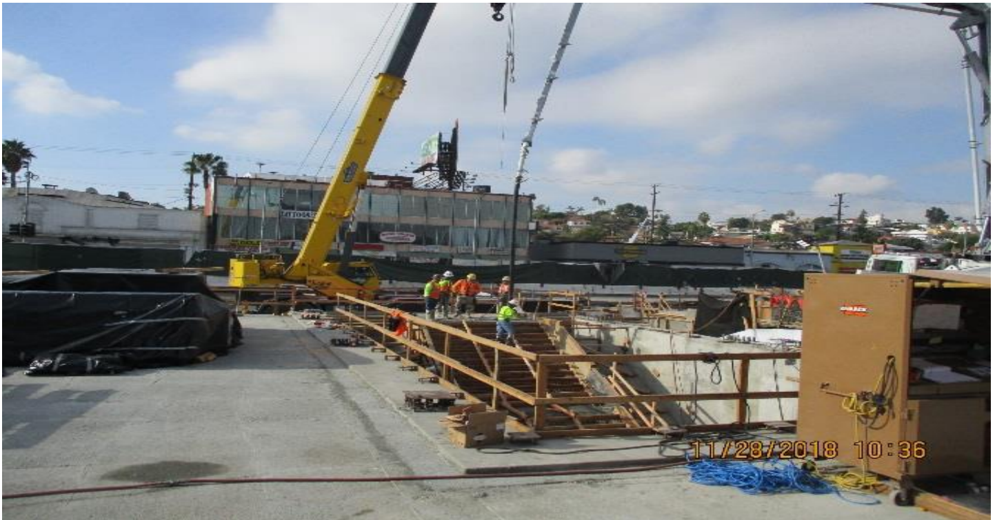
LEIMERT PARK STATION – Concrete placement for Stair #1 at the entrance structure.
