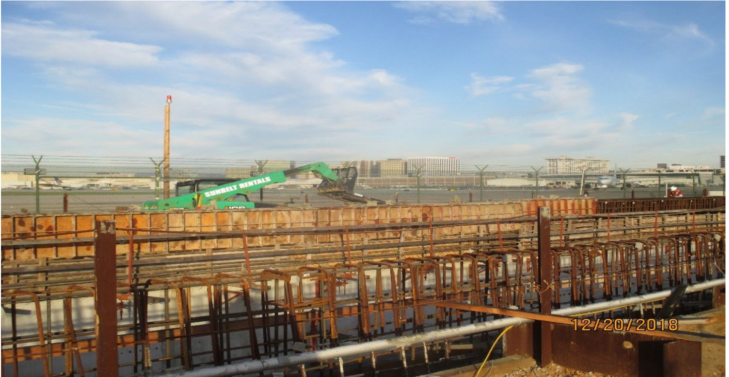
UG1- Stripping barrier wall forms at UG-1
