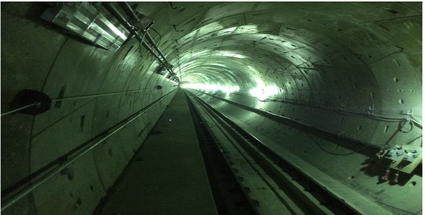
TUNNEL – Southbound tunnel between EXPO and MLK Station.
