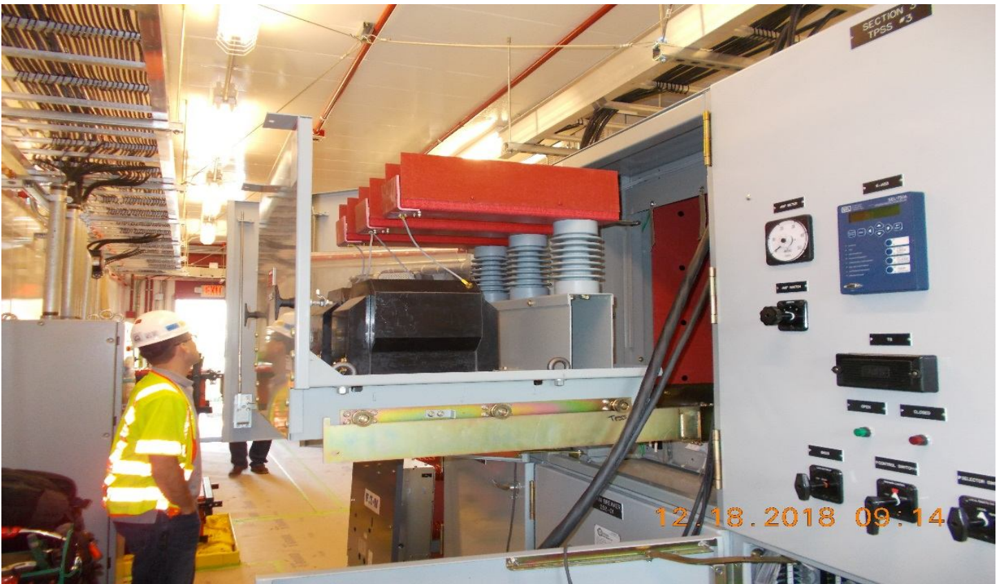
TPSS- TPSS #3. Pre-LFAT testing.
