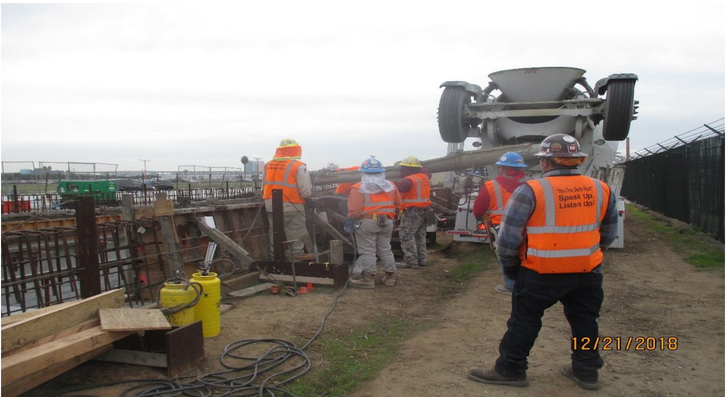
UG1- Placing concrete for the barrier wall at UG-1.
