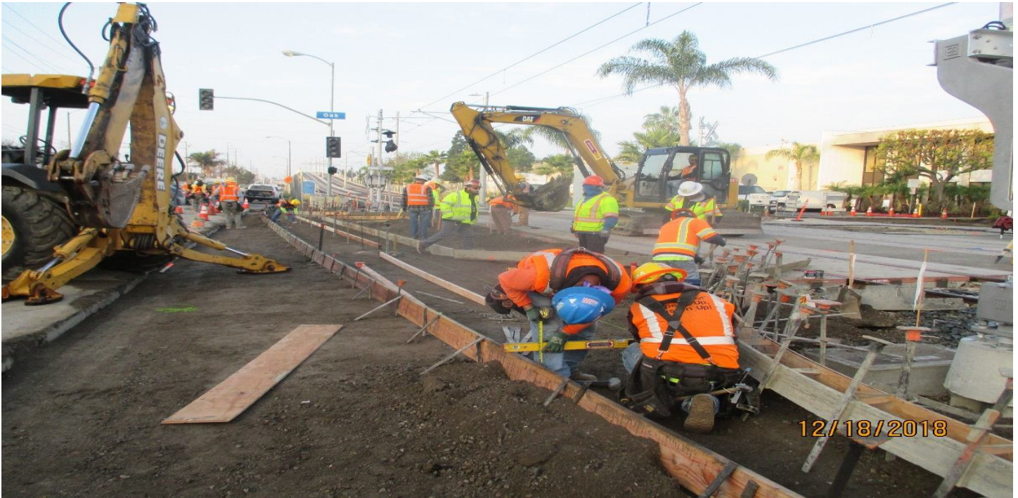
B1 GUIDEWAY - Setting forms for the Oak Street cross gutter.
