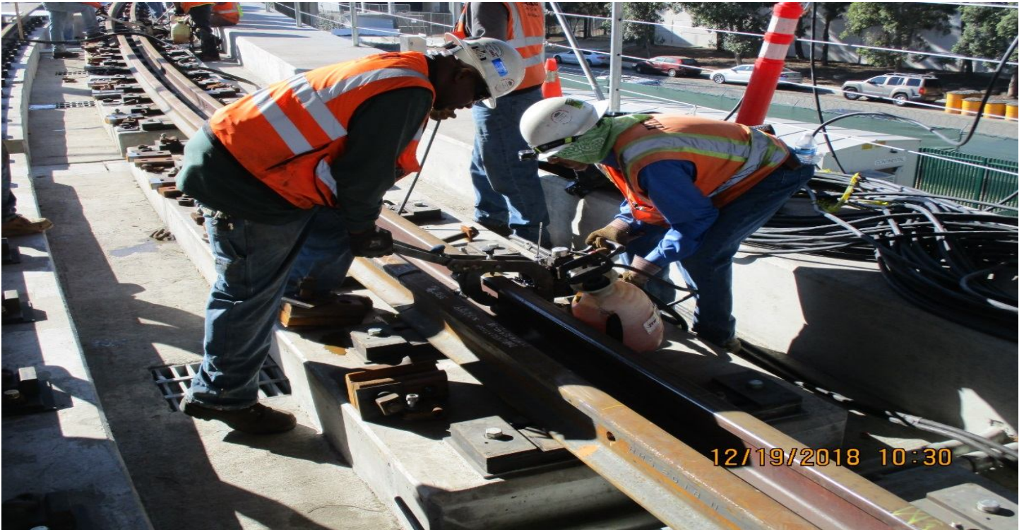
GREENLINE UNDERPASS- Restraining rail placement and drill at SBW track.
