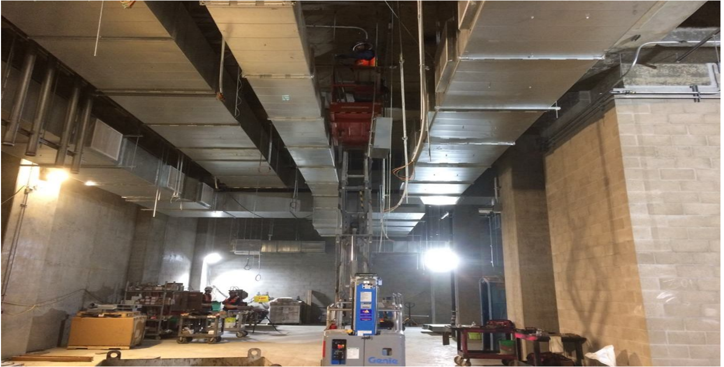
EXPOSITION/CRENSHAW STATION – Installation of electrical conduit at TPSS 10.
