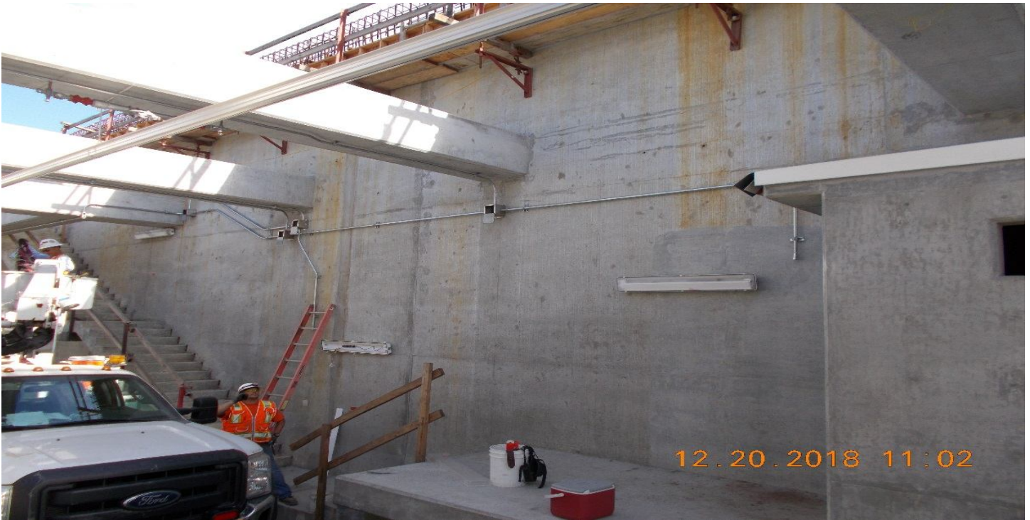
UG1- Neal Electric installing tunnel lighting conduit near radio room.
