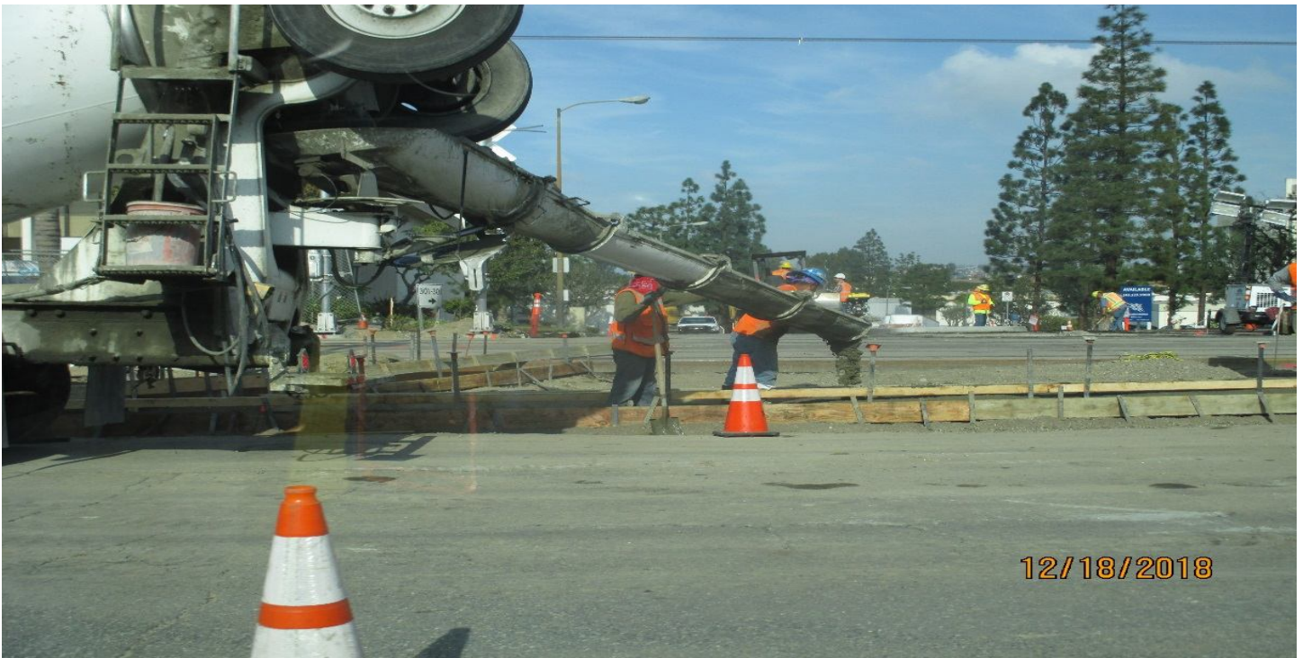
B1 GUIDEWAY - Placing concrete for the Oak Street cross gutter.
