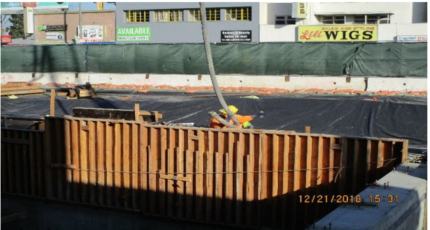
MARTIN LUTHER KING JR. STATION- Concrete placement for wall EW-25.
