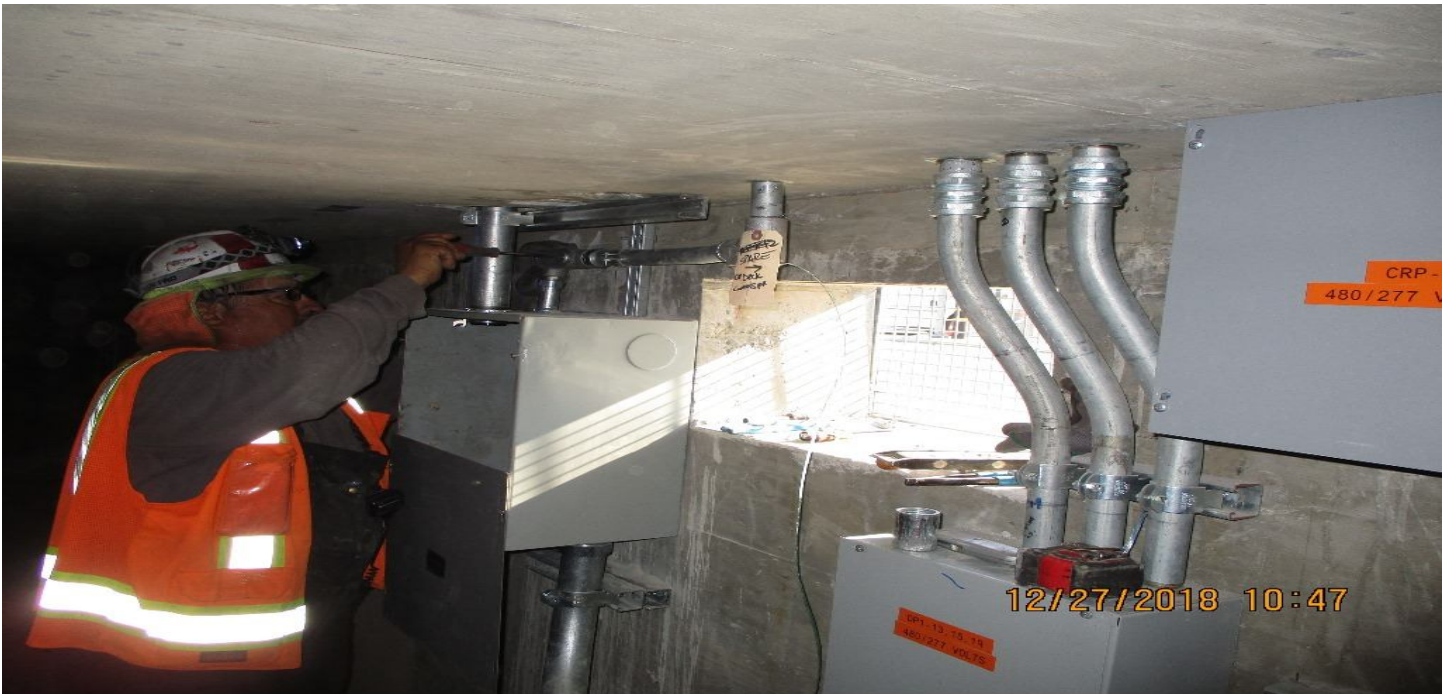
WESTCHESTER STATION- Neal E running CCTV conduit under NB Platform at.
