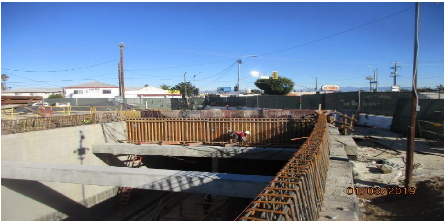
UG3 - Construction of the bulkhead wall at the south portal.
