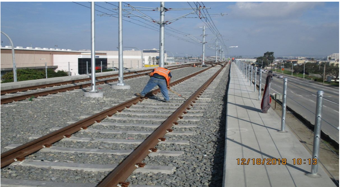
MSE17- Top ballast rock cribbing.
