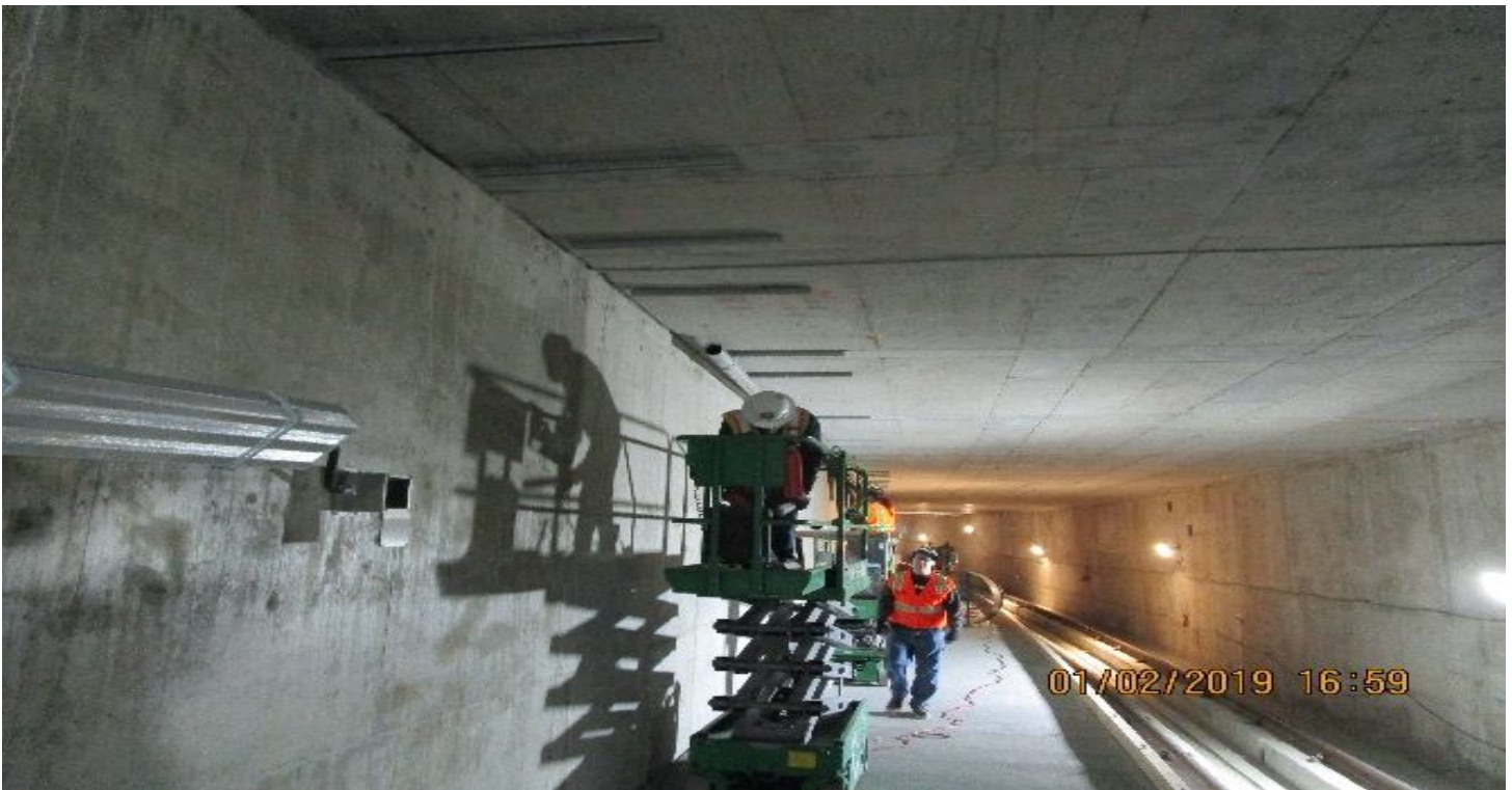
UG4 – Installation of electrical conduit at the northbound tunnel.
