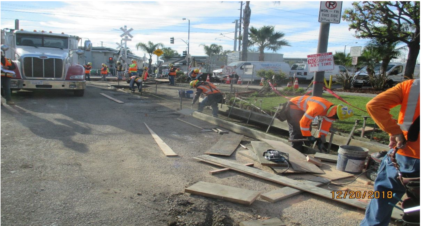
B1 GUIDEWAY - Forming the drive approach on Oak.
