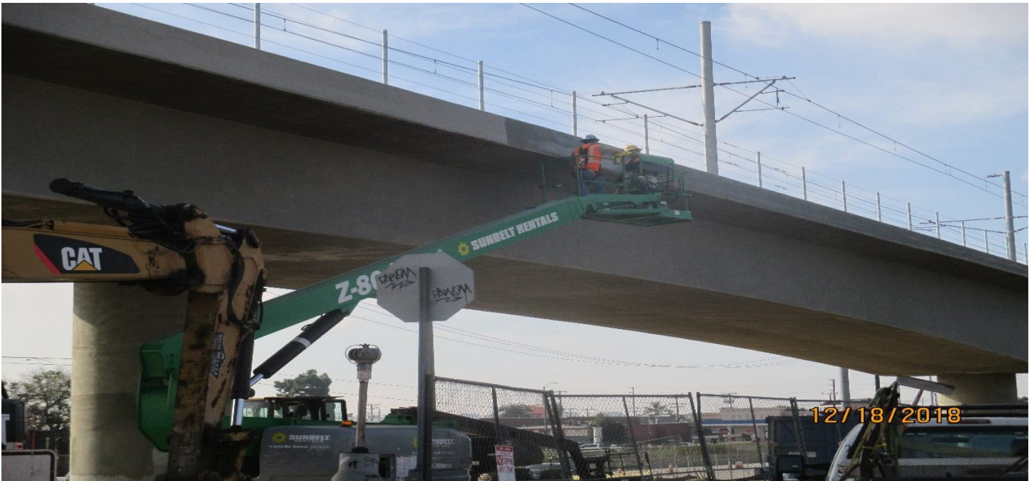
AG) I 405 BRIDGE- Working on the concrete finish for the 405 Bridge.
