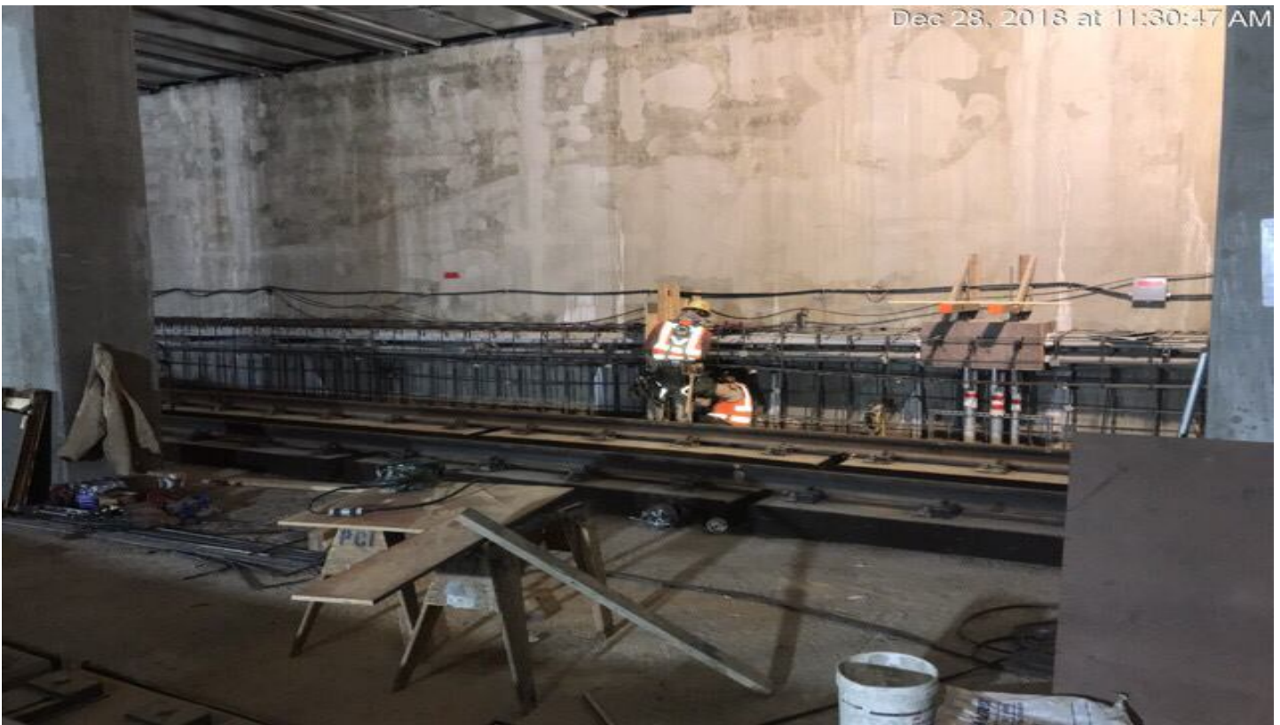
EXPOSITION/CRENSHAW STATION – Installation of formwork for safety walkway.
