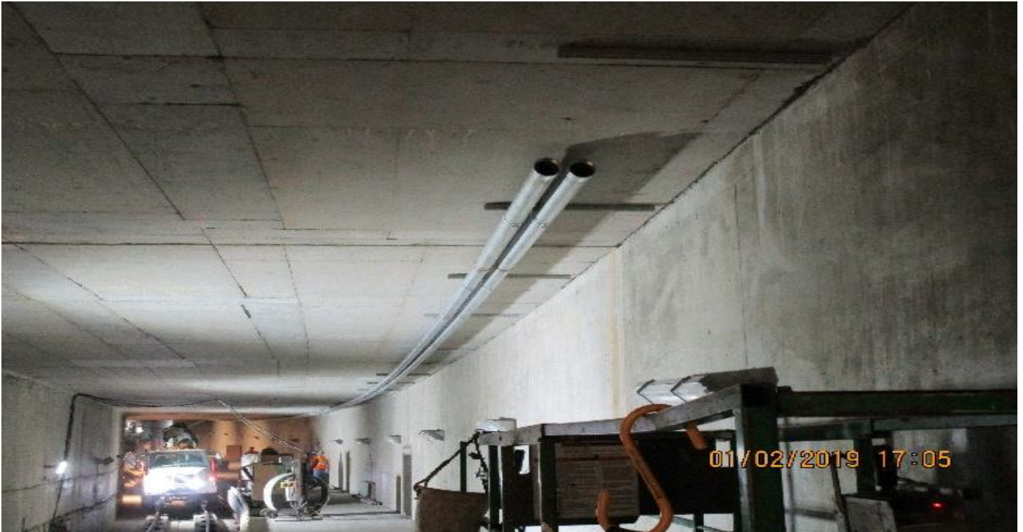
UG4 – Installation of electrical conduit at the southbound tunnel.
