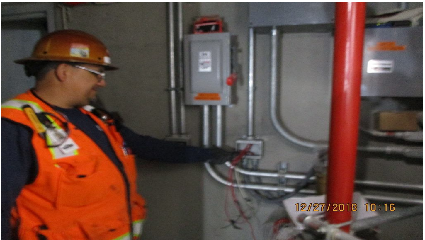
WESTCHESTER STATION - RBT terminating Fire alarm Devices at Hindry Station.
