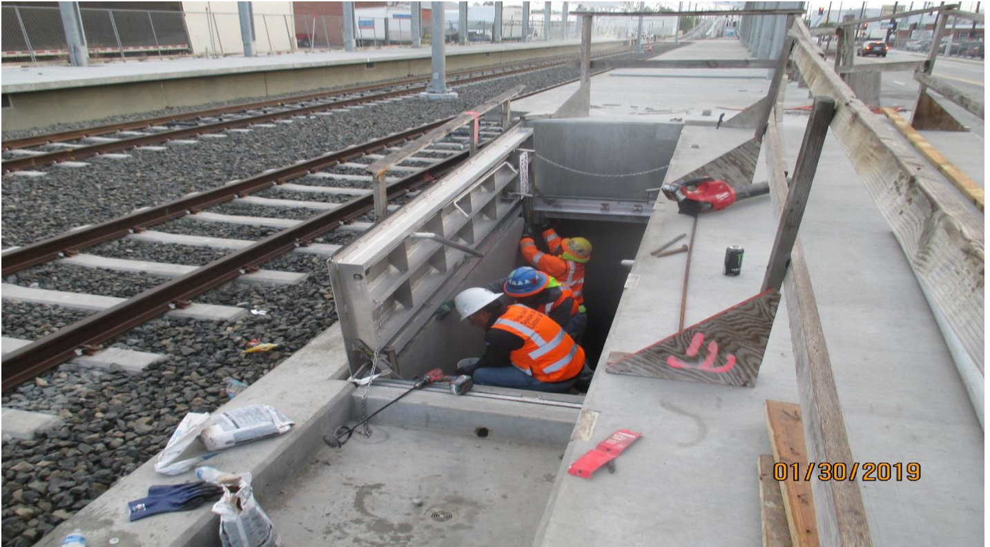
WESTCHESTER STATION- Dry pack around the hatch door for the Westchester Station.
