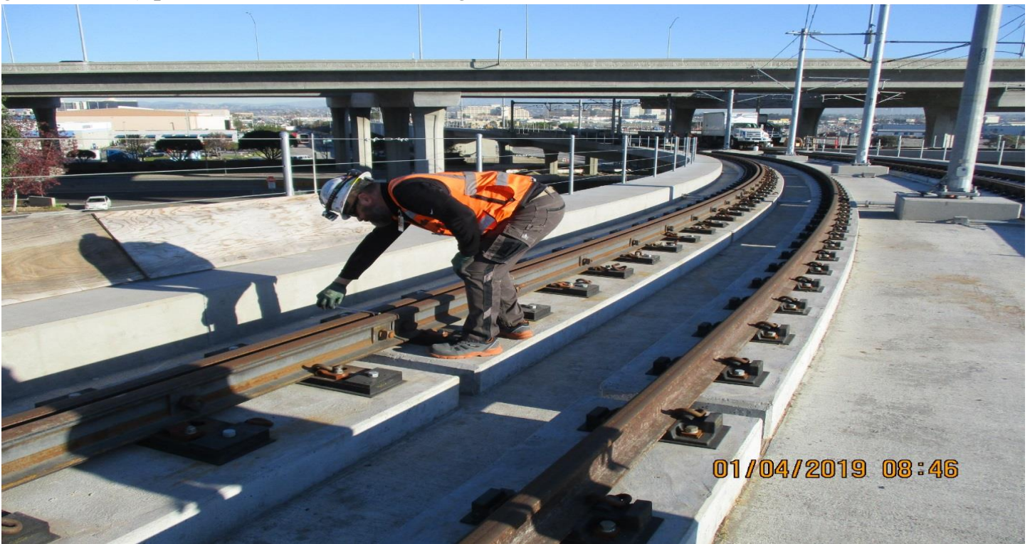
GREENLINE UNDERPASS- A Guideway at Greenline Up restaing rail bolt torquing and galv walkway placement.fasteners at Hinge 14.
