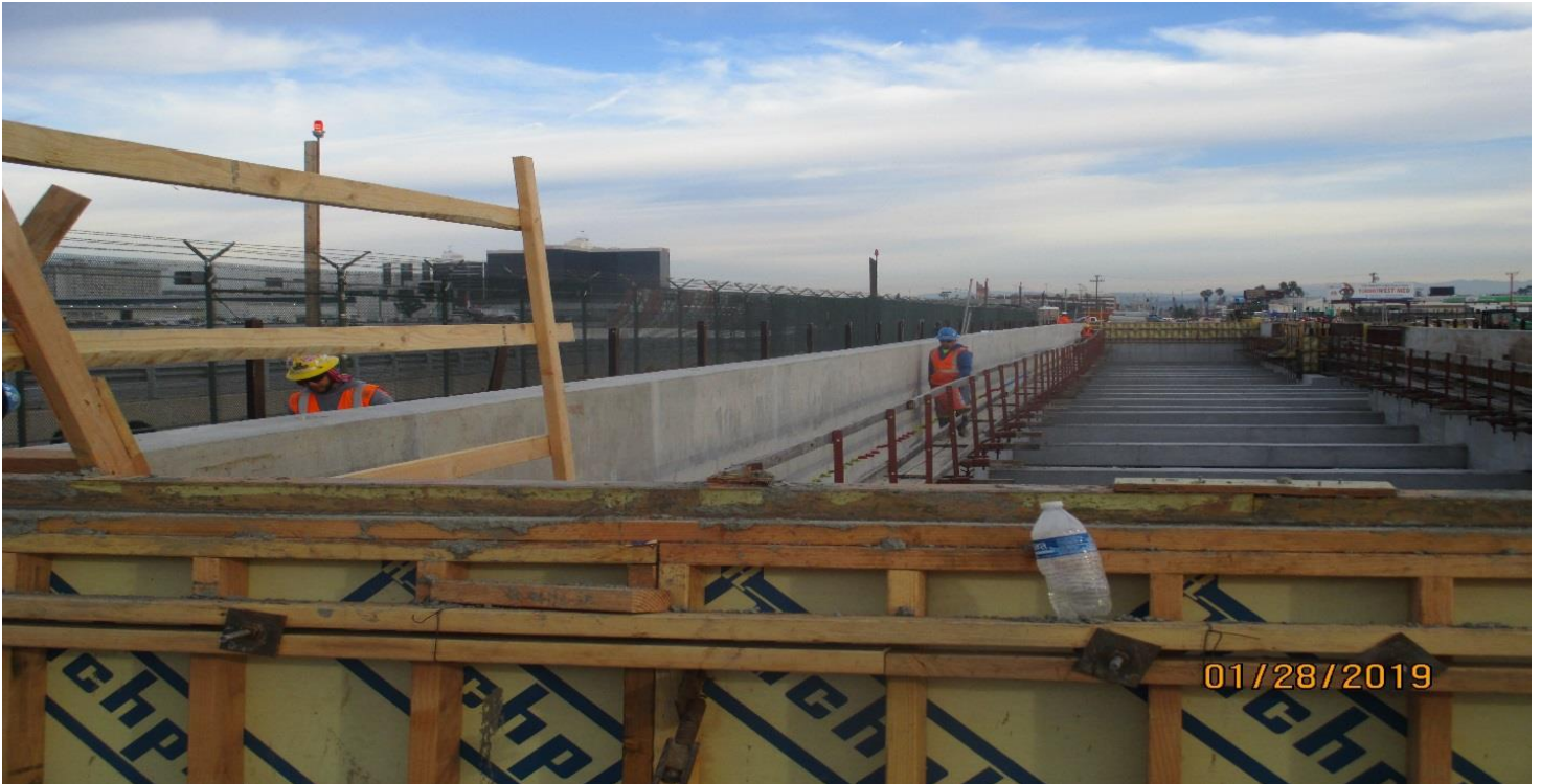
UG1- Concrete finish work for the SB barrier wall at UG1.
