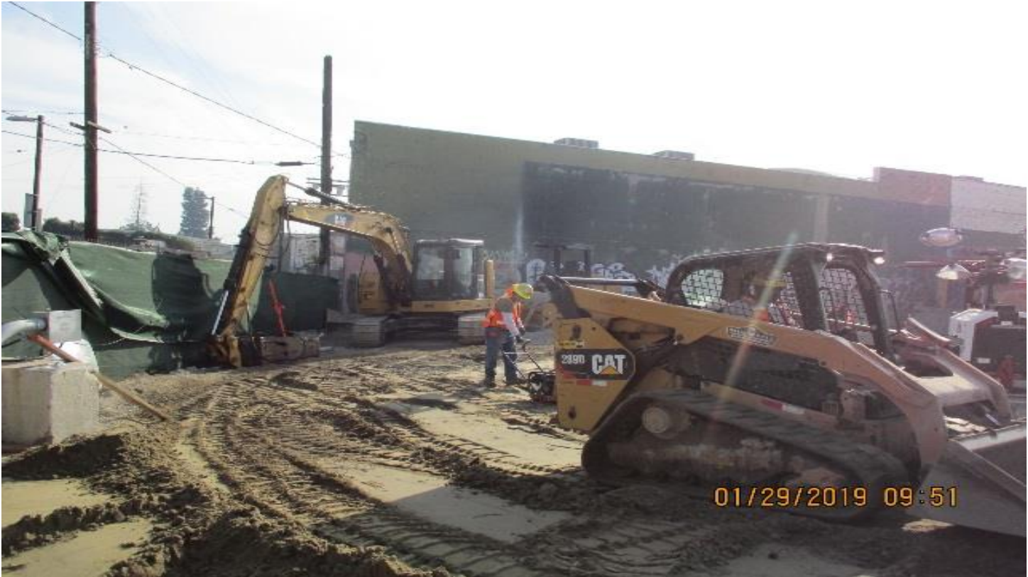
LEIMERT PARK STATION – Backfill and compaction at the plaza level.
