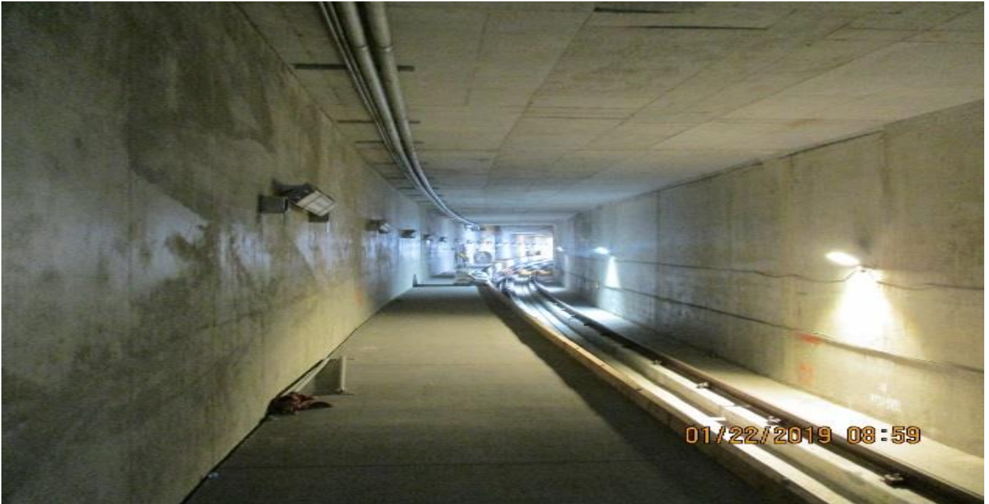
UG4 – Northbound tunnel. (No progress since last progress report)
