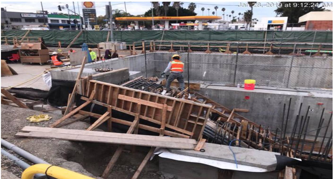
EXPOSITION/CRENSHAW STATION – Installation of formwork for Emergency Exit stairs #3.
