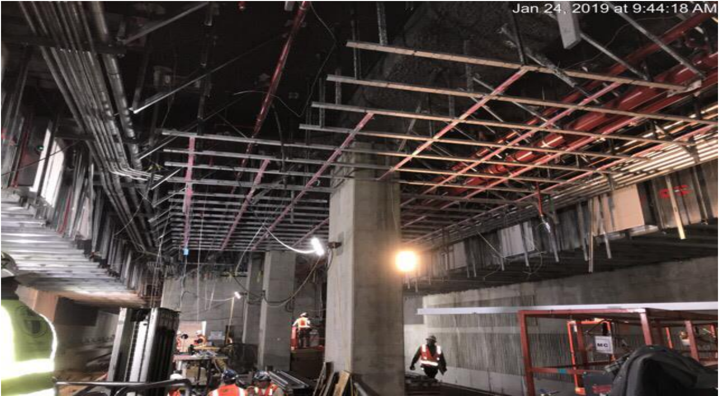
EXPOSITION/CRENSHAW STATION – Installation of metal ceiling at platform level.
