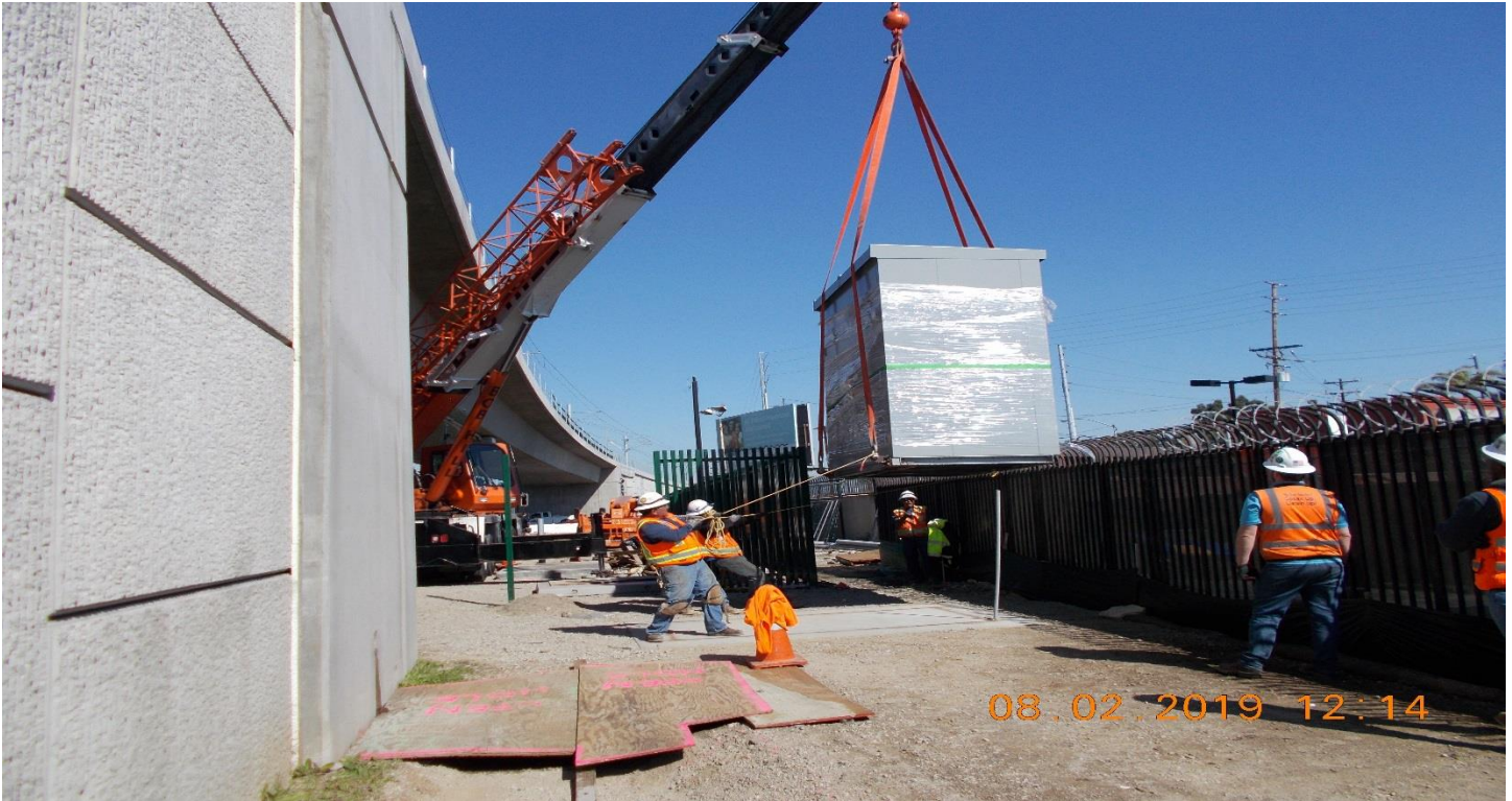
TPSS- TPSS #3. Crane operator and Neal Electric getting the load managed.
