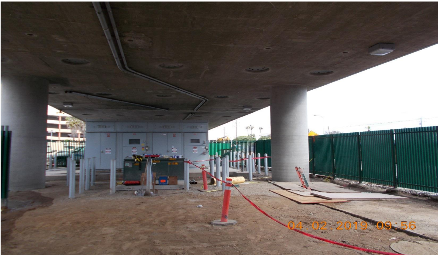
TPSS- TPSS #2. Conduit racks being prepared for negative returns.
