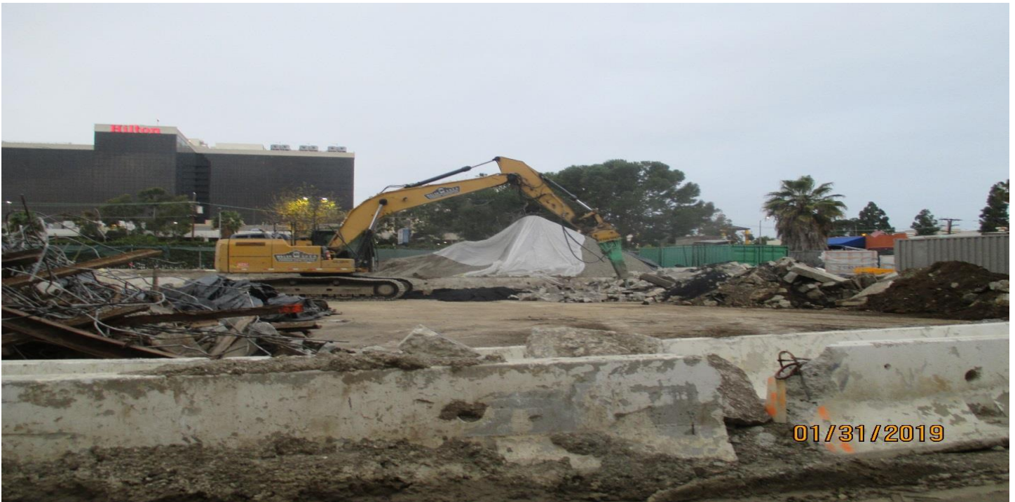
AVIATION/CENTURY- Rubble Demo at the Aviation/Century Station Yard.
