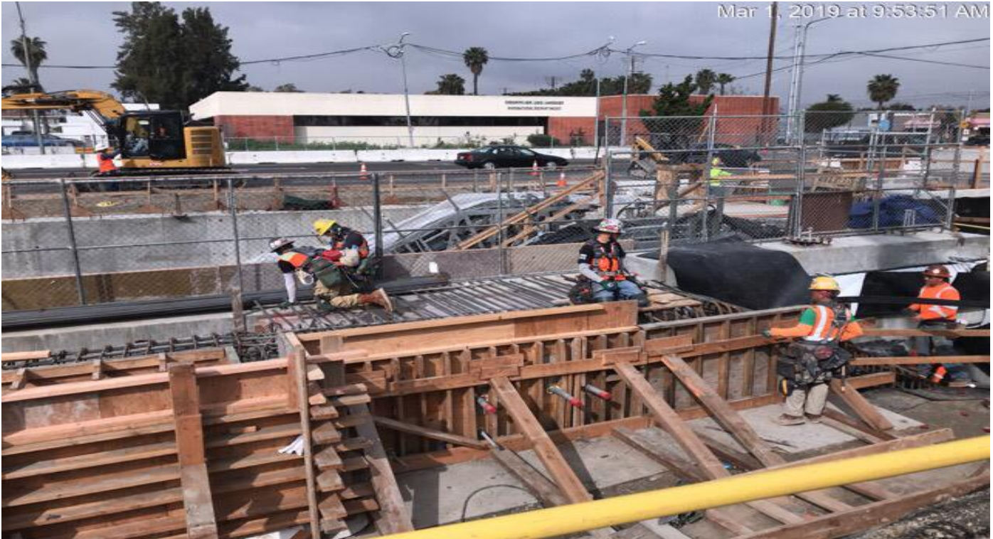
EXPOSITION/CRENSHAW STATION – Installation of formwork for Emergency Exit Staircase #3.
