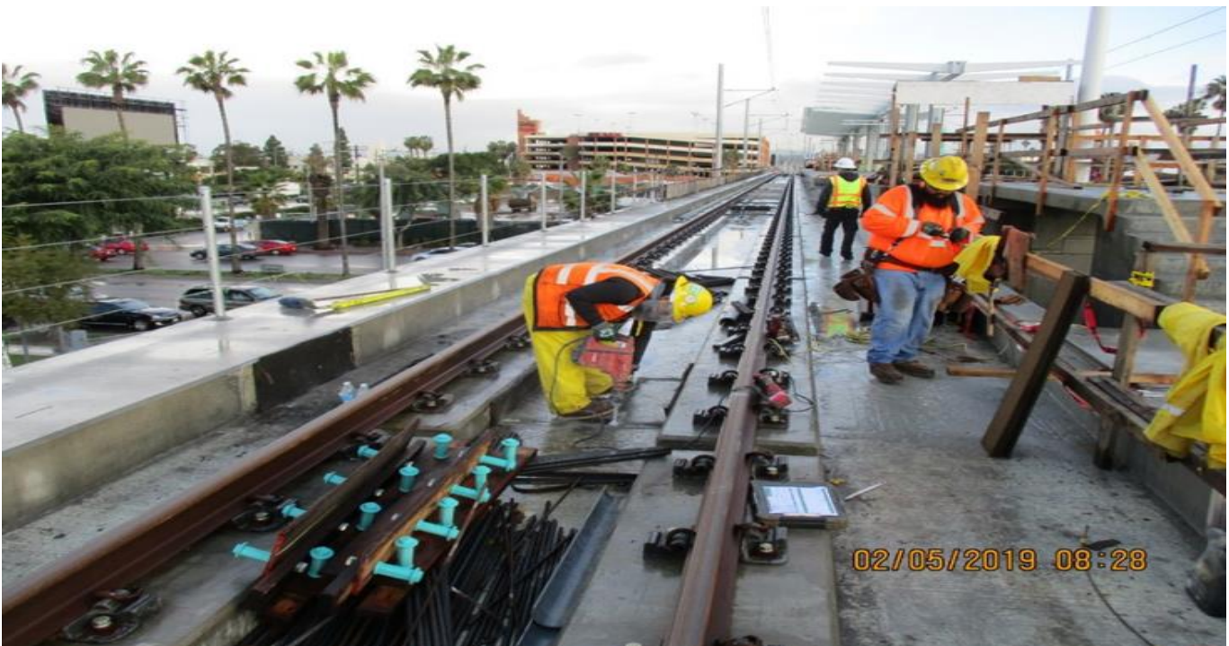
AVIATION/CENTURY- A Guideway UP NB-SB crosswalk forming.
