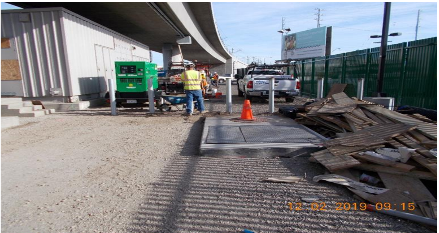
TPSS- TPSS #3. Ace Fence Co finishing bollard install.
