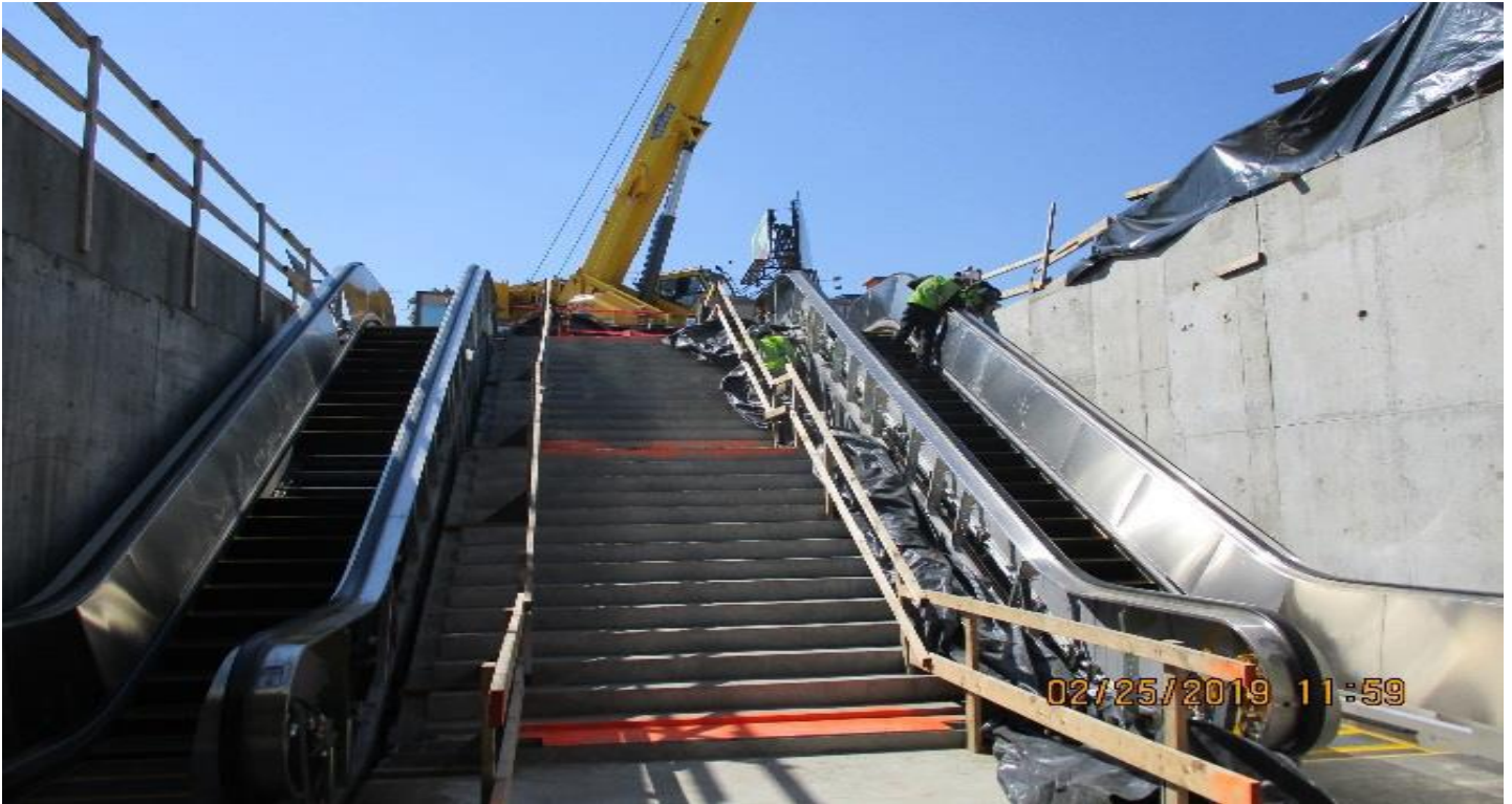
LEIMERT PARK STATION – Installation of escalator 1&2 at the entrance.
