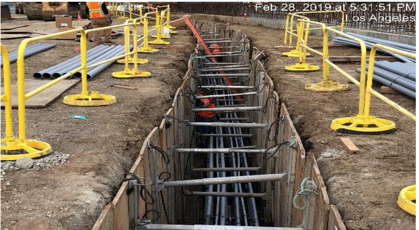
UG3- Installation of conduit in trench at Victoria yard.
