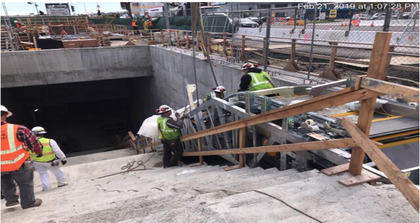
EXPOSITION/CRENSHAW STATION – Installation of escalators in the main plaza entrance.
