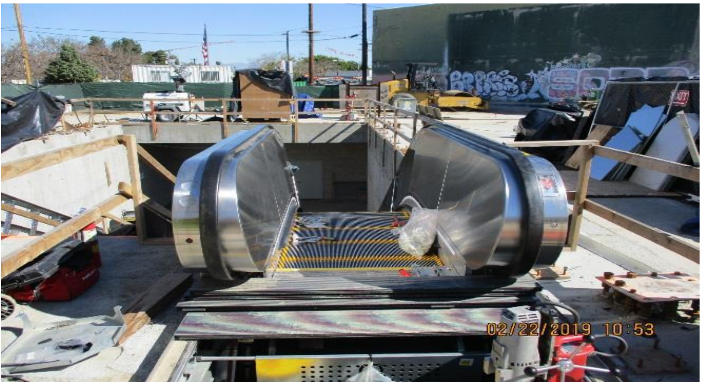
LEIMERT PARK STATION – Installation of escalator 1&2 at the entrance.
