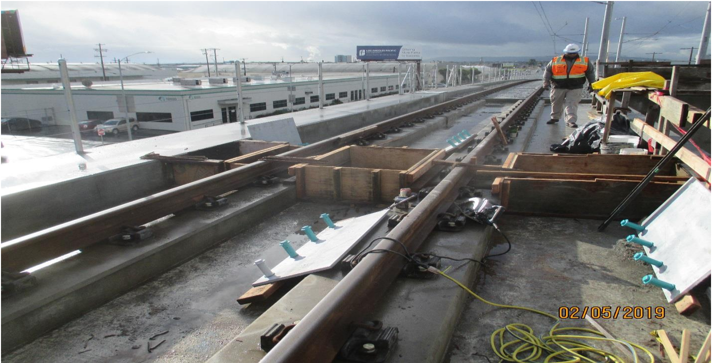
AVIATION/CENTURY- Forming the concrete walkway at STA.66+20 at the Aviation Station.
