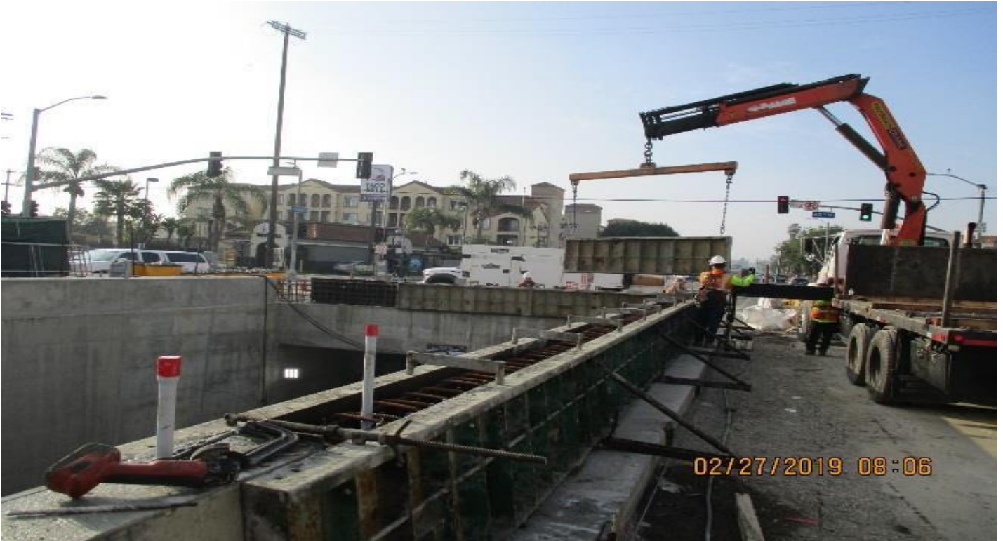
UG3- Installation of the barrier wall at the North Portal.
