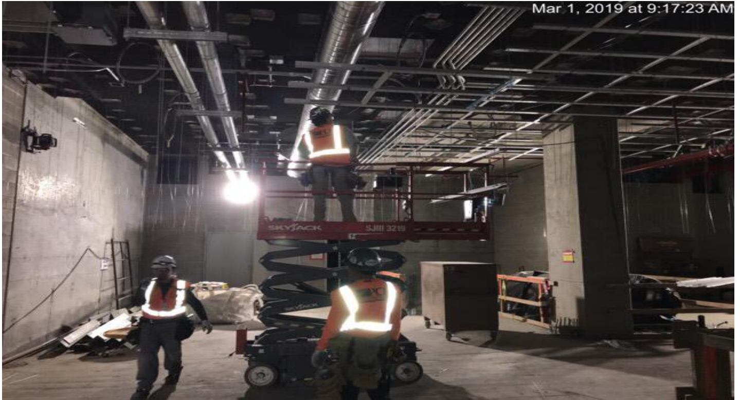
EXPOSITION/CRENSHAW STATION – Installation of metal ceiling at the Paid Area.
