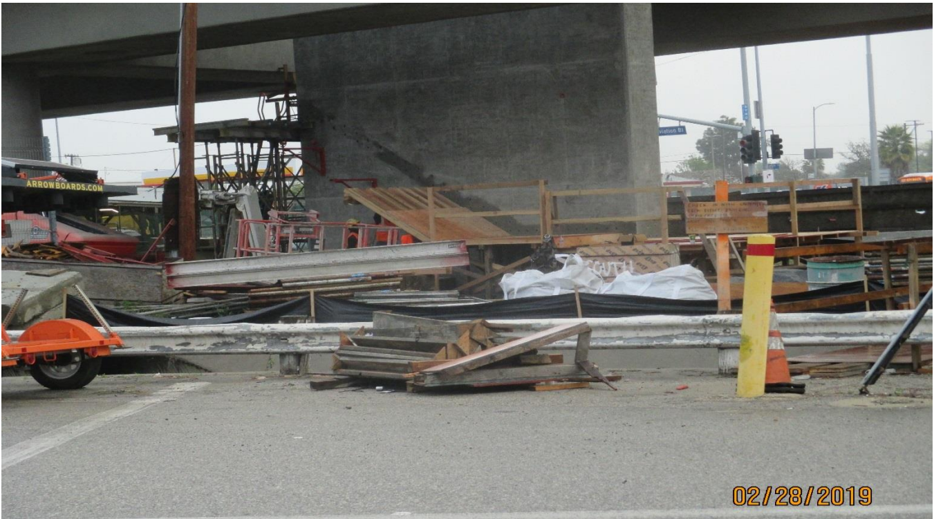
AVIATION/CENTURY- Forming the south stairway at the Aviation Station.
