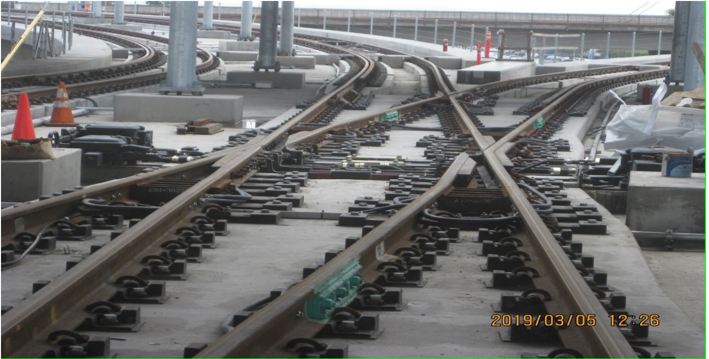
GREENLINE UNDERPASS- Crossing 3 switch machine installation.
