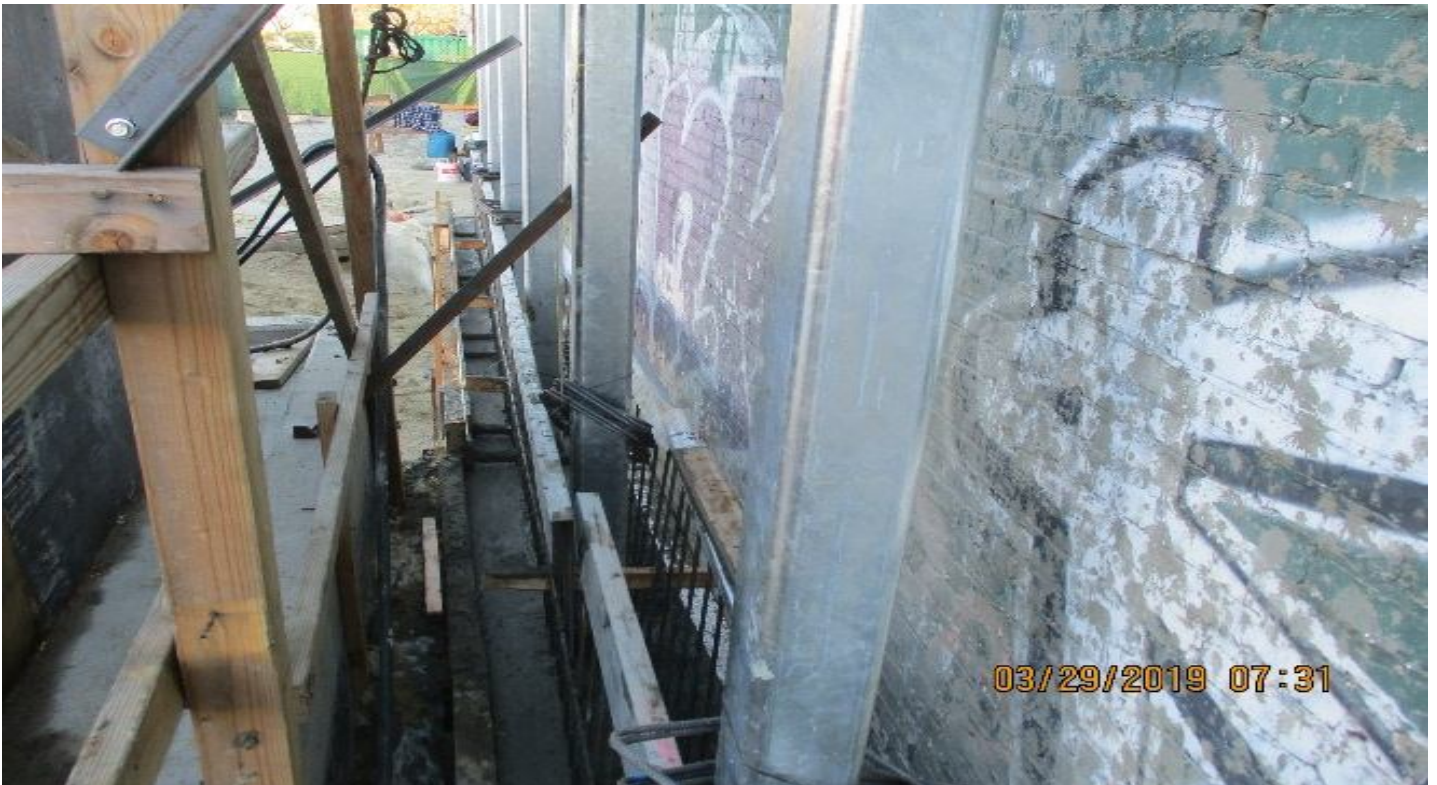
LEIMERT PARK STATION – Concrete placement for green wall at the plaza.
