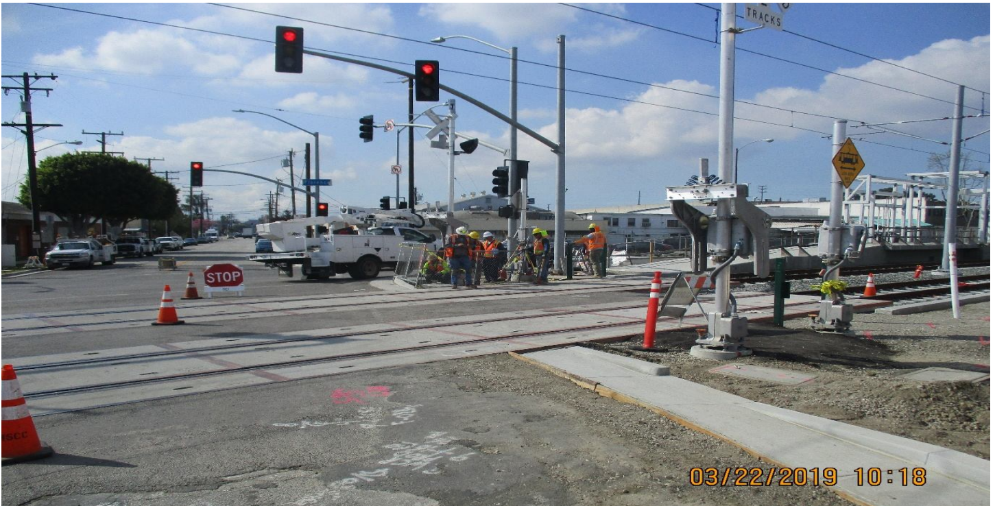
HINDRY & FLORENCE - Pulling wire and resetting traffic signal at Intersection.
