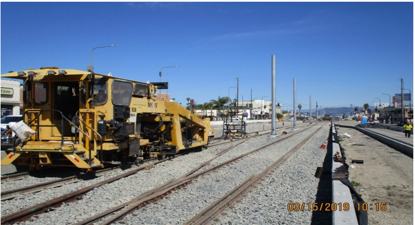
B2 GUIDEWAY 54 th to 57 th Streets – Rail surface, line, ballast tamping and dressing.
