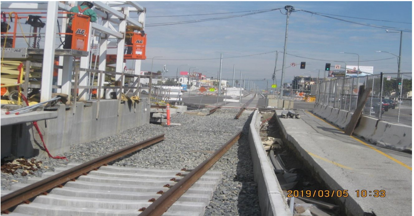
HYDE PARK STATION TRACK #4 NB – Rail & Tie removed for MH #97 rework
