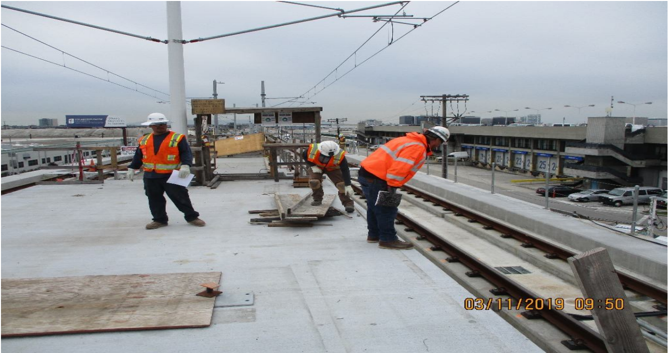
AVIATION/CENTURY- Surveying lighting conduits on the Platform.
