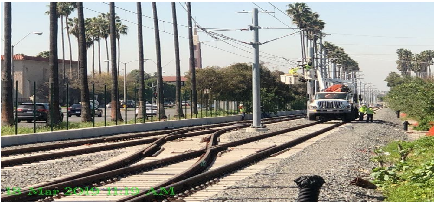
B1 GUIDEWAY - #3 SB Attaching messenger and contact wire WR#S1 to the yoke plate.
