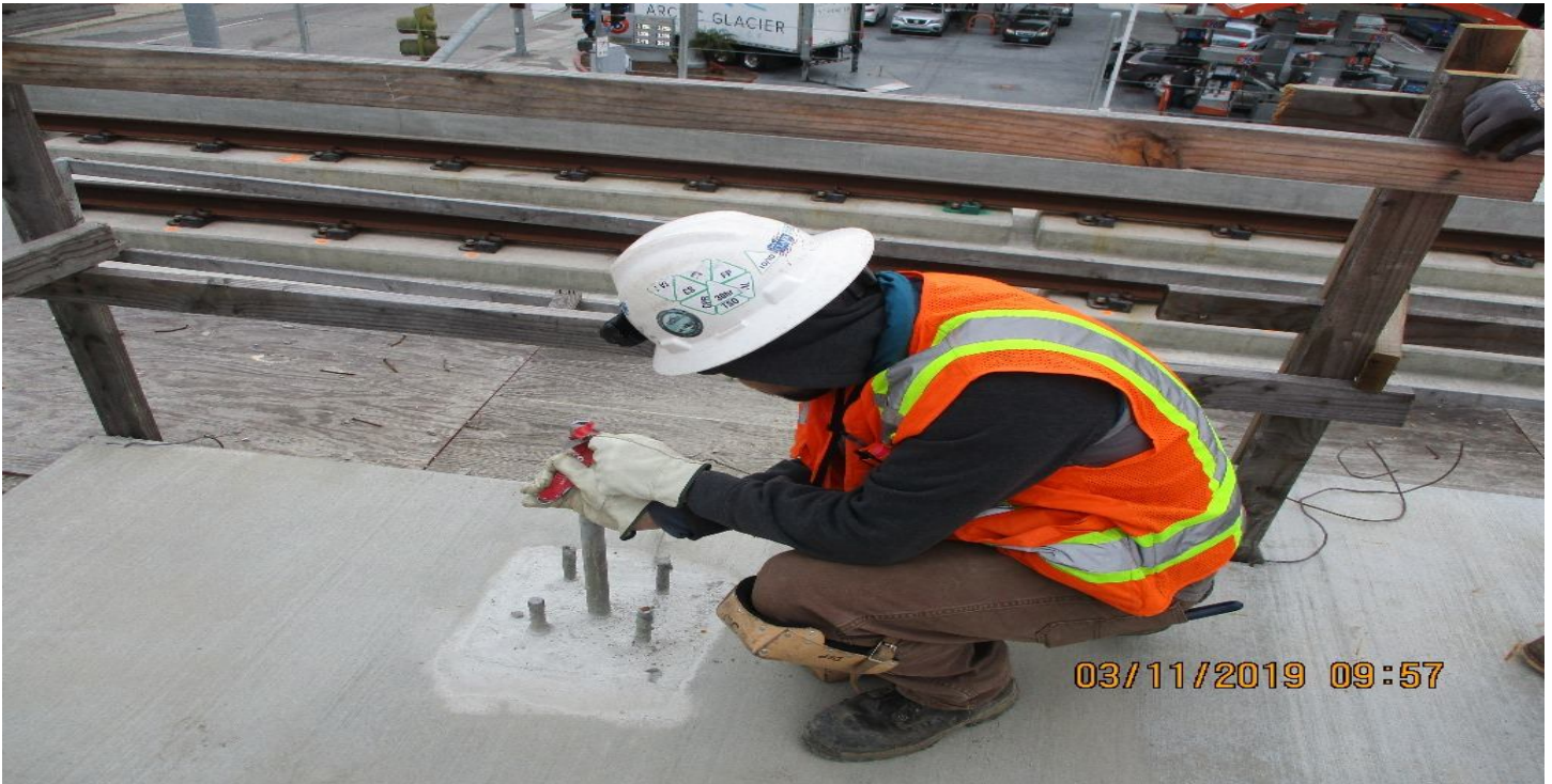
WESTCHESTER STATION- Surveying lighting conduits on the Platform.
