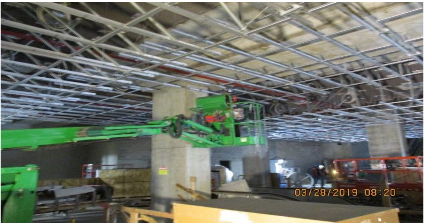
LEIMERT PARK STATION – Installation of the supports for the metal ceiling at the Concourse level.
