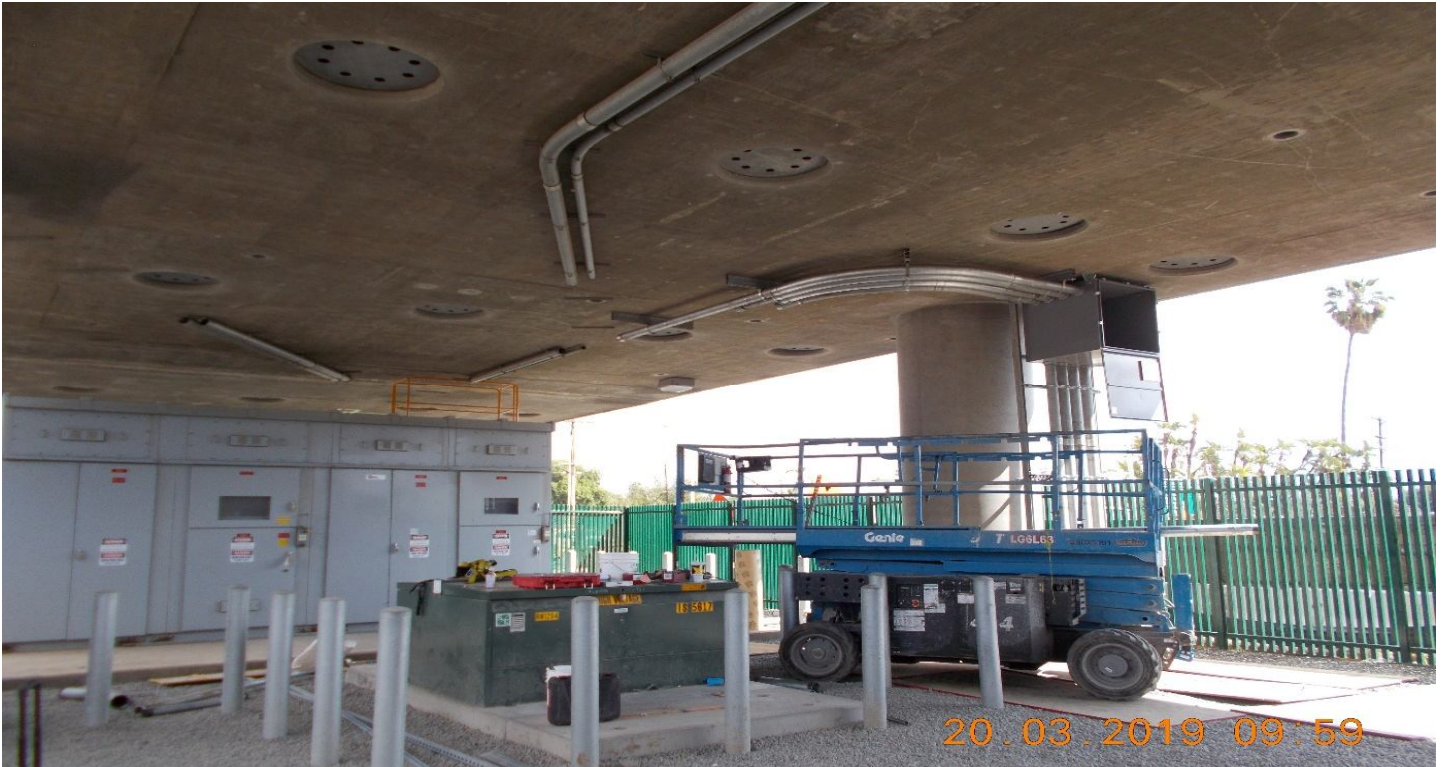
TPSS- Continuing to install negative return conduits.
