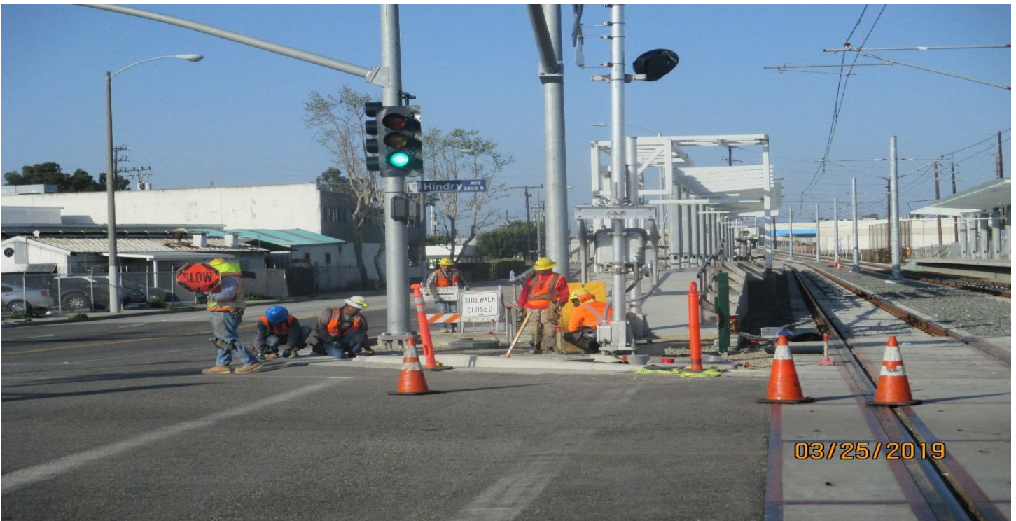
HINDRY CROSSING - Setting forms for the sidewalk for the northwest quadrant.
