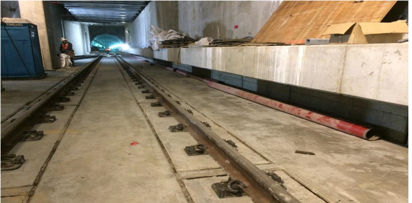
TUNNEL – UG4 Northbound Tunnel between the MLK and Expo Stations.
