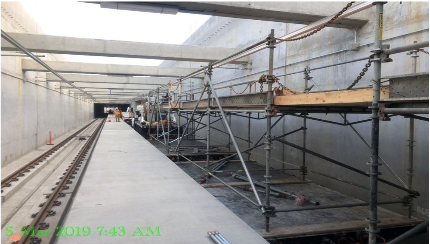
UG1- Installing 350 KCMIL contact wire run WR#08.
