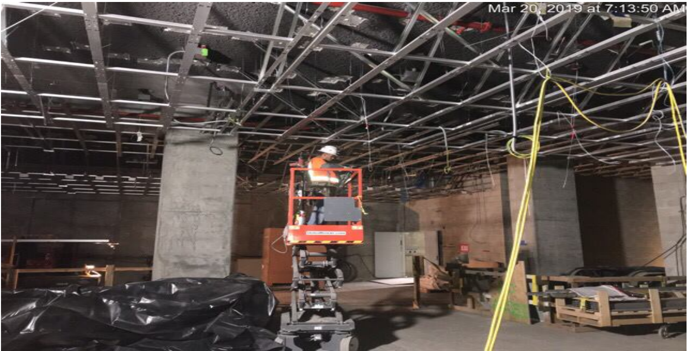
EXPOSITION/CRENSHAW STATION – Installation of metal ceiling at Concourse level.
