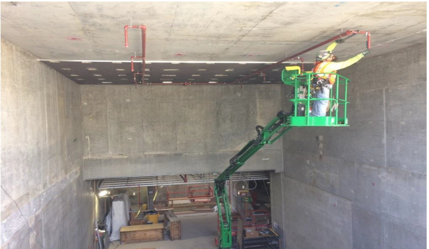
EXPOSITION/CRENSHAW STATION – Installation of fire sprinklers at the Concourse level.
