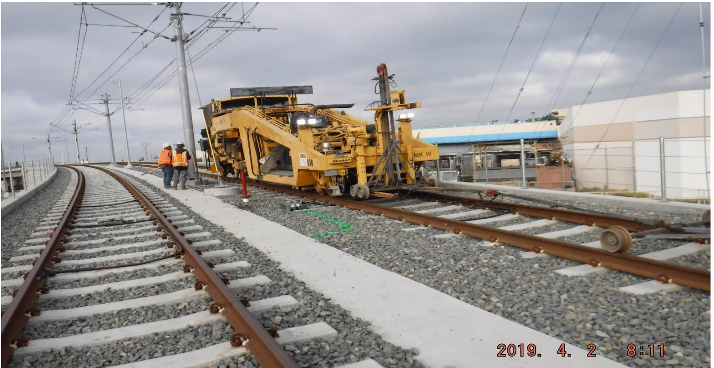
MSE 122 - STA125+64 looking South re-tamp & dress track ballast.
