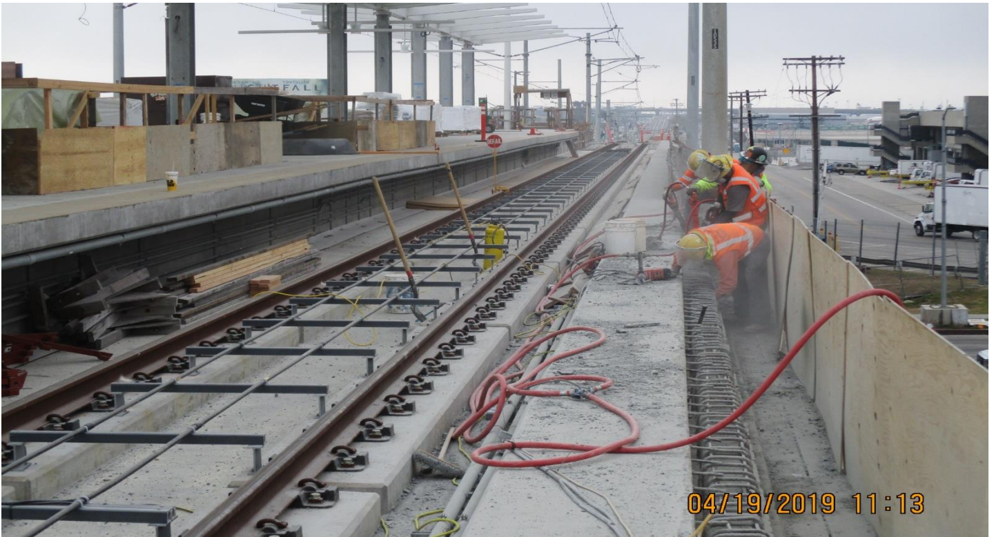
AVIATION/CENTURY- UP chipping of SB track coping slab for U bars.
