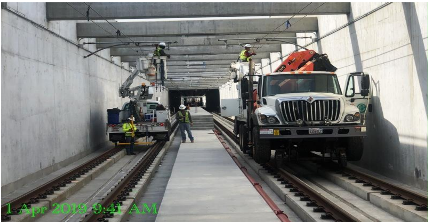
UG-1- LKC lineman continue finalization of WR#07 and WR#08.
