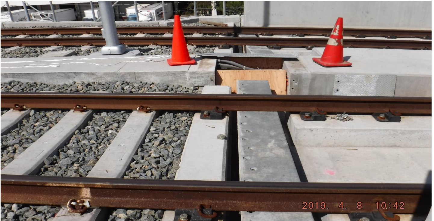
111 th STREET- STA27+03 looking West - Removed bridge joint plates.
