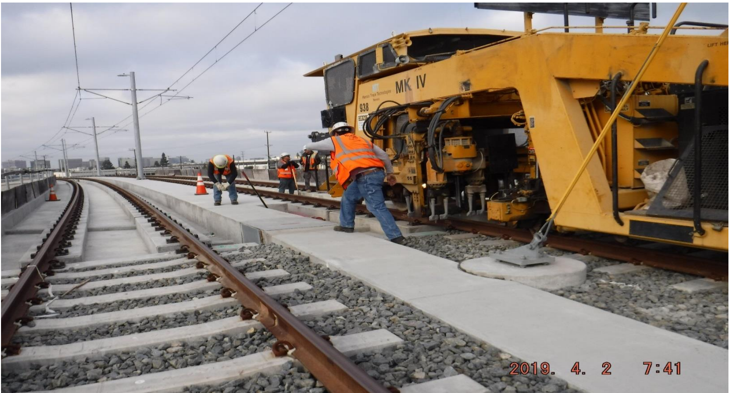
MSE 122 -STA121+50 looking South re-tamp & dress track ballast.
