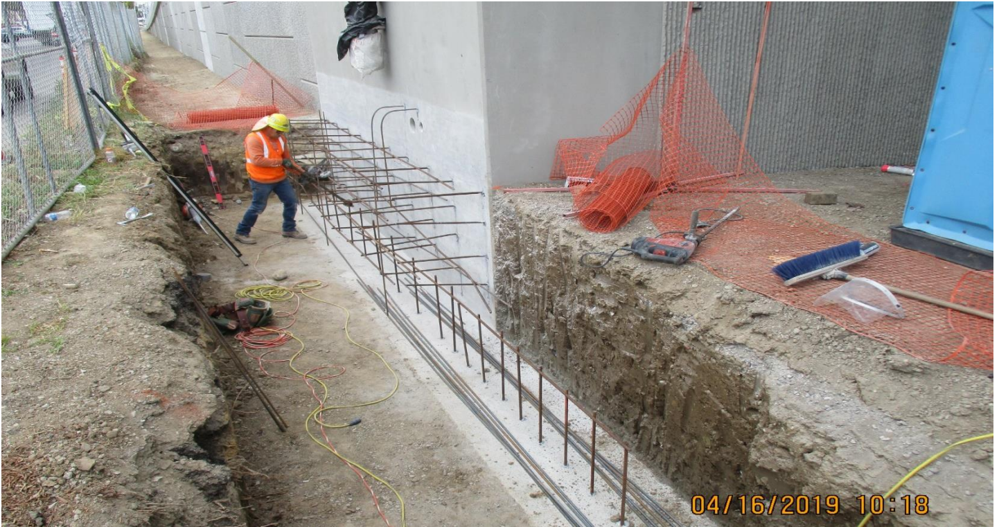
405 BRIDGE - Forming for drainage and COS protection system.
