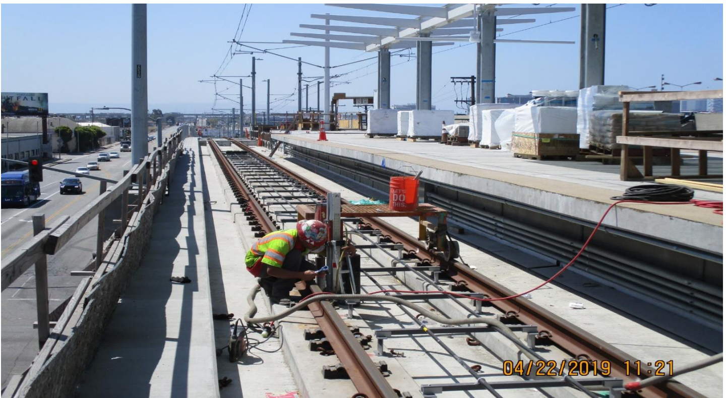
AVIATION/CENTURY- UP coring epoxy insert at NB track STA 68+00 to 70+10.
