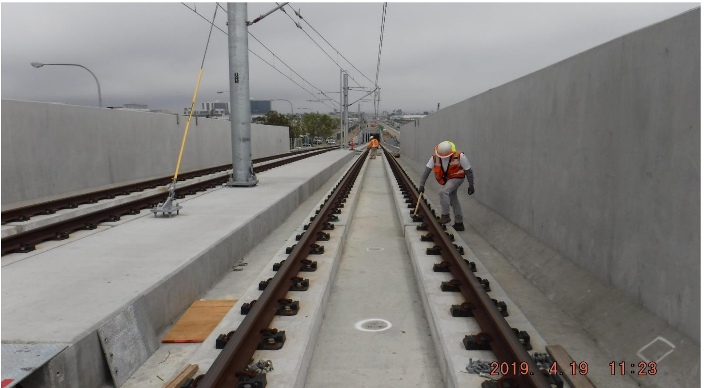
111 th STREET - STA27+00 looking North - adjusting e-clip.
