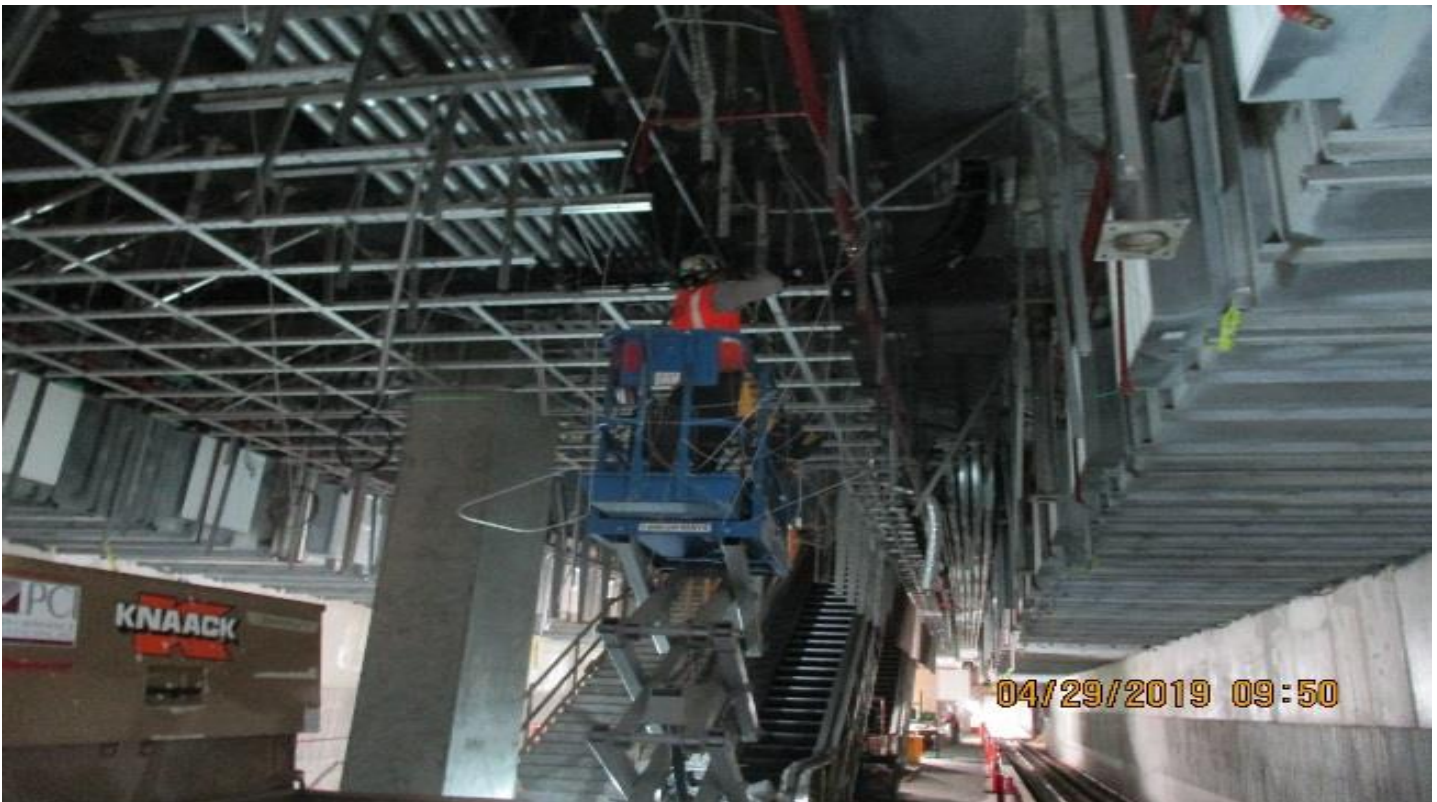
LEIMERT PARK STATION – Installation of metal ceiling grid at the platform.
