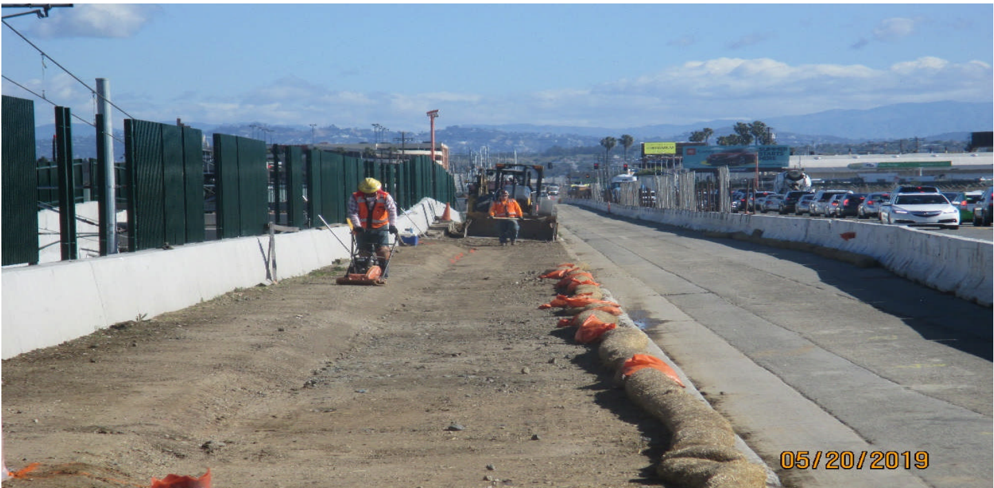
UG1- Compaction of the contour grading at UG-1.
