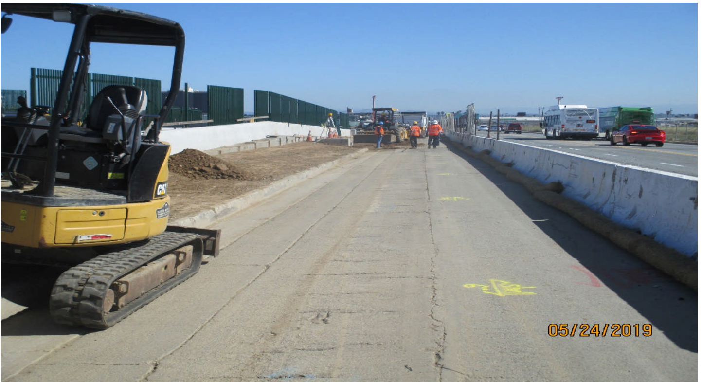
UG-1- Cutting the I beam shoring and backfilling at UG-1.
