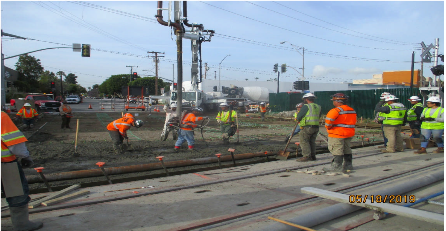
CEDAR STREET- Placing concrete for the Cedar street roadway.
