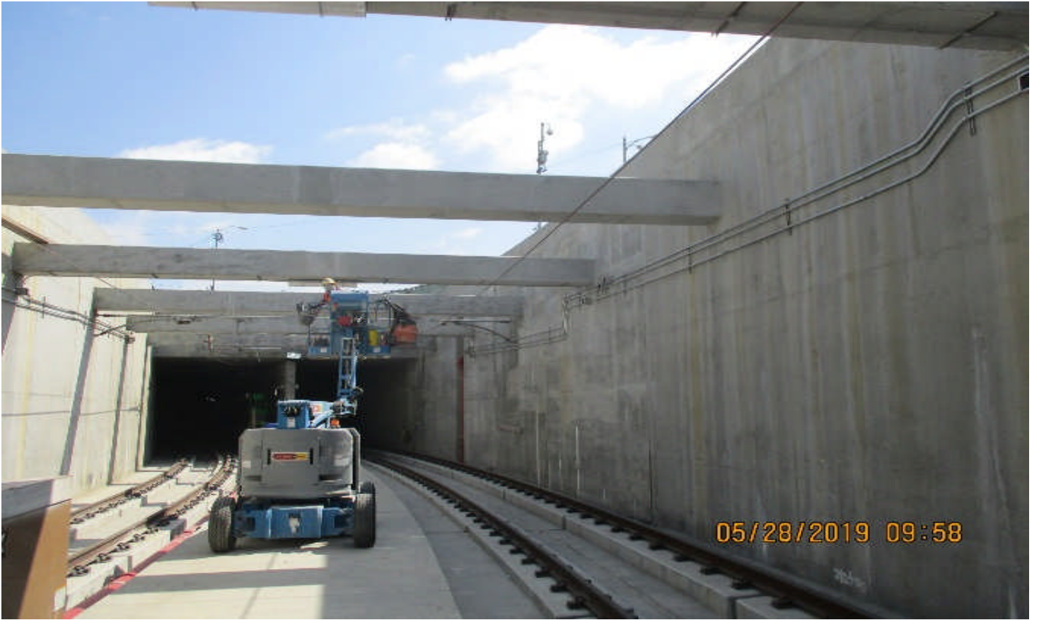
UG3- Grind sack and patch CIP struts at south portal.
