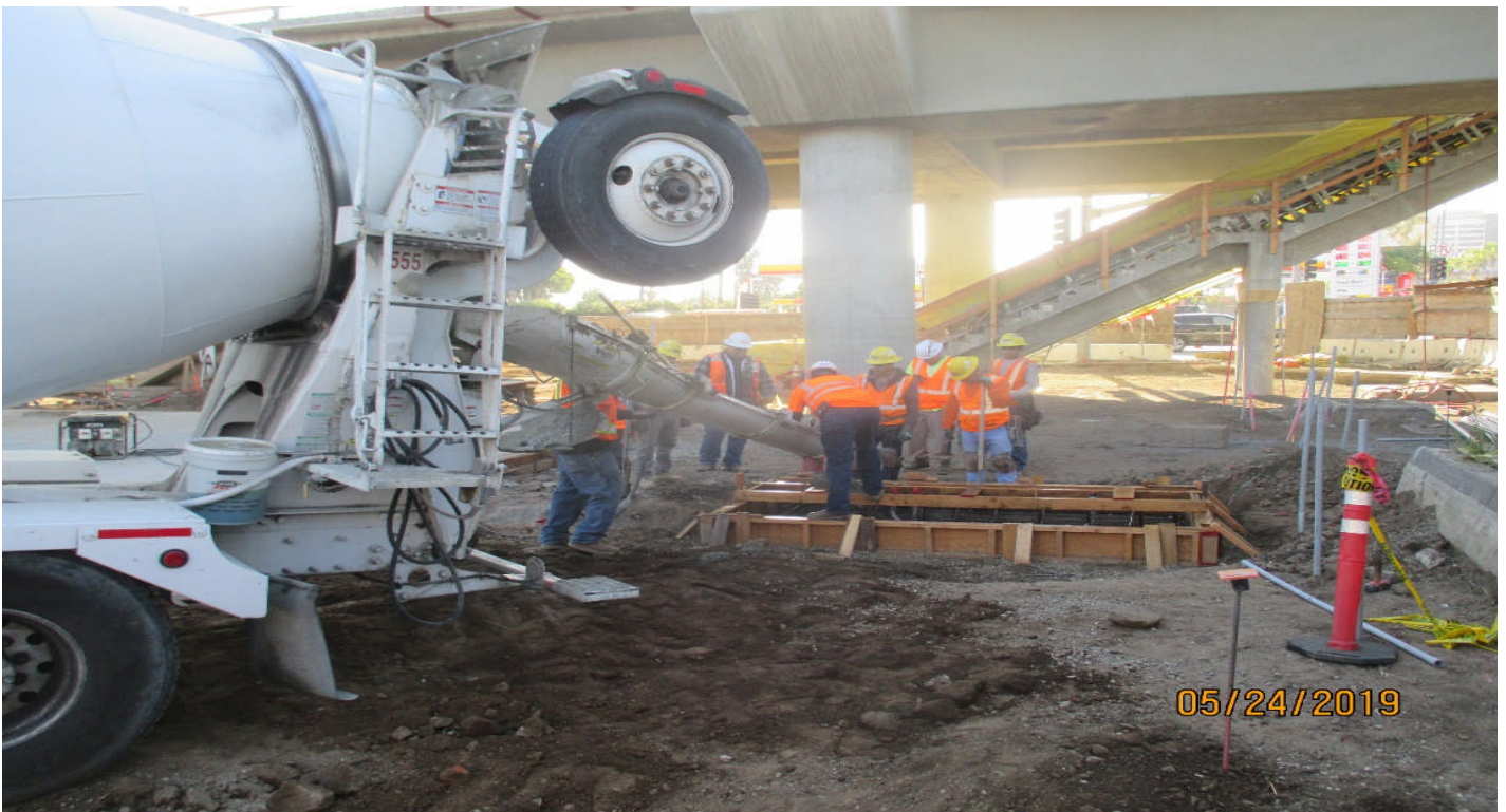
AVIATION/CENTURY- Placing concrete for the map cabinet at the Aviation Station.
