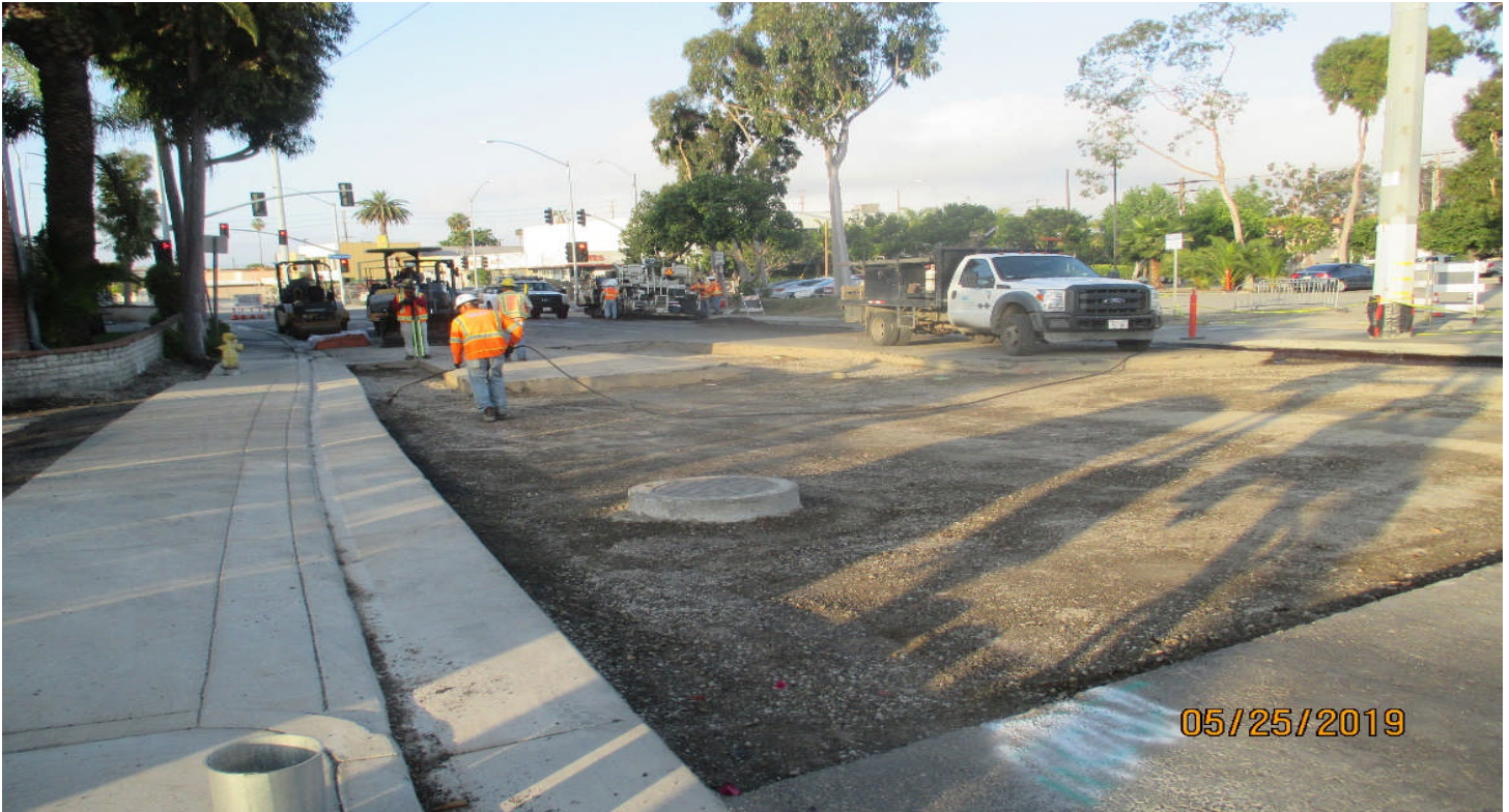
EUCALYPTUS - Applying emulsion tack prior to AC placement on Eucalyptus.
