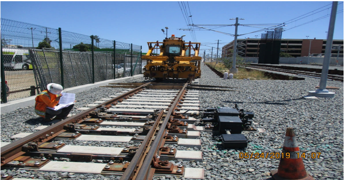
GUIDEWAY at ARBOR VITAE- STA 85+00 to 86+50 - Re-tamping of NB track.
