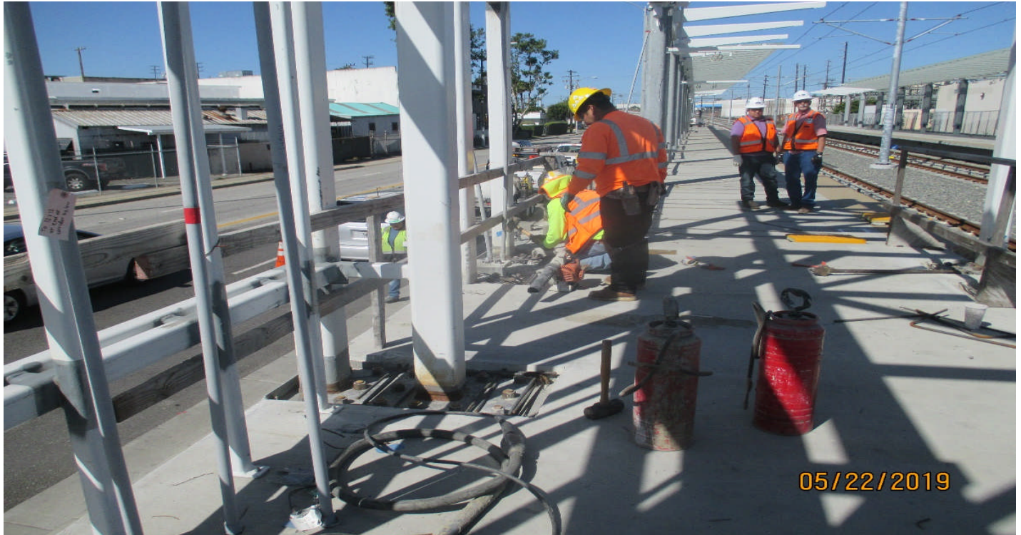
FLORENCE/HINDRY - Hindry Station TVM columns prior to concrete placement.
