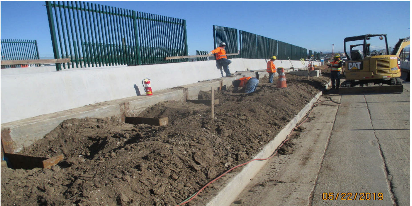
UG-1- Cutting the I beam shoring and backfilling at UG-1.
