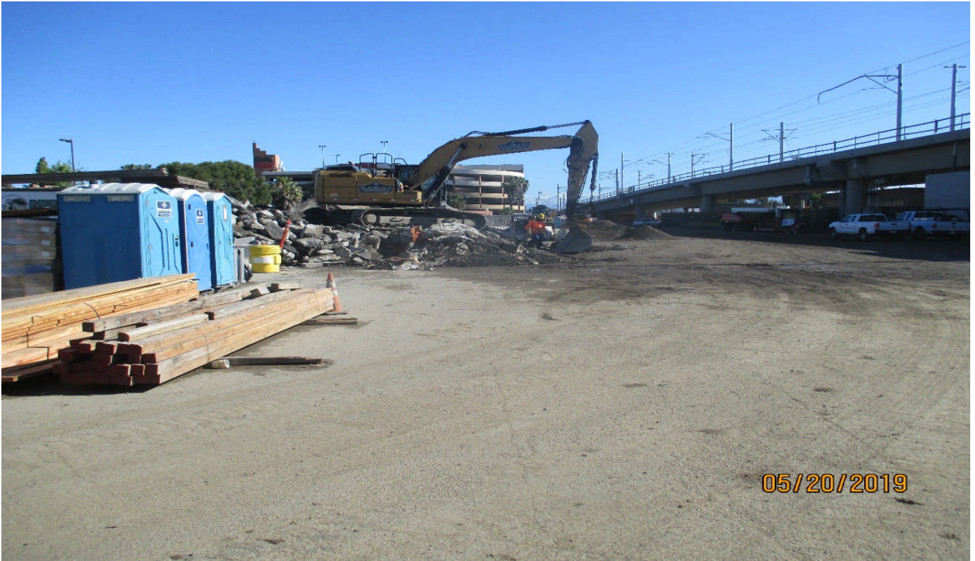
AVIATION/CENTURY- Construction debris demo at the Aviation Station yard.
