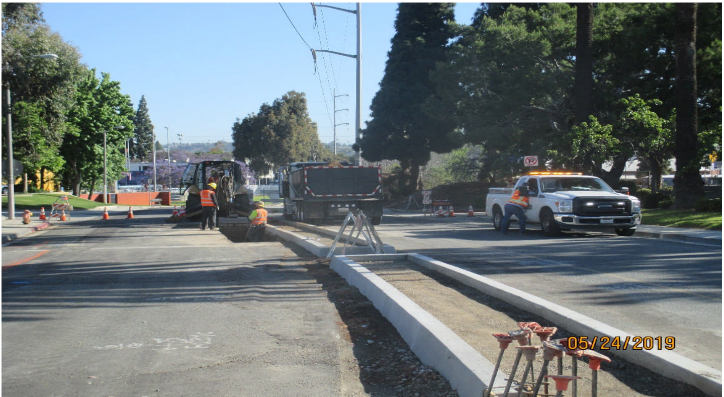
EUCALYPTUS - Over excavation for the median on Eucalyptus.
