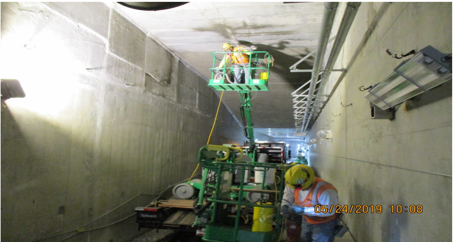
UG3- Guideway at UG3 finishing of cut and cover.
