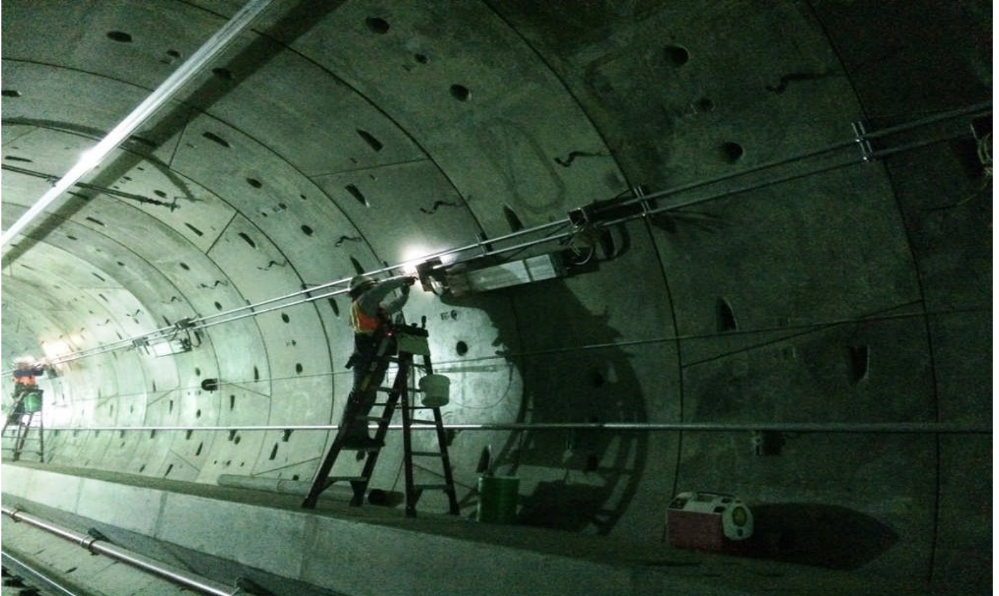
TUNNEL – Installation of emergency lighting at southbound tunnel.
