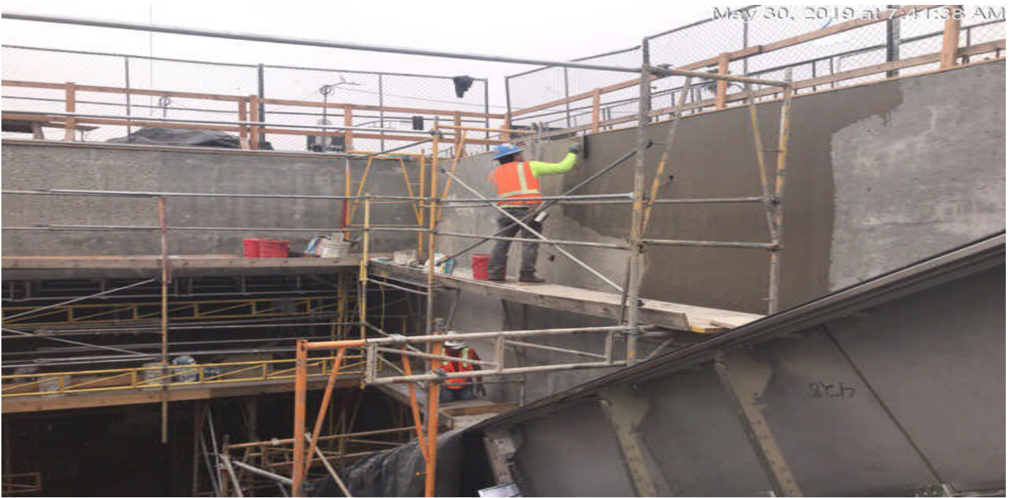
EXPOSITION/CRENSHAW STATION – Installation of skin coat at plaza walls.
