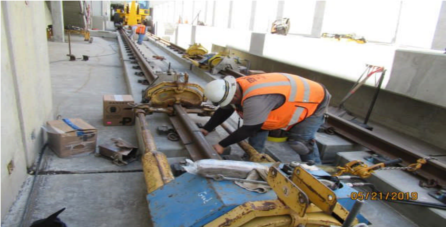
UG1- HCC welder aligning right rail for destress welding on NB.
