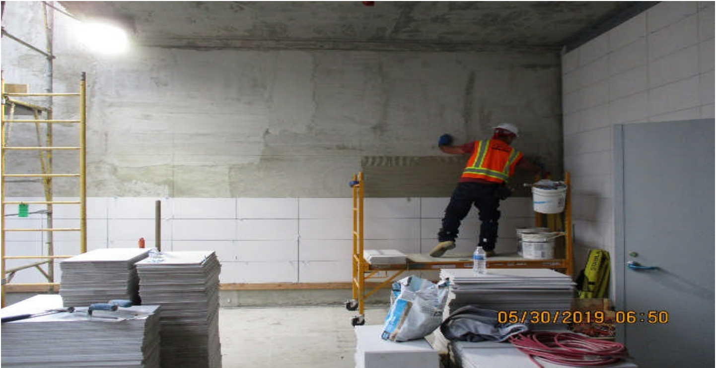
LEIMERT PARK STATION – Installation of ceramic tile at Entrance stairs #1.
